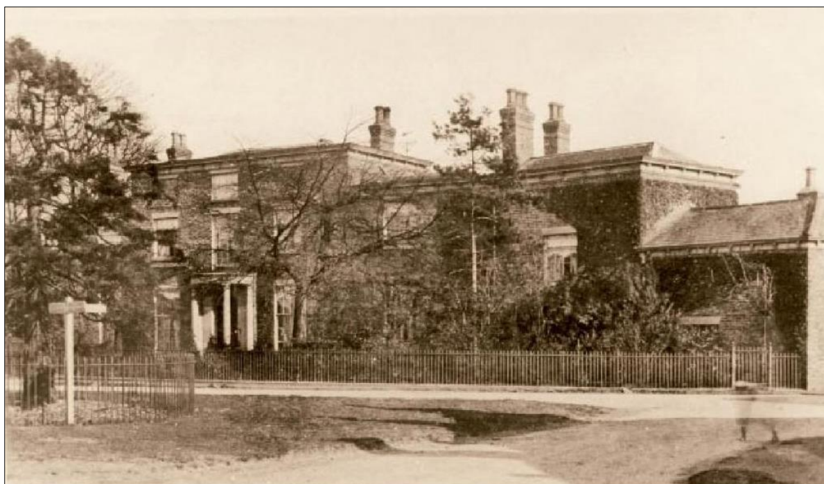
Undated photograph, probably late nineteenth or early twentieth century. Note the shallow pitched roofs over modillion cornices covering the three blocks of the house and the balcony above the main entrance (Chrystal 2015)
