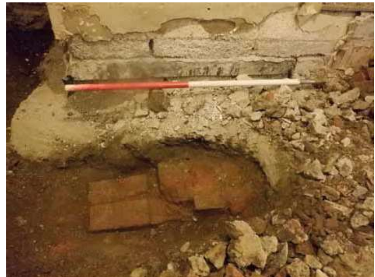
Plate 4. Wall 11, looking north-west
