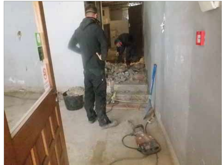
Plate 2. Inside the building, looking north-west
