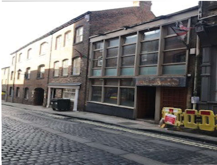
Plate 1. No 9, King Street, looking south-west
