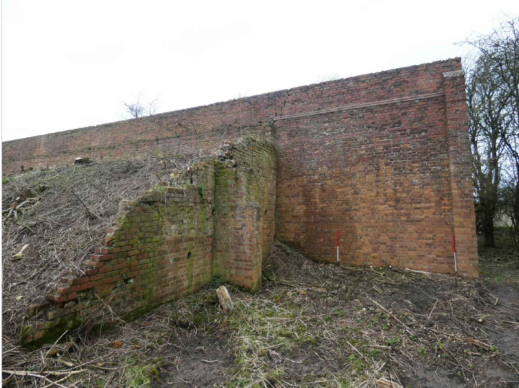
PLATE 35: Machine gun butts, east end showing revetment walls, looking NW (photo 4/748).
