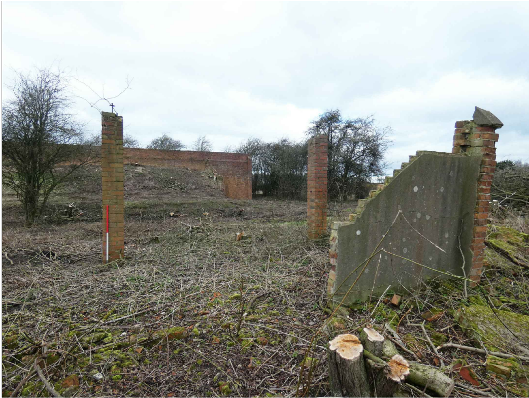
PLATE 40: Machine gun range, showing relationship between firing shed, catch pit and butts, looking NW (photo 4/759).
