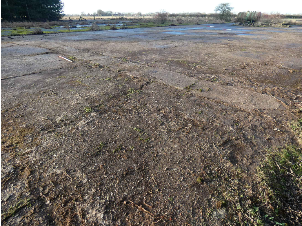
PLATE 7: West runway, area of repair towards north end, looking W (photo 3/515).
