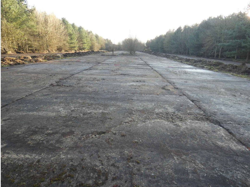
PLATE 13: East runway after vegetation clearance, looking S (photo 3/549).
