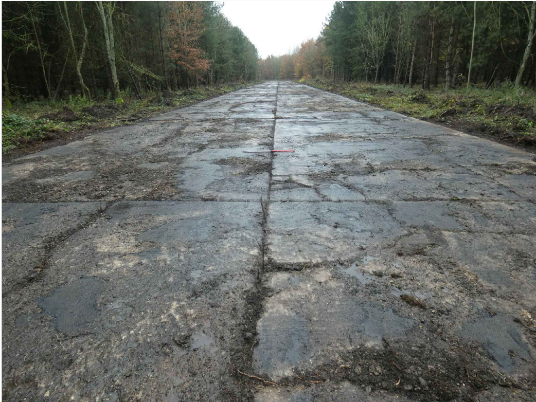
PLATE 16: East taxi-way after vegetation clearance, looking N (photo 2/472).
