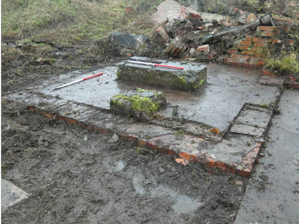
PLATE 25: Bulk petrol installation, south pump house after clearance and excavation, looking SW (photo 1/451).
