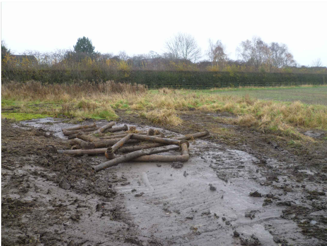
PLATE 22: Bulk petrol installation, ex situ sections of cast-iron pipes, looking S.
