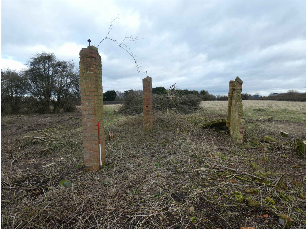
PLATE 39: Machine gun range, remains of firing shed with south wall and pillars to north wall, looking NE (photo 4/758).
