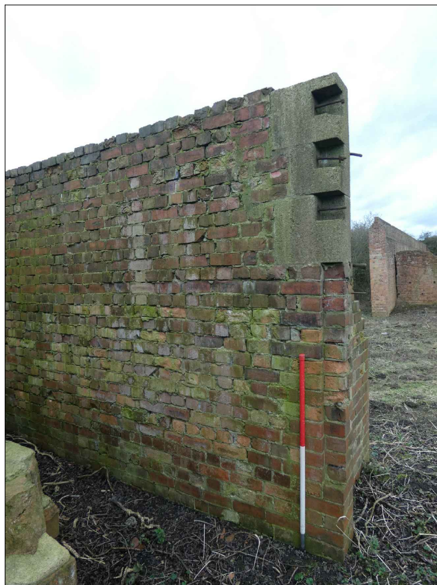
PLATE 30: Cannon butts, detail of wall end to easternmost bay showing rebates and concrete blocks, looking E (photo 4/789).
