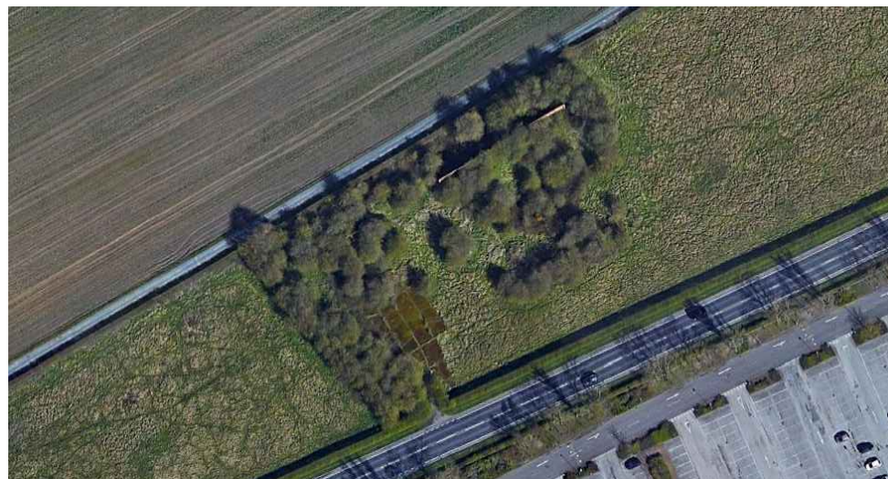
F) Clifton Moor canon butts and machine gun range (source: Google Earth aerial photograph, August 2015).
