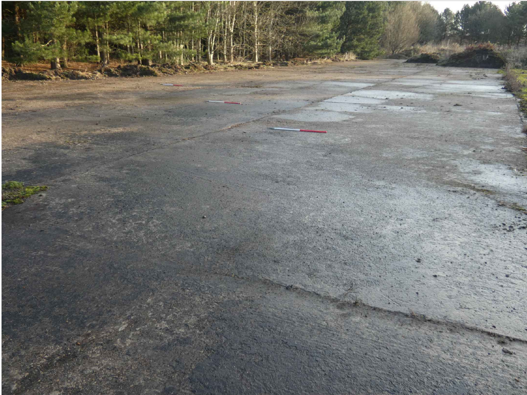
PLATE 6: West runway after vegetation clearance, looking E (photo 3/505).
