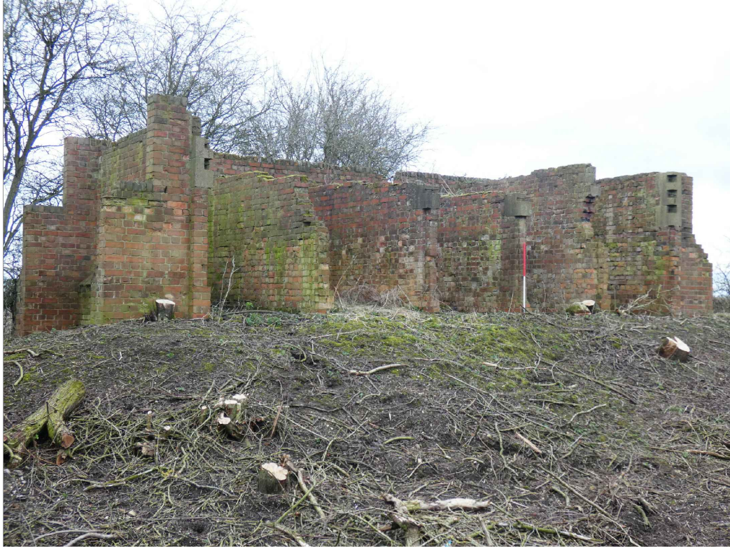
PLATE 29: Cannon butts, front (south) elevation, looking NE (photo 4/782).
