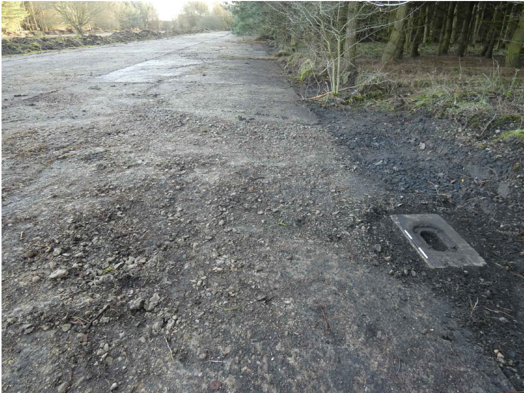
PLATE 14: East runway, excavated landing light on west side, looking S (photo 3/541).
