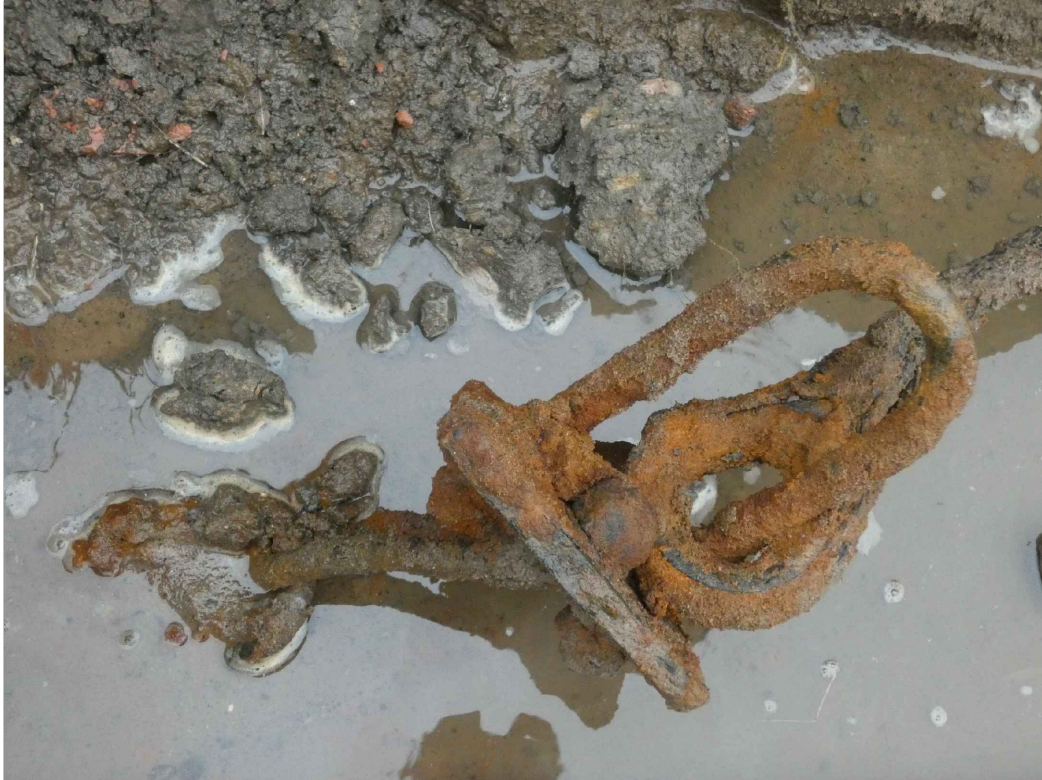
PLATE 21: Bulk petrol installation, mound A, detail of steel cable anchor, looking S (photo 1/440).
