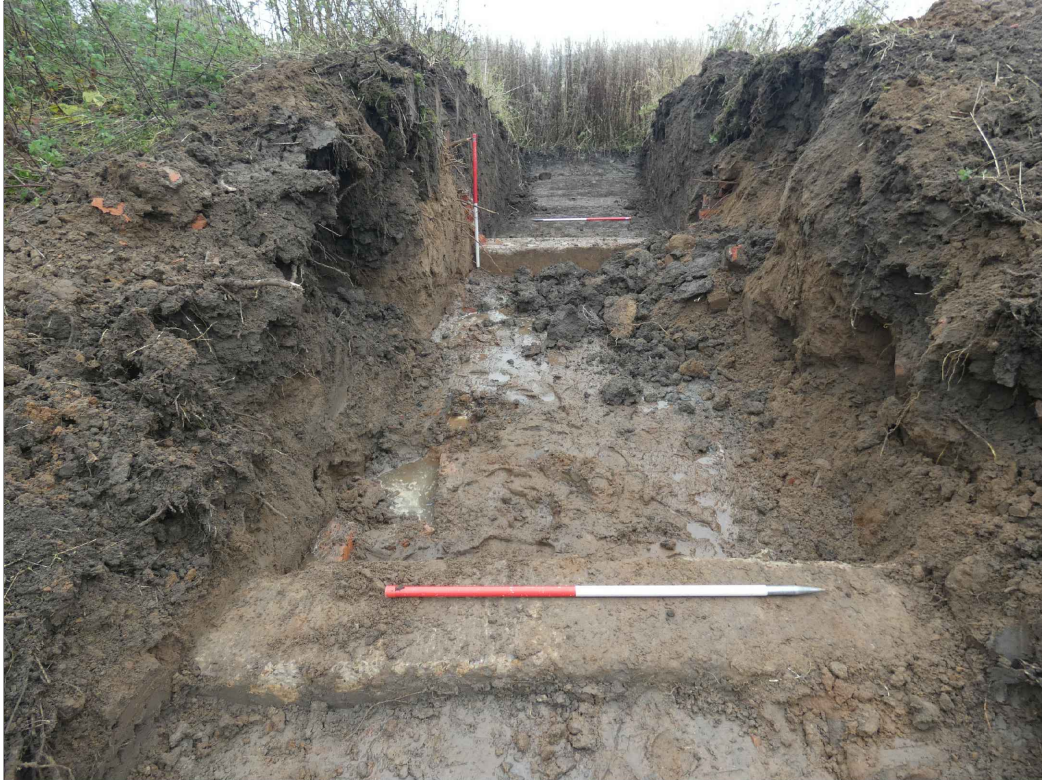
PLATE 23: Bulk petrol installation, mound B after excavation, showing walls of internal chamber, looking W (photo 1/411).
