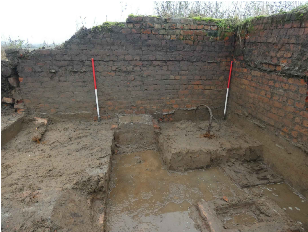
PLATE 20: Bulk petrol installation, mound A after excavation, showing brick walls and piers, with one anchor point, looking N (photo 1/435).
