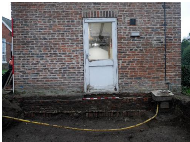
Figure 10: The exposed foundations of the late 18 th century range comprised of a single course of bricks laid in rowlock, bonded with clay straight onto the ground. Above this row are six courses of brick laid in stretcher, bonded with light brown mortar.
