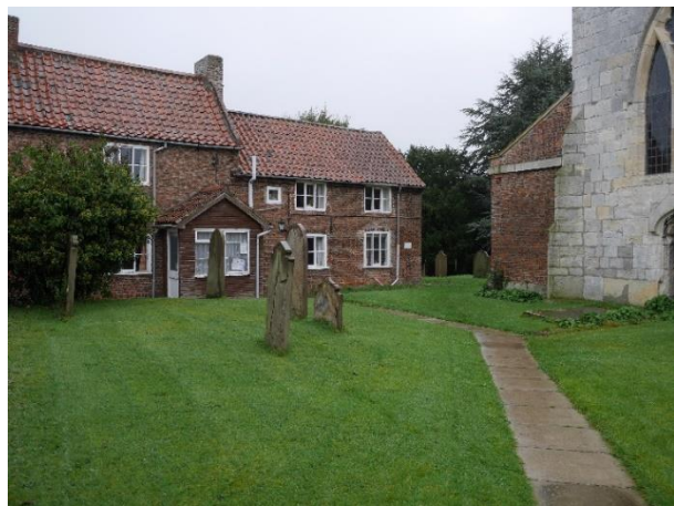
Figure 8: Front aspect of Church Cottage and proximity to St Helen's Church.
