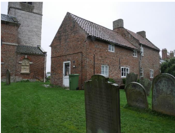
Figure 7: Rear aspect of Church Cottage and its position with St Helen's Churchyard.
