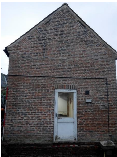
Figure 9: Tumbled brick gable detail as seen on the east facing elevation of the late 18th century range.
