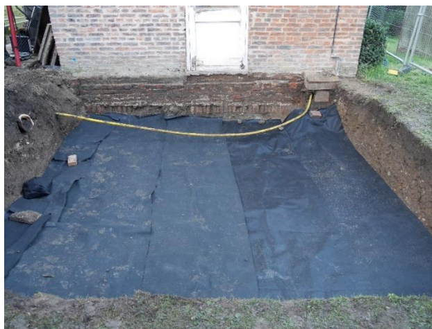
Figure 6: Excavation area sealed with the polypropylene fabric
