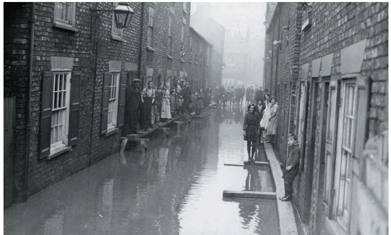
Plate 6 Flooding in Lower Wesley Place, Hungate, 23rd February 1933
