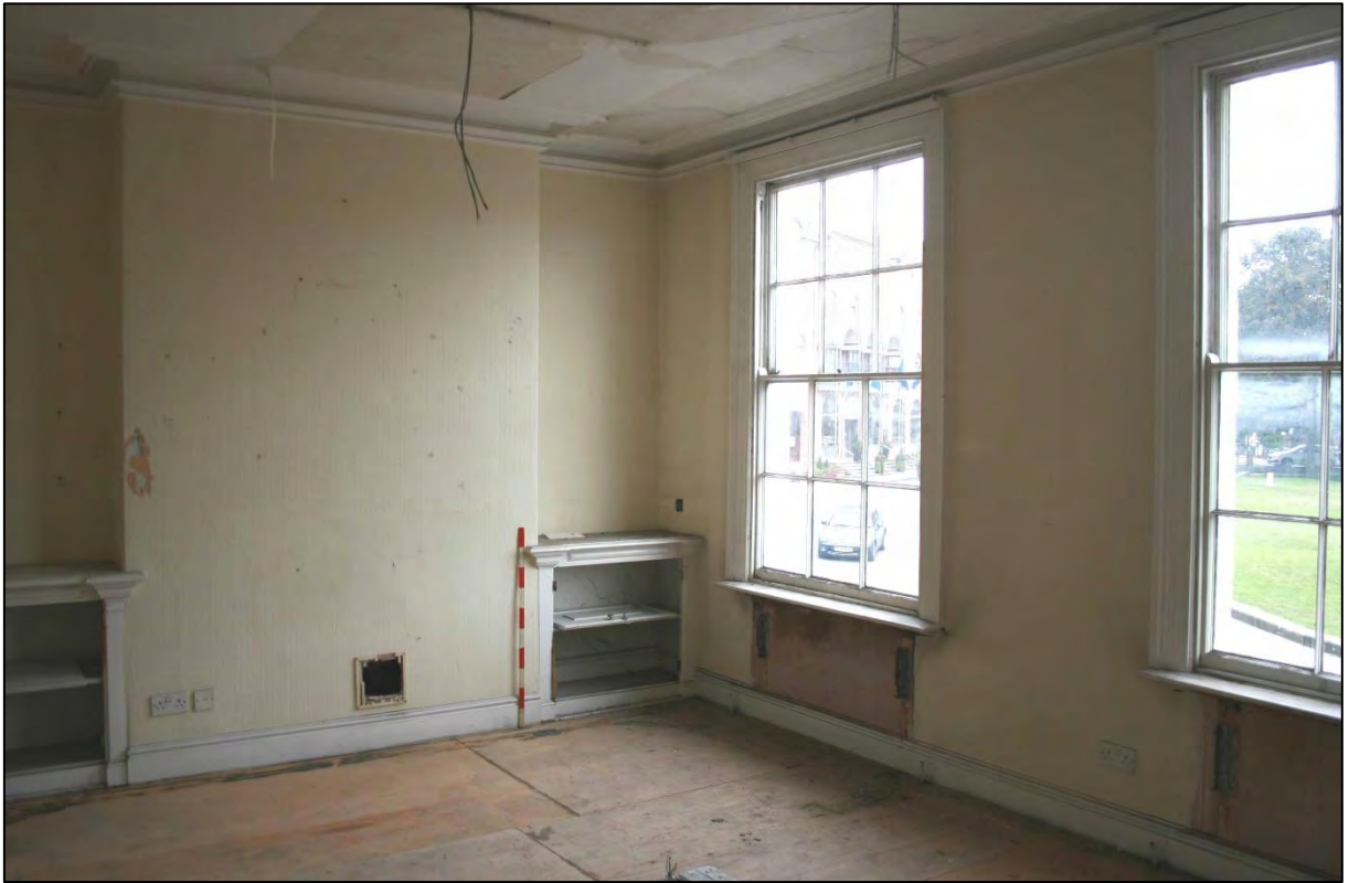
Plate 43. Room F8, looking northeast.
