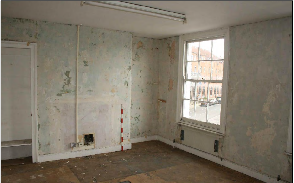
Plate 55. Room S11, looking northeast.
