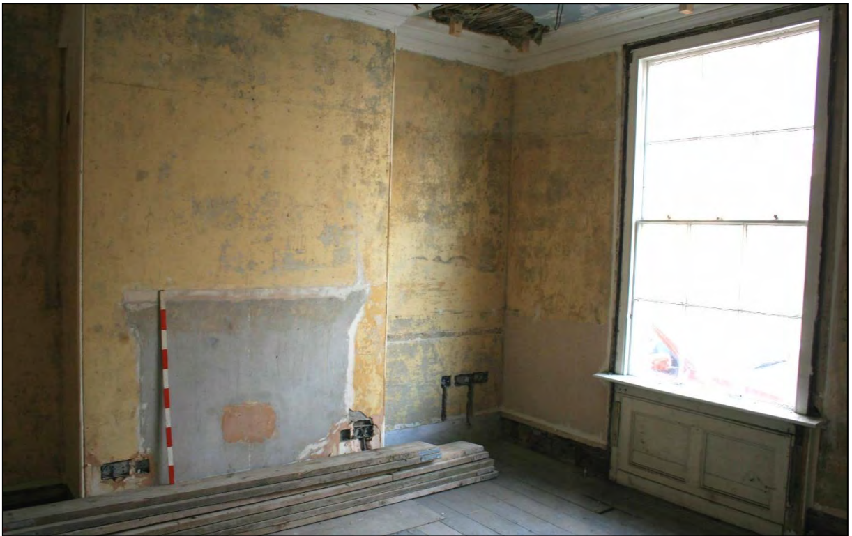
Plate 15. Room G1, looking northwest.
