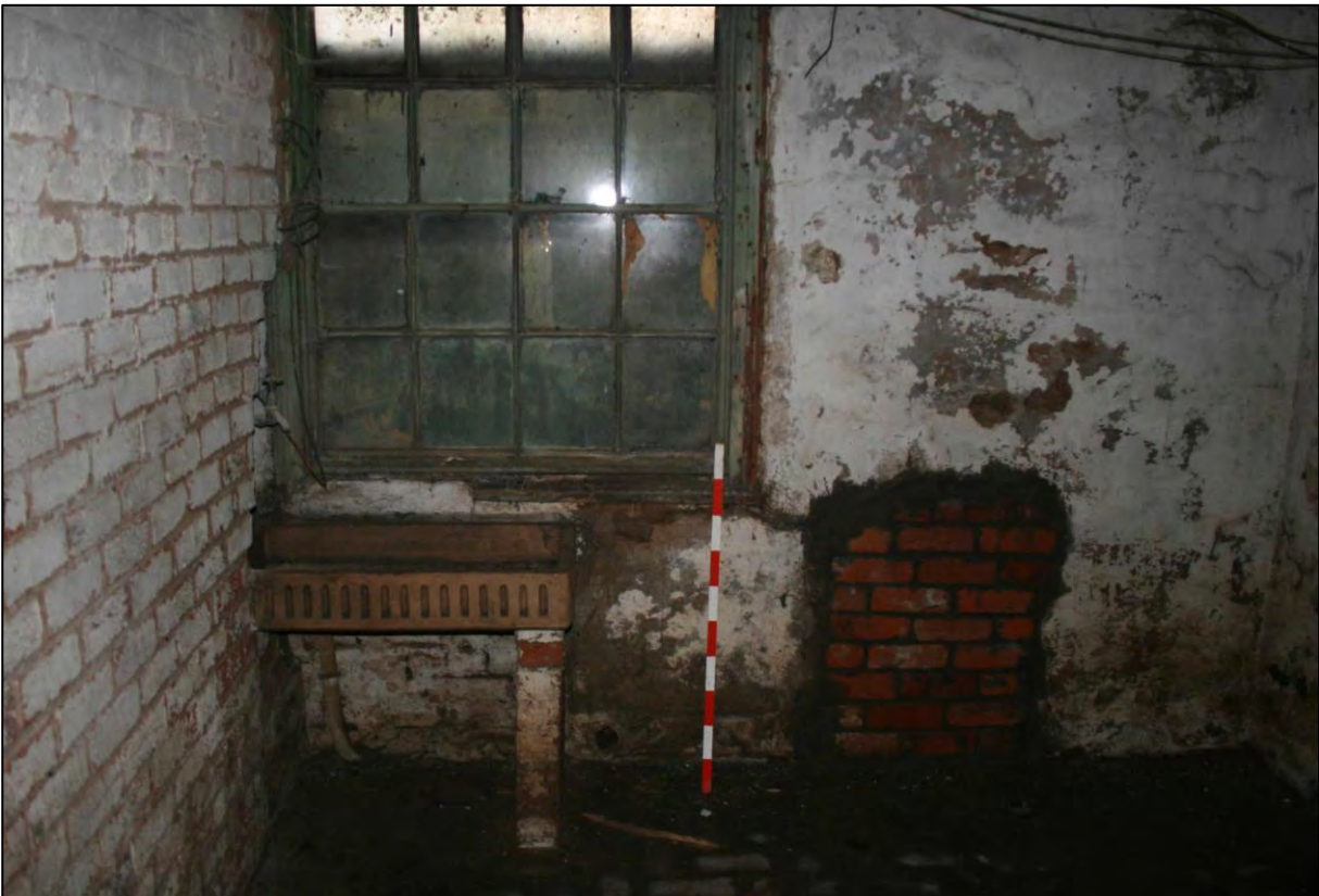
Plate 10. Room B2, window and sink, looking north.
