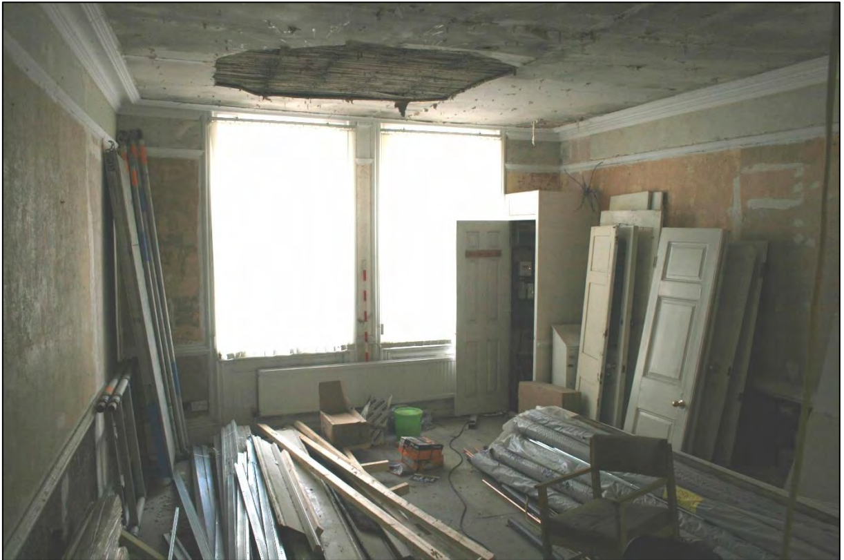
Plate 20. Room G6, looking east.
