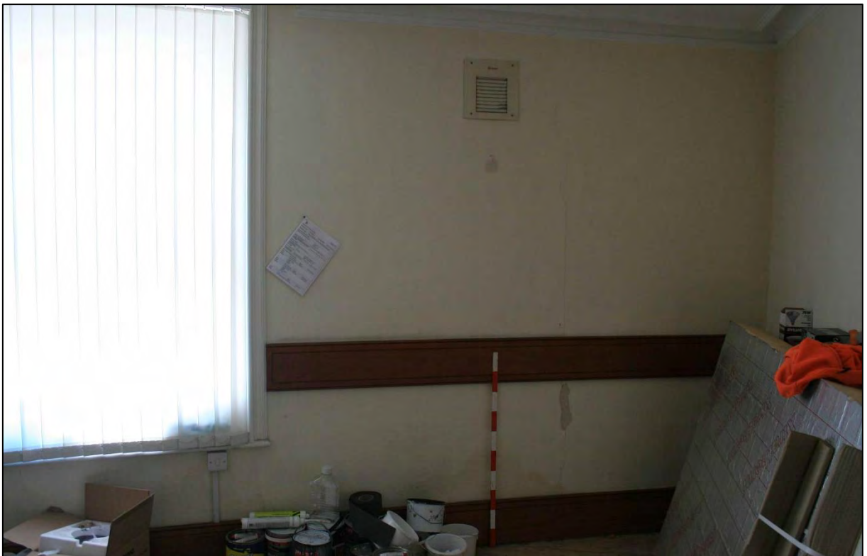
Plate 18. Room G4, looking east.
