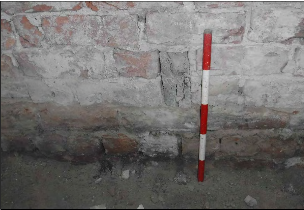
Plate 31. Room G9, example of floor joist.
