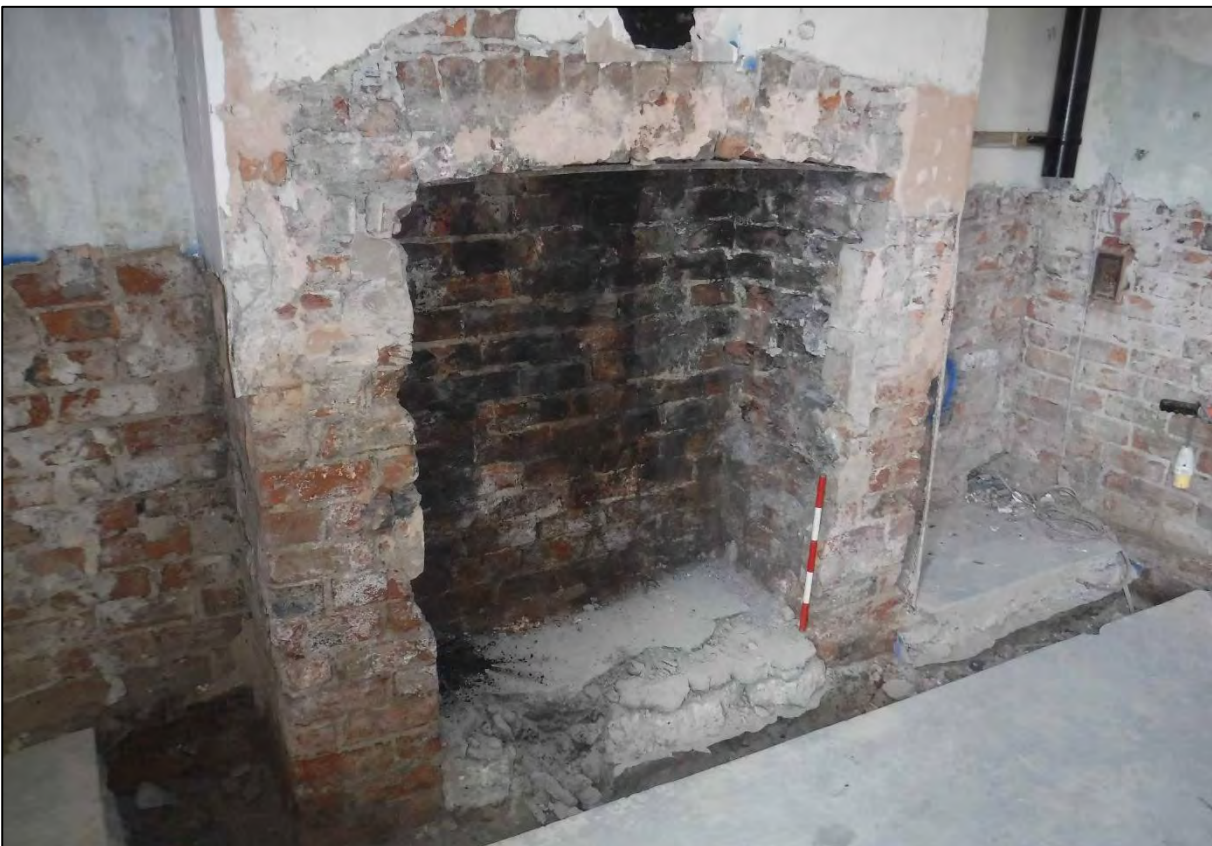
Plate 28. Room G9, fireplace.
