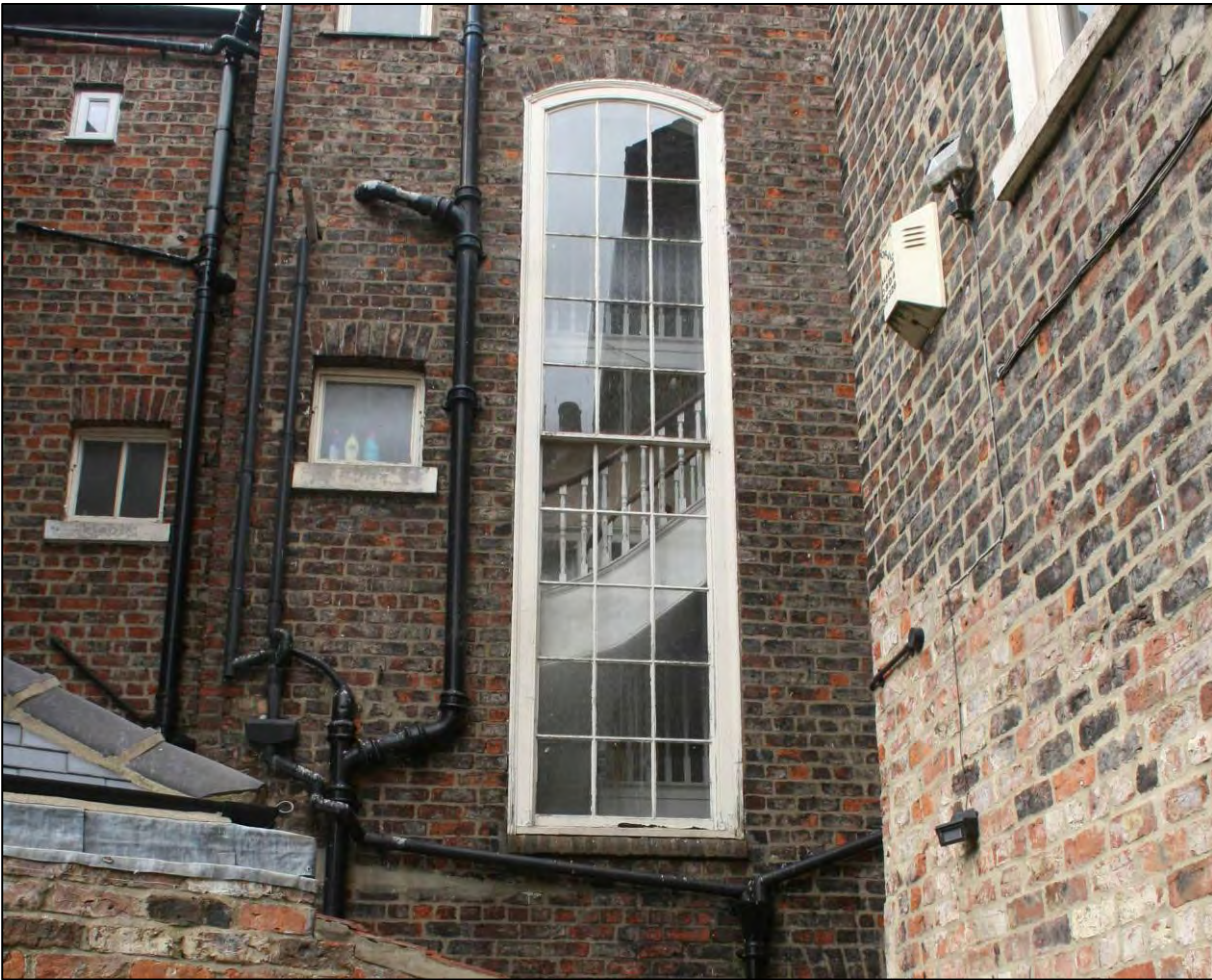
Plate 38. External view of stair tower window.
