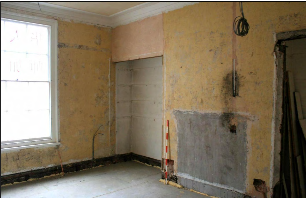
Plate 34. Room F2, looking northeast.
