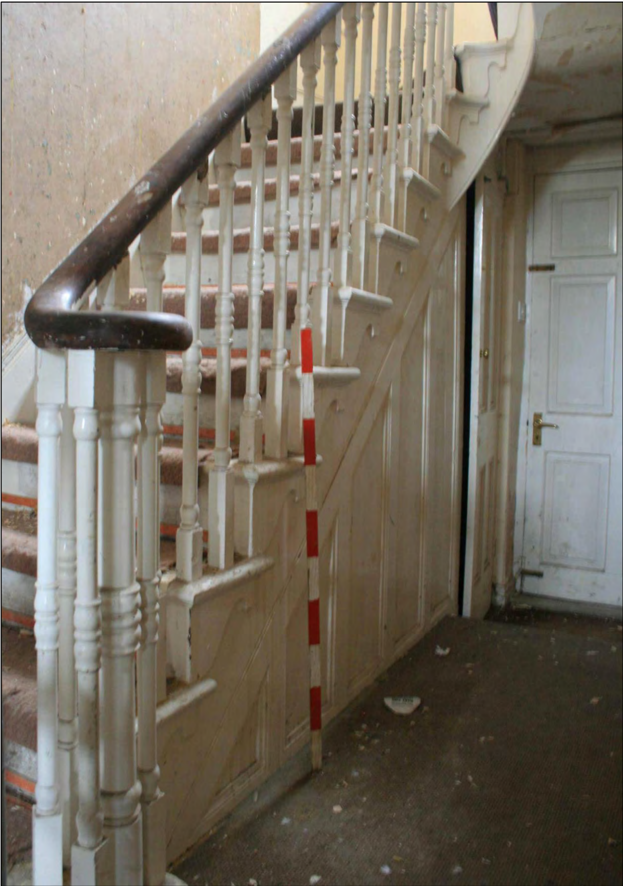
Plate 25. Room G8, stairs.
