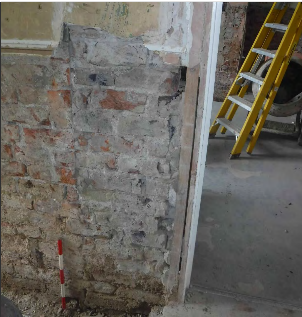
Plate 32. Repositioned doorway between Rooms G8 and G9.
