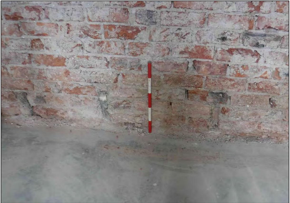
Plate 24. Room G7, floor joists in west wall.
