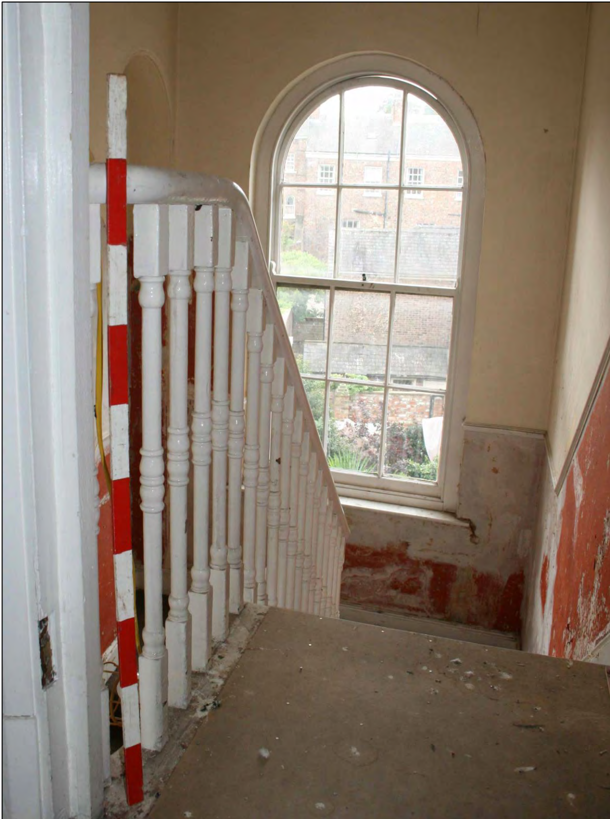
Plate 56. Room S12, stairs.
