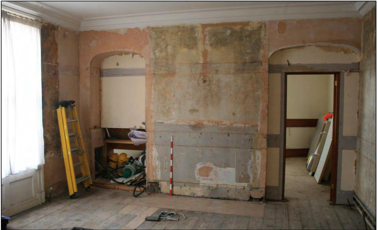
Plate 17. Room G3, looking east.
