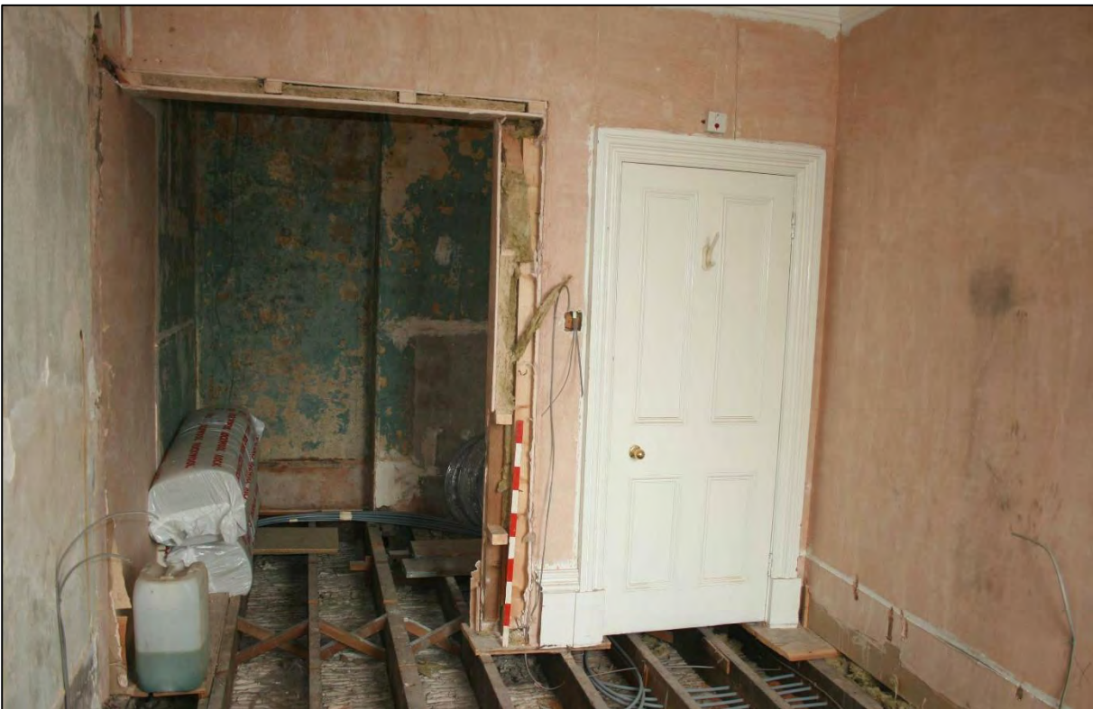
Plate 39. Stud wall dividing Rooms F6 and F7, looking west.
