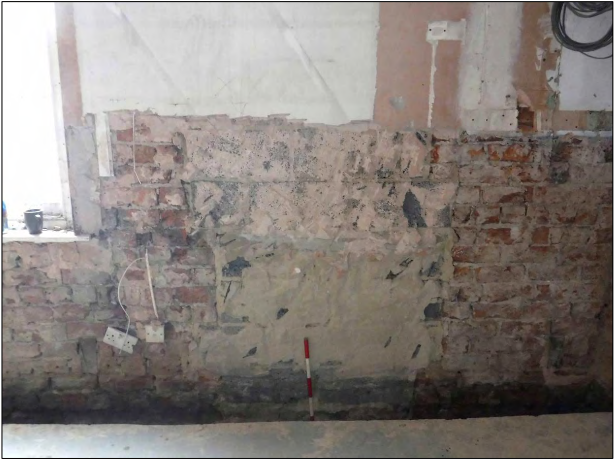
Plate 29. Room G9, blocked doorway in west wall.
