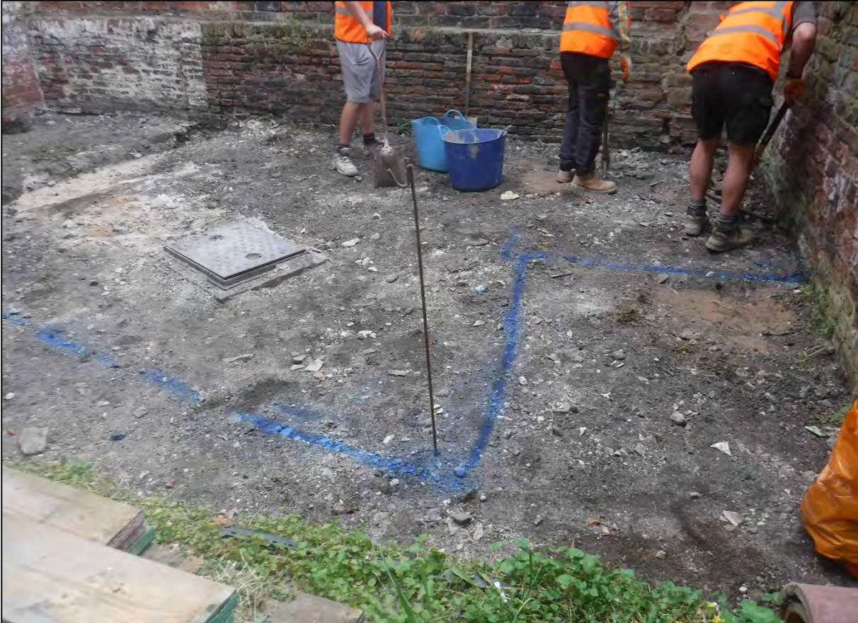
Plate 1. General view of excavation area following removal of yard surface concrete.
