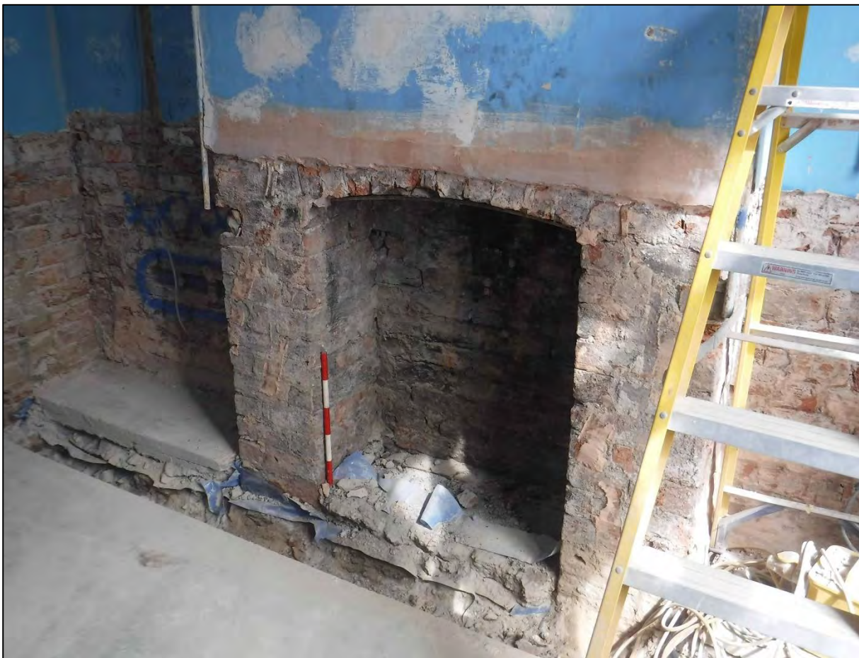
Plate 23. Room G7, fireplace.
