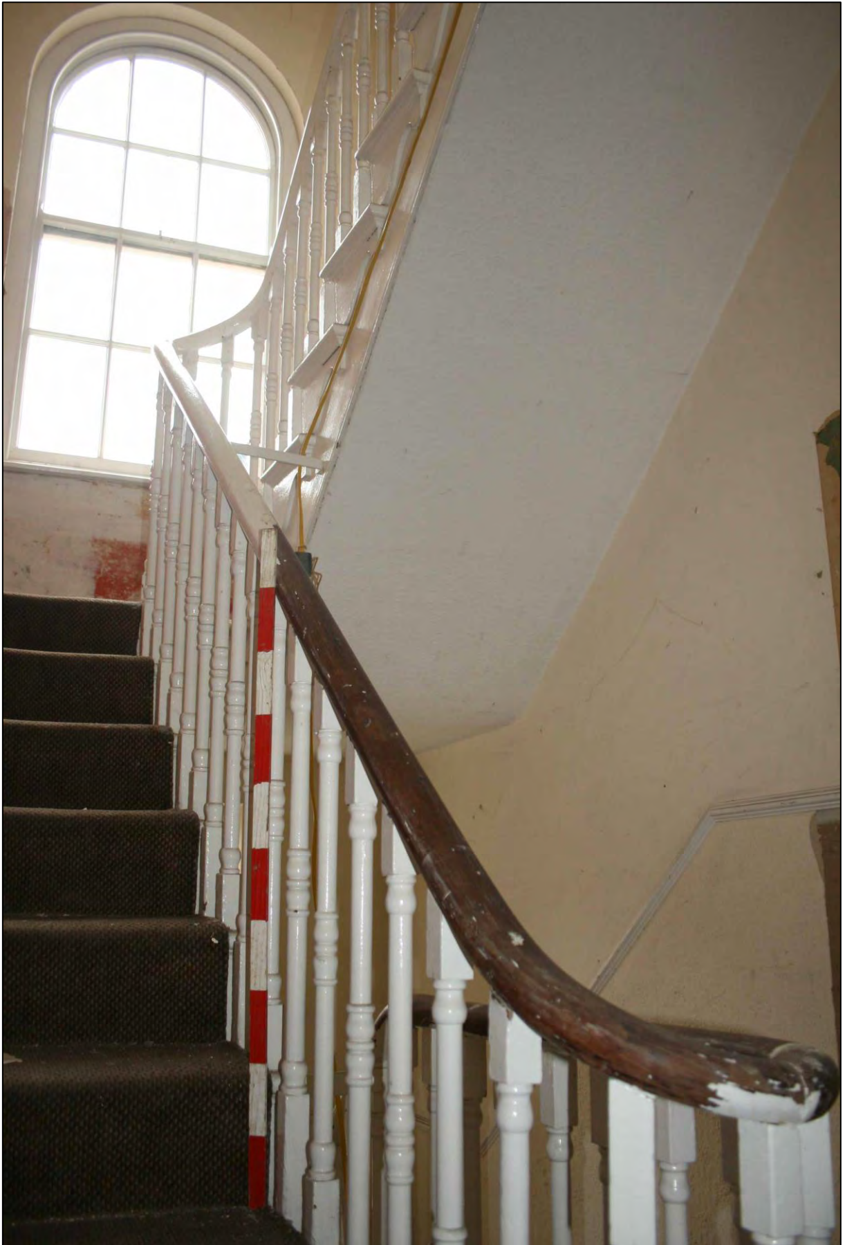
Plate 49. Room F11, stairs, looking south.
