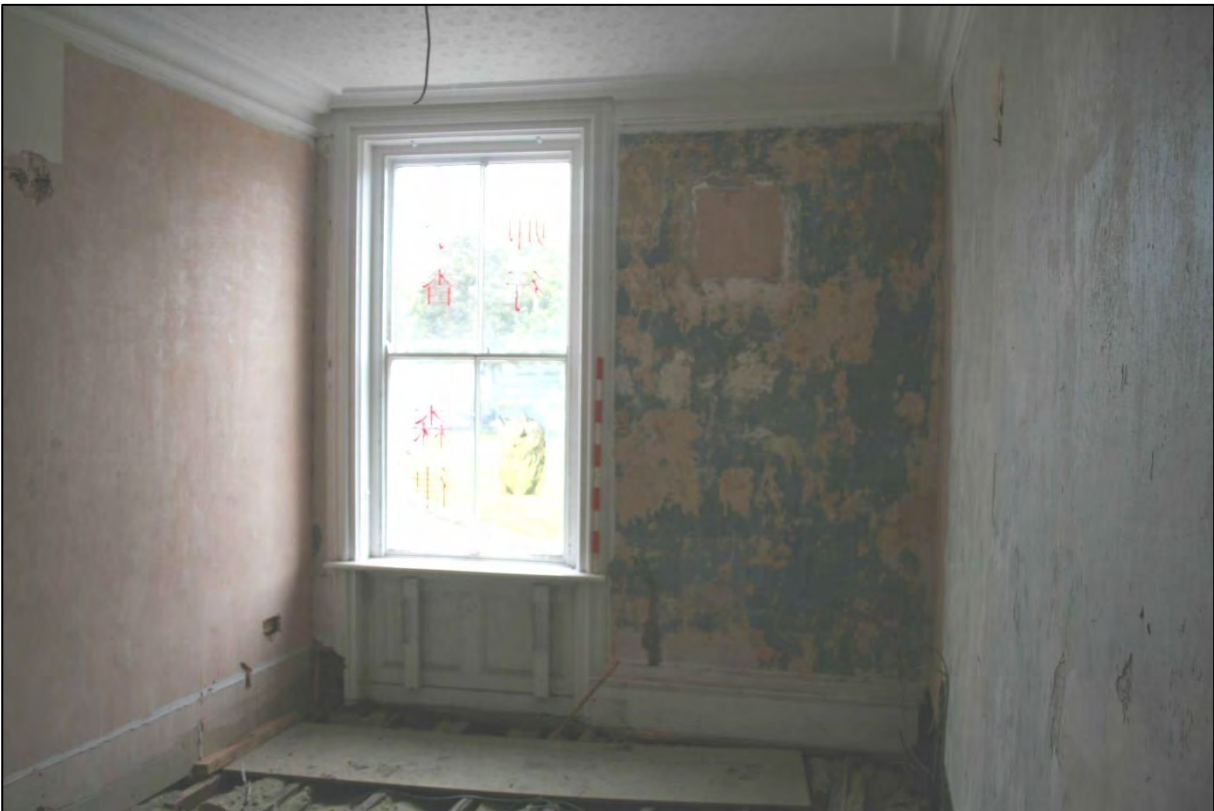
Plate 42. Room F7, looking east.
