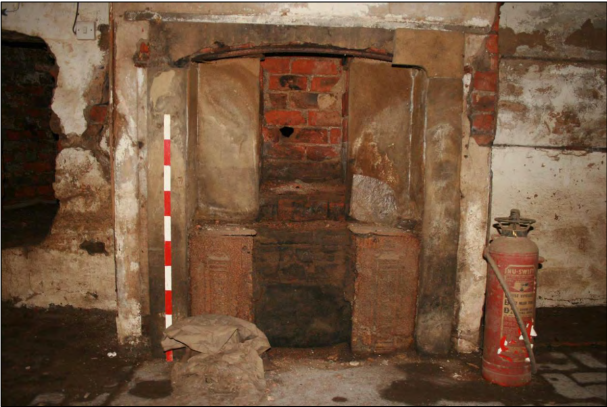
Plate 9. Room B2, grange.
