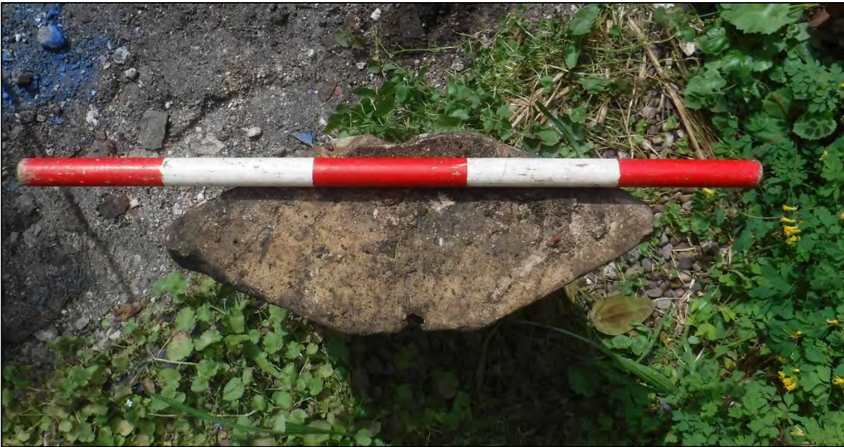
Plate 5. Example of window mullion profile.
