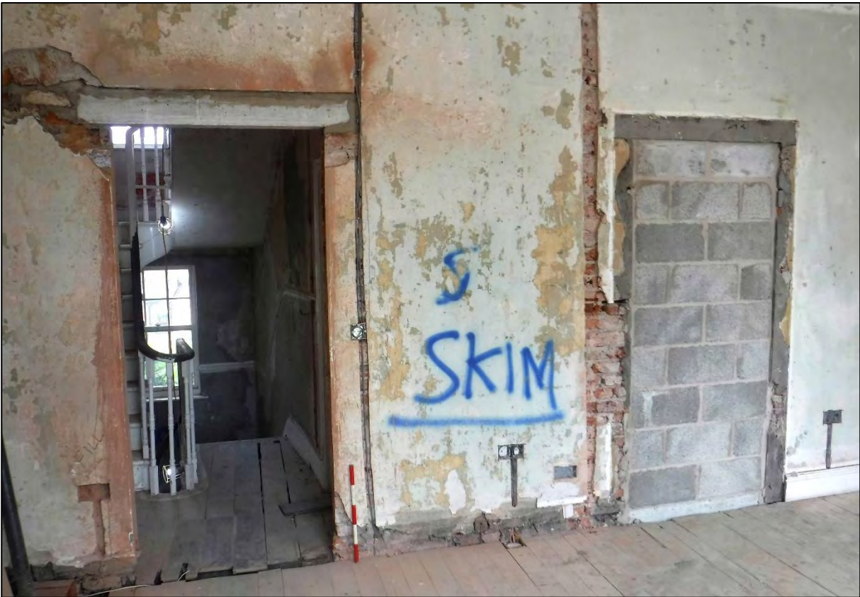
Plate 45. Room F8, blocked and new doorway.
