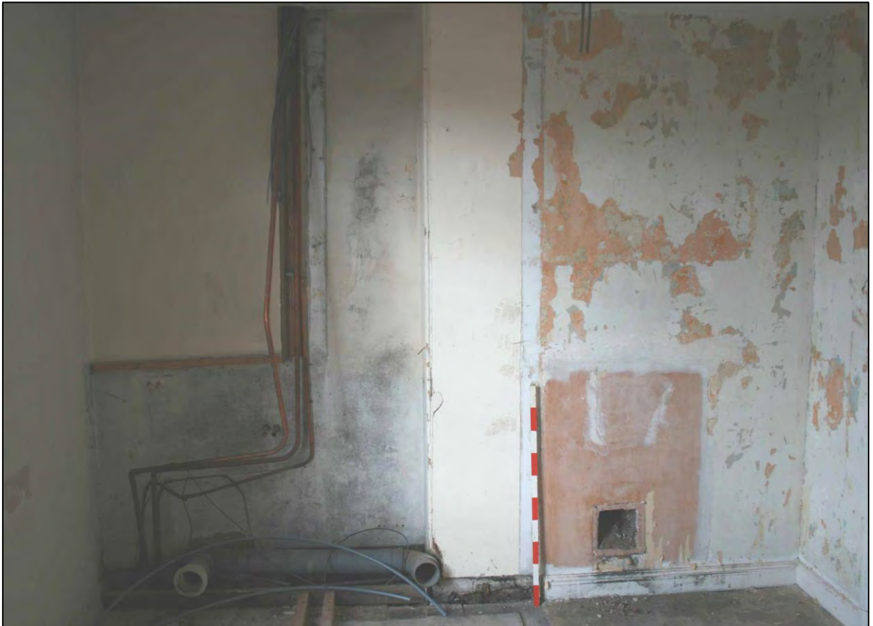
Plate 53. Room S9, location of chimney breast.
