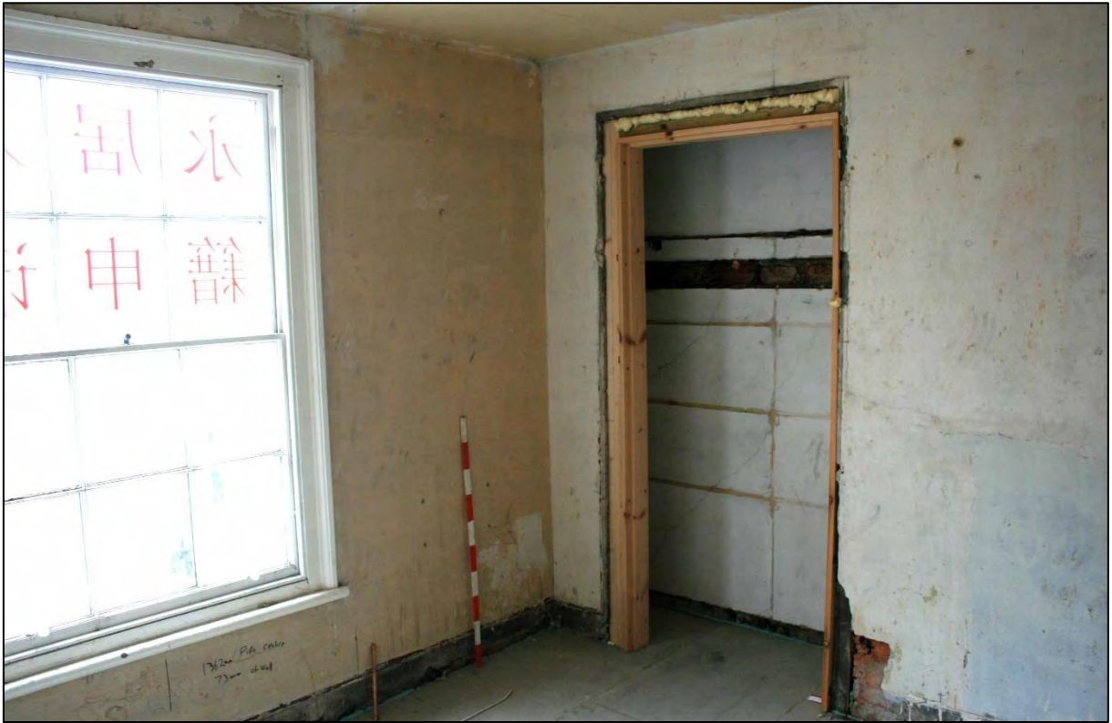
Plate 50. Room S3, example of 20 th century office.
