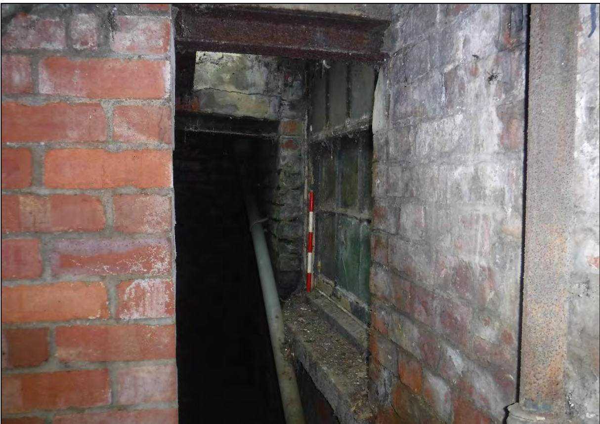
Plate 14. External view Room B2 window.
