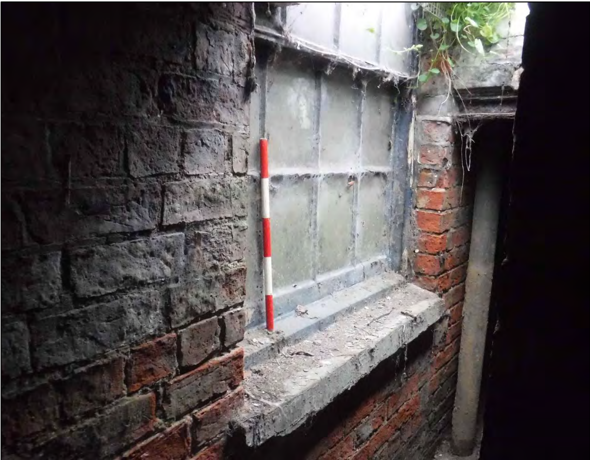
Plate 13. External view Room B1 window.
