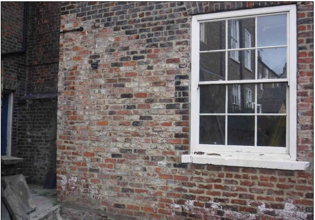
Plate 30. External view of Room G9 rebuilt west wall.
