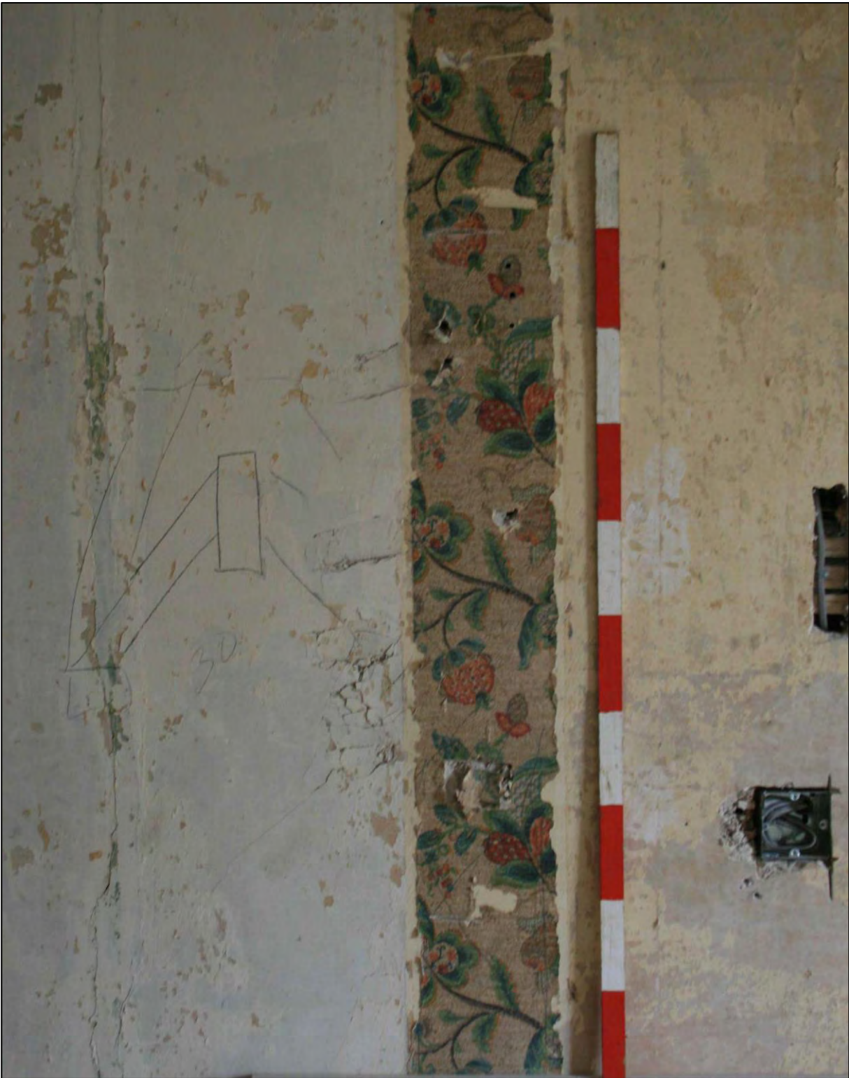
Plate 52. Rooms S7 and S8, wallpaper revealed by removing stud wall.
