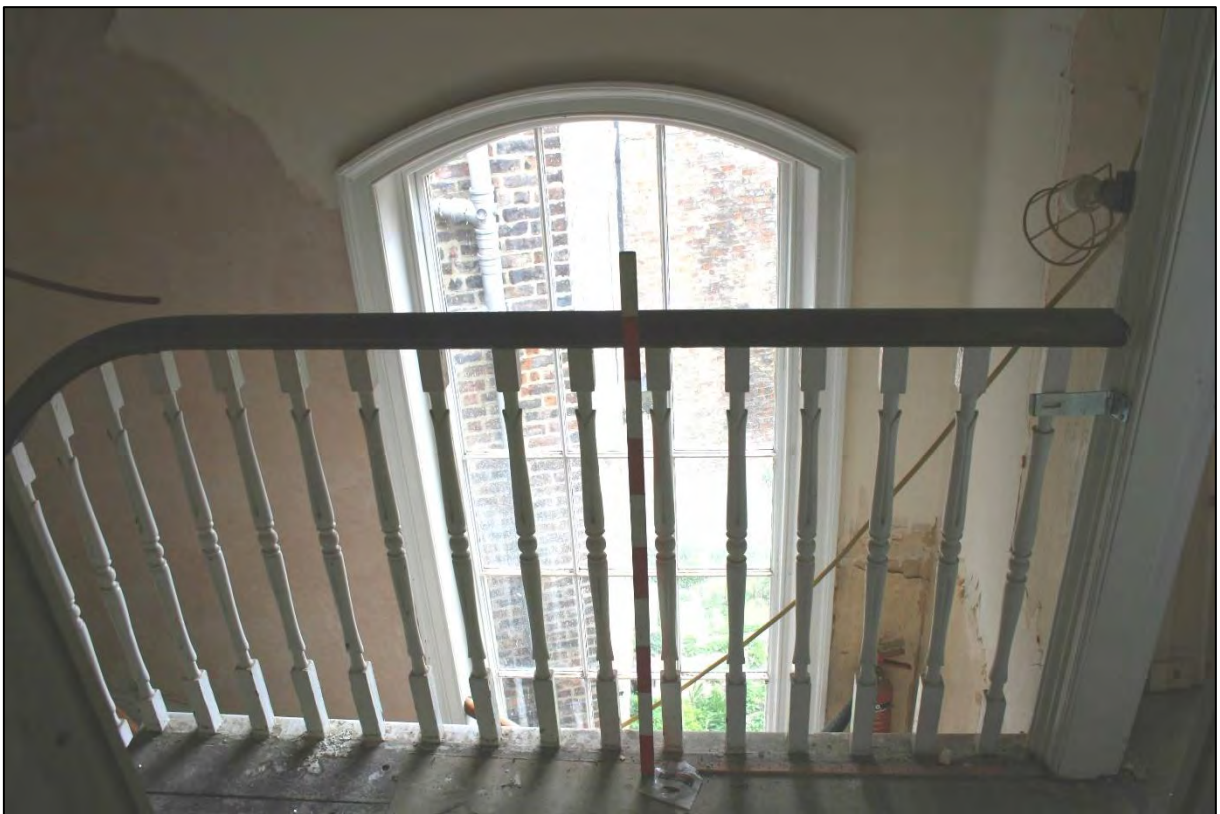
Plate 51. Room S6, banister and window.
