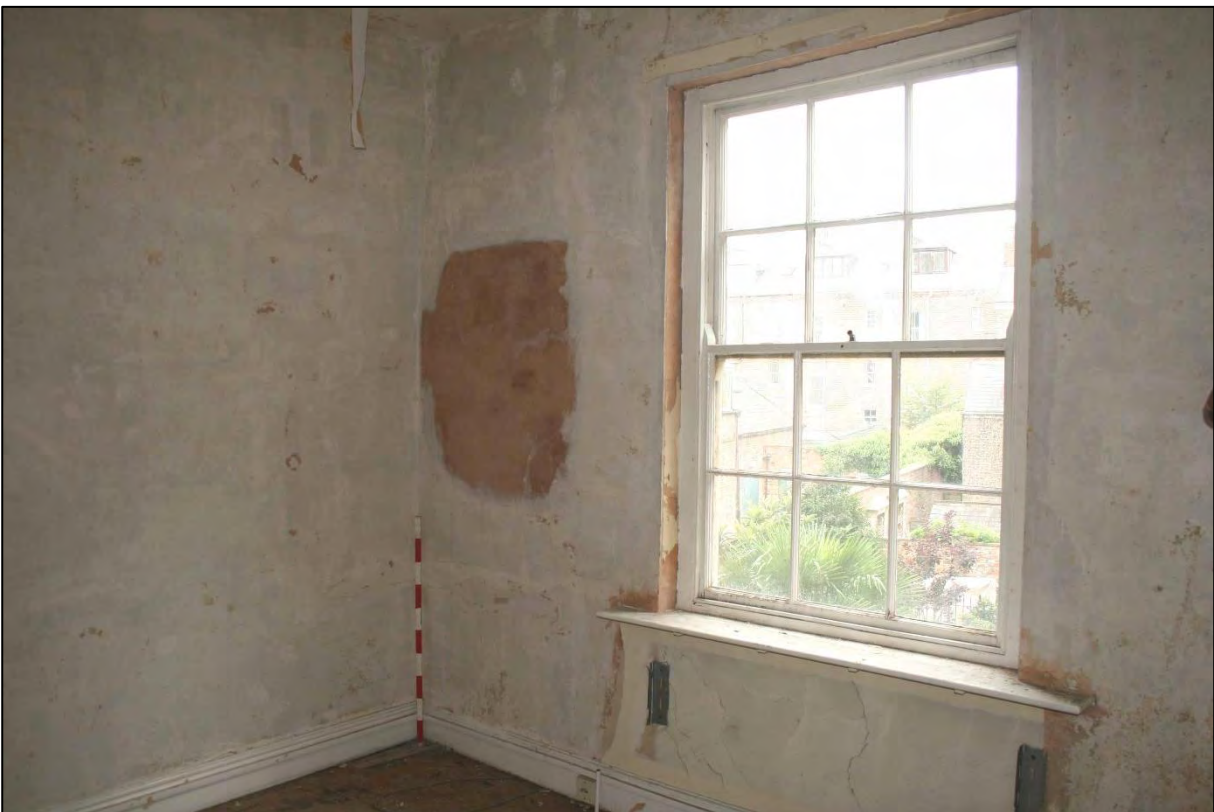
Plate 48. Room F10, looking southwest.
