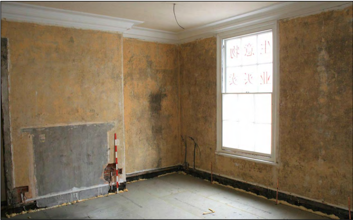
Plate 33. Room F1, looking northwest.
