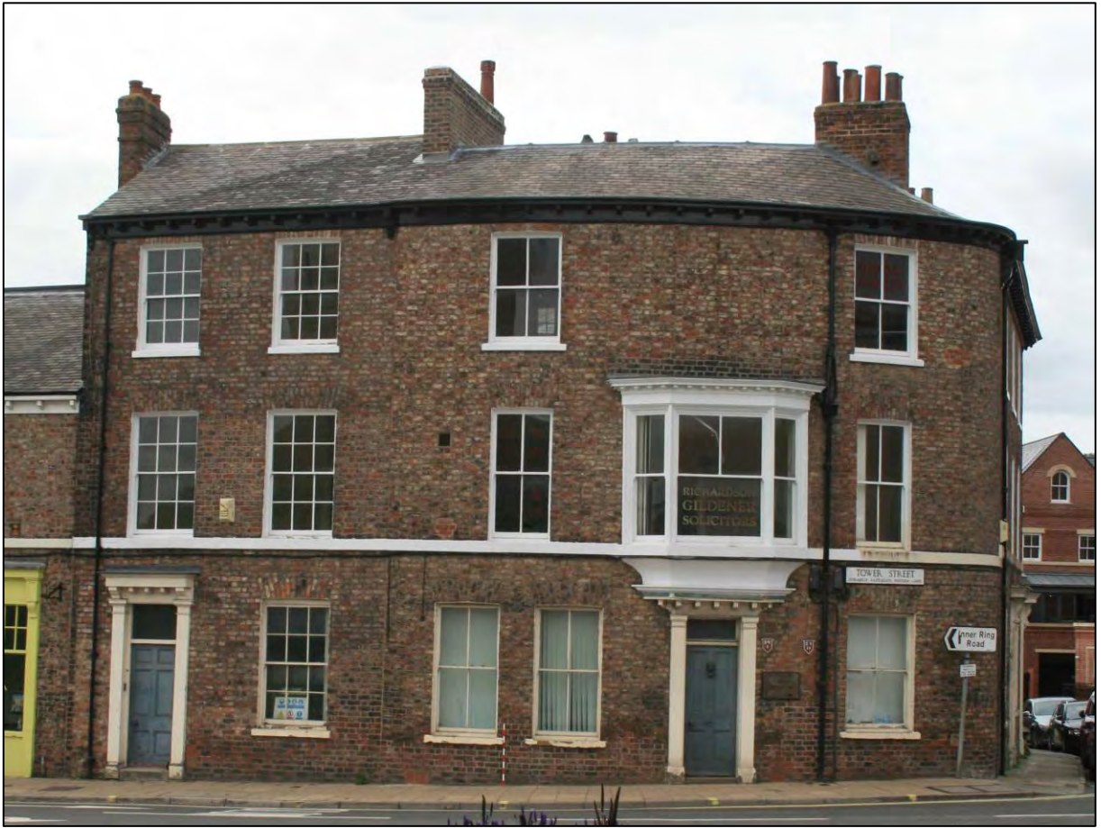
Plate 7. External view 6 and 7 Tower Street, looking west.
