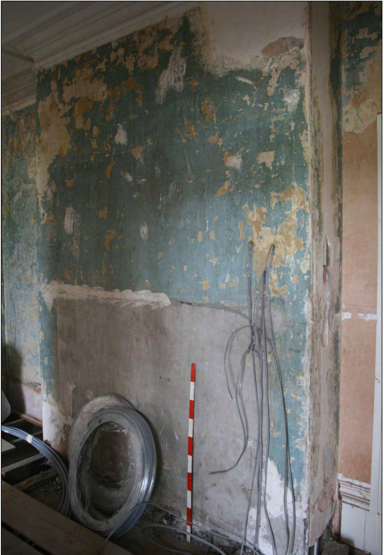
Plate 40. Room F6, chimney breast looking southwest.
