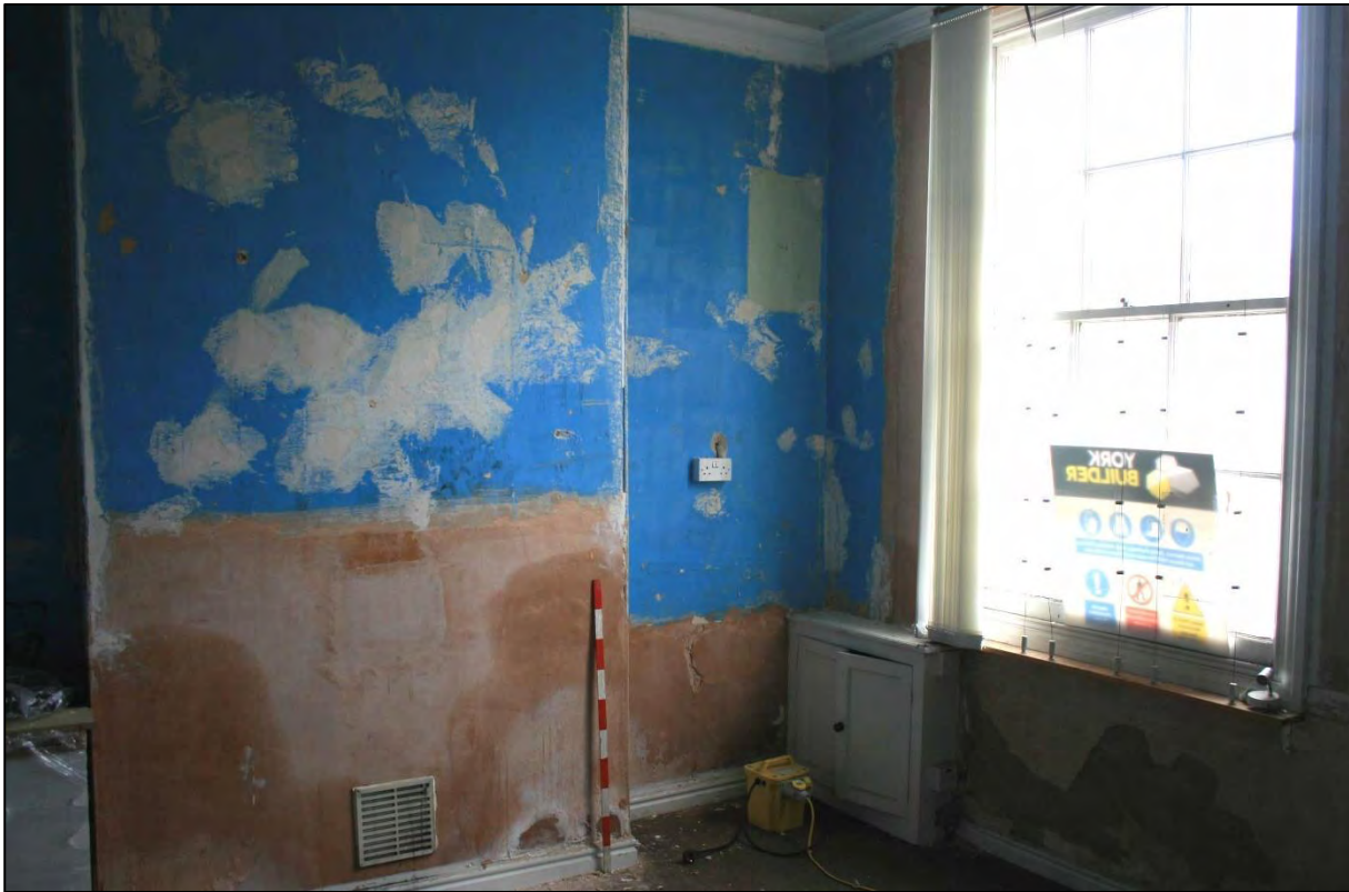
Plate 22. Room G7, looking northeast.
