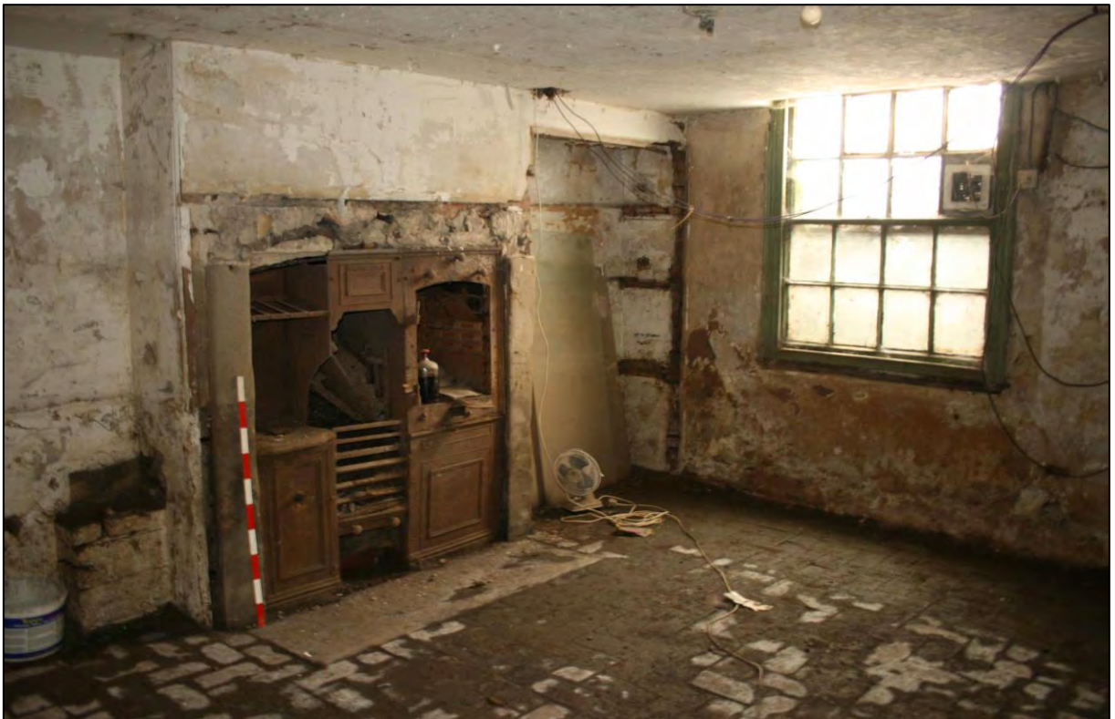
Plate 8. Room B1, showing grange and window.
