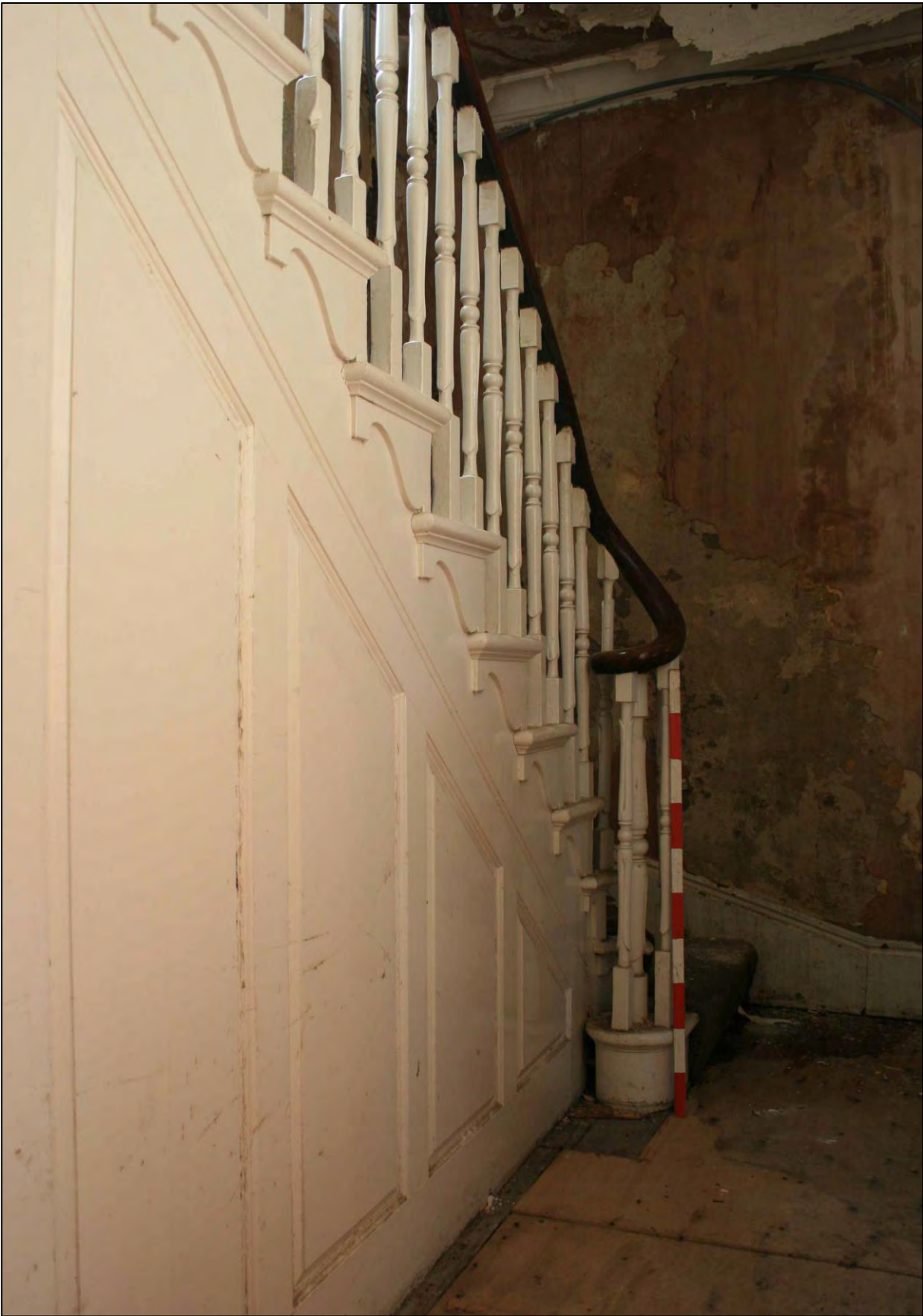
Plate 19. Room G5, stairs.
