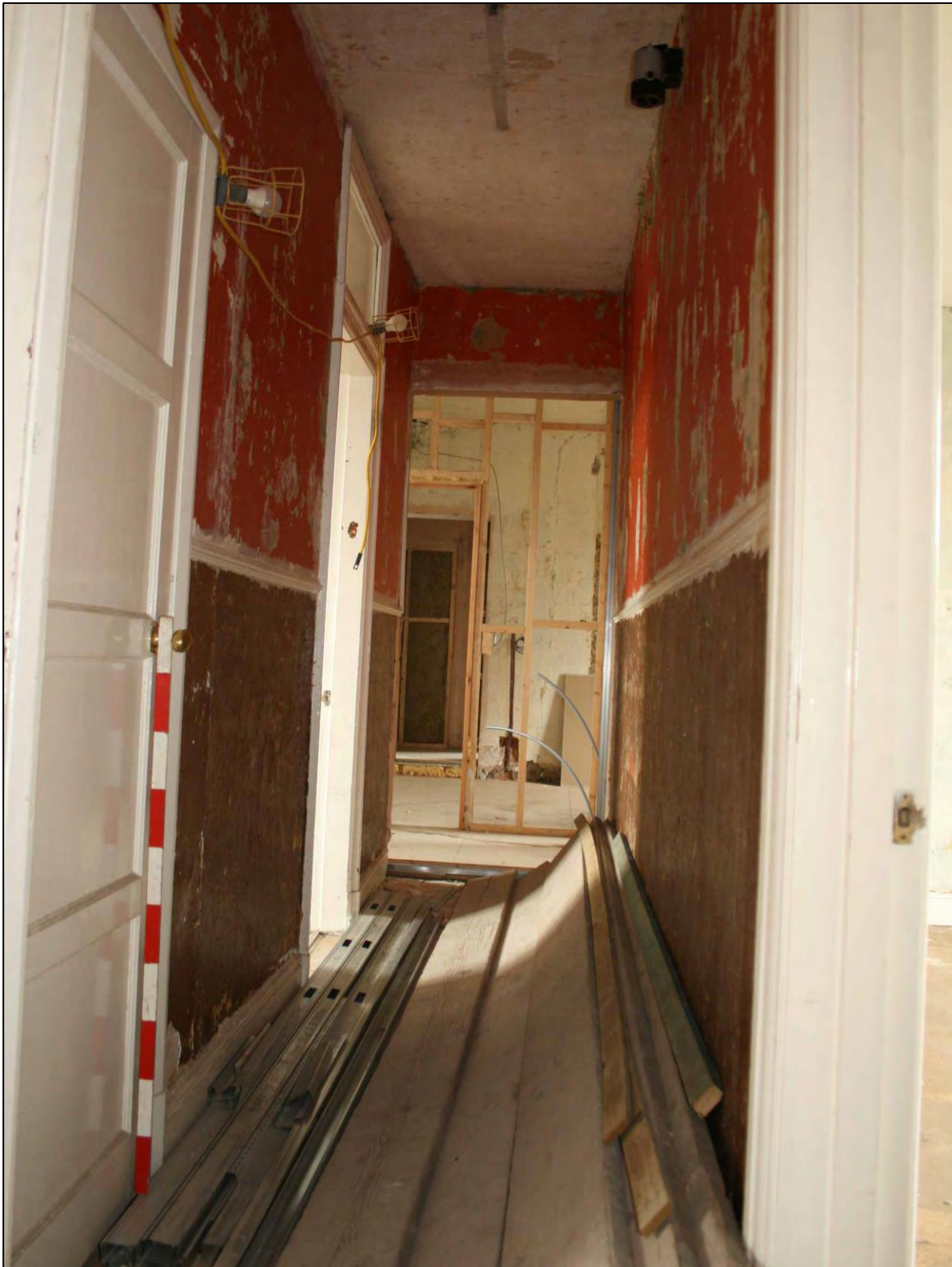
Plate 54. Room S10, looking north prior to blocking.
