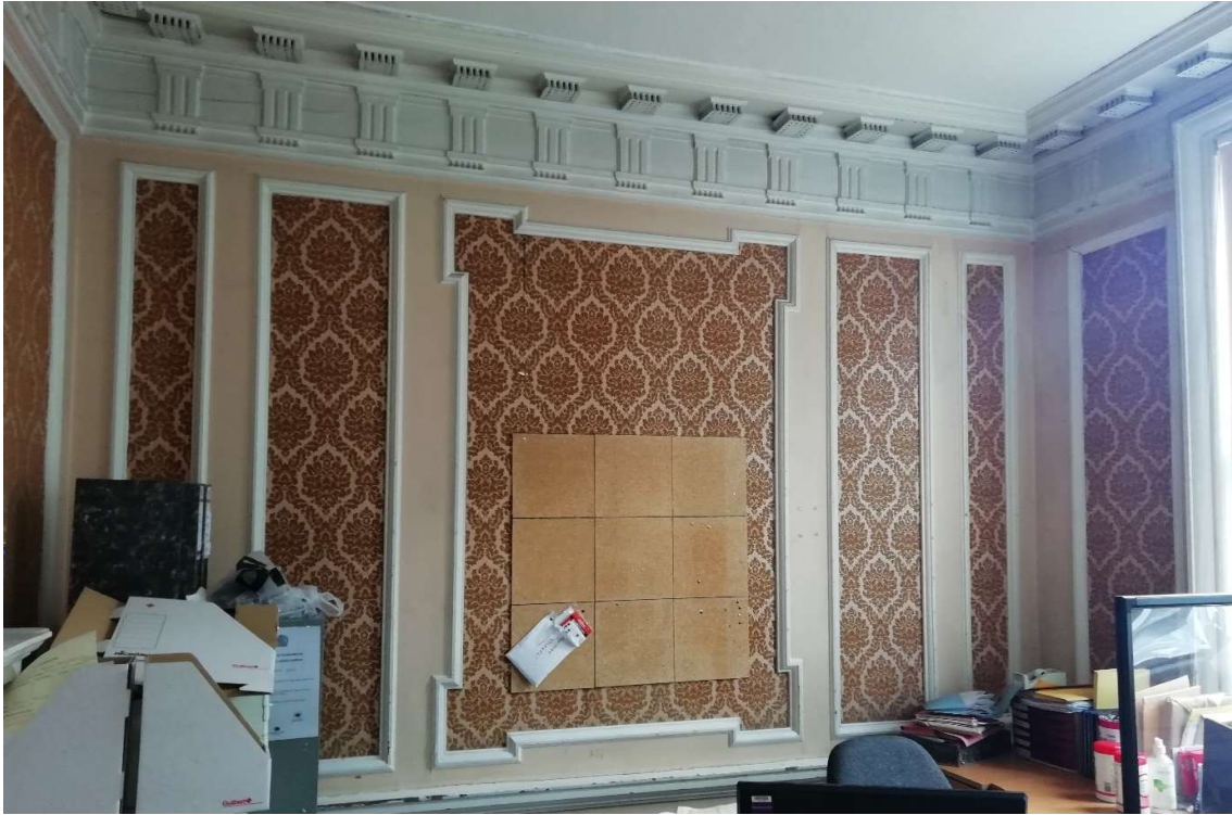
Fig 19 First floor, front, right hand room
