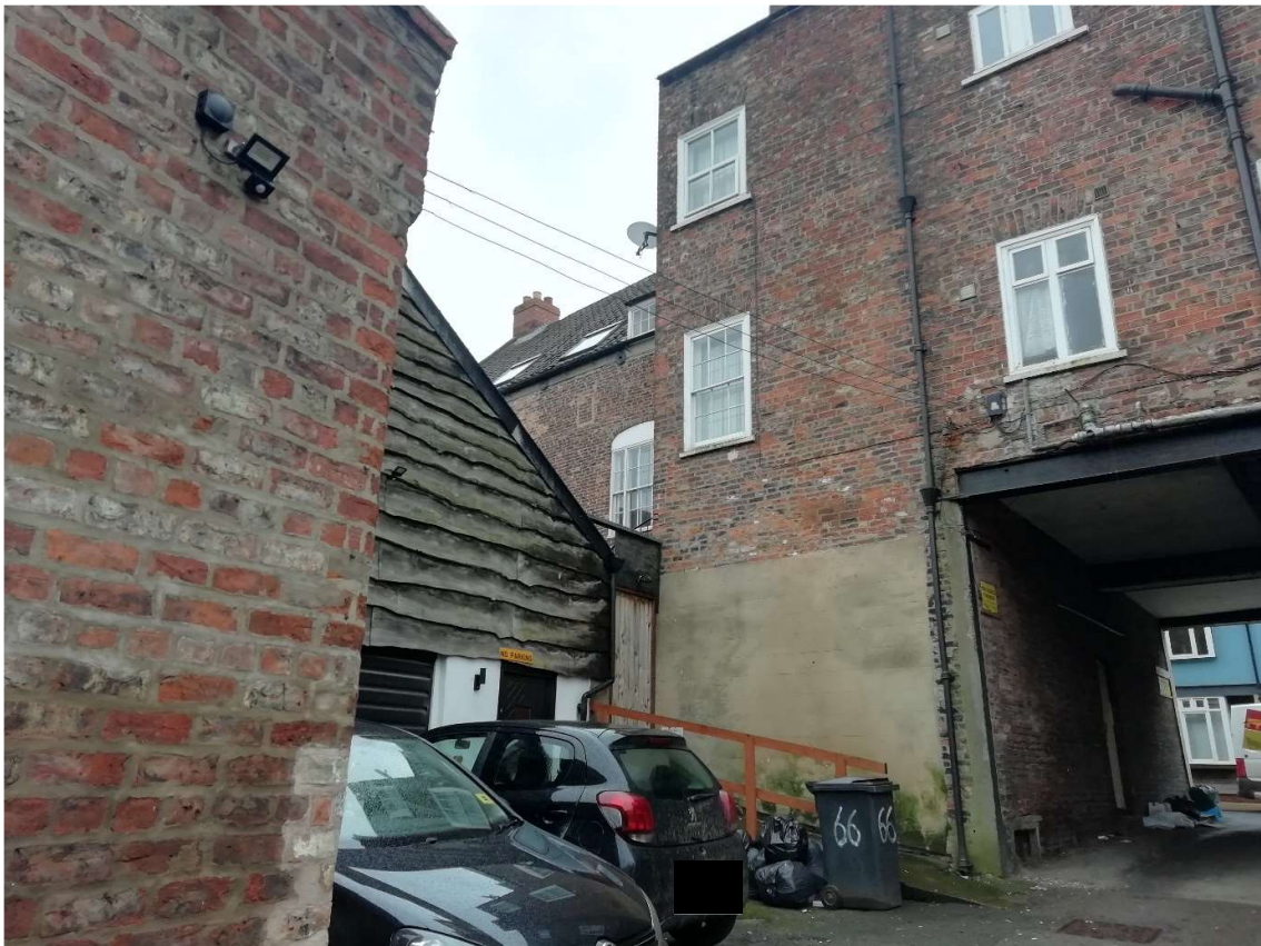
Fig 33 Limited view afforded of rear elevation from Melrose's Yard (note ramp/gate access to yard) Large Velux windows to be replaced with 3 no. smaller, conservation roof lights
