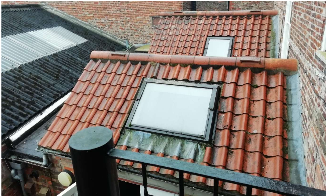
Fig 16 Double pile, rear extension with flat roof utility wing from fire escape
