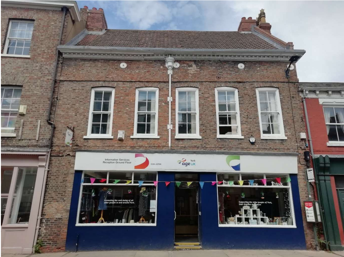
Fig 29D Modern shop front and lintol beneath to be removed and ground floor restored to residential use with four sash windows, a central doorway and reclaimed brick to match
