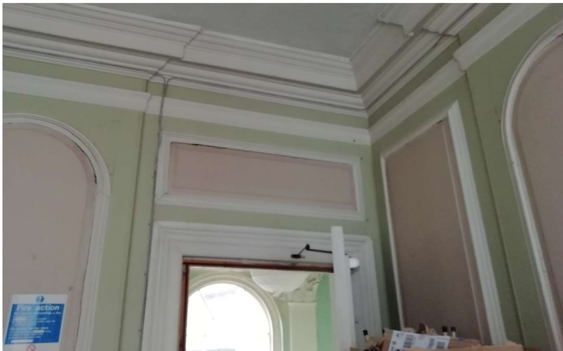
Fig 18 First floor, front, left room: bolection moulding and deep cornice
