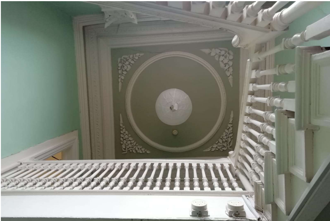
Fig 22 Decorative plasterwork above stair bay (wall mounted electrics to be removed)
