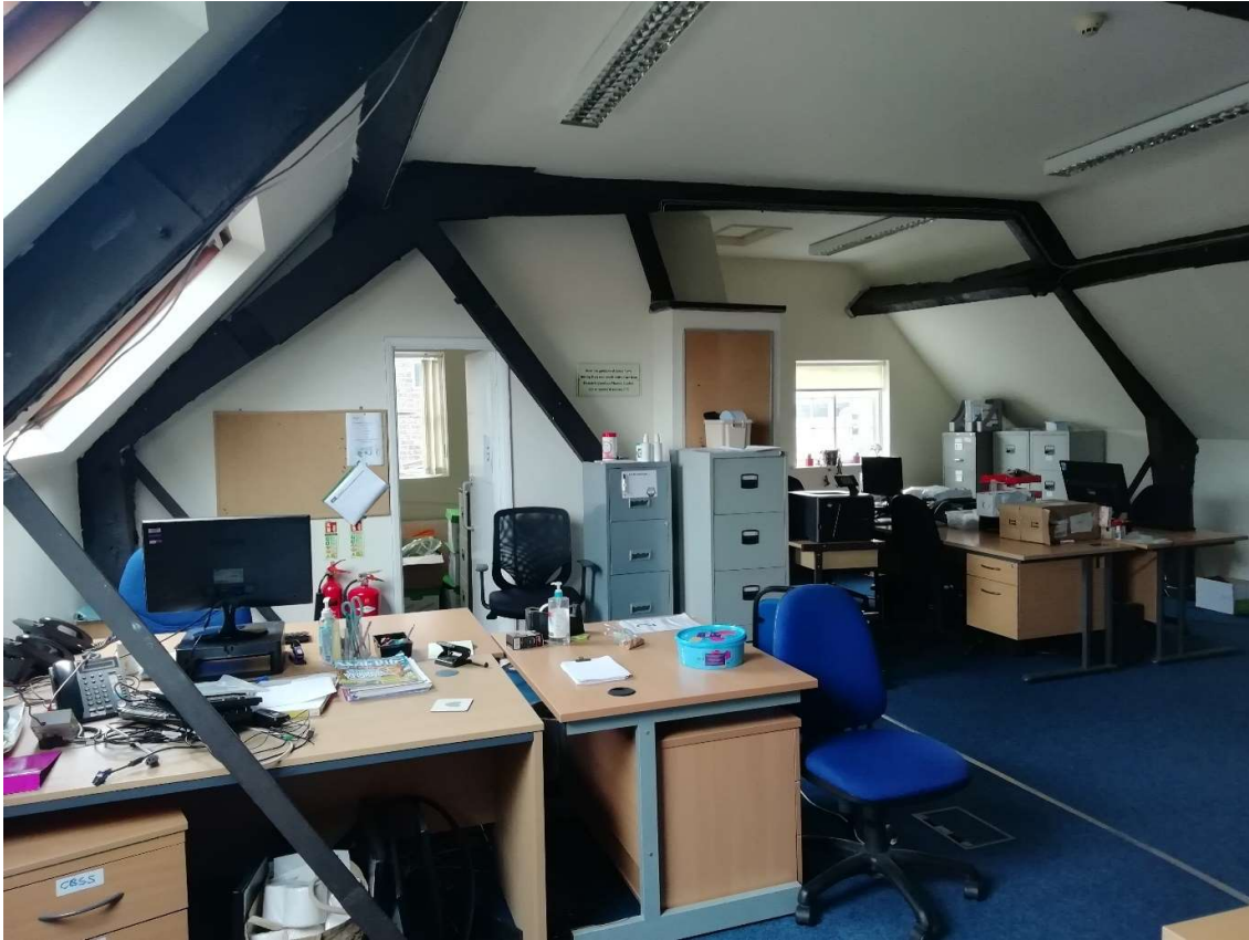
Fig 12 Attic (west to east) with gable windows and steel, strap ties
