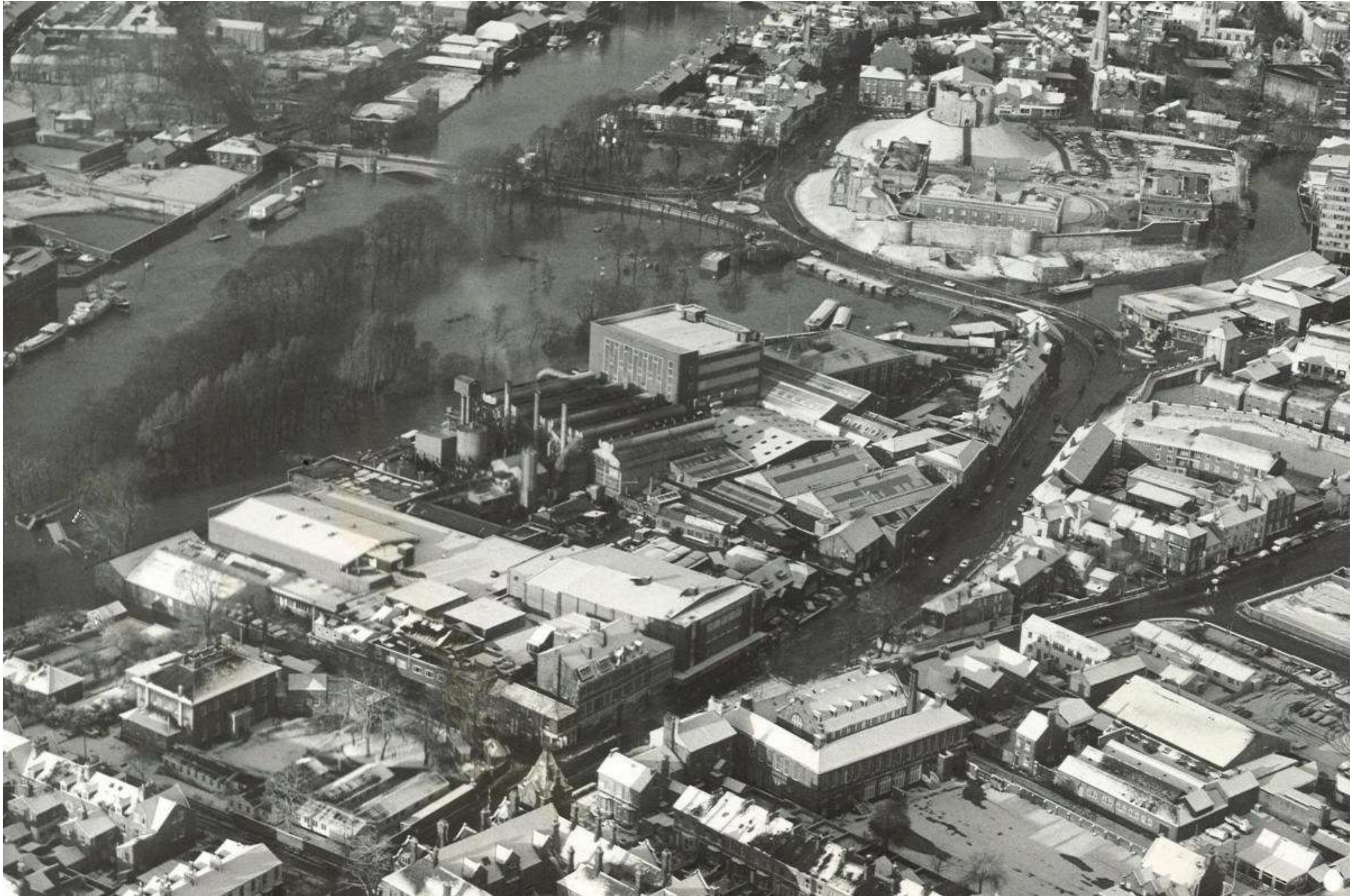
3.4.14 Aerial Photograph of the 'site' and area around, taken in 1978 (source: York Press)
