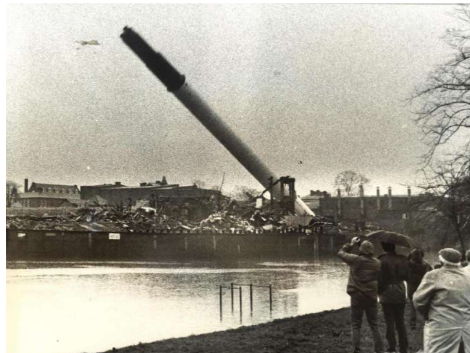
Chimney being demolished in 1986 (source: York Press)
