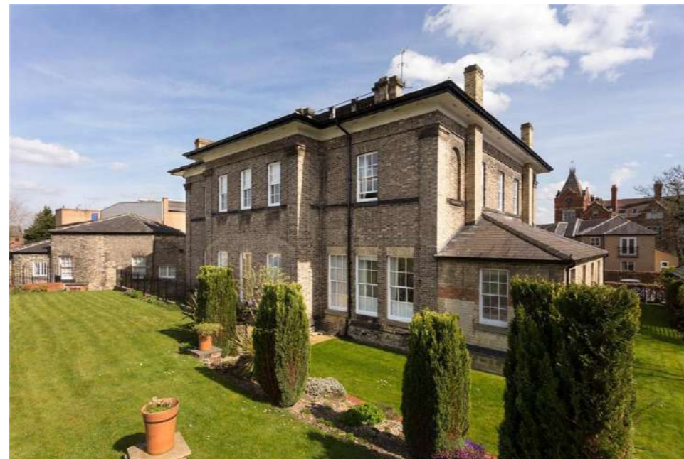
Fishergate House West Elevation (source: On The Market)
