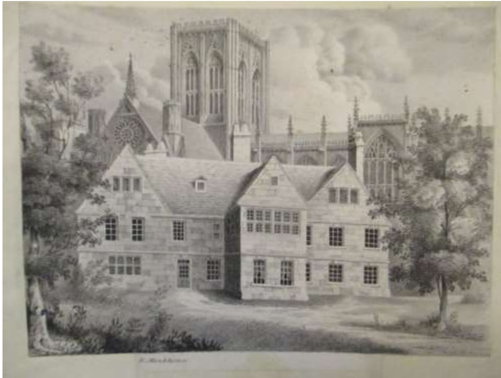
Above Fig. 15: Clearly an engraving by the same artist W Monkhouse as Fig 11 of the north frontage this view shows the south elevation of the old deanery and is similar to Fig 13. It clearly shows the quality and sheer size of the building. Here it should be borne in mind that the south west service wing and west wing extended to the west (left) and are not shown
