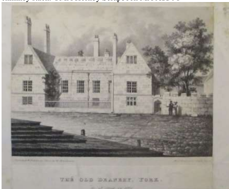
Above Fig 12: Another view of the old deanery from the north showing the hall and flanking projecting cross wings with a mixture of mullioned and sash windows. The crenelated wall has been replaced by railings in part. At right the south west range can be seen behind the tree and on the right the west range returning northwards. YMA Hornby Scrapbook MA Add 91
