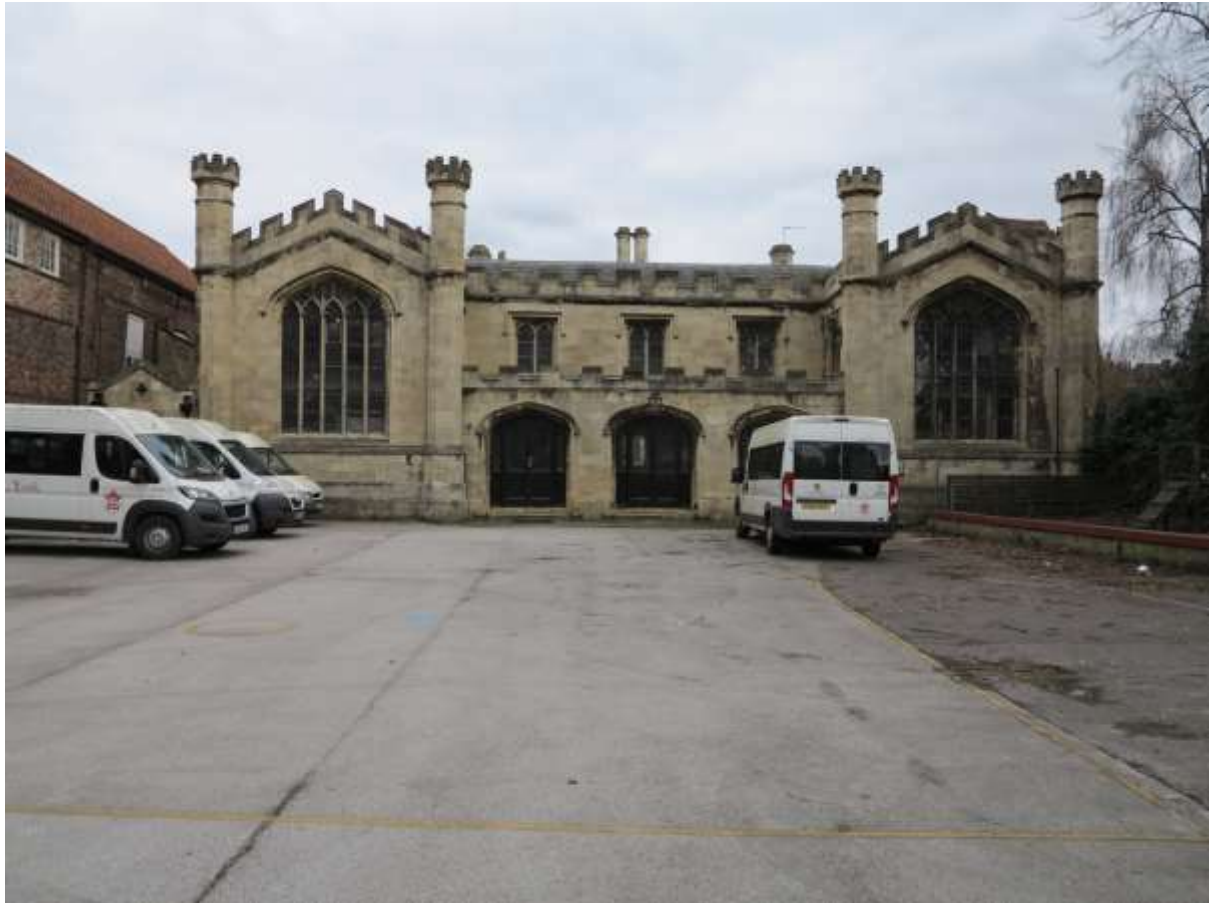
Above Fig 30 The school building as it appears today largely unchanged since it was first built
