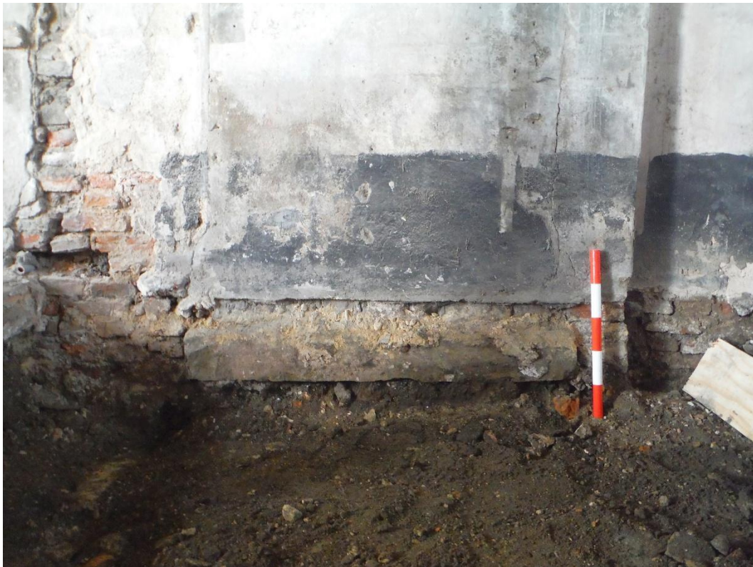
Plate 1 Blocked doorway room 1. Facing southeast scale unit 100mm
