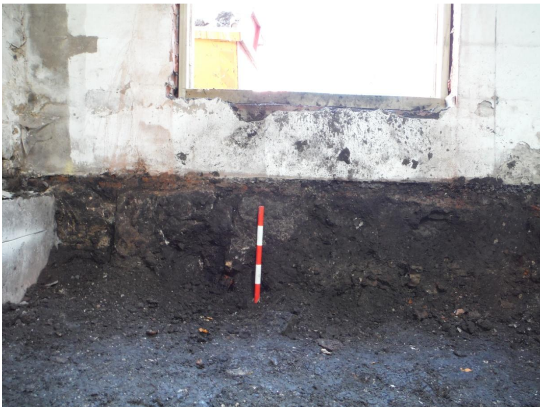
Plate 8 Rear boundary wall, room 9. Facing northeast, scale unit 100mm
