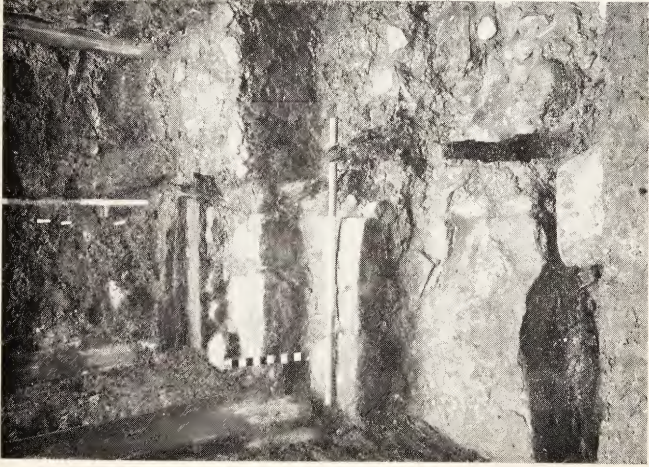
PLATE I. The excavation—showing flight of steps.
