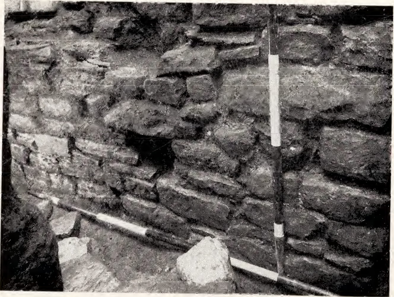
PLATE X. Trench 6. South-west wall of barrack block showing opening for drain.
