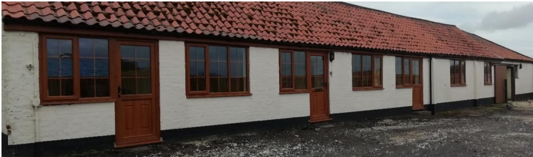
Fig 40 Left door & window and 3 rd door from left to be blocked & fascia boards removed
