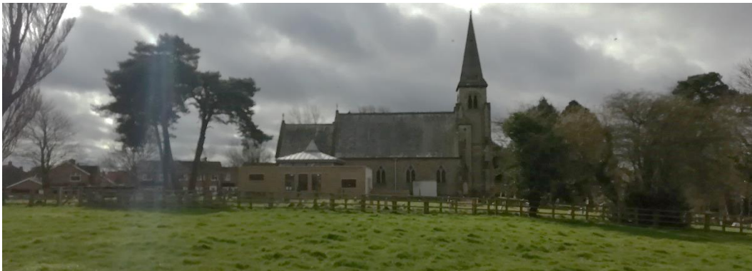
Fig 30 St Mary's Church from the north with geometrical extension
