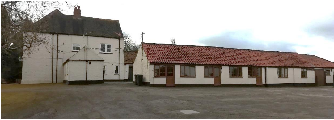
Fig 7 Office range to norther of house with modern openings and plastic fittings
