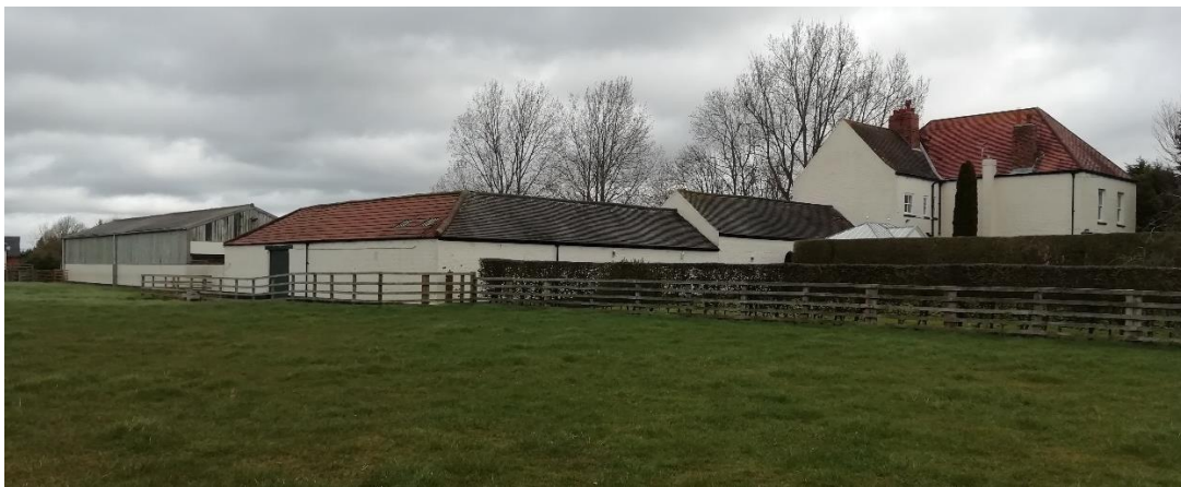
Fig 8 In views from the fields the white masonry unifies the farmhouse and the farmyard
