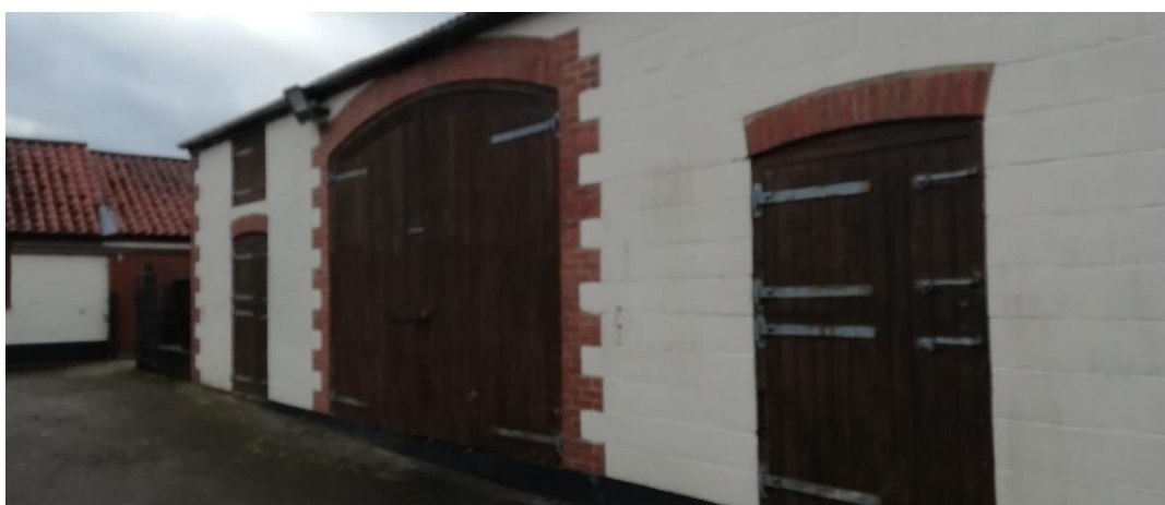
Fig 27 Arched openings, albeit on too large a scale, inspired by traditional cart openings
