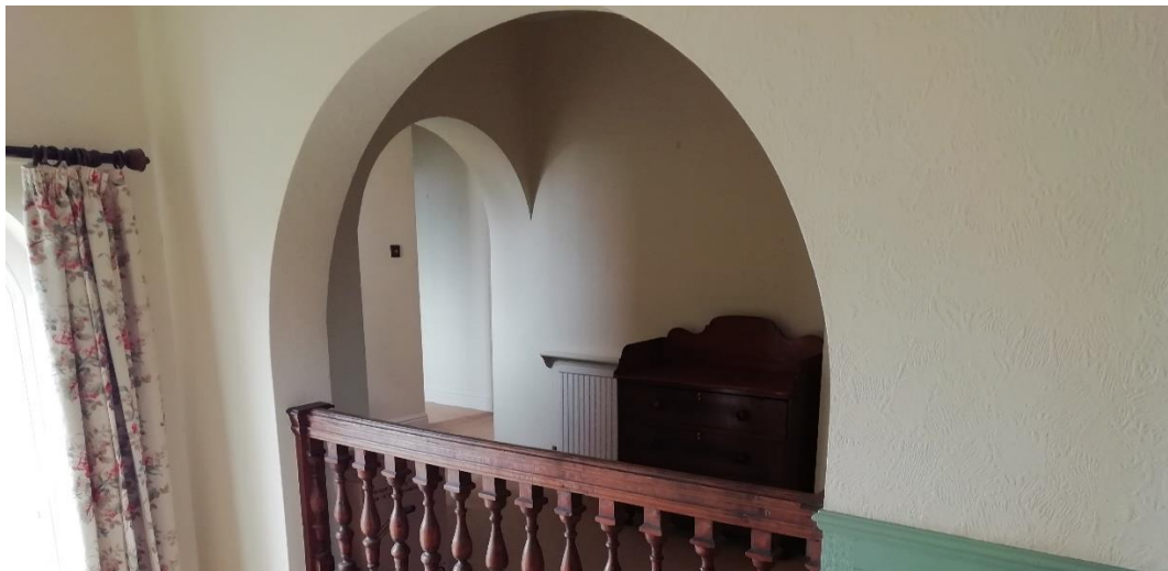
Fig 35 Two 1980’s arches formed from stud walling to be squared off
