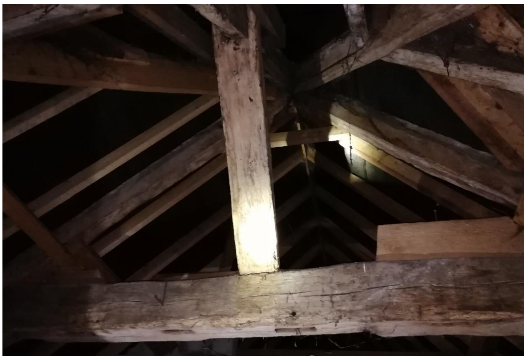
Fig 11 Roof structure with modern rafters and felt and breezeblock supporting wall
