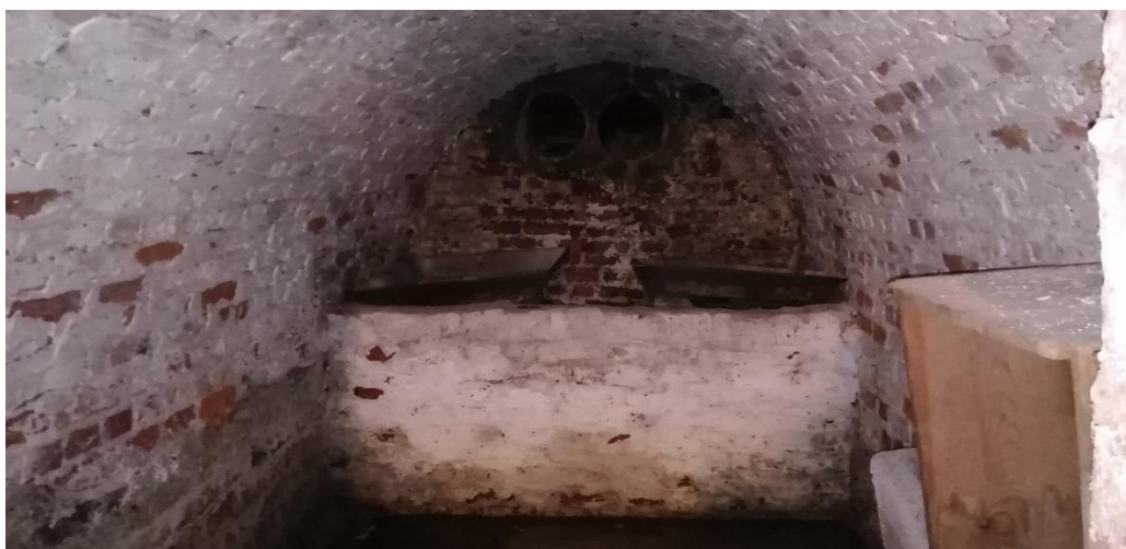
Fig 10 Former coal chute (now blocked) in current cellar
