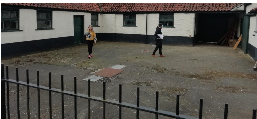
Fig 6 Split level tarmac foldyard bisected by modern steel fence
