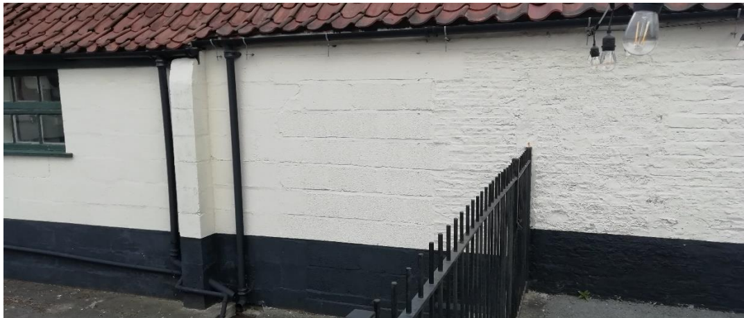
Fig 41 Blocked opening to be re-opened
