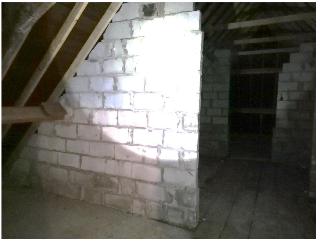
Fig 12 Breezeblock supporting walls within attic space with modern roof timbers
