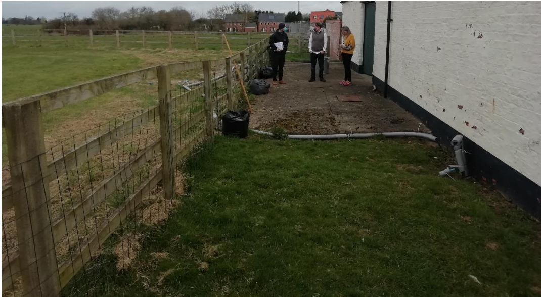
Fig 41 Concrete hardstanding and narrow, non-vernacular enclosure to be removed
