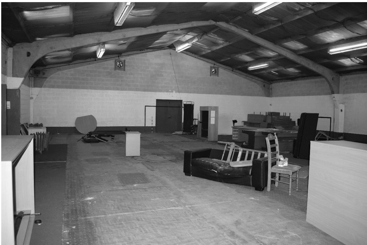
Plate 122. Gym: Interior (DSC_0670). Facing North-west.
