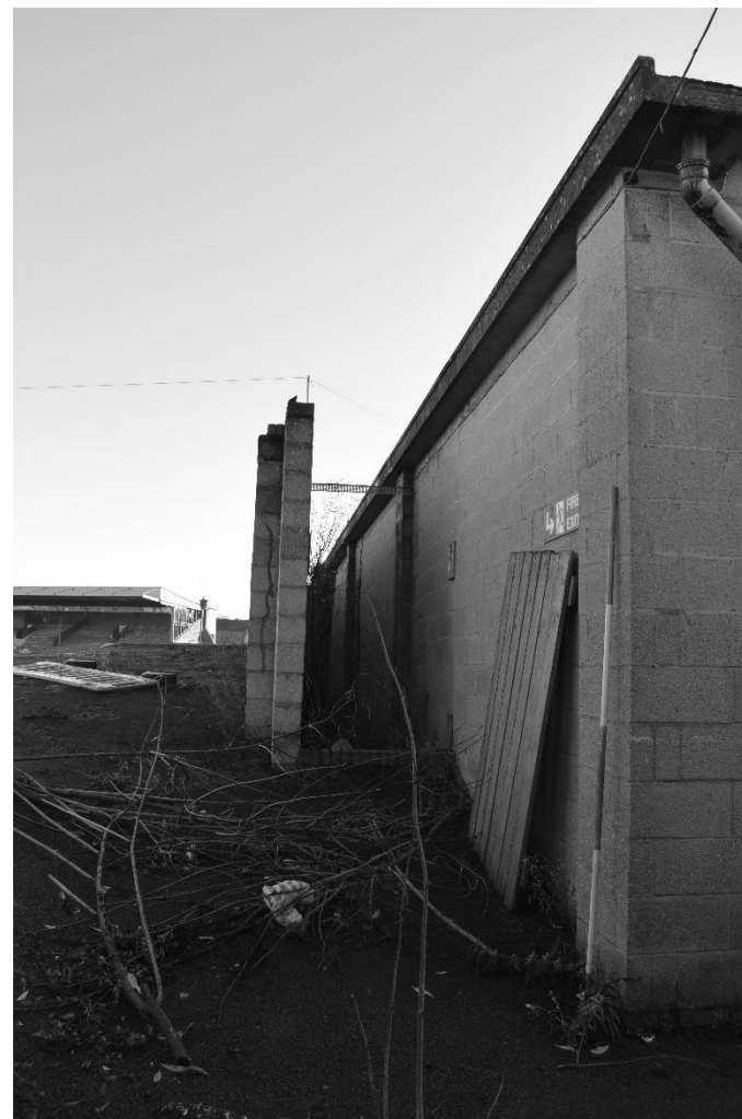
Plate 68. Gym: Exterior North Elevation (DSC_0789). Facing South-east.
