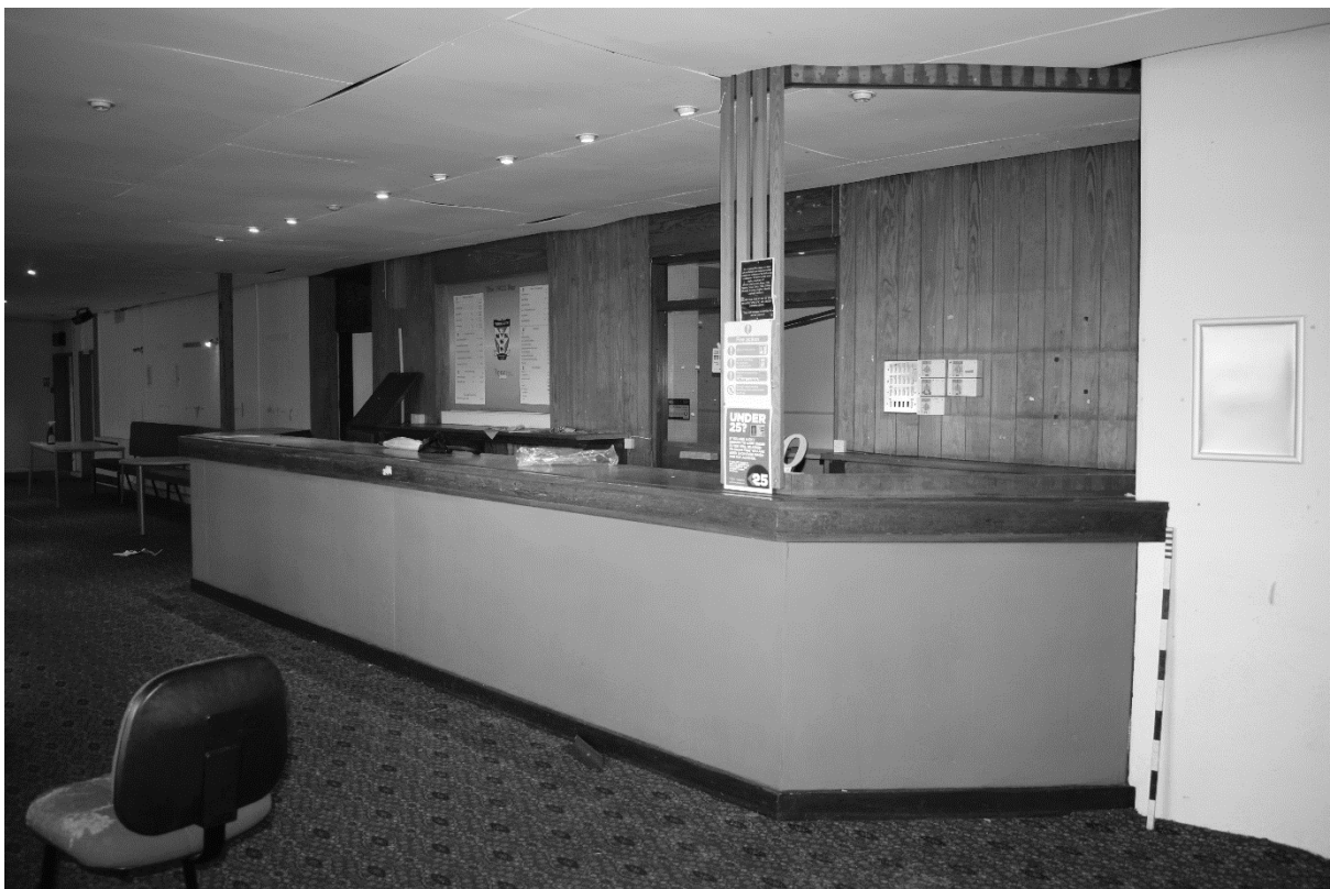
Plate 72. 1922 Bar: Interior Ground Floor (DSC_0575). Facing North-east.
