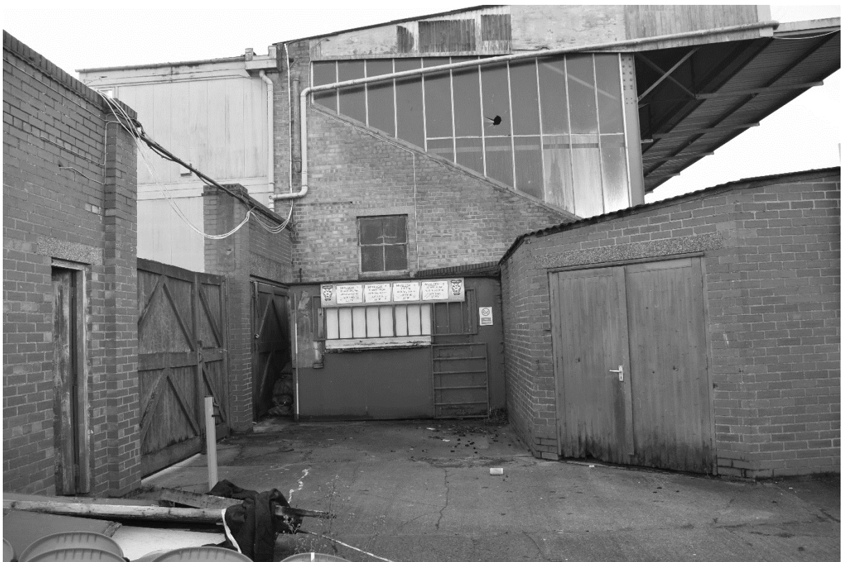
Plate 14. Entrances at north end of car park (DSC_0723). Facing South.
