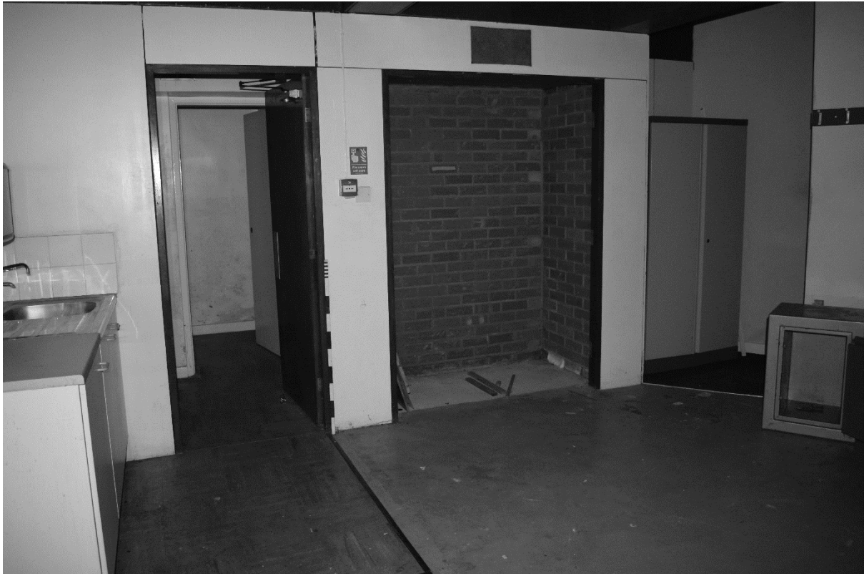
Plate 89. Club Shop: Interior (DSC_0607). Facing North.
