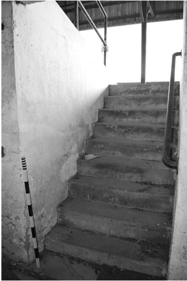
Plate 63. Popular Stand Tunnel Stairs (DSC_0687). Facing East.
