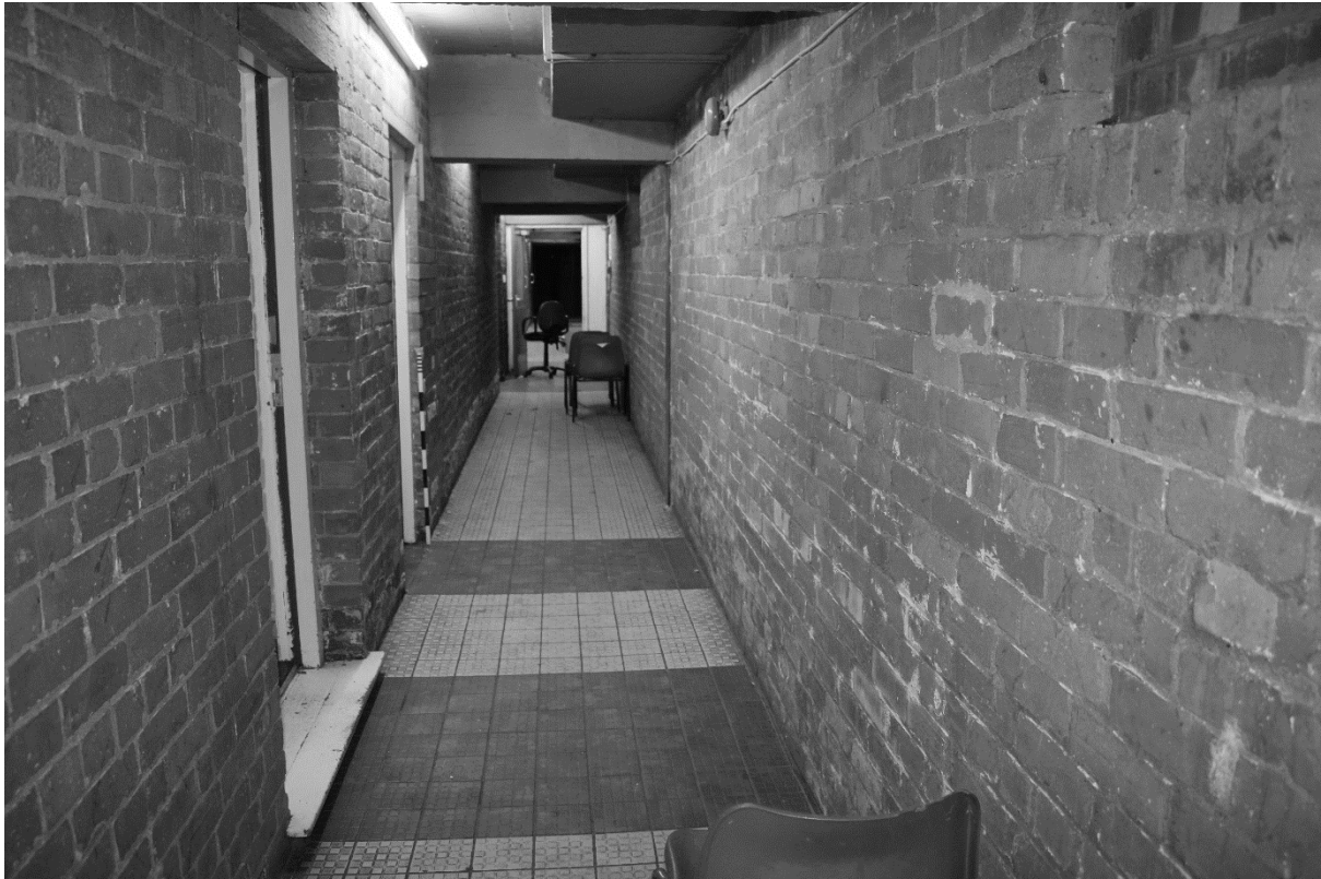
Plate 91. Main Stand: Interior Ground Floor (DSC_0650). Facing South.
