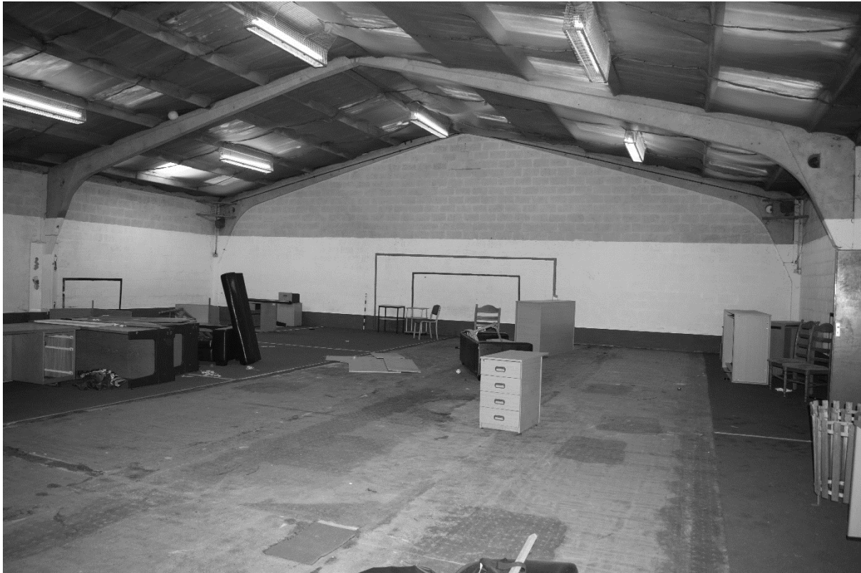
Plate 123. Gym: Interior (DSC_0671). Facing North-east.
