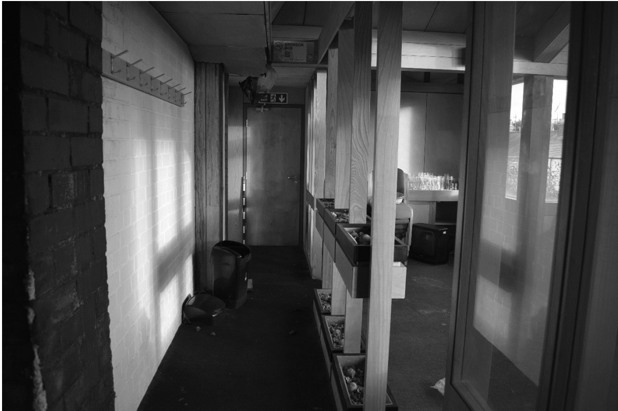
Plate 119. Main Stand: Interior Second Floor (DSC_0616). Facing North.
