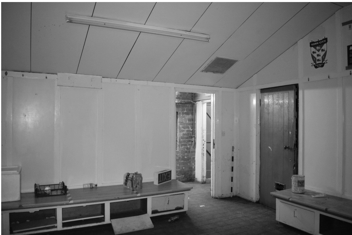
Plate 98. Main Stand: Interior Ground Floor (DSC_0664). Facing North-west.
