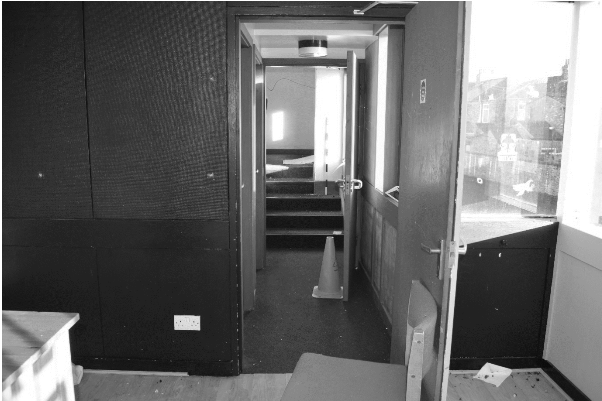
Plate 105. Main Stand: Interior First Floor (DSC_0627). Facing North.
