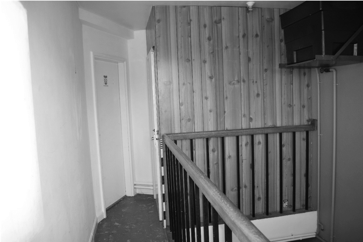
Plate 81. 1922 Bar: Interior First Floor (DSC_0594). Facing North-west.
