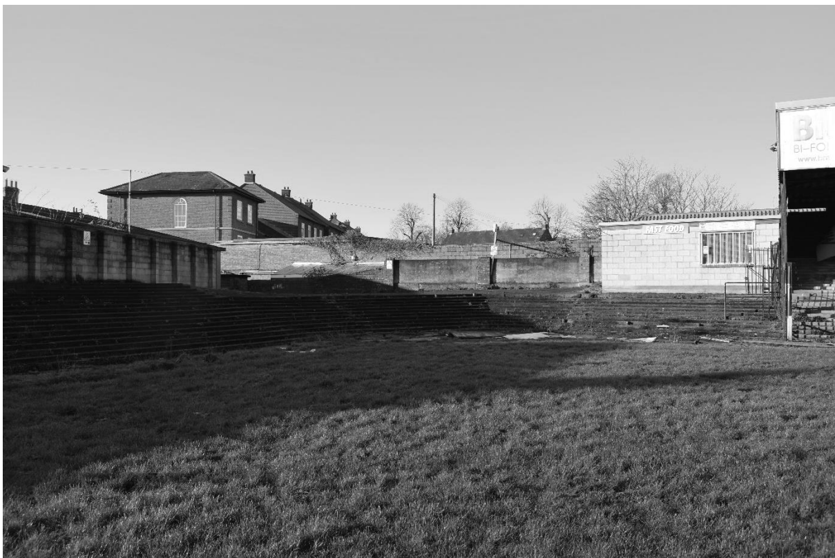
Plate 30. Grosvenor Road End (DSC_0784). Facing West.
