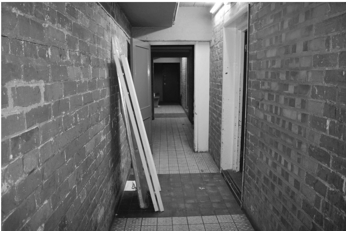
Plate 90. Main Stand: Interior Ground Floor (DSC_0646). Facing North.
