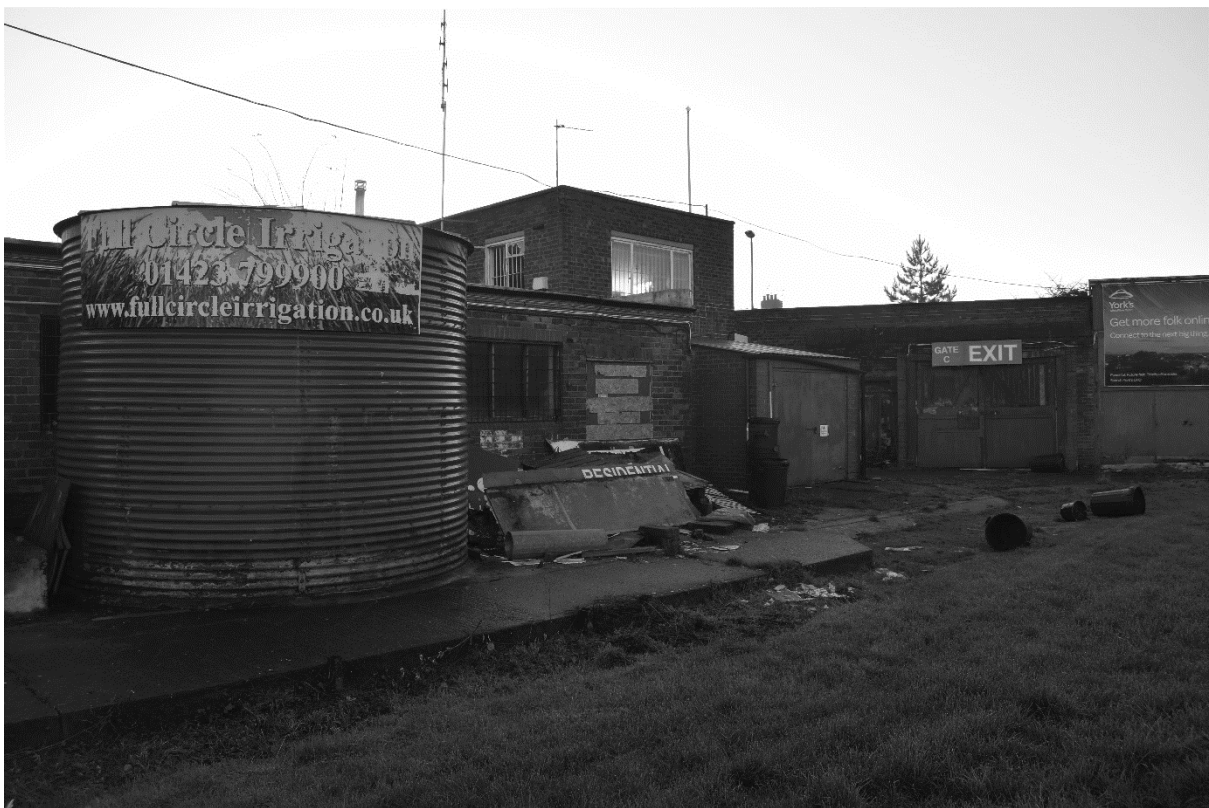
Plate 16. Entrances at east side of Grosvenor Road End (DSC_0725). Facing South.
