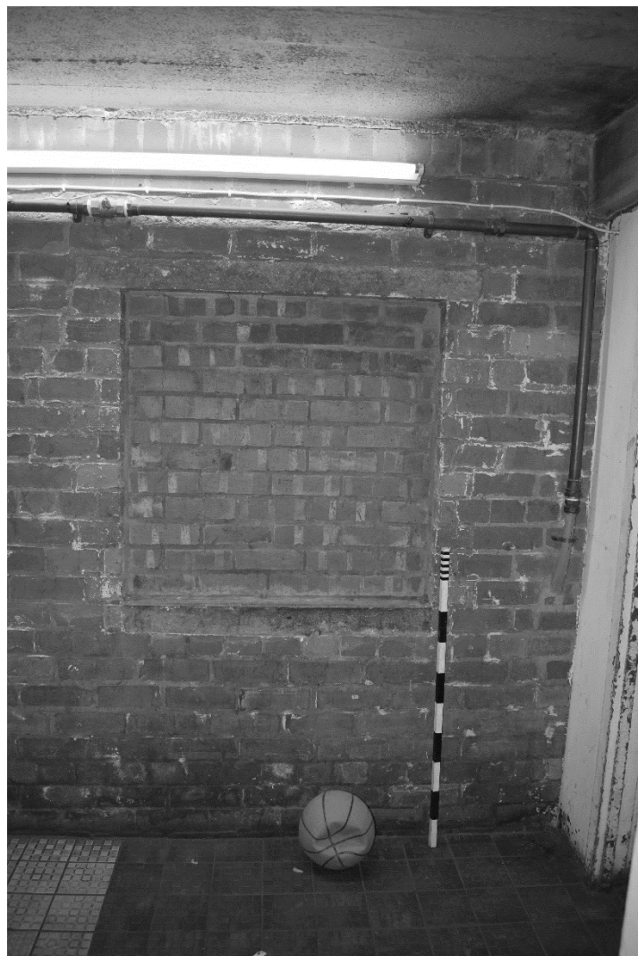
Plate 100. Main Stand: Interior Ground Floor (DSC_0655). Facing West.
