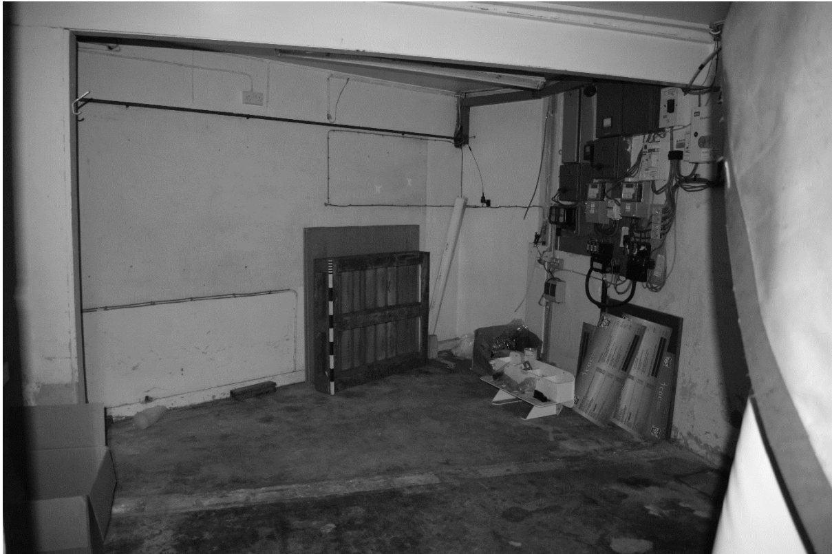
Plate 75. 1922 Bar: Interior Ground Floor (DSC_0585). Facing East.
