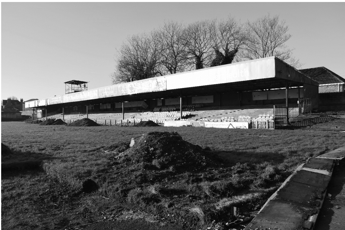
Plate 54. Popular Stand: Exterior North and East Elevations (DSC_0776). Facing South-west.
