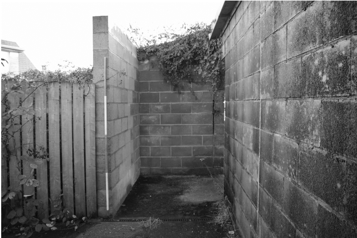
Plate 53. Rear Access to David Longhurst Stand (DSC_0768). Facing East.
