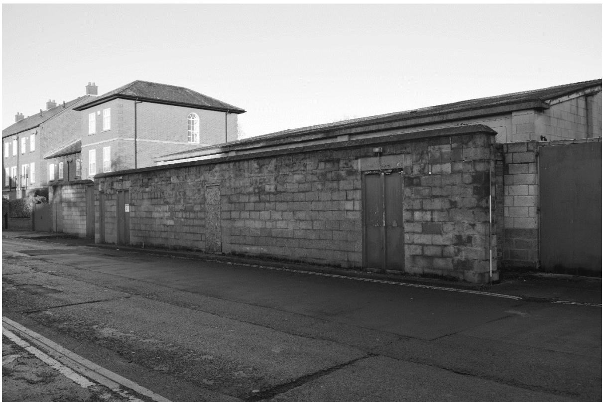
Plate 8. Entrances on Grosvenor Road (DSC_0704). Facing North-west.
