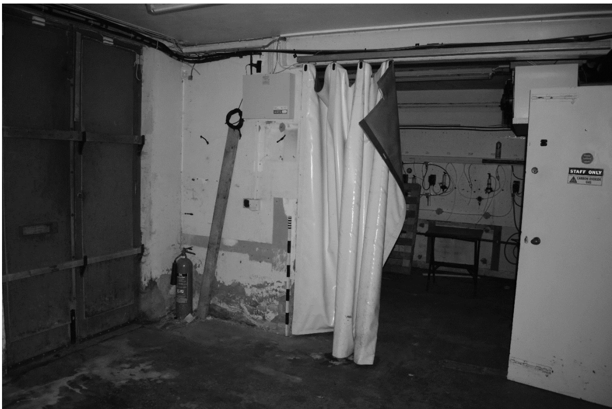
Plate 76. 1922 Bar: Interior Ground Floor (DSC_0586). Facing West.
