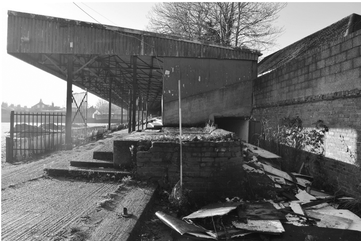
Plate 56. Popular Stand: Exterior North Elevation and Tunnel (DSC_0772). Facing South.
