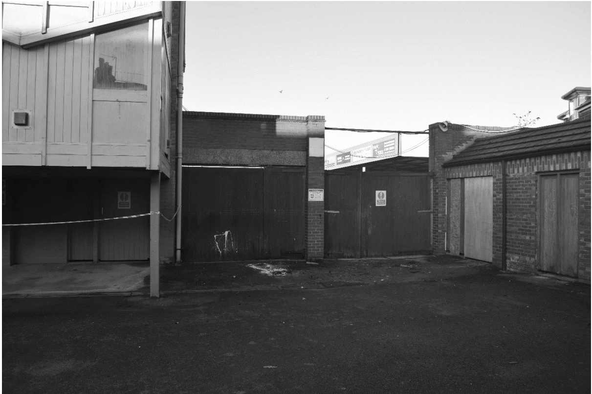
Plate 11. Entrances at north end of car park (DSC_0721). Facing West.
