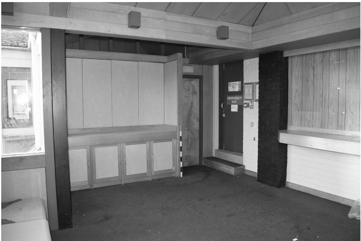
Plate 118. Main Stand: Interior Second Floor (DSC_0614). Facing South-west.
