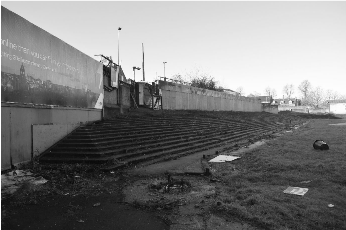
Plate 27. Grosvenor Road End (DSC_0730). Facing West.
