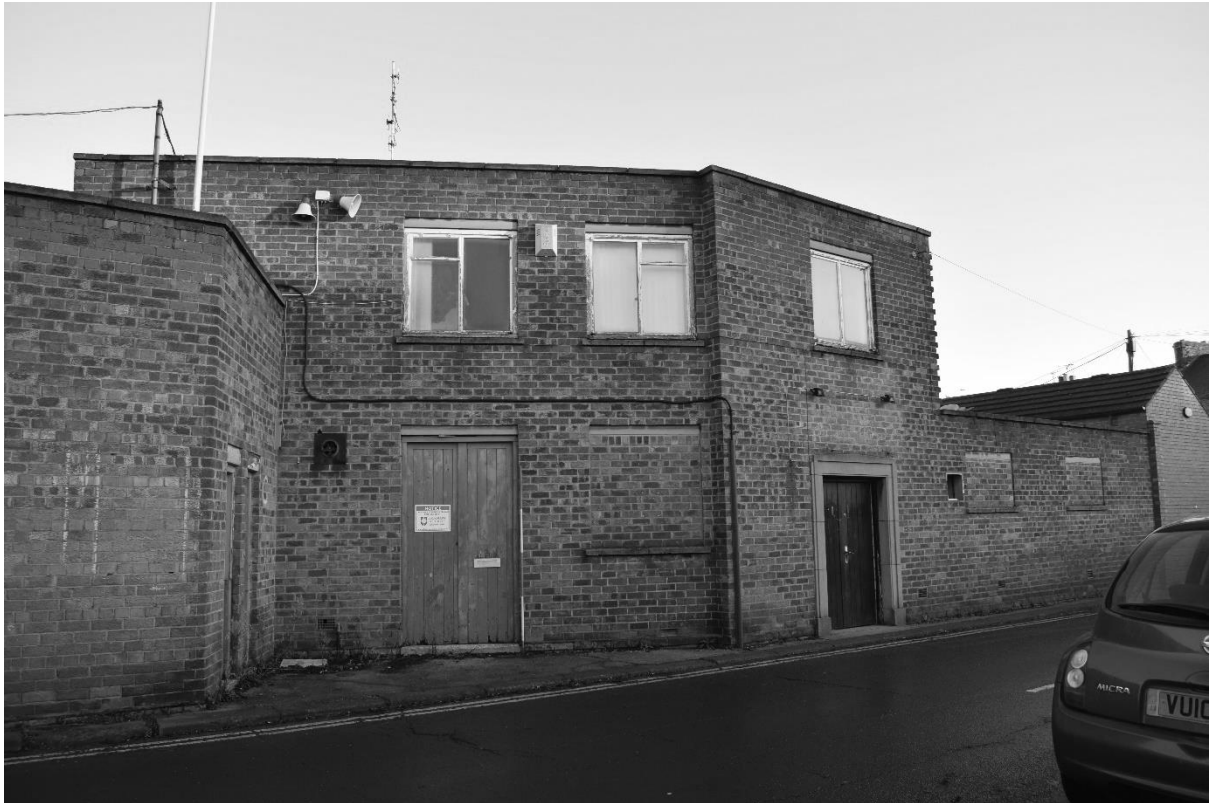
Plate 35. 1922 Bar: Exterior South Elevation (DSC_0697). Facing North.
