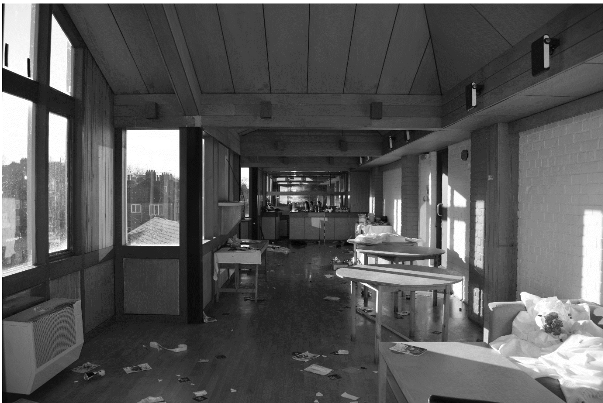
Plate 114. Main Stand: Interior Second Floor (DSC_0628). Facing South.
