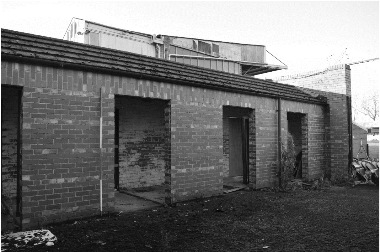
Plate 13. Entrances at north end of car park (DSC_0759). Facing South-west.
