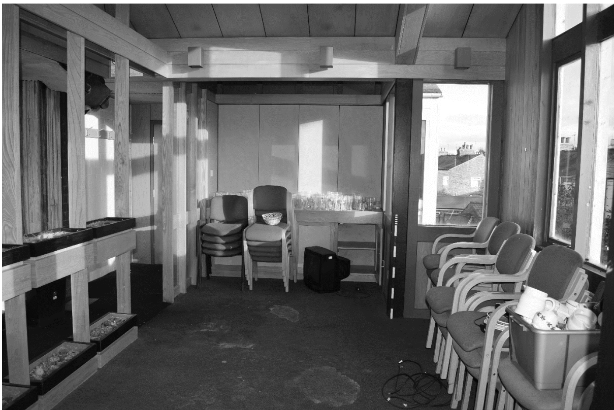
Plate 120. Main Stand: Interior Second Floor (DSC_0617). Facing North.
