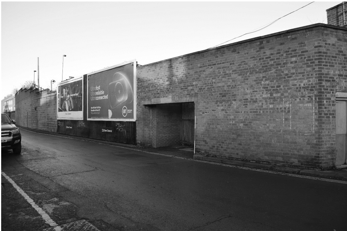
Plate 6. Grosvenor Road Boundary Wall (DSC_0700), Facing West.
