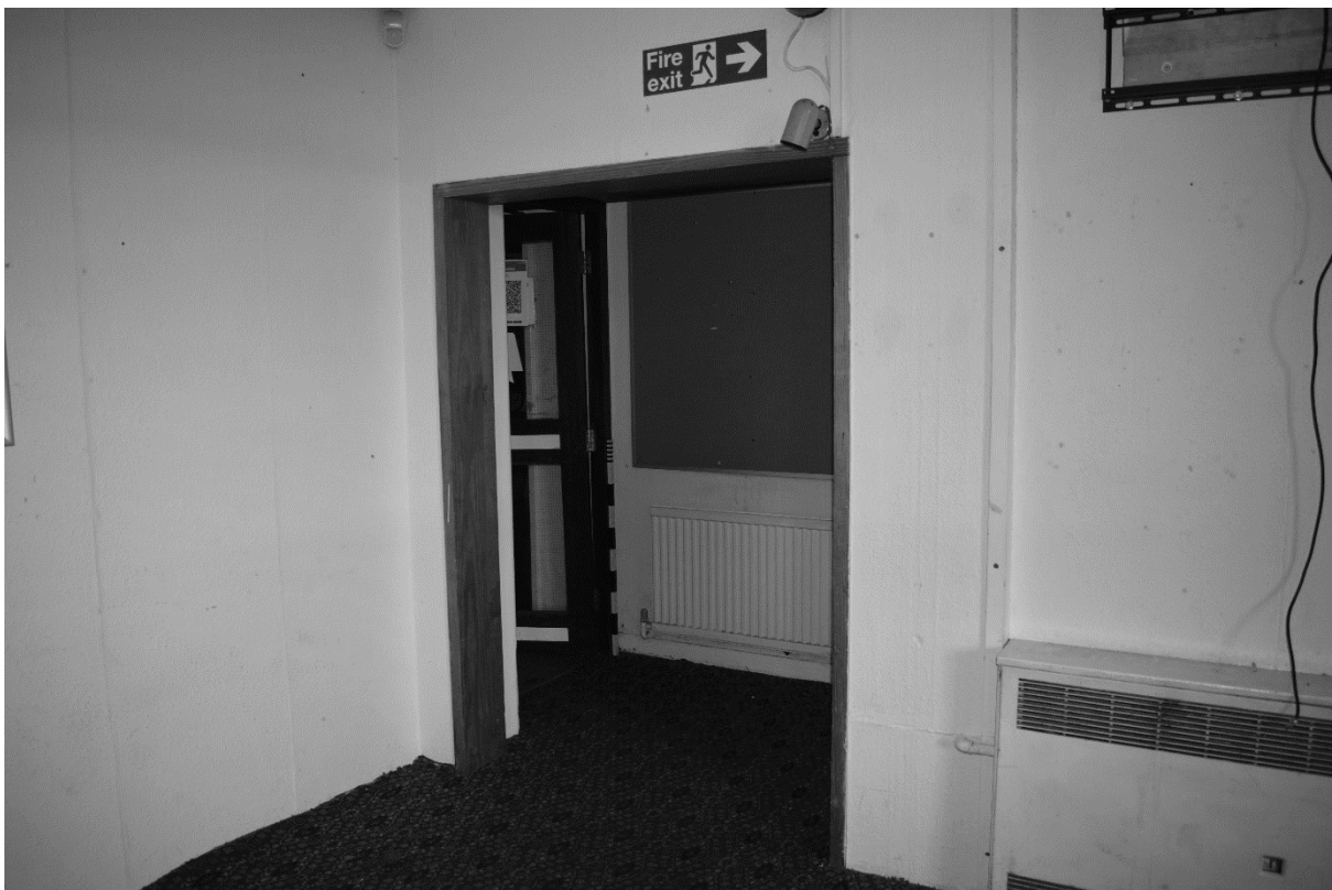
Plate 74. 1922 Bar: Interior Ground Floor (DSC_0581). Facing North.
