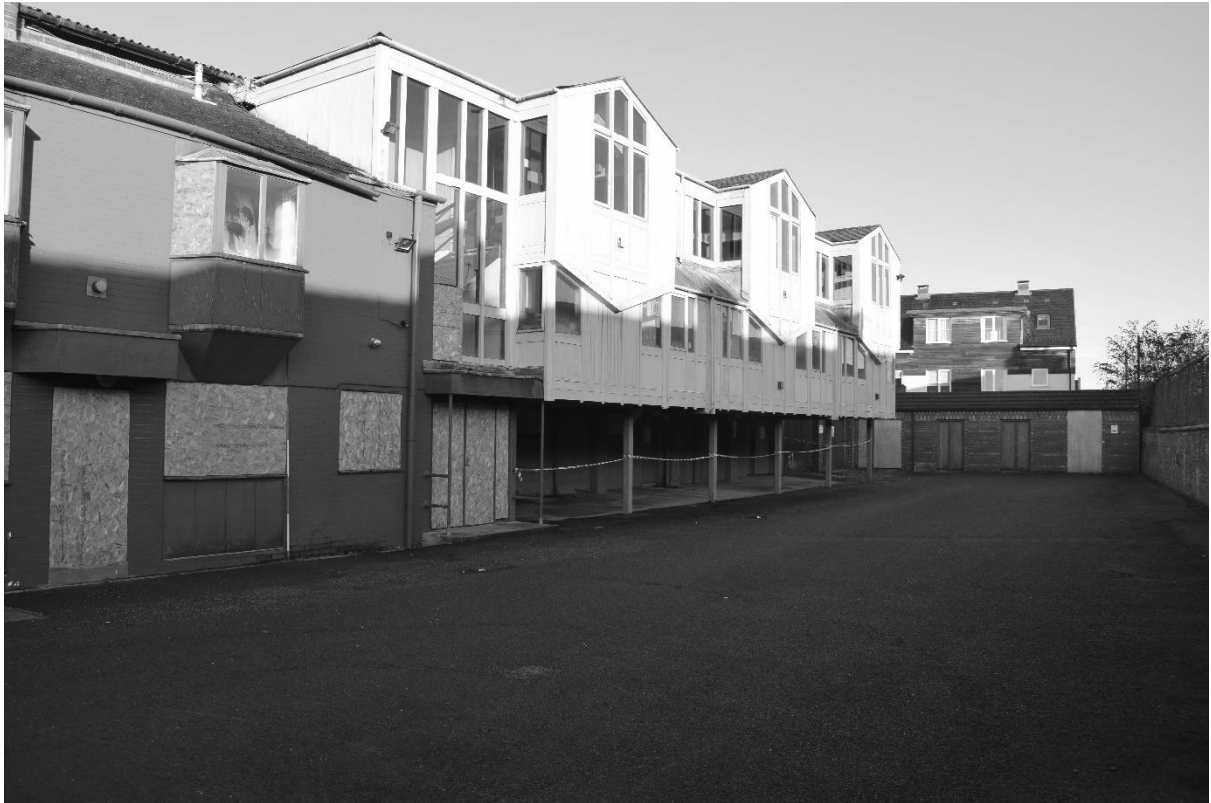
Plate 43. Main Stand: Exterior East Elevation (DSC_0719). Facing North-west.
