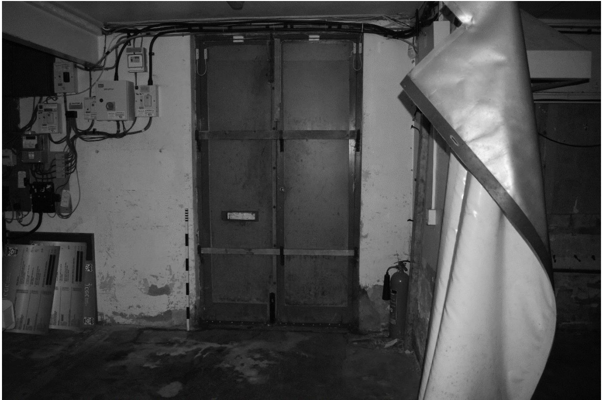
Plate 77. 1922 Bar: Interior Ground Floor (DSC_0587). Facing South-west.
