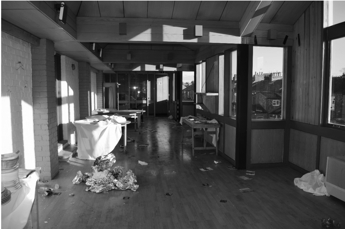
Plate 115. Main Stand: Interior Second Floor (DSC_0629). Facing North.
