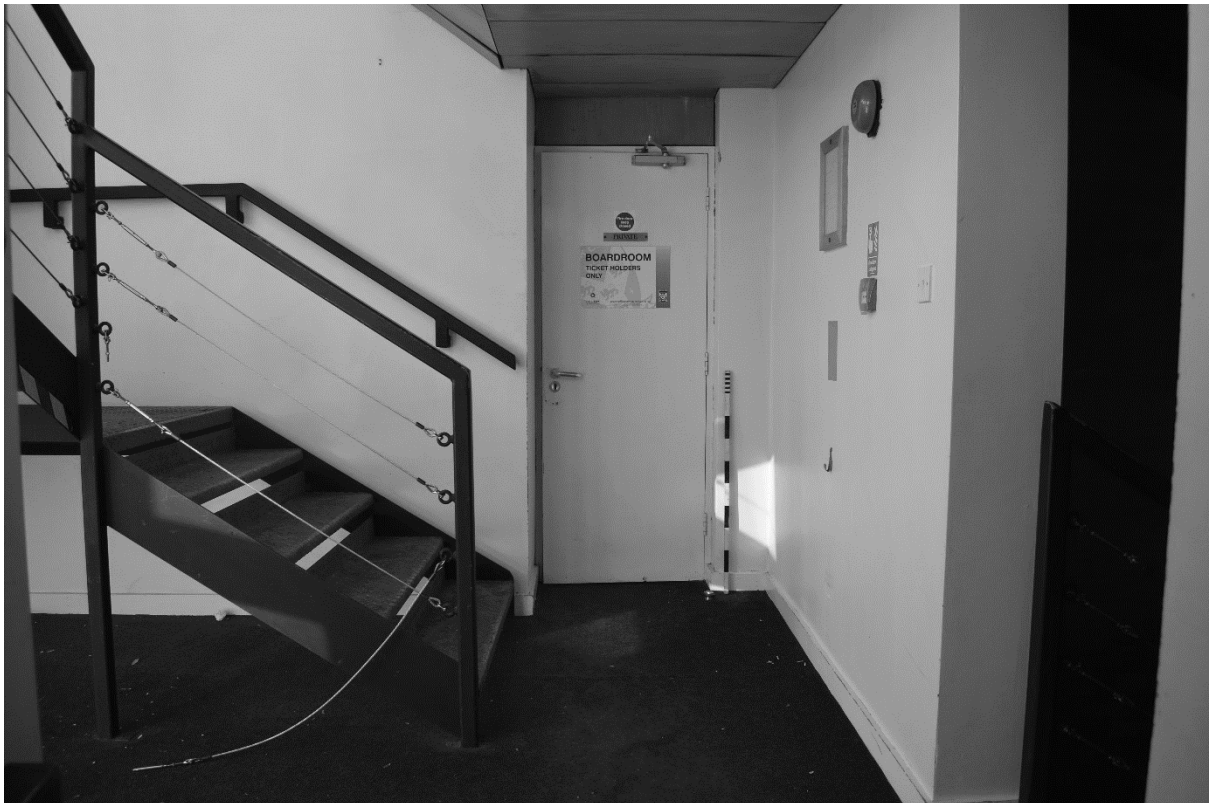
Plate 110. Main Stand: Interior First Floor (DSC_0637). Facing South
