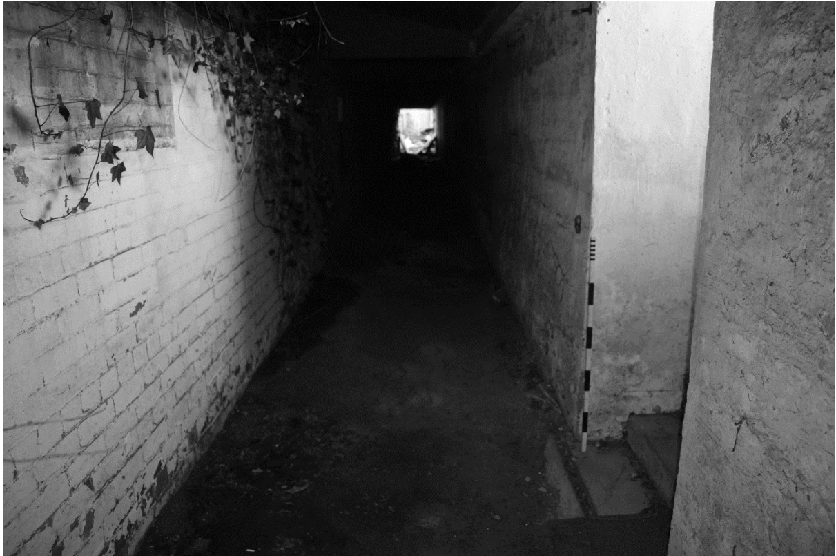
Plate 61. Popular Stand Tunnel (DSC_0686). Facing North.
