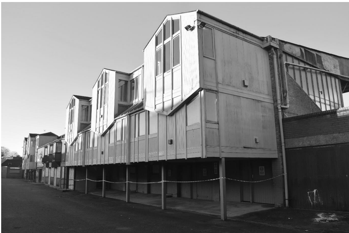
Plate 42. Main Stand: Exterior East and North Elevations (DSC_0718). Facing South-west.
