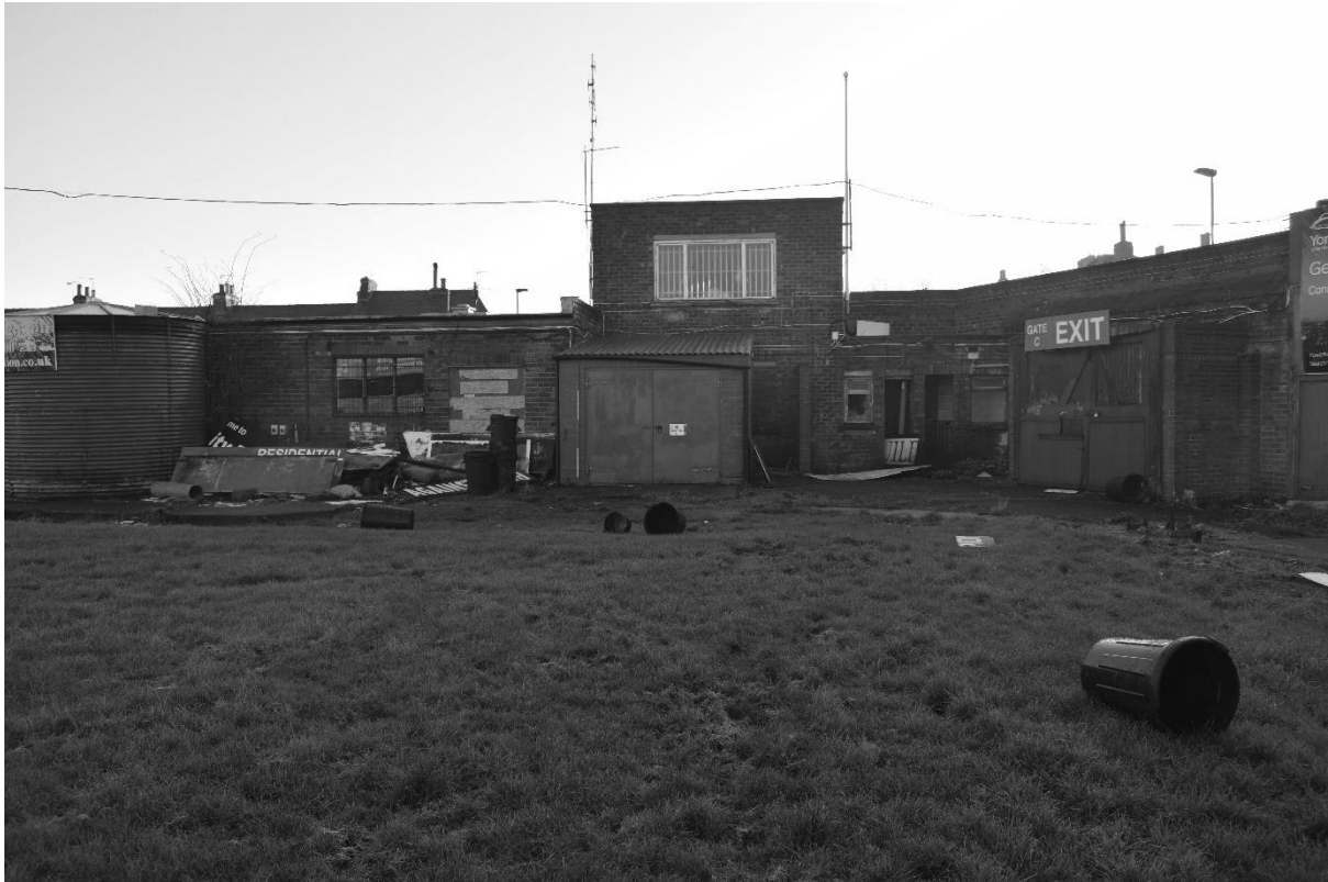
Plate 37. 1922 Bar: Exterior West Elevation (DSC_0726). Facing East.
