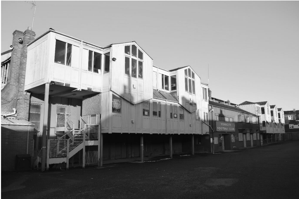
Plate 39. Main Stand: Exterior East Elevation (DSC_0714). Facing North-west.
