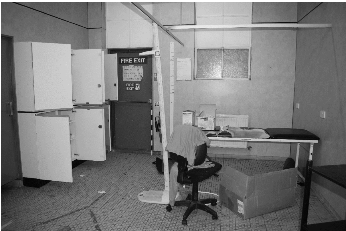
Plate 92. Main Stand: Interior Ground Floor (DSC_0647). Facing East.
