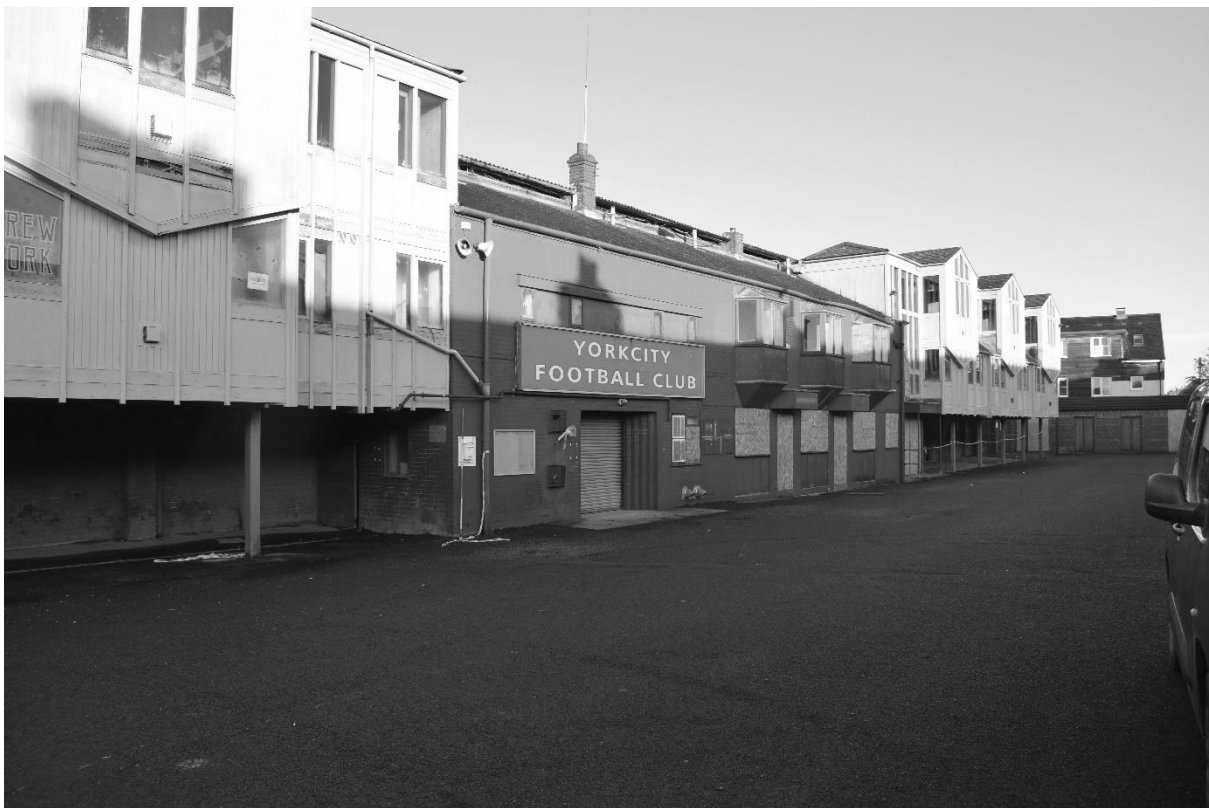
Plate 40. Main Stand: Exterior East Elevation (DSC_0715). Facing North-west.
