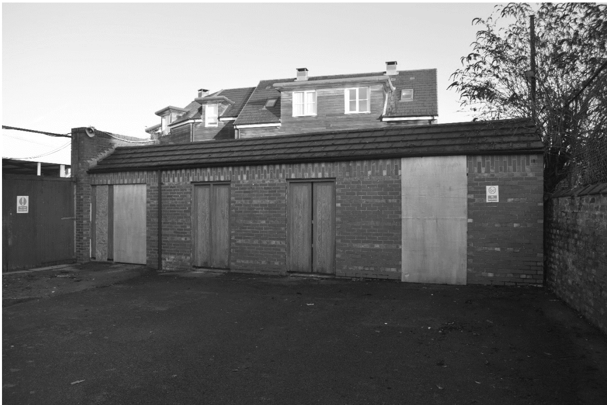
Plate 10. Entrances at north end of car park (DSC_0723). Facing North.
