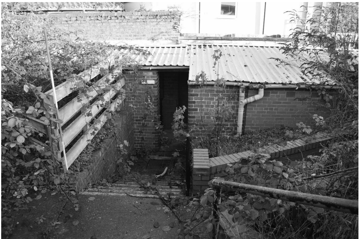
Plate 34. Toilet Block behinds David Longhurst Stand (DSC_0771). Facing North.
