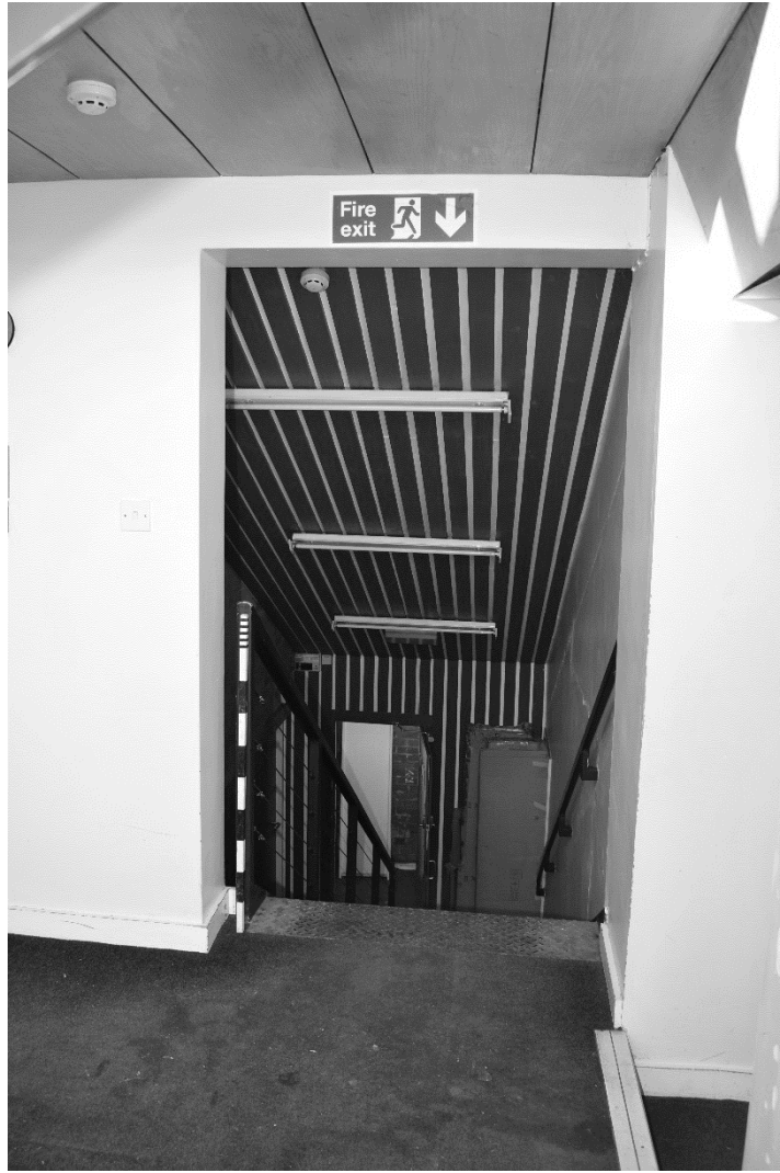
Plate 109. Main Stand: Interior First Floor (DSC_0635). Facing West.
