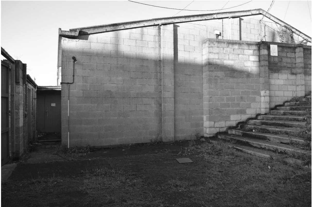
Plate 65. Gym: Exterior East Elevation (DSC_0739). Facing West.
