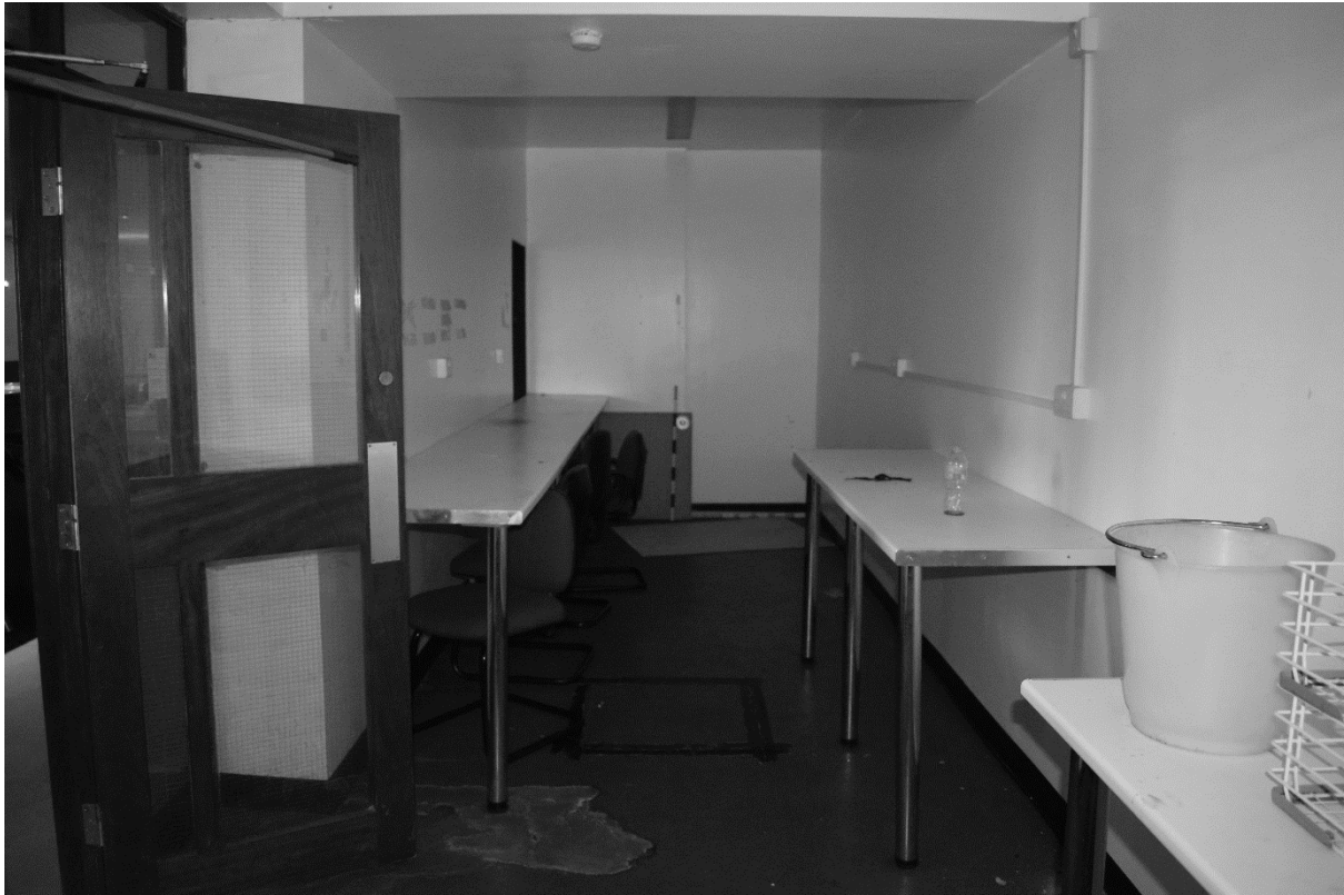
Plate 73. 1922 Bar: Interior Ground Floor (DSC_0579). Facing North.
