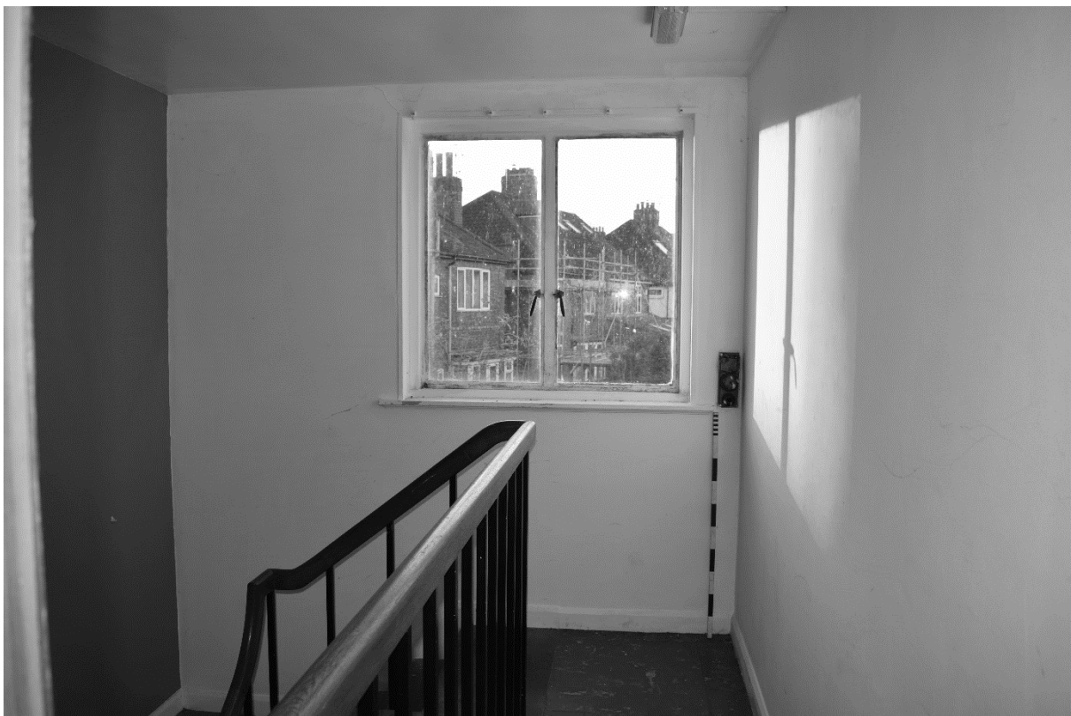
Plate 80. 1922 Bar: Interior First Floor (DSC_0593). Facing South-west.
