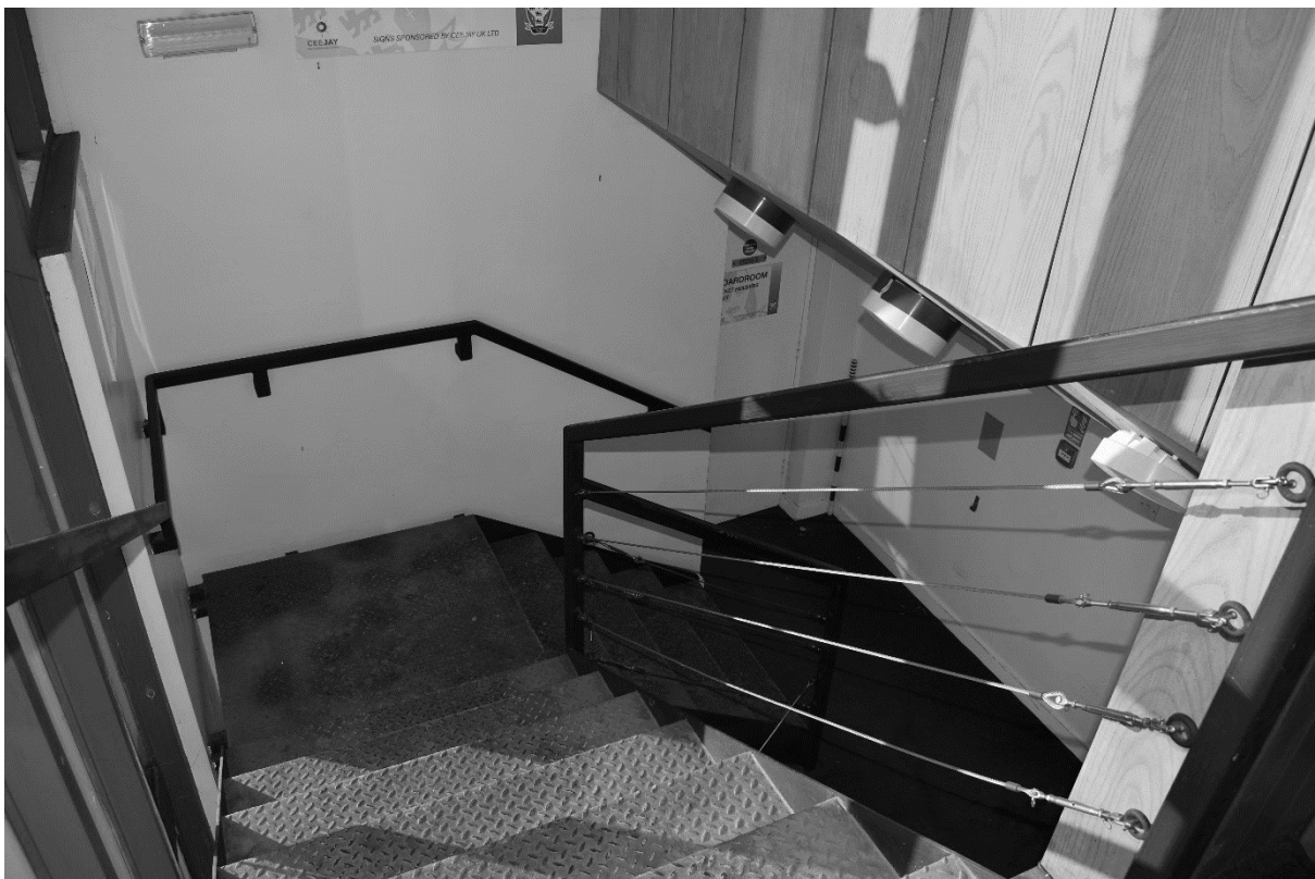
Plate 116. Main Stand: Interior Second Floor Stairs (DSC_0624). Facing North.
