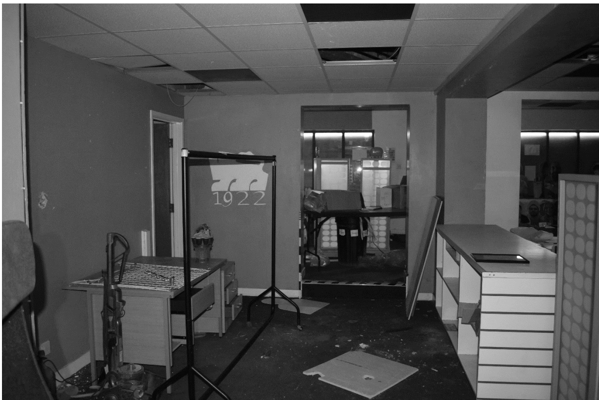
Plate 88. Club Shop: Interior (DSC_0603). Facing East.
