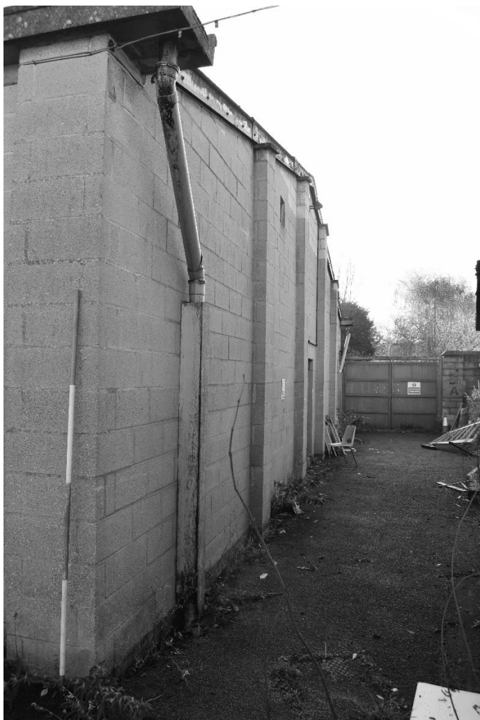
Plate 67. Gym: Exterior West Elevation (DSC_0788). Facing South.
