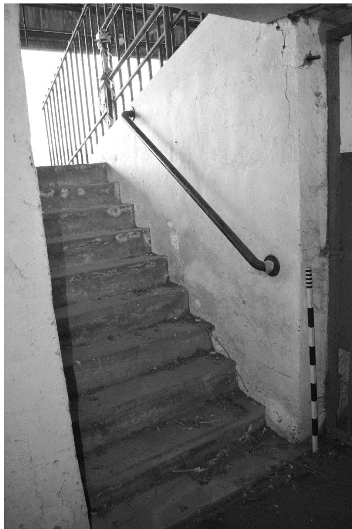
Plate 62. Popular Stand Tunnel Stairs (DSC_0685). Facing South-east.
