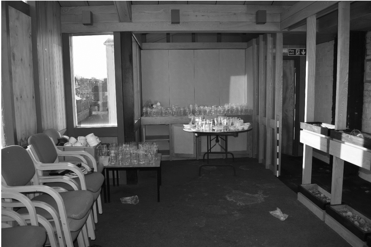
Plate 121. Main Stand: Interior Second Floor (DSC_0618). Facing South.
