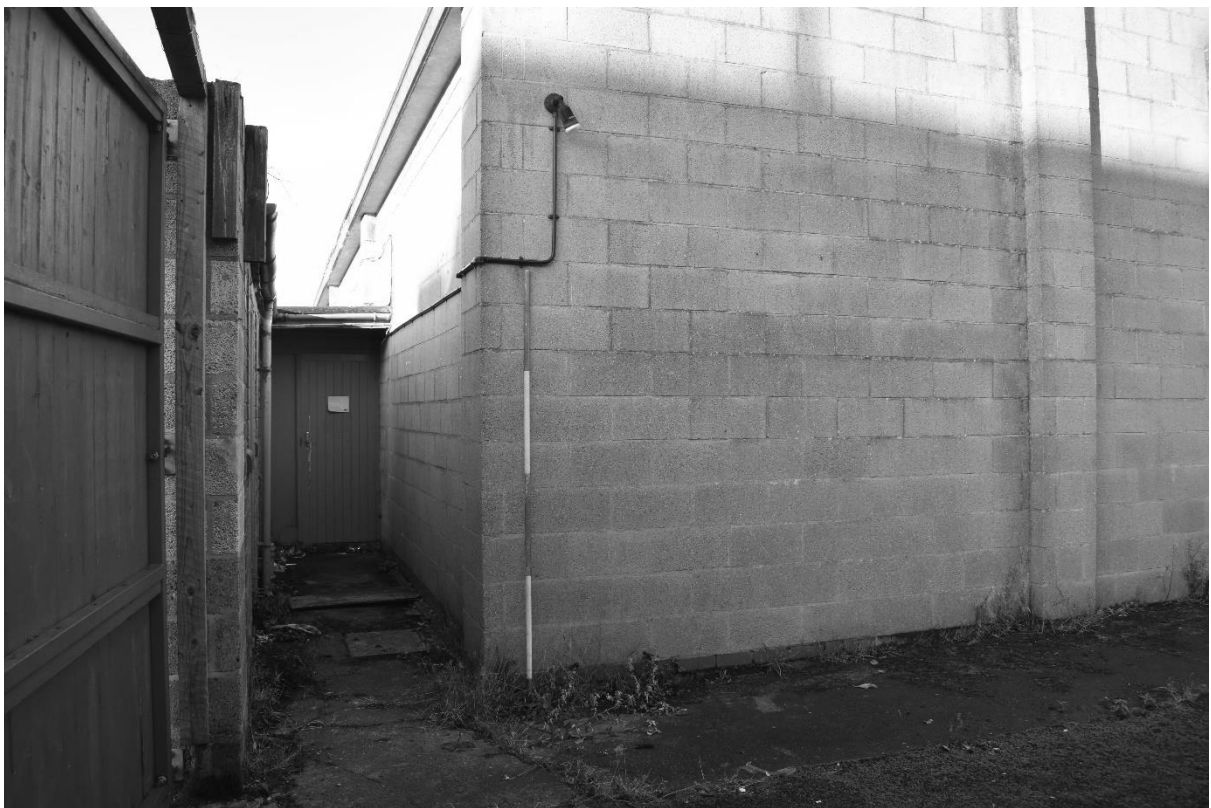
Plate 66. Gym: Exterior East and South Elevations (DSC_0741). Facing West.
