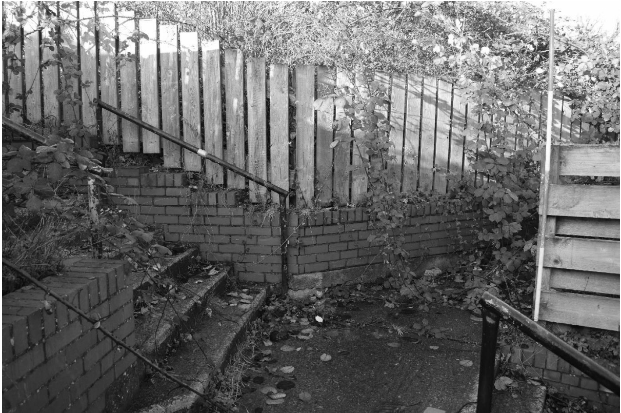
Plate 33. Access to rear of David Longhurst Stand (DSC_0770). Facing West.
