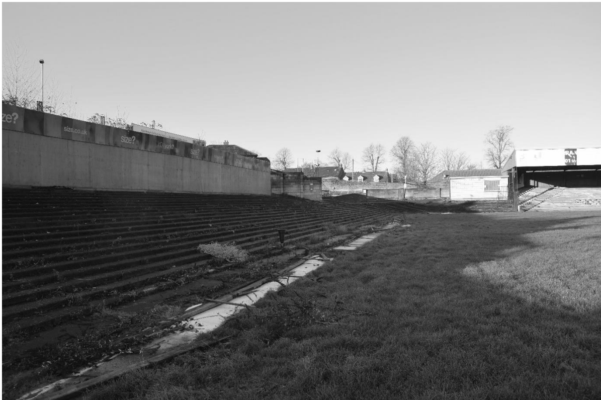
Plate 28. Grosvenor Road End (DSC_0734). Facing West.
