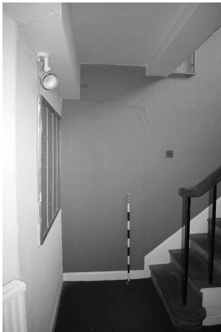
Plate 78. 1922 Bar: Interior Ground Floor (DSC_0589). Facing North-west.
