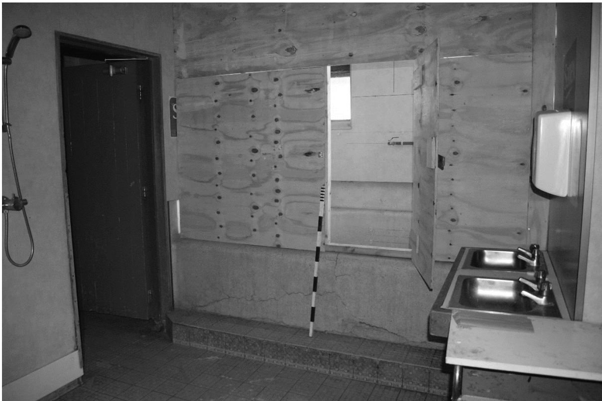
Plate 102. Main Stand: Interior Ground Floor (DSC_0669). Facing East.
