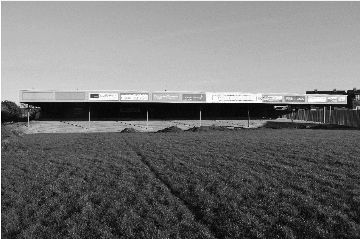
Plate 51. David Longhurst Stand: Exterior South Elevation (DSC_0764). Facing North.
