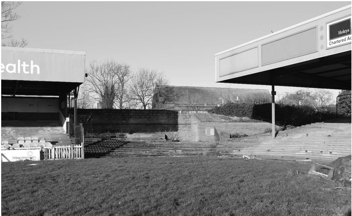
Plate 31. Terraces between the Popular and David Longhurst Stands (DSC_0775). Facing West.
