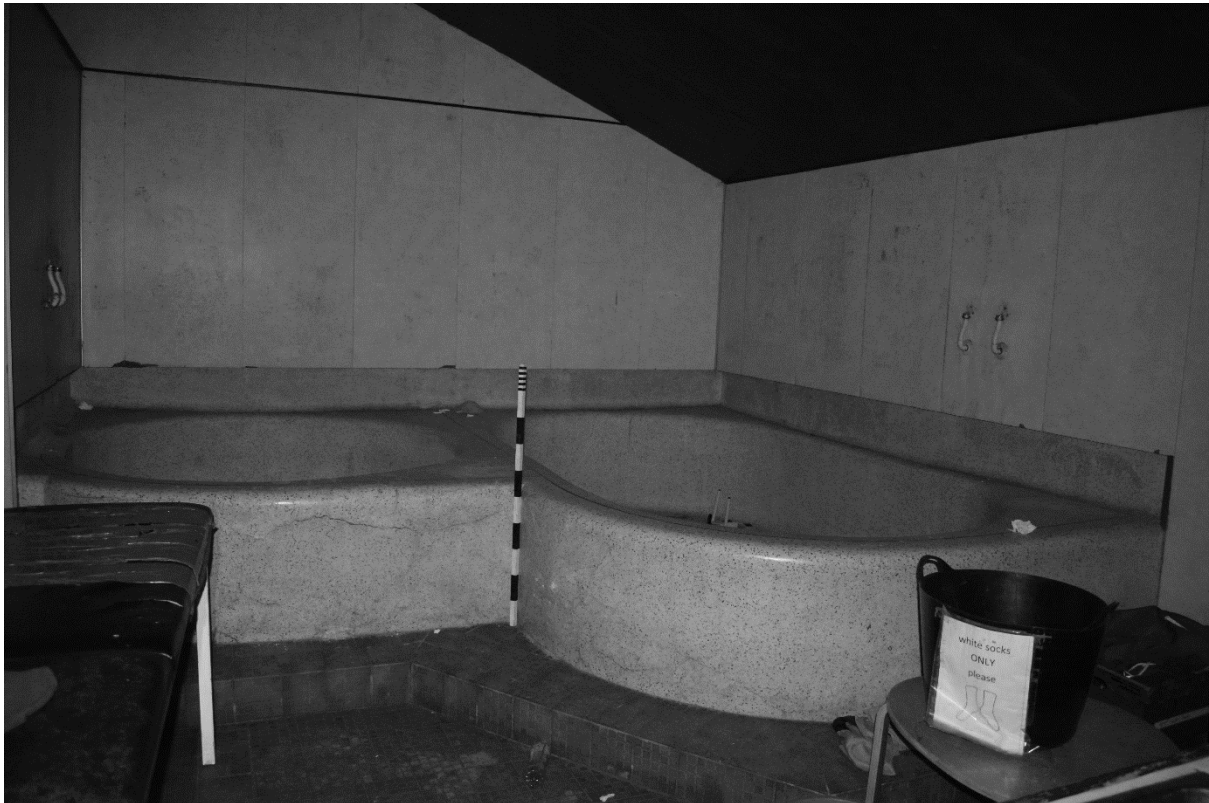
Plate 96. Main Stand: Interior Ground Floor (DSC_0661). Facing East.
