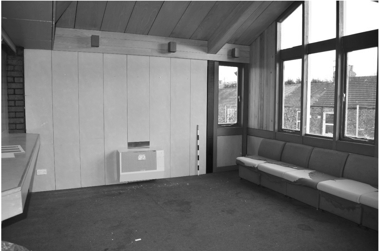
Plate 117. Main Stand: Interior Second Floor (DSC_0613). Facing South.
