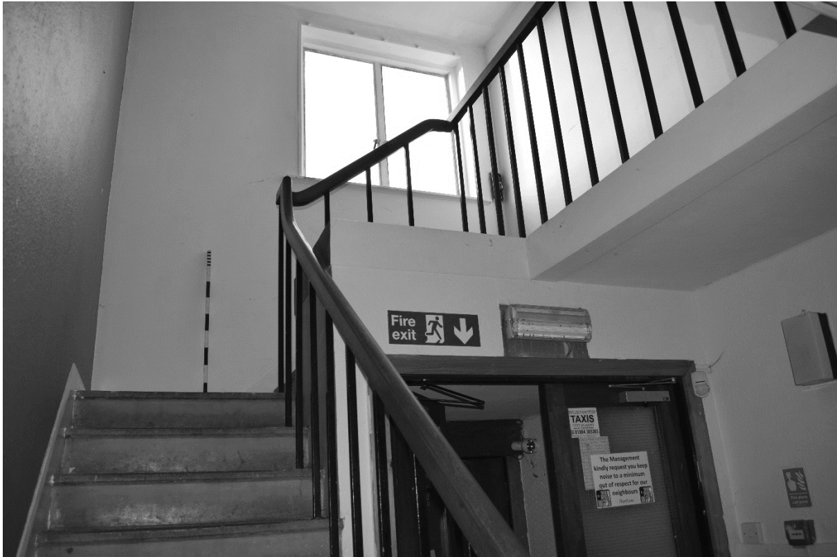
Plate 79. 1922 Bar: Interior Stairs (DSC_0590). Facing South-west.
