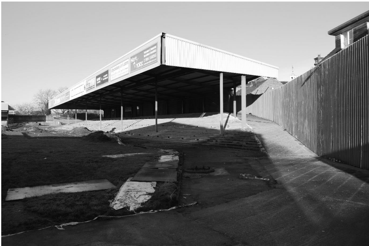
Plate 50. David Longhurst Stand: Exterior South and East Elevations (DSC_0761). Facing North-west.
