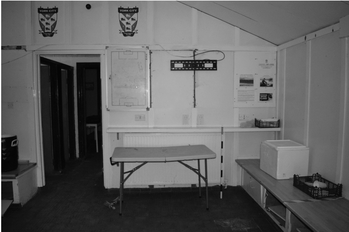
Plate 99. Main Stand: Interior Ground Floor (DSC_0665). Facing South.
