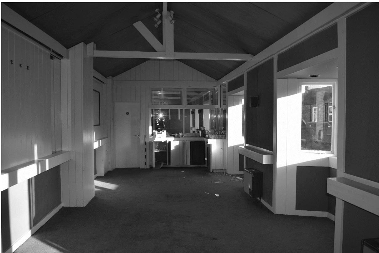
Plate 108. Main Stand: Interior First Floor (DSC_0634). Facing North.
