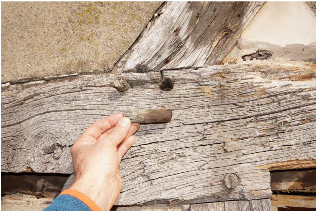
Plate 8: Joint between tie-beam 5 and the left gable brace 9 with later ornamental short peg
