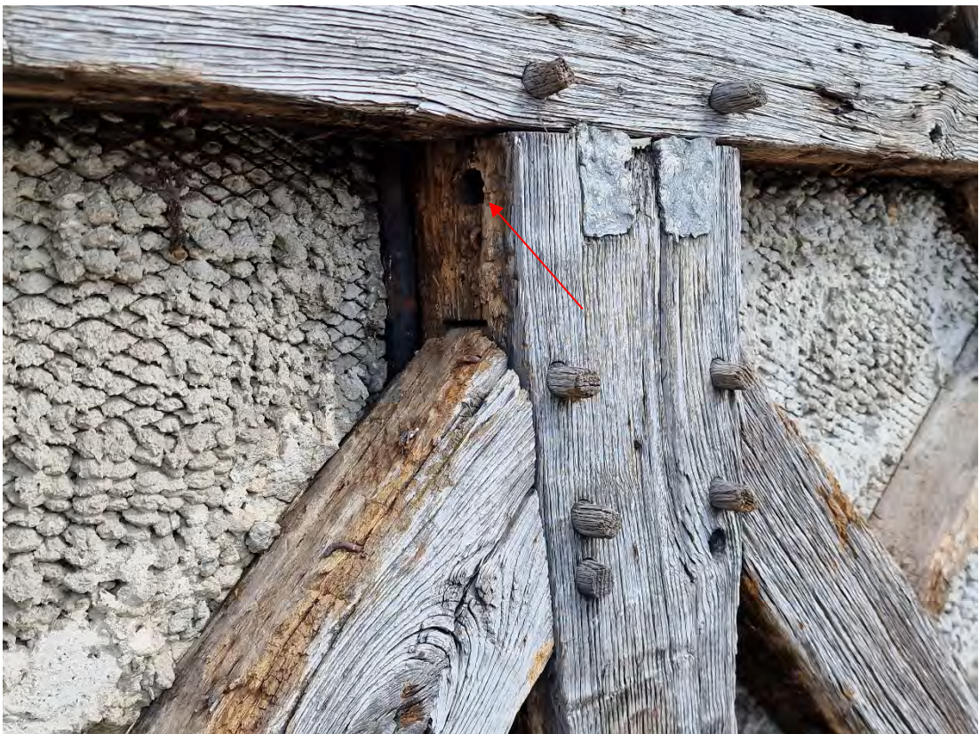
Plate 26: Crown post 15 with lead-filled mortices of former crown purlin and related empty peg hole (arrow)
