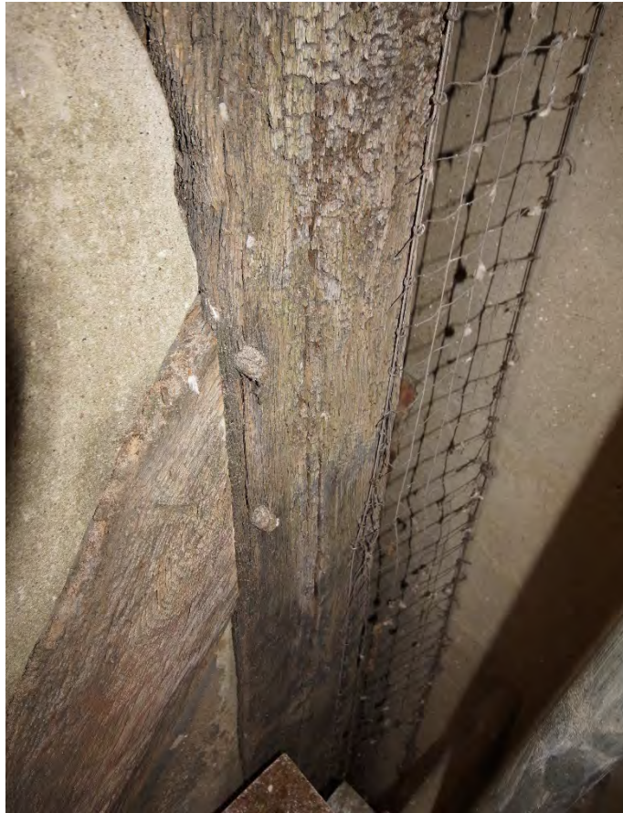
Plate 21: Joint between post 2 and first-floor brace 25 with pegs
