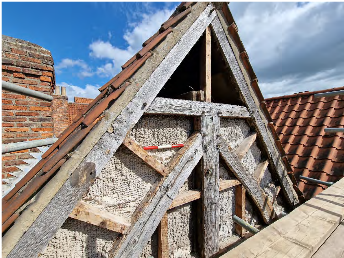
Plate 24: Gable with partially removed infill panels
