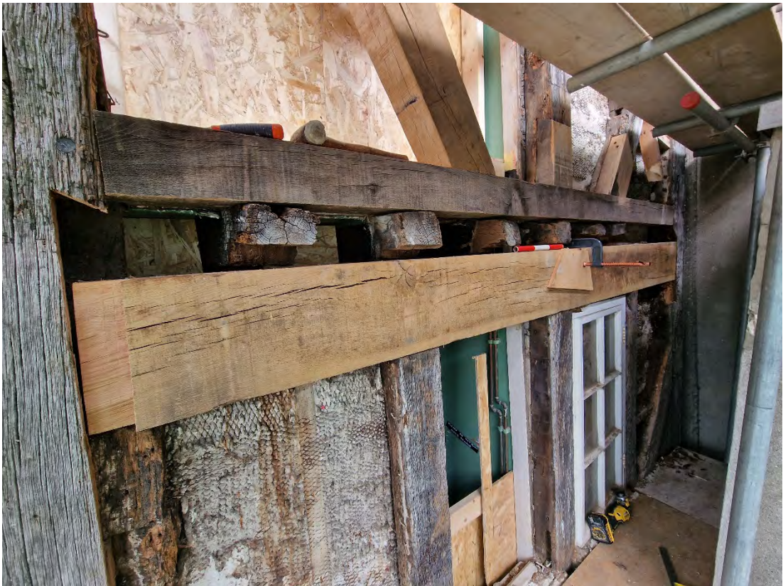
Plate 38: Replaced beam 7 and second-floor joist 26
