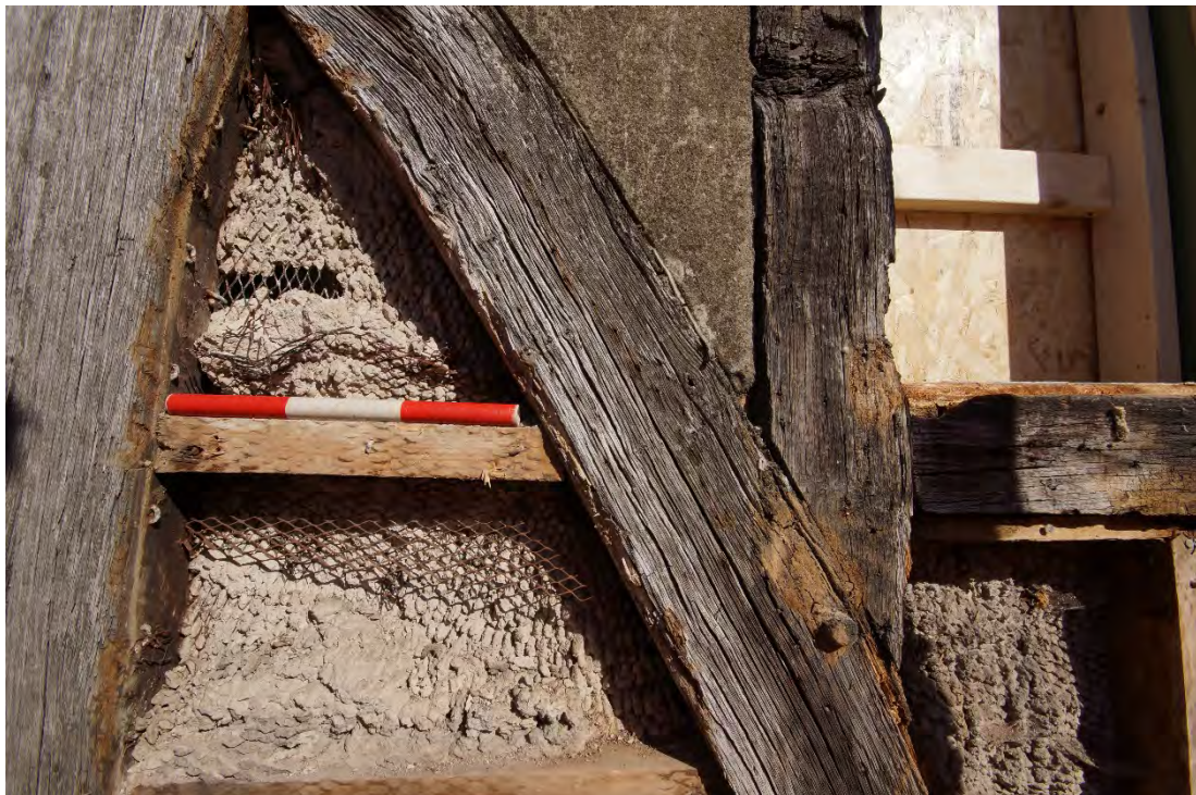
Plate 14: Detail of partially removed infill panels between post 1 and second-floor brace 11
