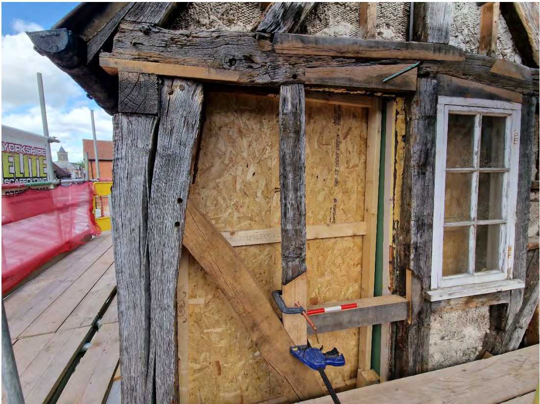
Plate 34: Jowl post 1 with iron bracket attached to the underside of tie-beam 5
