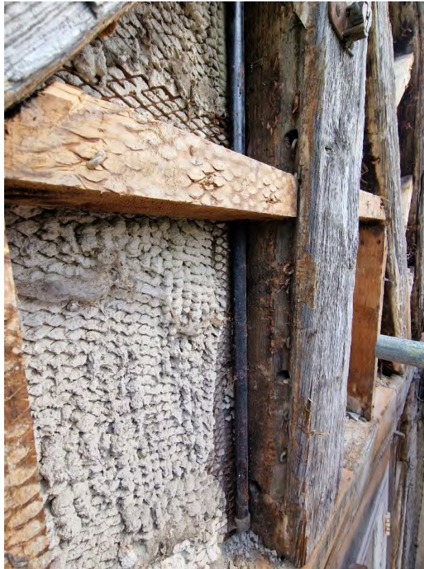
Plate 29: Southwest face of the crown post 15 with stave groove and empty peg holes
