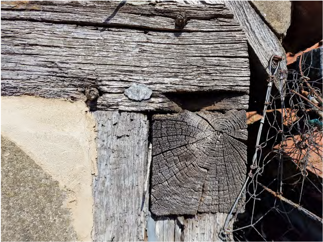
Plate 11: Detail of partially decayed upper section of the wall plate and dovetail mortise above it
