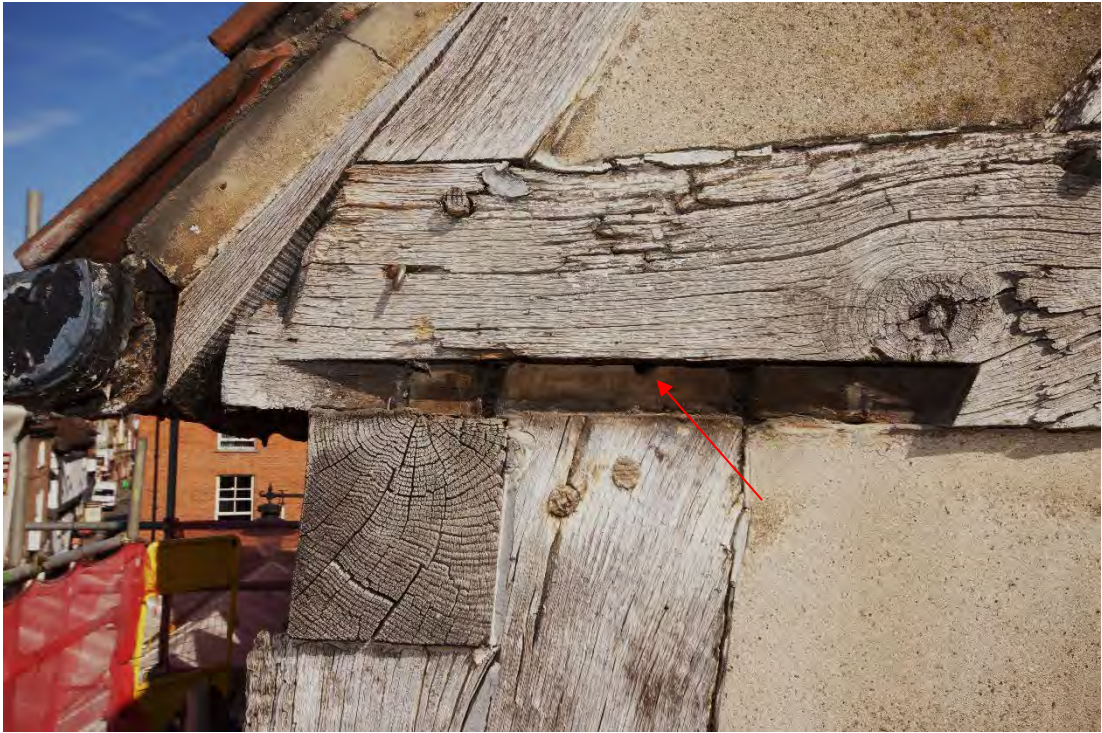
Plate 7: Removed splice revealing a teazle tenon of jowl post 1 with empty peg hole (arrow)
