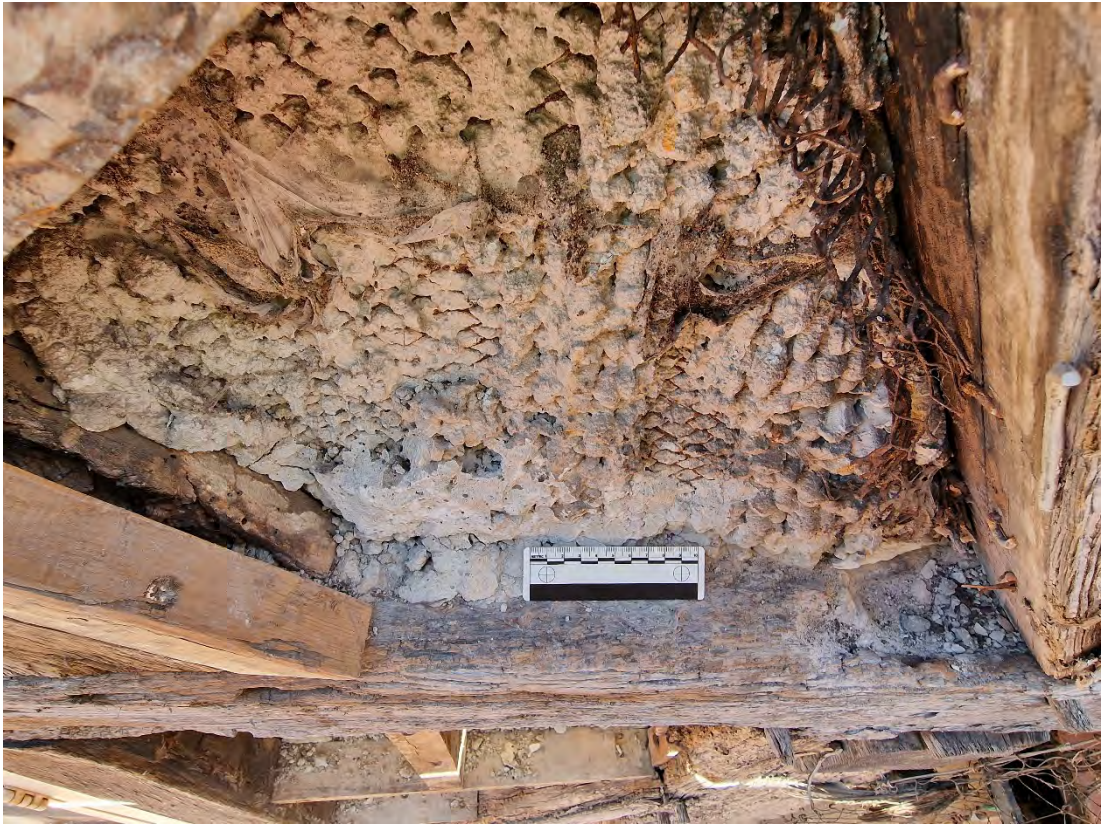
Plate 33: Tie-beam with partially filled-in mortice for rafter 4
