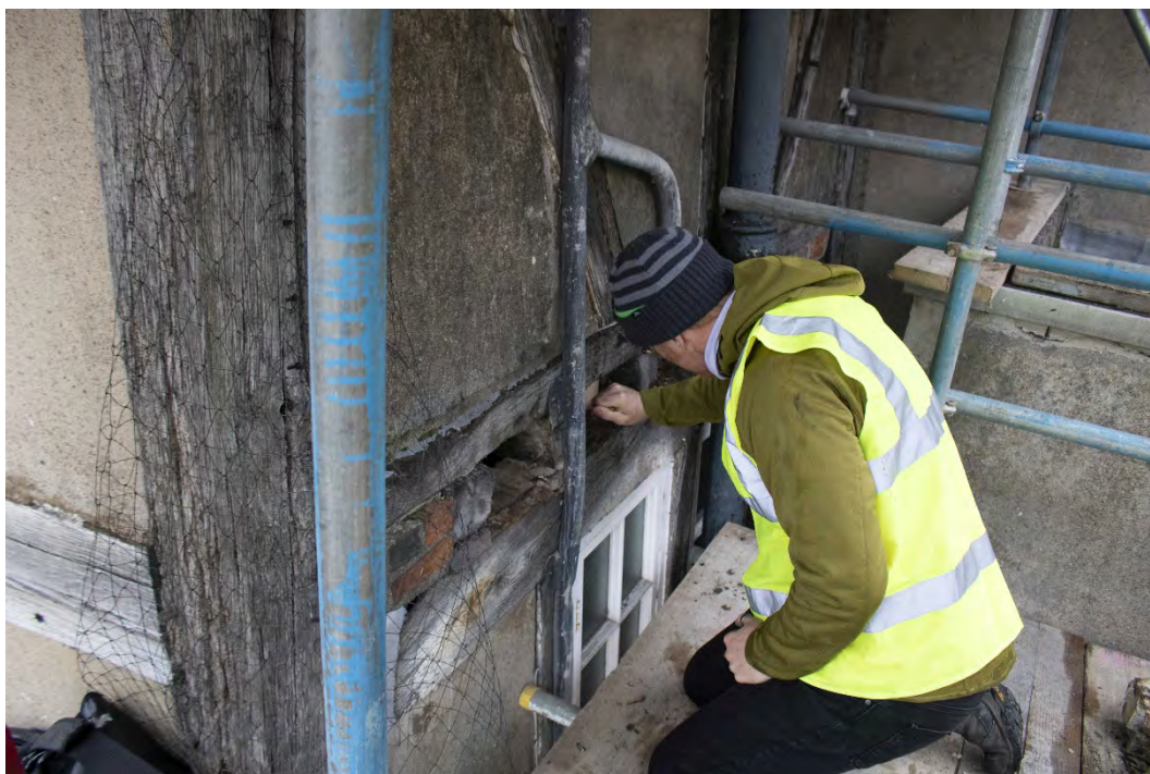
Plate 1 Inspection of timber frame, facing north
