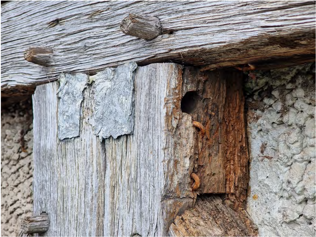
Plate 27: Detail of empty peg hole of former crown purlin within the right lateral side
