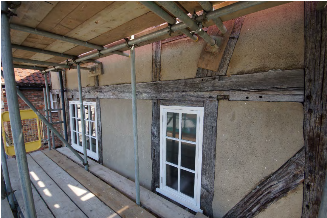
Plate 22: First-floor level of the southwest side elevation with reused girthing beam
