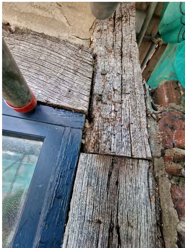
Plate 48: Detail of truncated post 1
