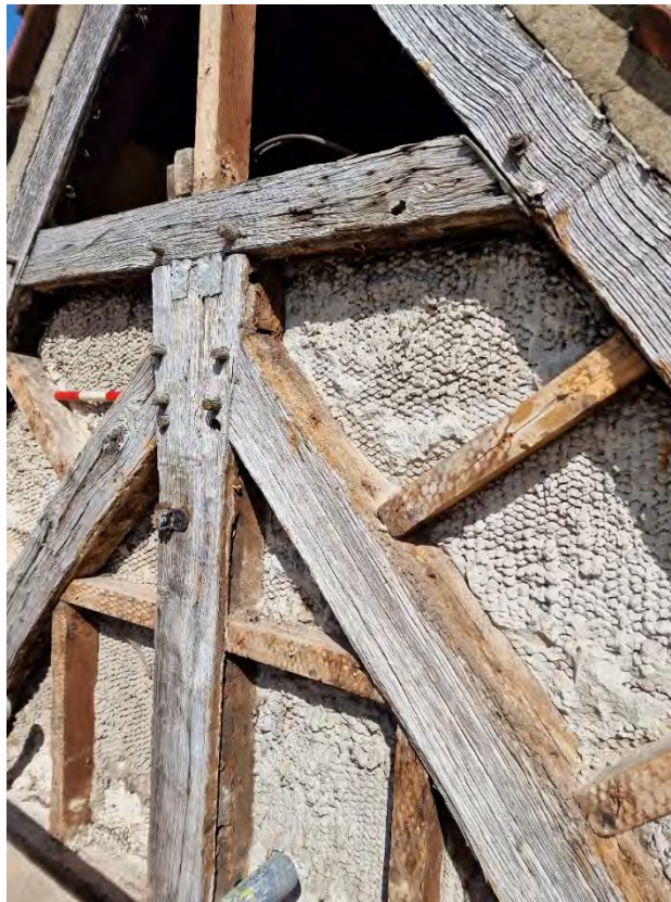
Plate 30: Northeast face of the crown post 15 with stave groove and empty peg holes
