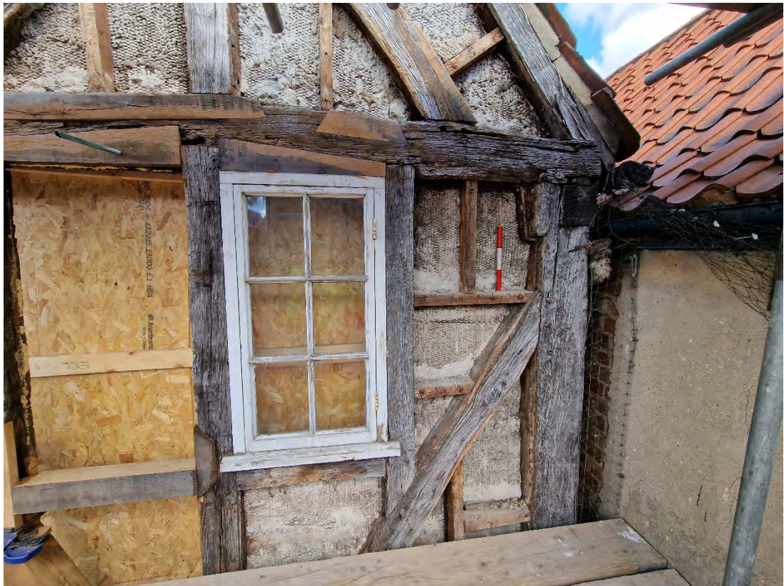
Plate 36: Post 2 with iron bracket attached to the underside of tie-beam 5
