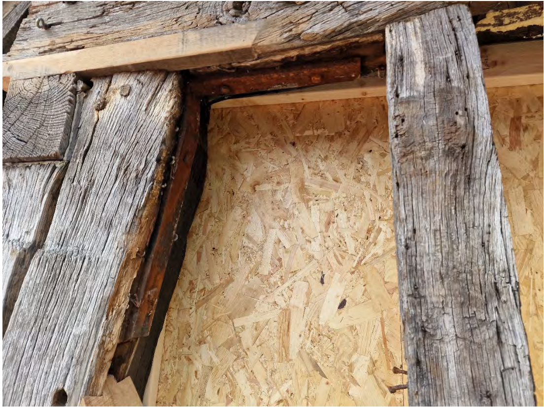
Plate 35: Detail of iron bracket attached to post 1 and tie-beam 5
