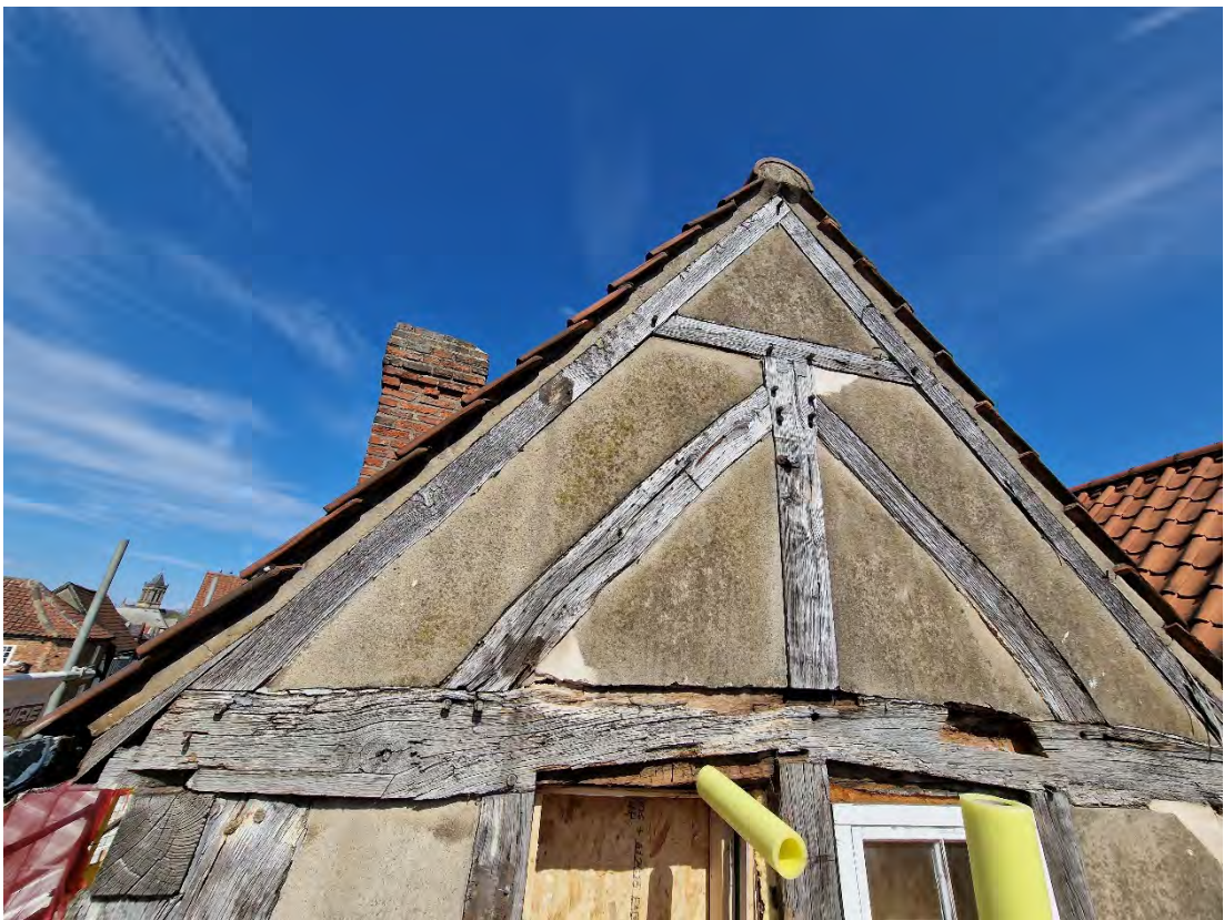
Plate 6: Southeast gable truss with removed splices within the tie-beam 5
