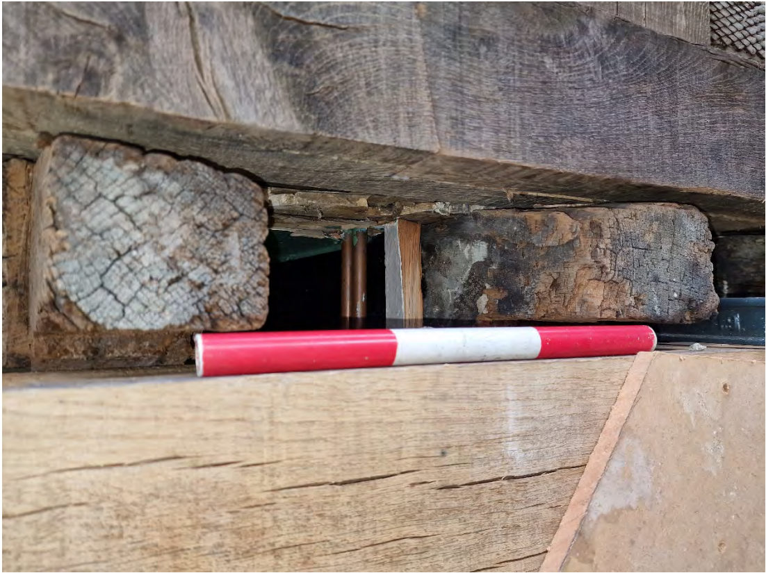
Plate 39: Floor joists 26 with plaster ceiling above them
