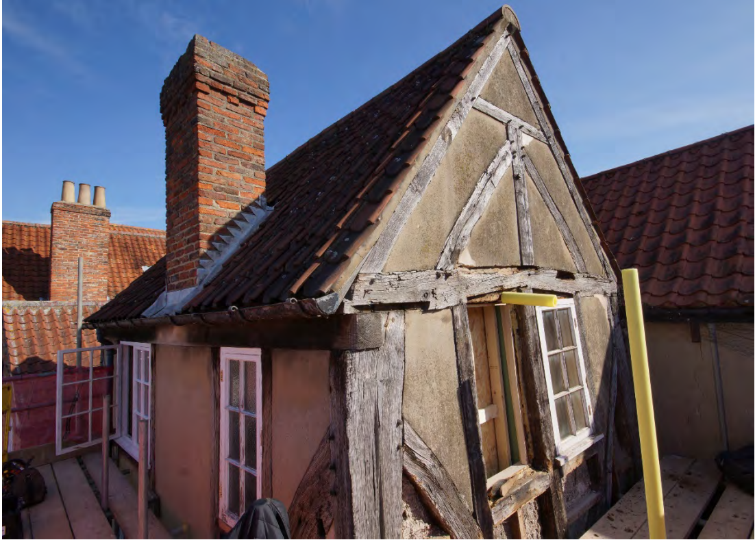
Plate 5: General view of the second-floor level during the recent repair work
