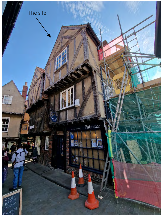
Plate 1: Front façade of the site at 1 Little Shambles, York
