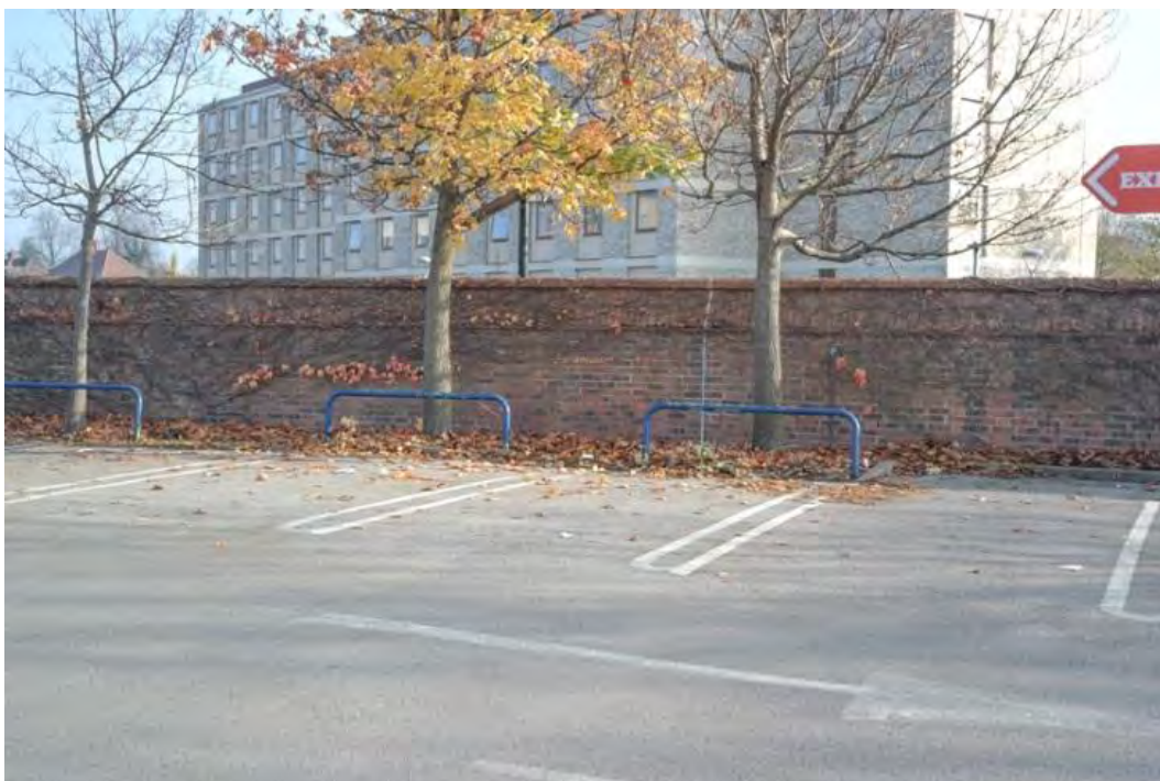
Plate 41 Metal crash barriers adjacent to the south-western car park boundary wall, facing east
