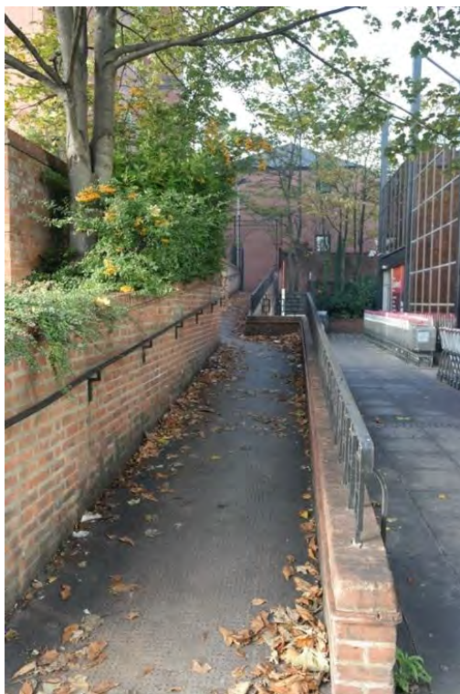
Plate 24 Disabled access ramp adjacent to the County Hospital, facing north-west
