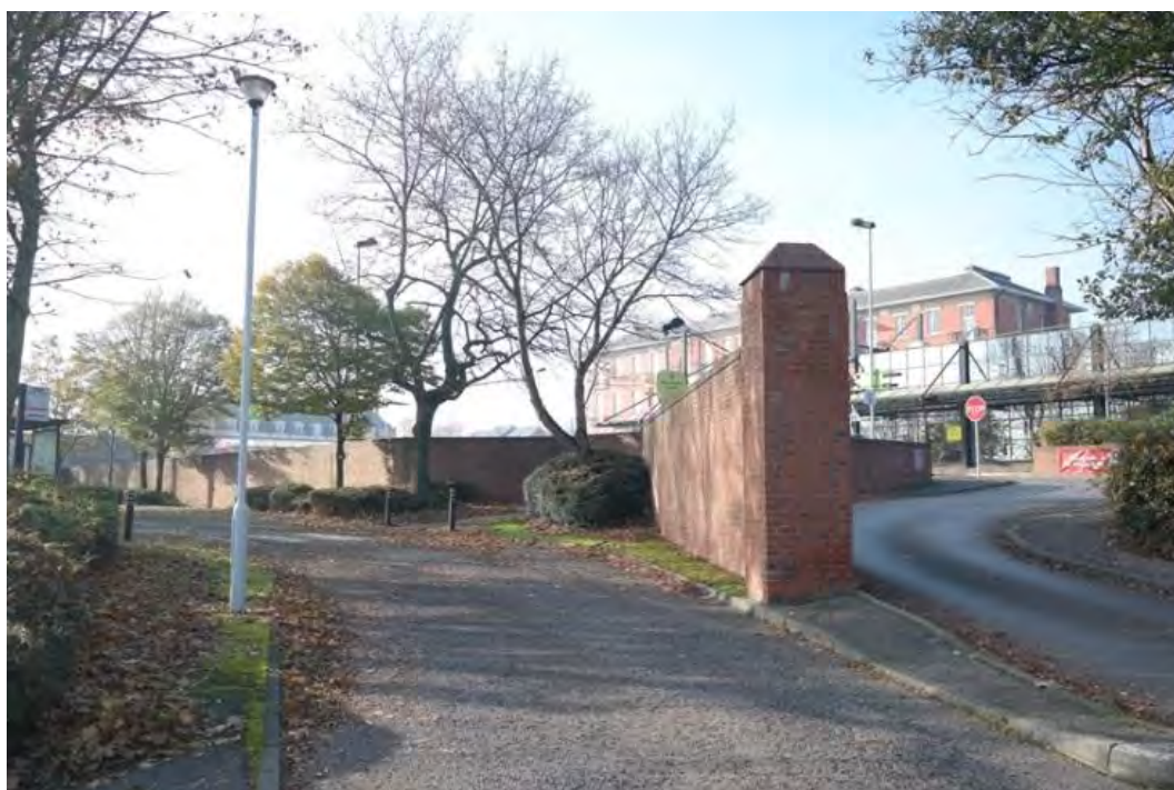
Plate 47 The entry to the bus layby, facing south-west
