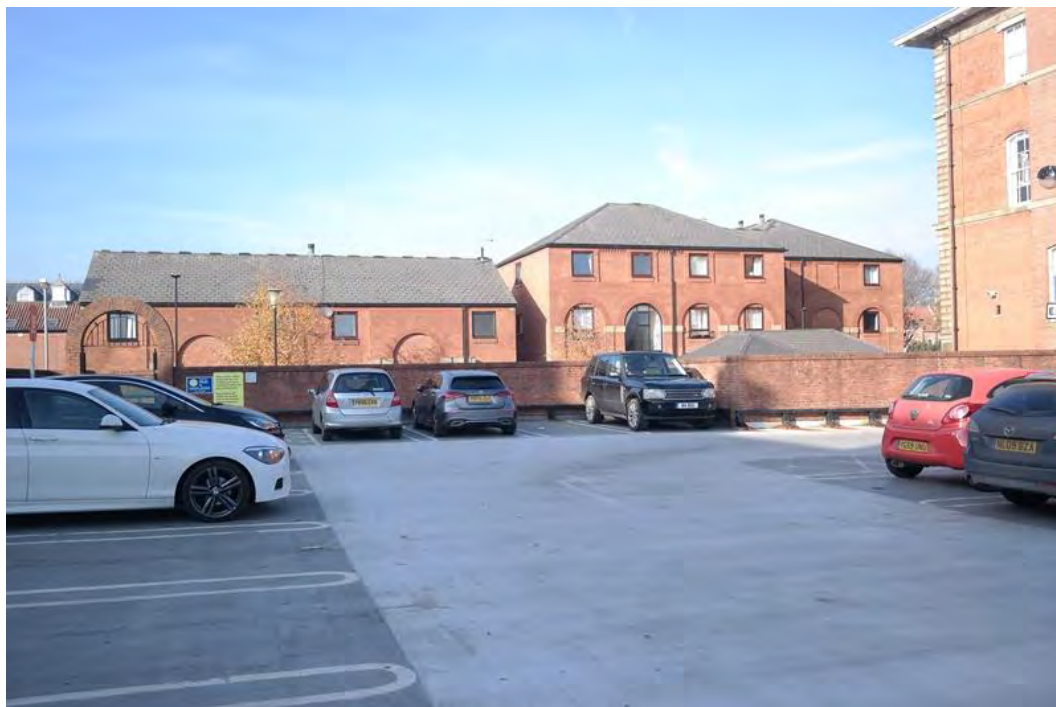
Plate 82 The brick wall around the north-western side of the upper floor of the two-storey car park, facing north-west
