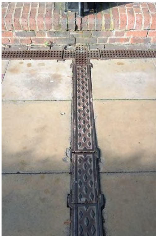
Plate 44 Drains in the pavements of Plot A, facing north-west
