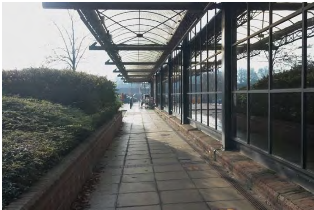
Plate 28 The covered walkway around the Sainsbury's store, facing south-west
