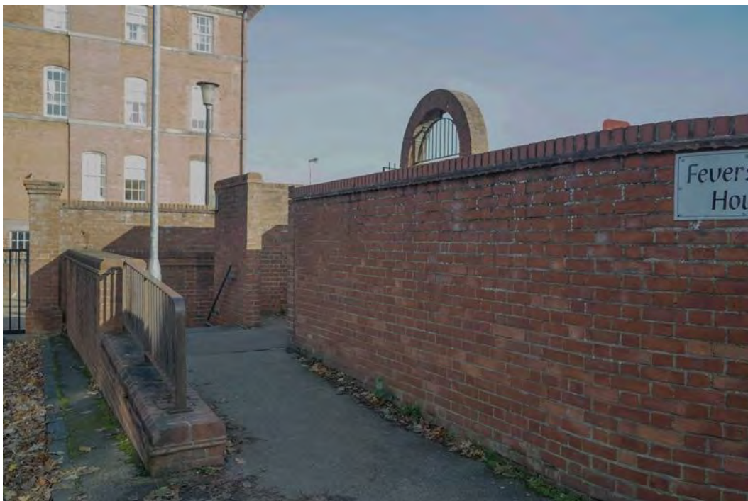
Plate 76 The ramp leading to pedestrian access to the upper floor of the car park on the north-western side, facing north-east
