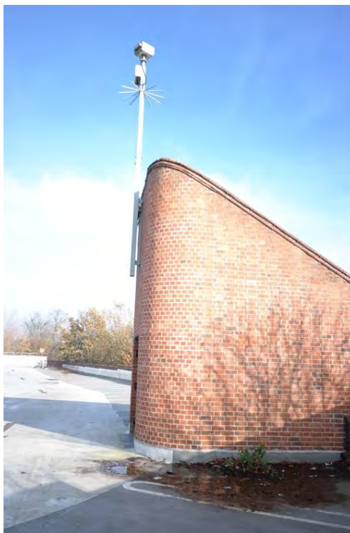
Plate 72 The brick stairwell giving access between the various floors of the three-storey car park, facing north-east
