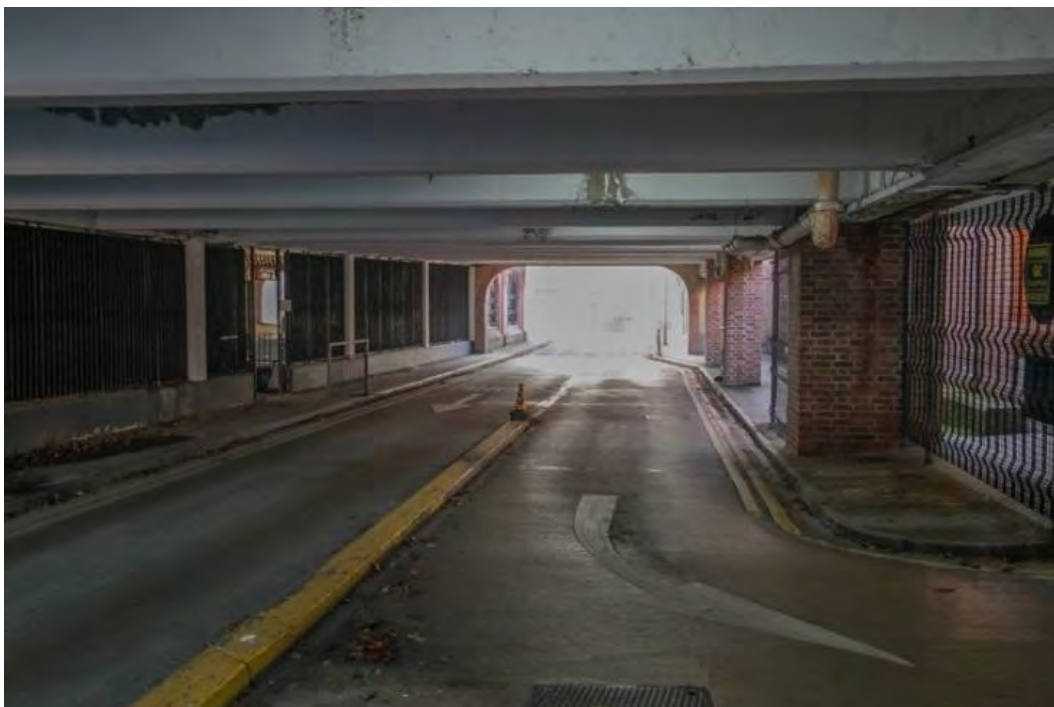
Plate 54 The entry road within the car park, facing south-west
