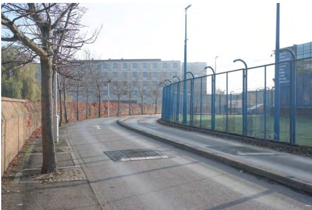
Plate 21 The access road into the car park at the northern end of the site, facing south-east
