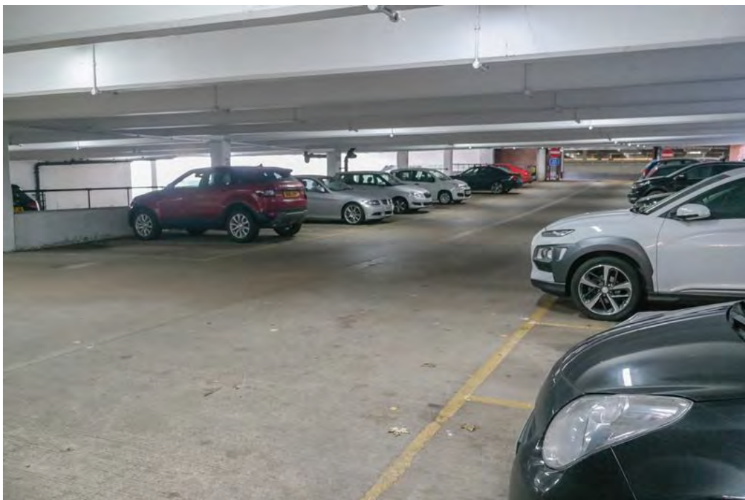
Plate 78 The south-western portion of the ground floor of the two-storey car park, facing south-east
