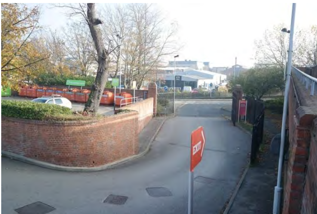
Plate 33 The slope for the car park exit onto Foss Bank and the brick retaining wall, facing east
