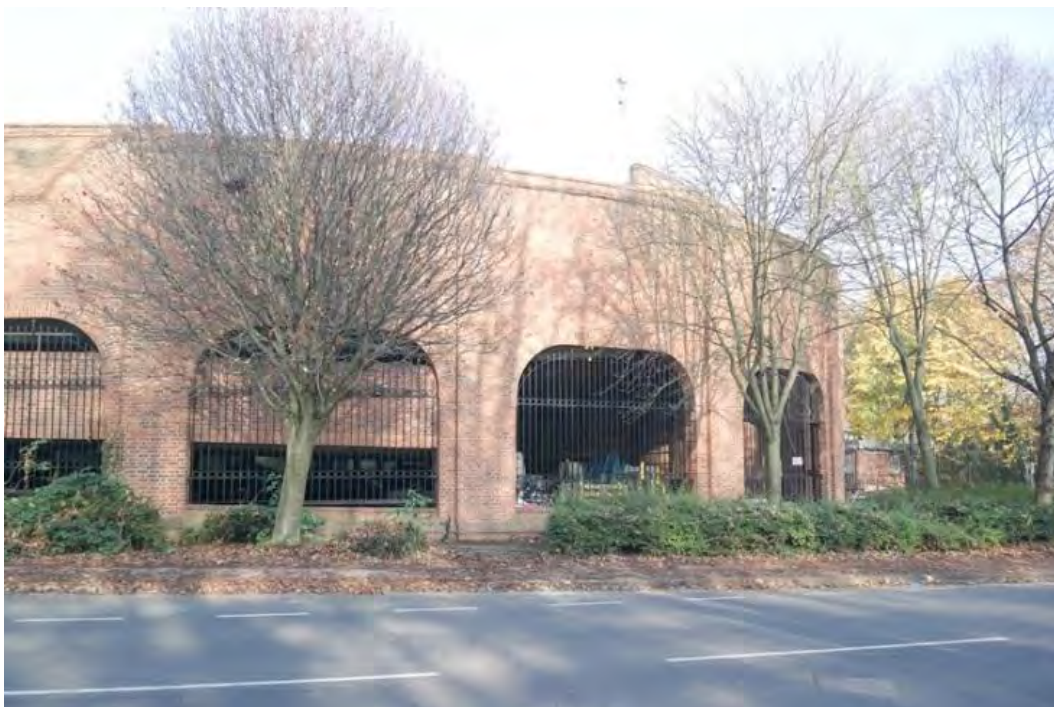
Plate 56 The south-eastern façade of the multi-storey car park, facing north
