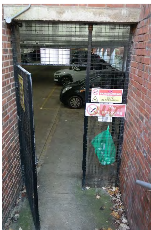
Plate 75 The lower part of the pedestrian access into the ground floor of the car park on the north-western side, facing south-east
