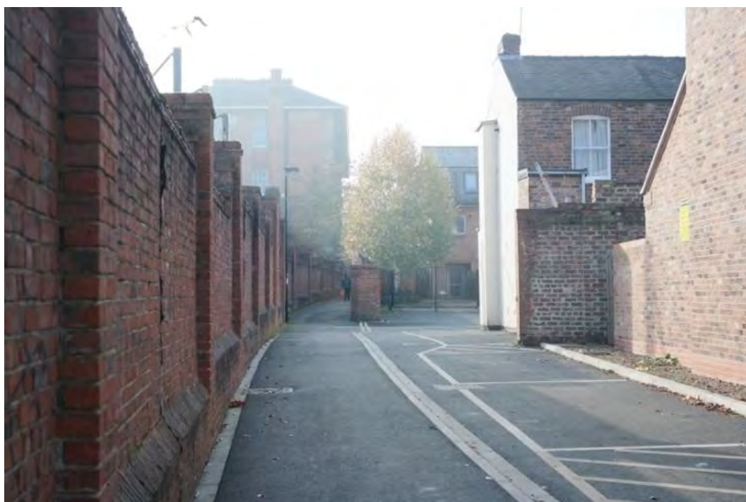
Plate 11 Love Lane facing south-west showing the ends of properties fronting onto St Wilfrid's Court and Agar Street
