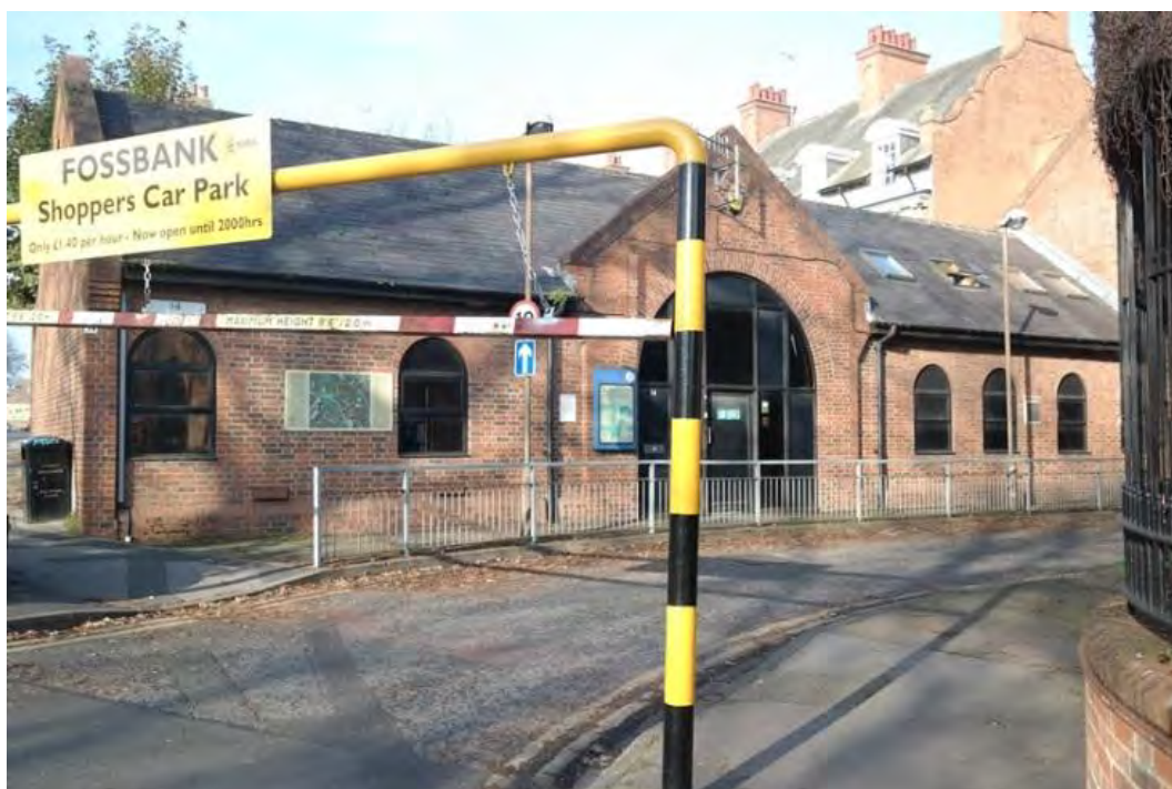
Plate 51 The building at the north-western side of Plot B, facing north
