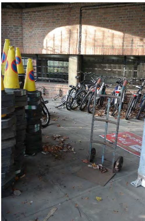
Plate 61 The small room at the southern end of the ground floor of the three-storey car park, facing north-west
