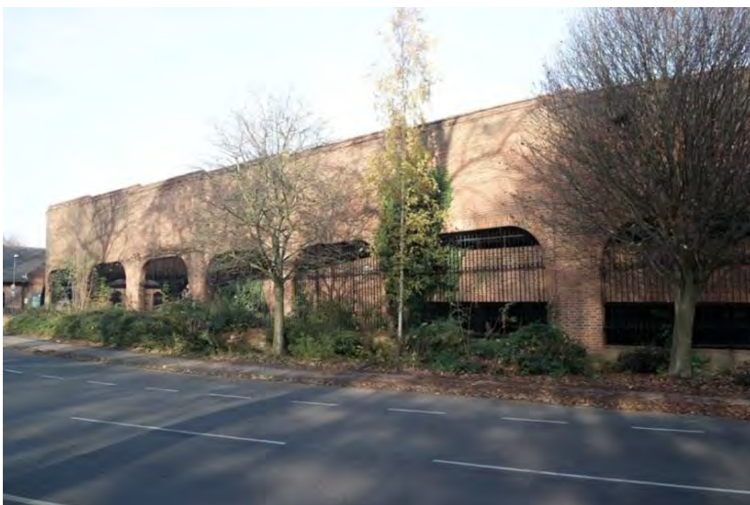
Plate 55 The south-western façade of the multi-storey car park, facing north-east
