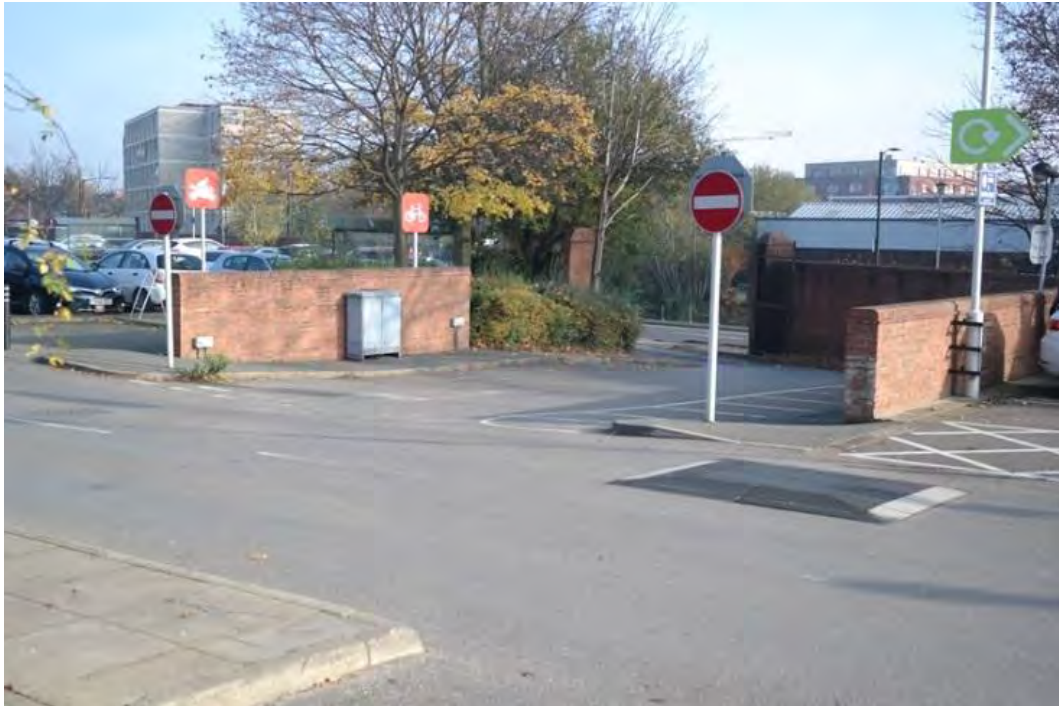
Plate 30 The entry ramp into the car park mid-way along the south-eastern side of Plot A, facing east
