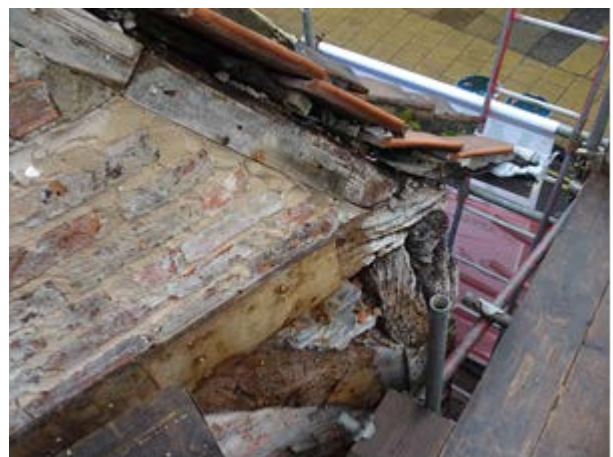
125 - LHS elevation – exposed timbers and previous repairs
