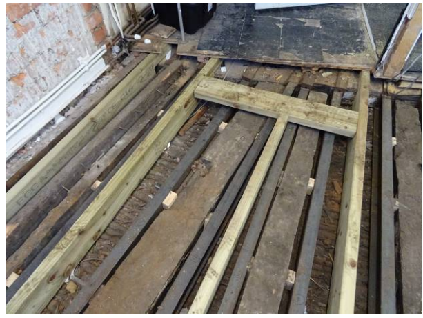
135 - Internals – First floor channel steel sections
