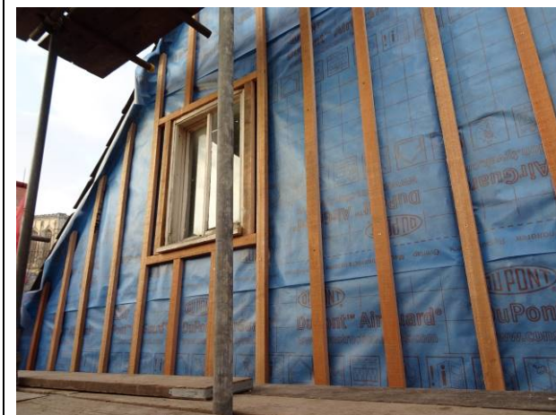
192 - New breather membrane and timber battens installed
