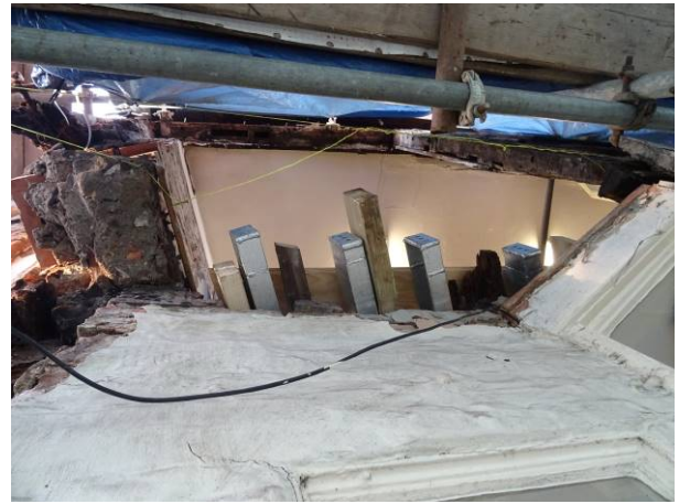
183 - Underside of the jetty structure
