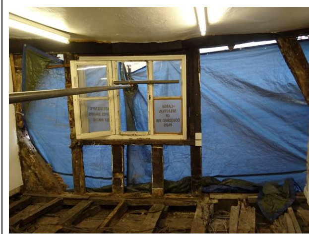
90 - Internals – structure at first floor level including exposed timbers
