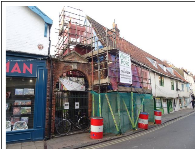
184 - Scaffold in place
