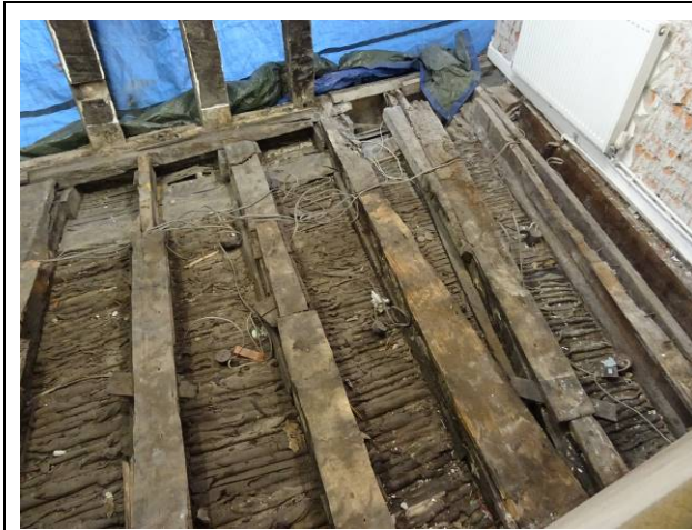
88 - Internals – structure at first floor level including exposed joists
