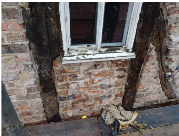
118 - LHS elevation – exposed timbers
