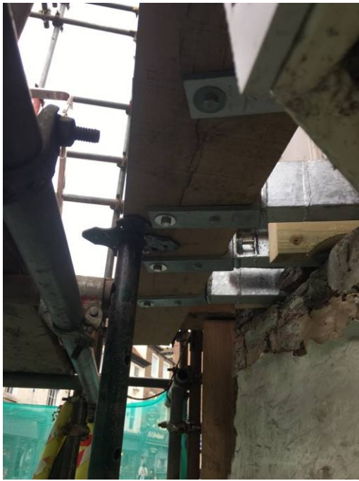
180 - Open construction to underside of jetty structure
