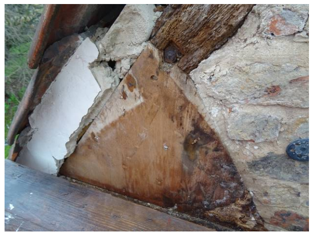
117 - LHS elevation - exposed timbers and previous repairs
