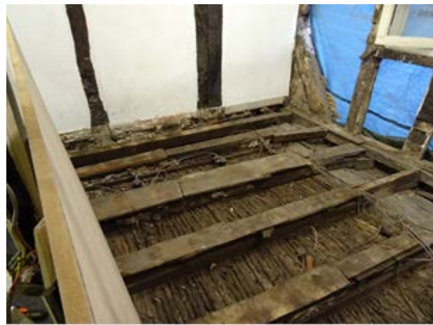
91 - Internals – structure at first floor level including exposed joists
