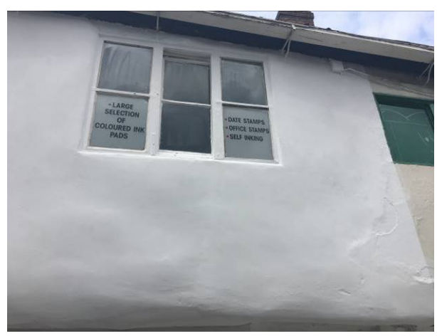
216 - Finished render at front elevation
