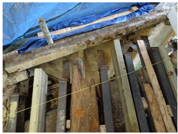
137 - Internals – First floor structural reinforcements with sole plates
