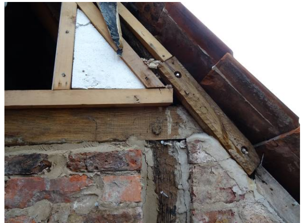
121 - LHS elevation – exposed timbers and previous repairs
