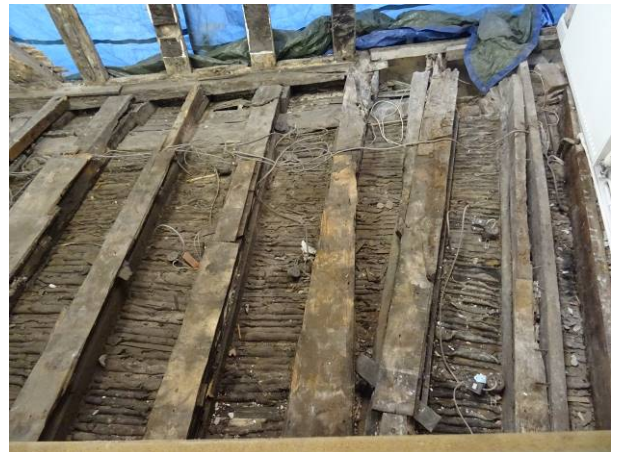
89 - Internals – structure at first floor level including exposed joists
