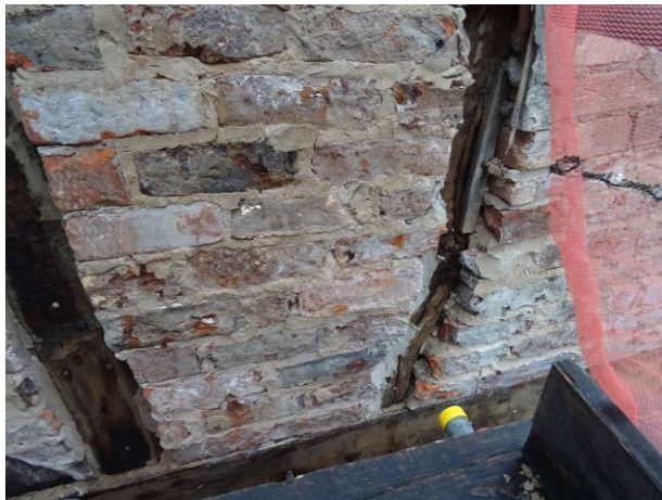
120 - LHS elevation – exposed timbers
