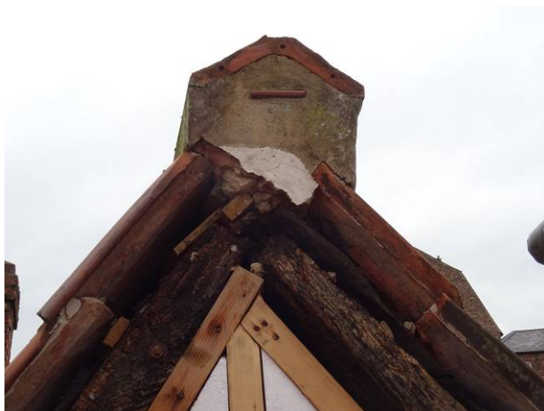
124 - LHS elevation – exposed timbers at roof apex
