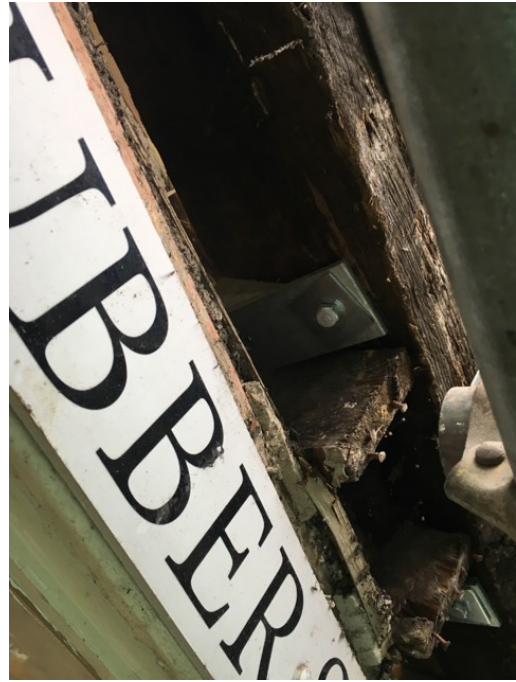
173 - Under side of jetty structure showing sole plates
