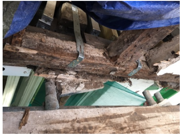
171 - New straps installed to the front of the property to tie into the structure
