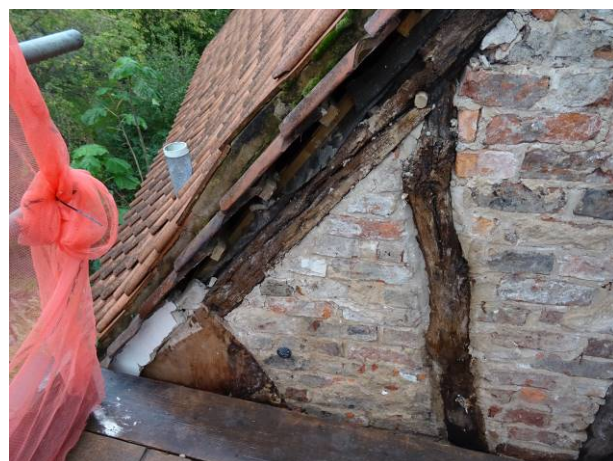
113 - LHS elevation - exposed timbers and previous repairs
