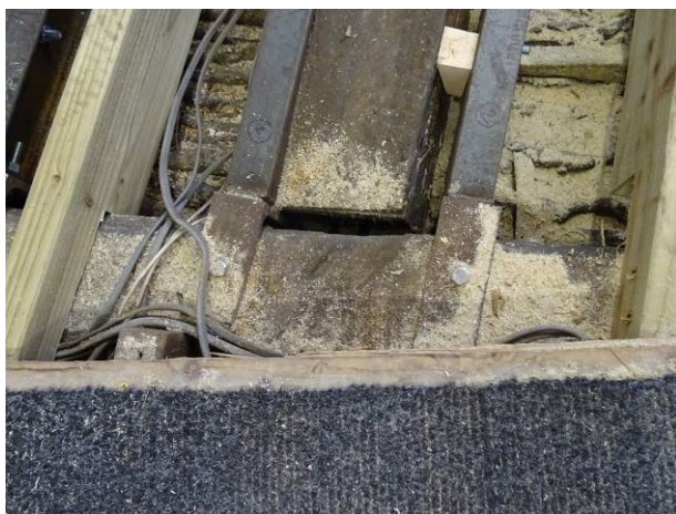
142 - Internals – First floor structural reinforcements / channel steel sections in pairs
