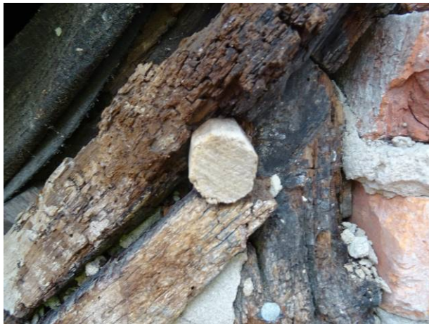
114 - LHS elevation - exposed timbers and previous repairs
