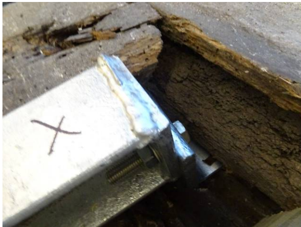
160 - Steel channel connected to the front elevation sole plate.
