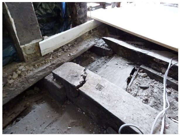
10 - Exposed timbers – taken from inside the property
