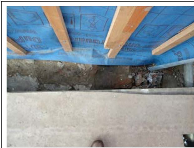
190 - New breather membrane and timber battens installed
