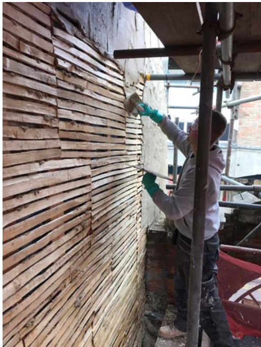
197 - Render being applied at the LHS elevation.
