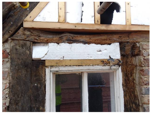
119 - LHS elevation – exposed timbers
