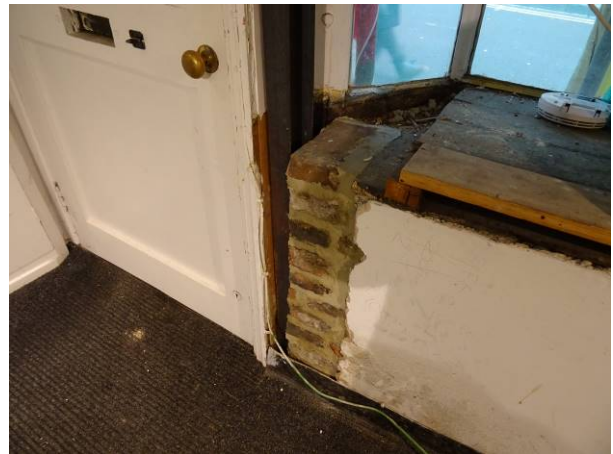
147 - Internals – Ground floor, newly installed prop at side of entrance door
