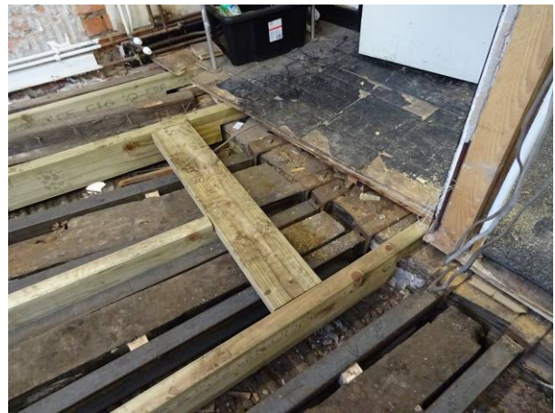
145 - Internals – First floor structural reinforcements / channel steel sections in pairs
