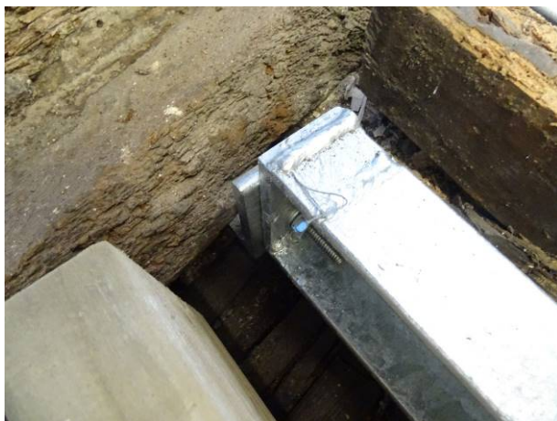
158 - Steel channel connected to the front elevation sole plate.
