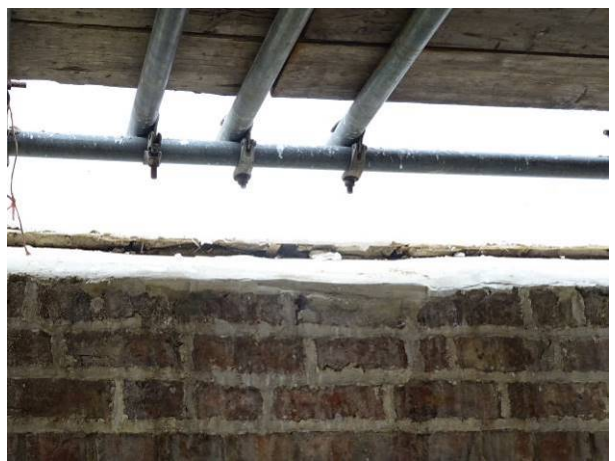
214 - Brickwork at LHS elevation
