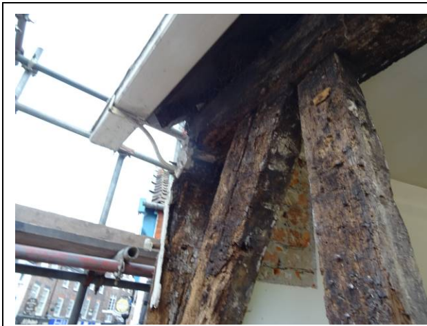
17 - Exposed timbers at front elevation
