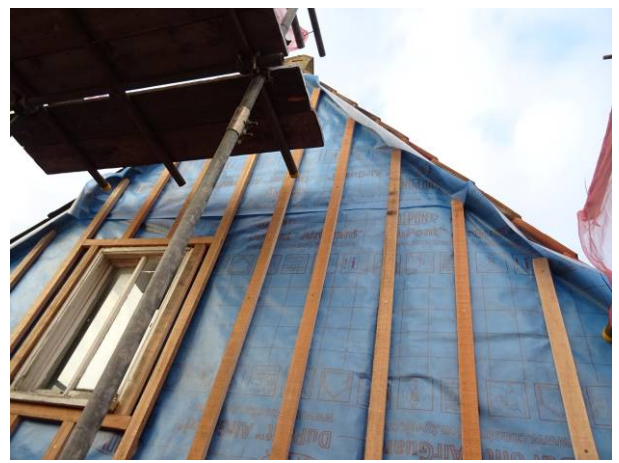
193 - New breather membrane and timber battens installed
