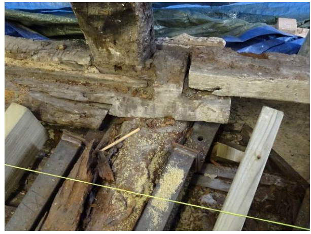
141 - Internals – First floor structural reinforcements with sole plates
