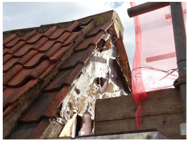
44 - LHS elevation - gable
