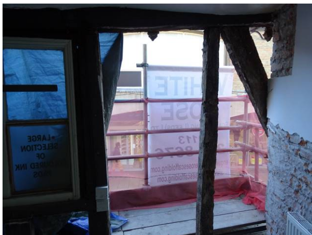
07 - Exposed timbers of front elevation – from internal
