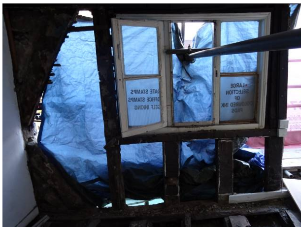
09 - Exposed timbers of front elevation – from internal
