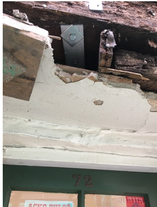
179 - Open construction to underside of jetty structure
