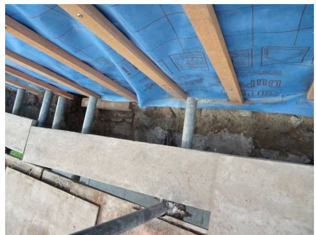
189 - New breather membrane and timber battens installed
