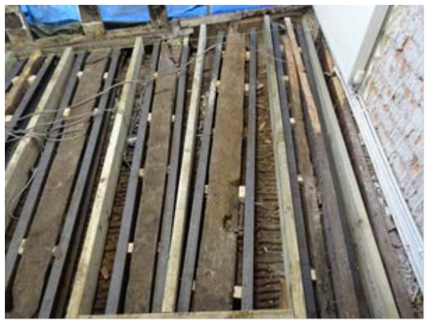
138 - Internals – First floor structural reinforcements / channel steel sections in pairs
