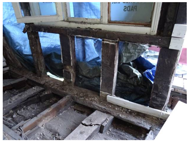
08 - Exposed timbers of front elevation – from internal
