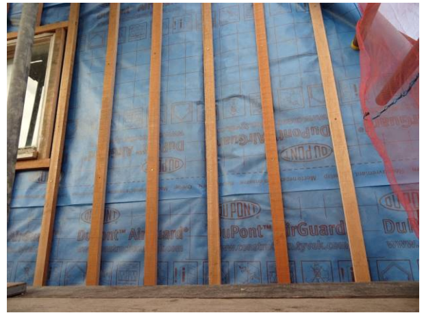
191 - New breather membrane and timber battens installed
