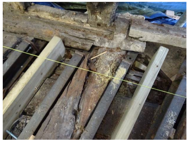
139 - Internals – First floor structural reinforcements with sole plates
