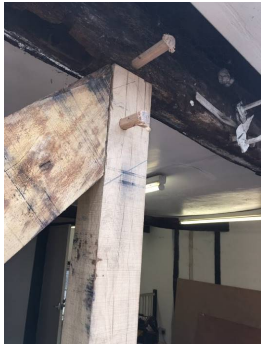
175 - New oak timbers to front LHS corner of the property
