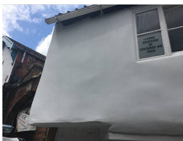
215 - Finished render at front elevation
