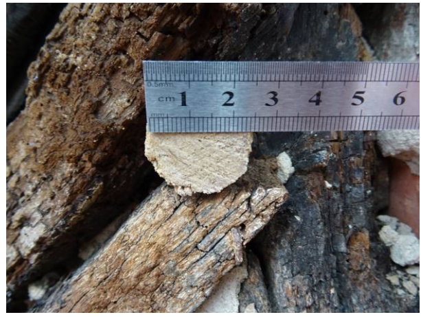
115 - LHS elevation - exposed timbers and previous repairs
