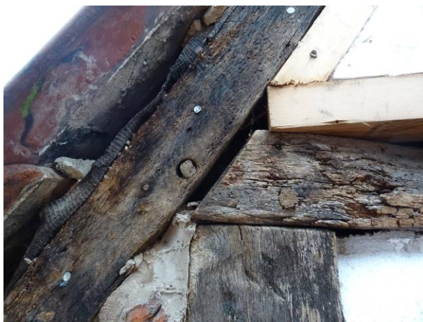
116 - LHS elevation – exposed timbers
