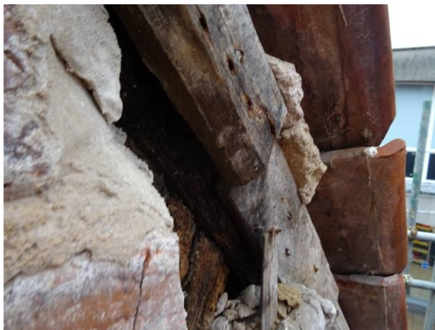
122 - LHS elevation – exposed timbers and previous repairs
