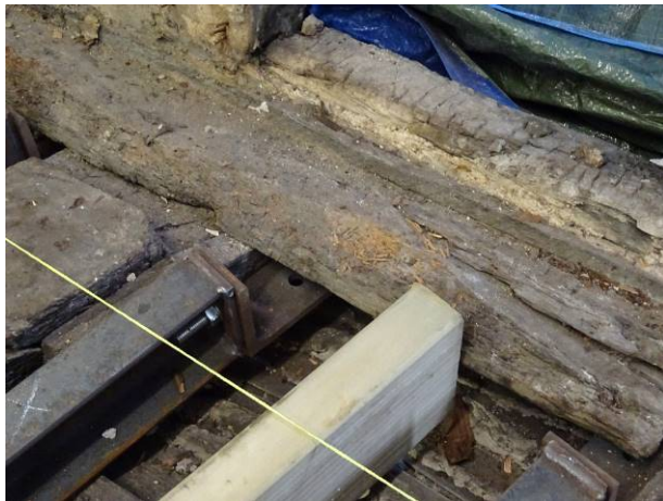
140 - Internals – First floor structural reinforcements with sole plates
