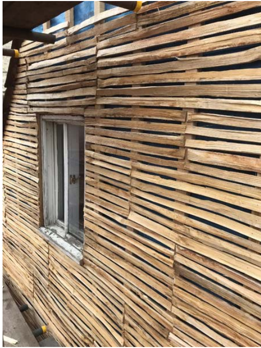
195 - New chestnut battens to LHS elevation
