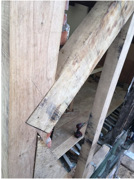
176 - New oak timbers to front LHS corner of the property
