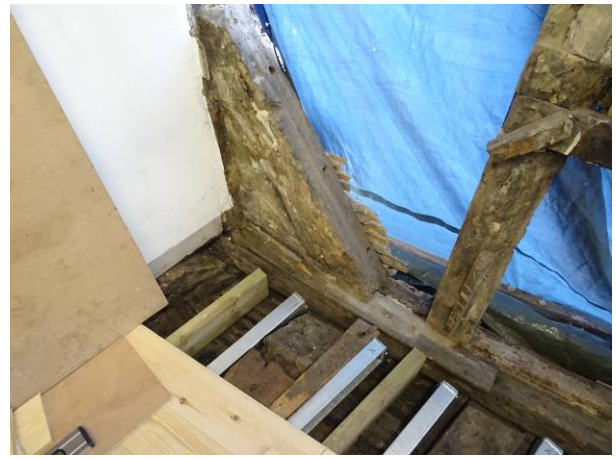
155 - Steel channels connected to the front elevation sole plate.
