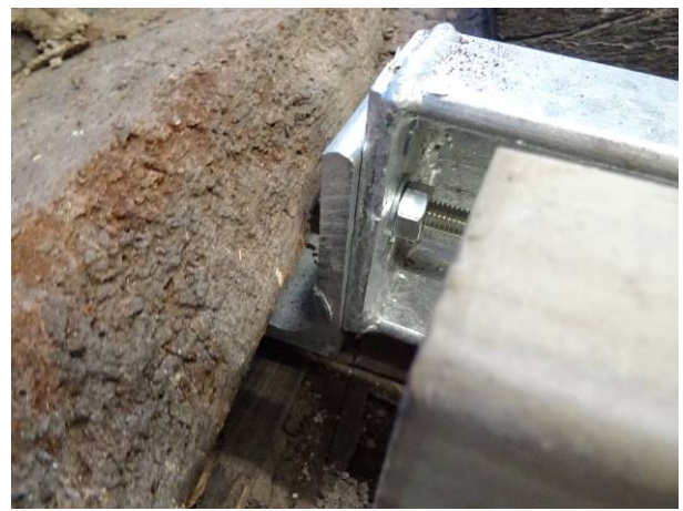
159 - Steel channel connected to the front elevation sole plate.
