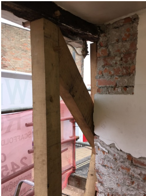
174 - New oak timbers to front LHS corner of the property
