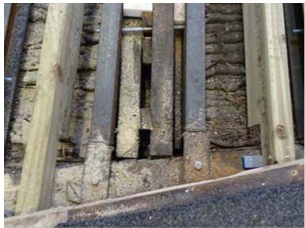
144 - Internals – First floor structural reinforcements / channel steel sections in pairs
