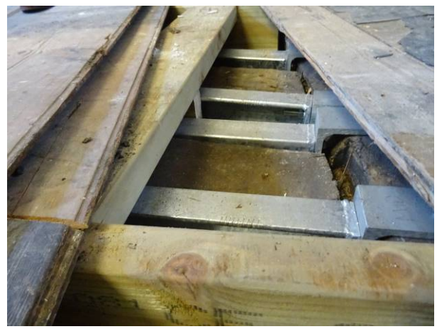
151 - Steel channels tied into the central beam
