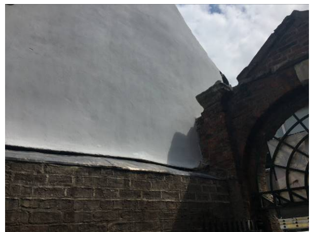
220 - Finished render at LHS elevation
