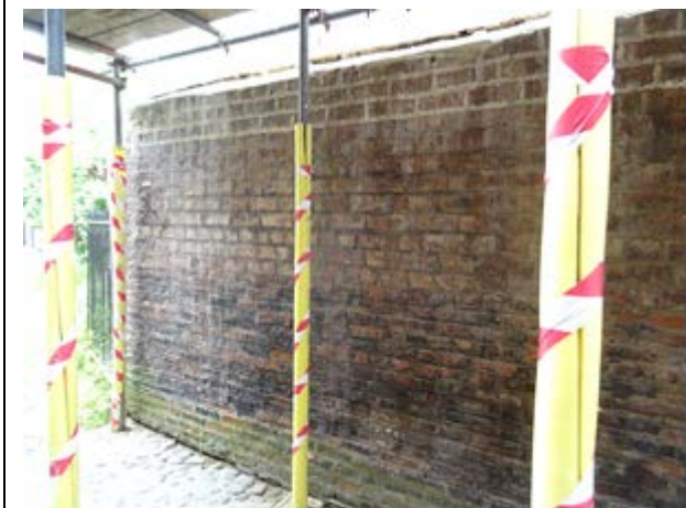
213 - Brickwork at LHS elevation
