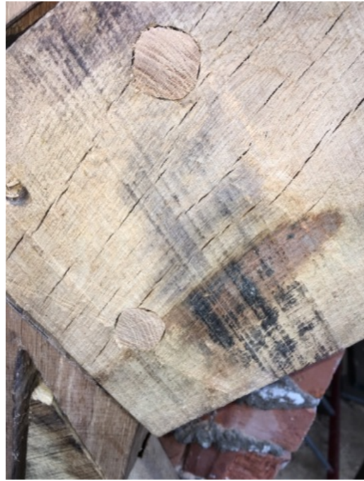
177 - New oak timbers to front LHS corner of the property
