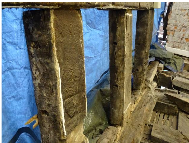
84 - Internals – exposed timbers of front elevation
