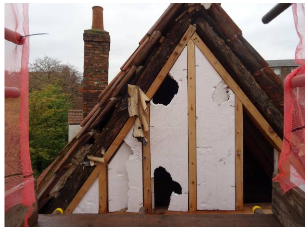
123 - LHS elevation – exposed timber and gable timbers
