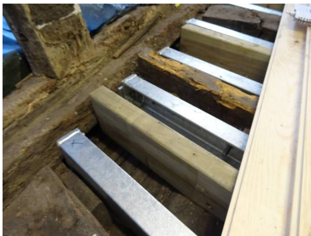
156 - Steel channels connected to the front elevation sole plate.
