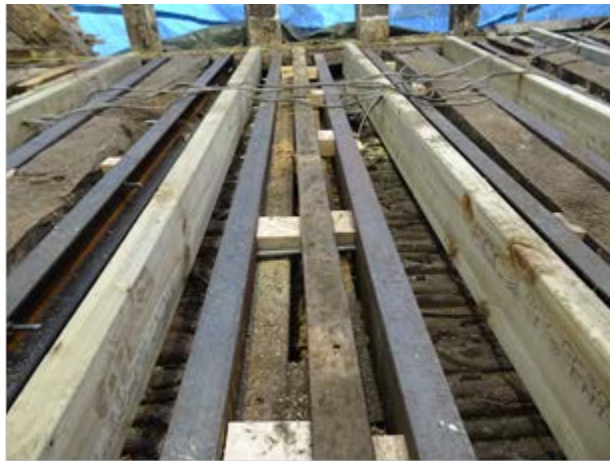
134 - Internals – First floor channel steel sections
