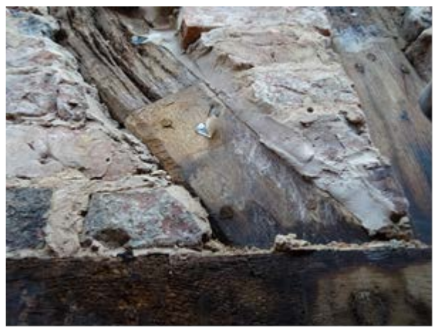
112 - LHS elevation – exposed timbers and previous repairs
