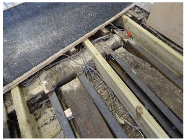
143 - Internals – First floor structural reinforcements / channel steel sections in pairs
