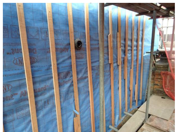
187 - New breather membrane and timber battens installed
