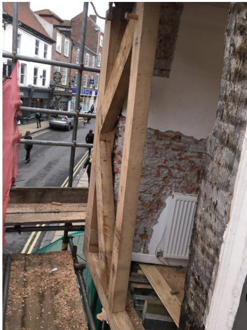
178 - New oak timbers to front LHS corner of the property
