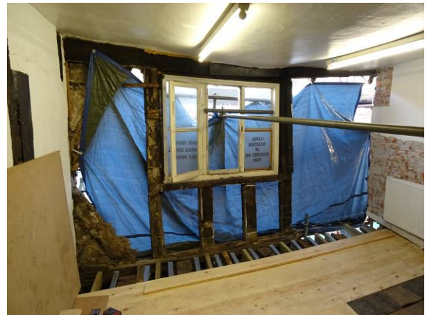
161 - Exposed timbers at the front elevation
