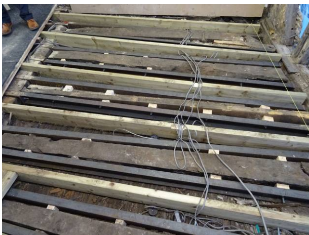
136 - Internals – First floor structural reinforcements / channel steel sections in pairs
