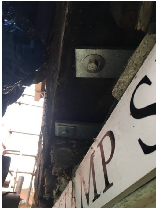
172 - Under side of jetty structure showing sole plates
