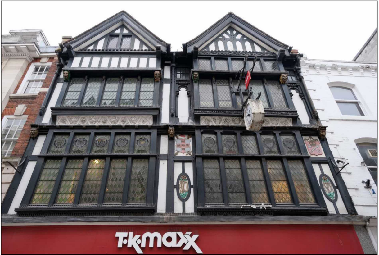
Plate 3. 48 Coney Street, detail of listed building frontage.
