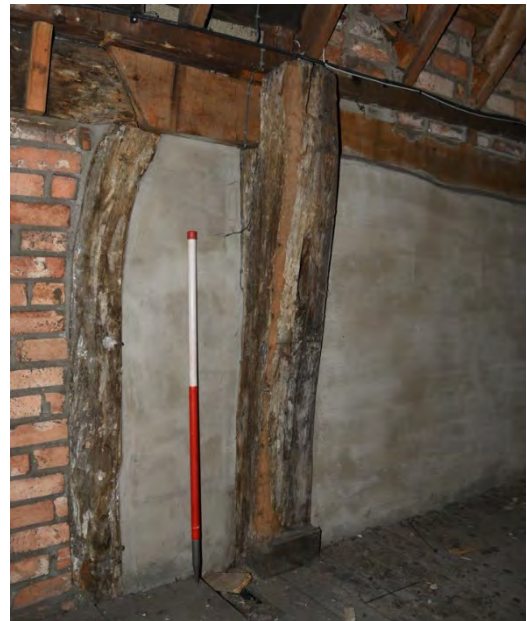
Plate 14 View of post D, looking S (YCY047)(scale 1.0m)
