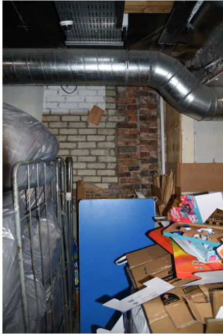
YCY011 Interior ground floor looking northeast showing wall scar (2m scale)
