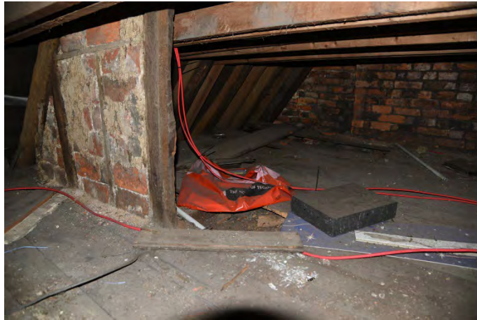
YCY052 Interior second floor looking south showing common rafters
