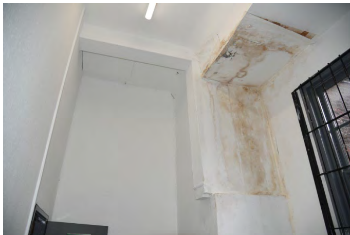
YCY026 Interior first floor looking east showing corbel with post above
