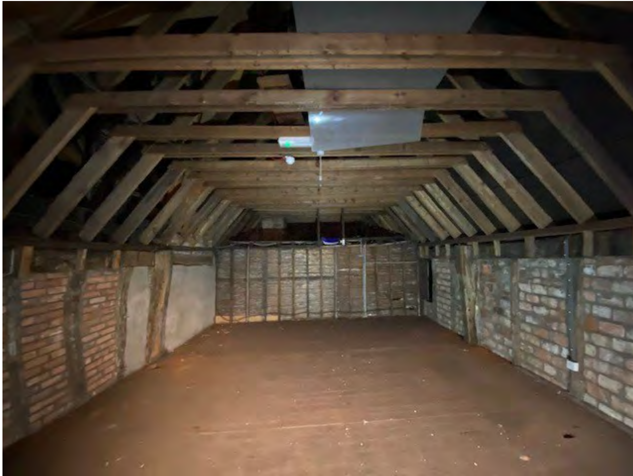
Figure 2: Posts and framing at second-floor level, photograph taken from the north
