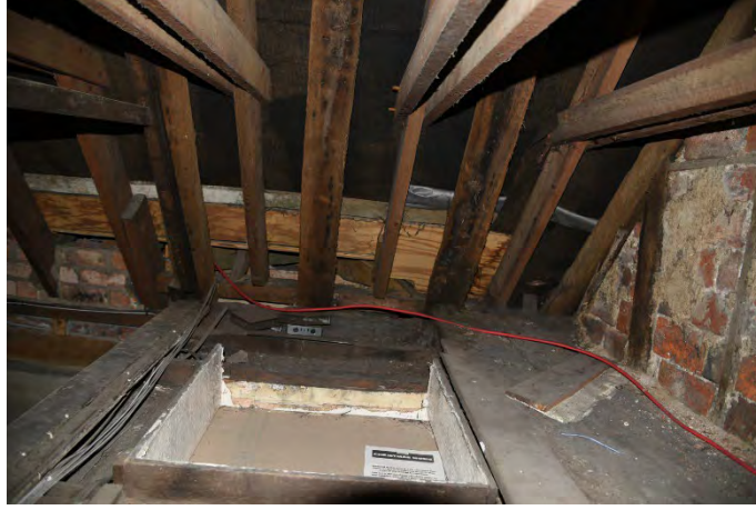
YCY051 Interior second floor looking southeast showing common rafters
