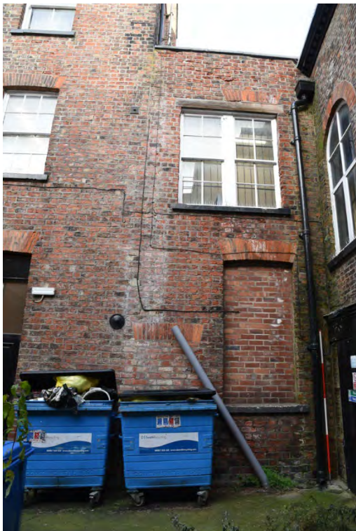
YCY003 External southeast elevation (2m scale)
