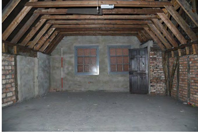
YCY043 Interior second floor looking northeast (2m scale)
