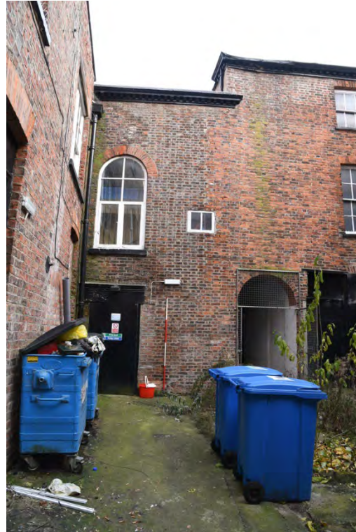
YCY002 External southwest elevation (2m scale)
