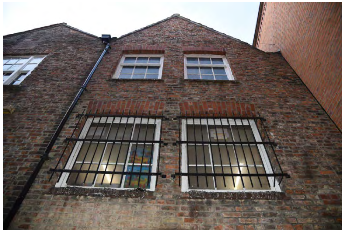
YCY009 Upper part of northeast elevation showing window openings
