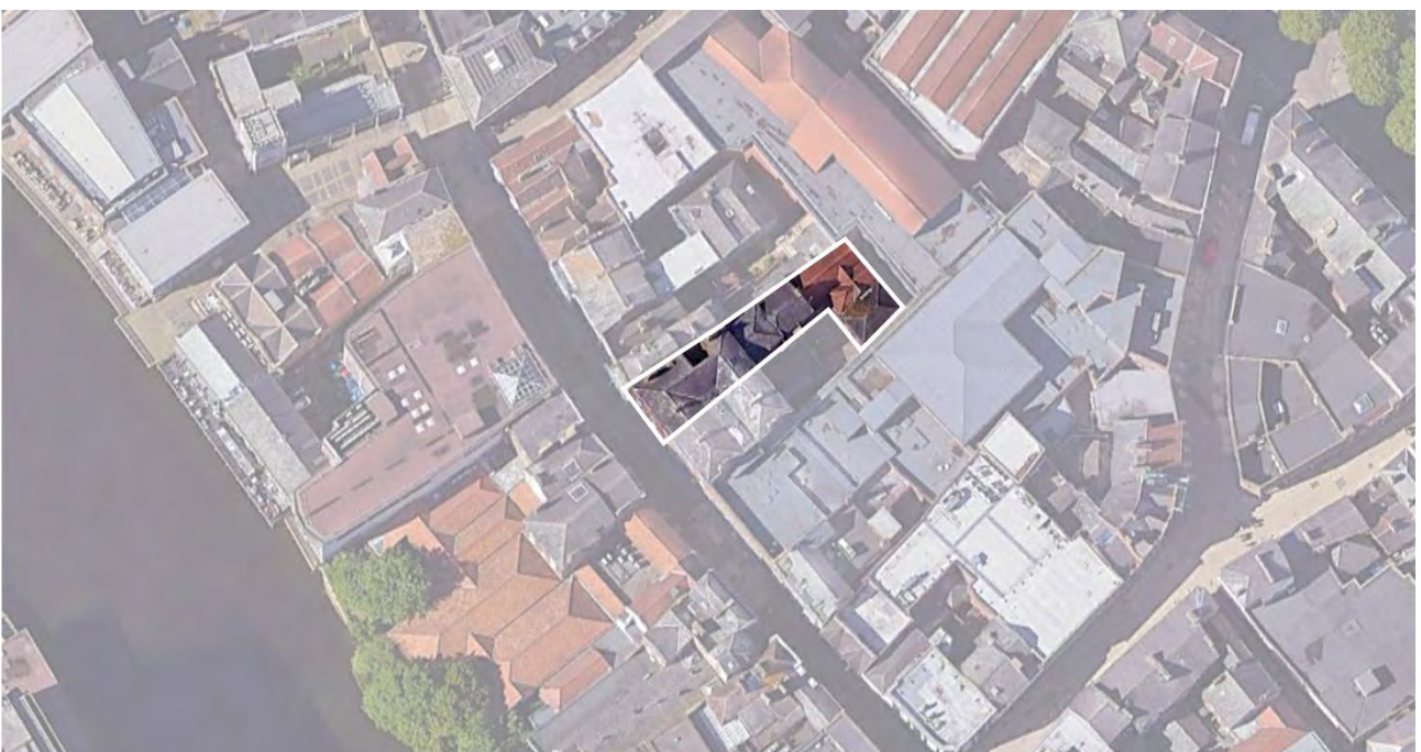
Plate 1 Aerial view of Coney Street, showing No. 36
