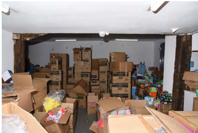
YCY022 Interior first floor looking northwest showing post A (left), post B (right) and wall plate
