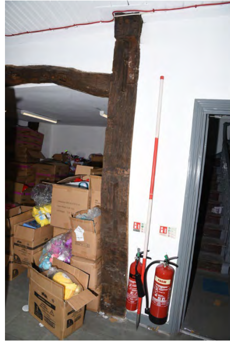
YCY018 Interior first floor looking north east showing post A and wall plate (2m scale)
