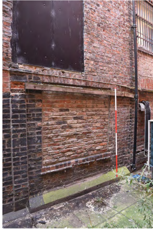
YCY006 Blocked opening in northeast elevation (2m scale)
