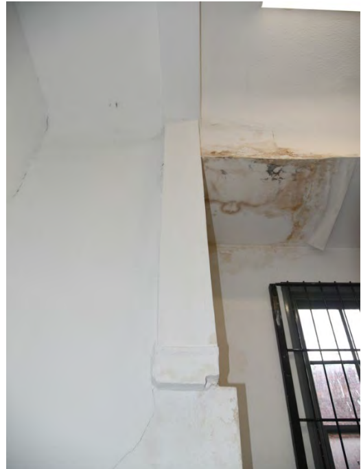
Plate 10 Corbel at first-floor level, between Bay 1 and Bay 2 (YCY025)
