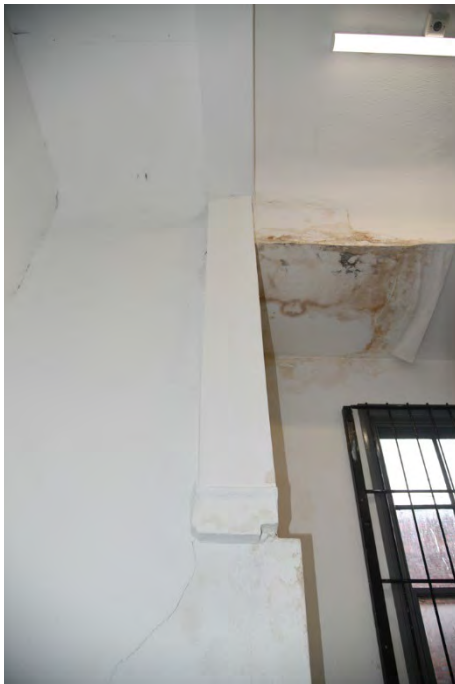
YCY025 Interior first floor looking southeast showing corbel with post above
