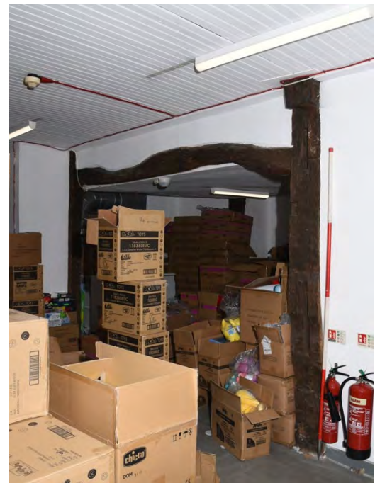
Plate 9 First floor showing posts A (right) and B (left) and wall plate (looking E, 2m scale) (YCY015)(scale 2.0m)
