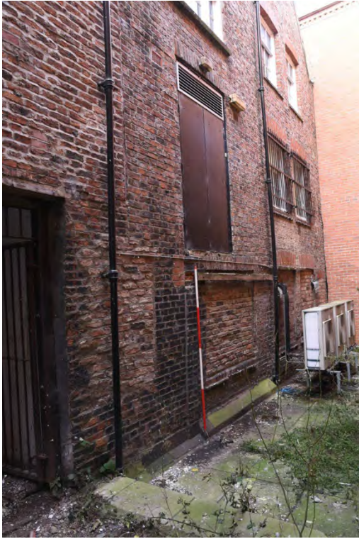
YCY005 External northeast elevation (2m scale)
