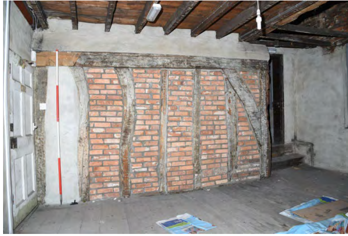
YCY031 Interior second floor looking north showing wall plate, studs, arch brace and post D (right) (2m scale)
