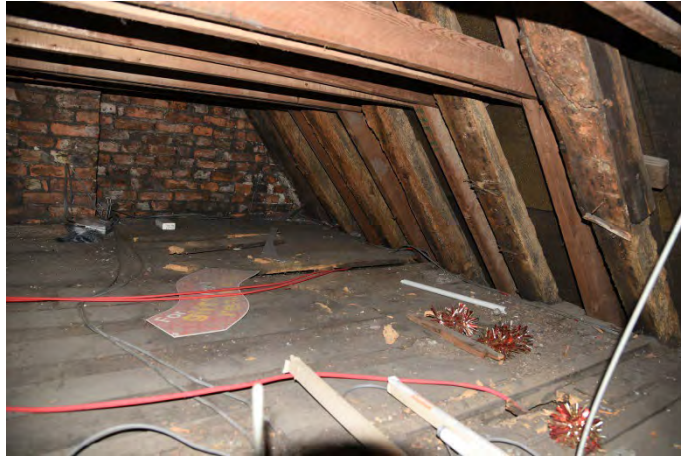
YCY054 Interior second floor looking west showing common rafters
