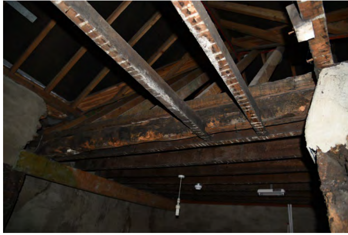
YCY037 Interior second floor looking south showing roof structure
