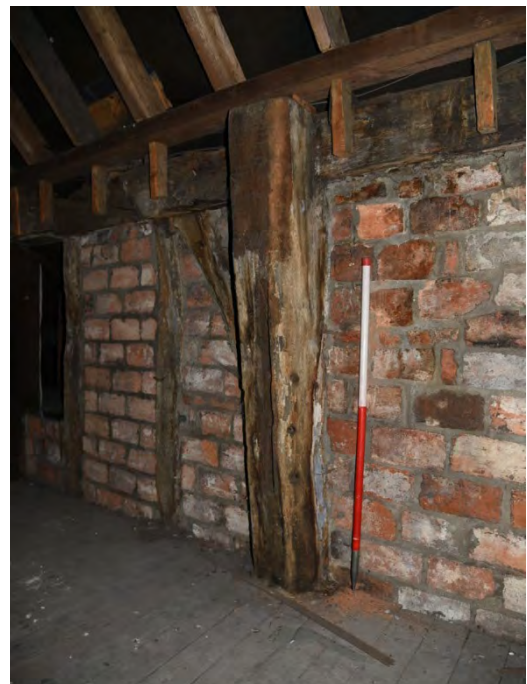
Plate 15 View of post G, looking W (YCY048)(scale 1.0m)
