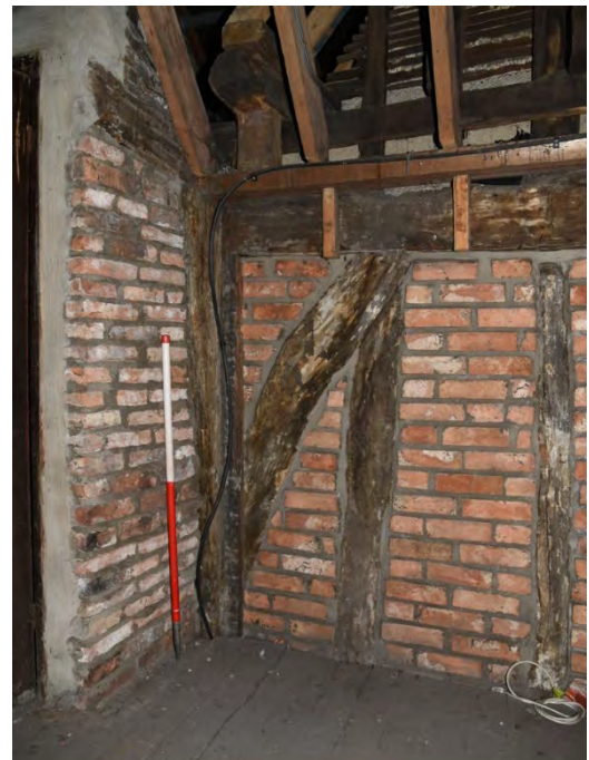
Plate 13 View of post E, looking E (YCY046)(scale 1.0m)
