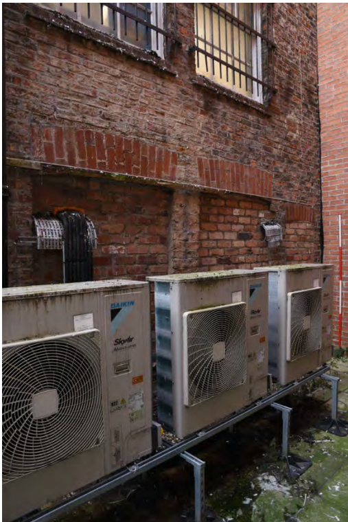
YCY007 Blocked window openings in northeast elevation (2m scale)
