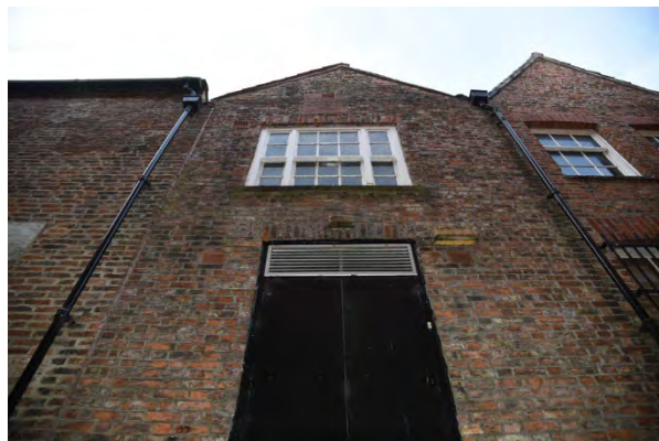
Plate 6 Exterior brick walls of the building (YCY008)
