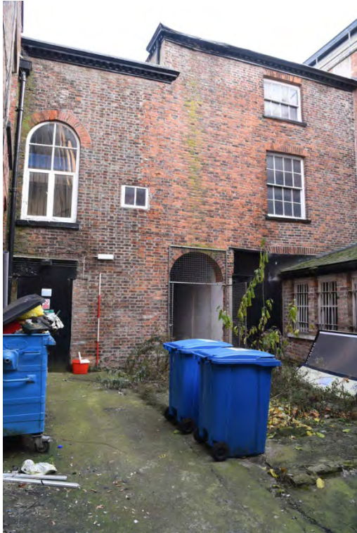
YCY001 External southwest elevation (2m scale)
