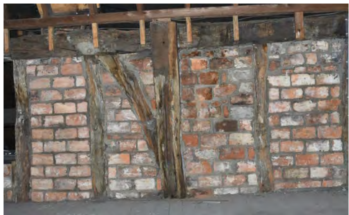
Plate 16 View of NW wall (YCY041)
