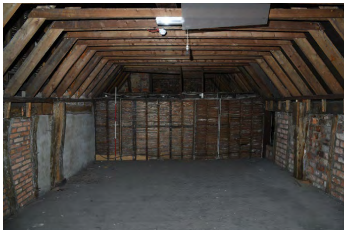
YCY039 Interior second floor looking southwest (2m scale)
