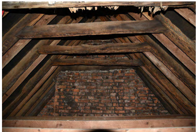
Plate 18 View of roof structure (YCY050)
