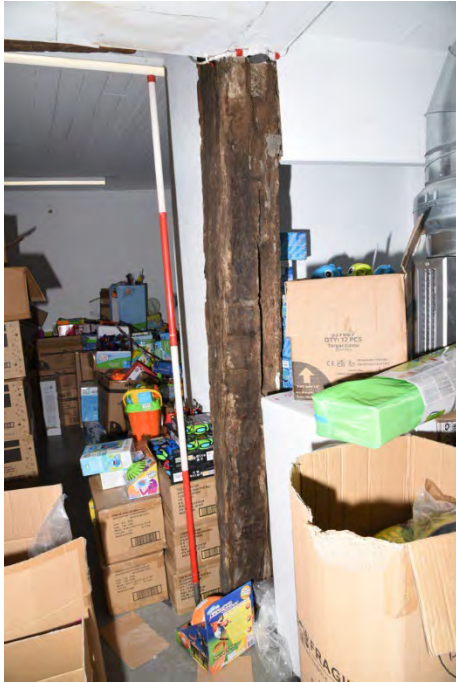
YCY017 Interior first floor looking north showing post B (2m scale)
