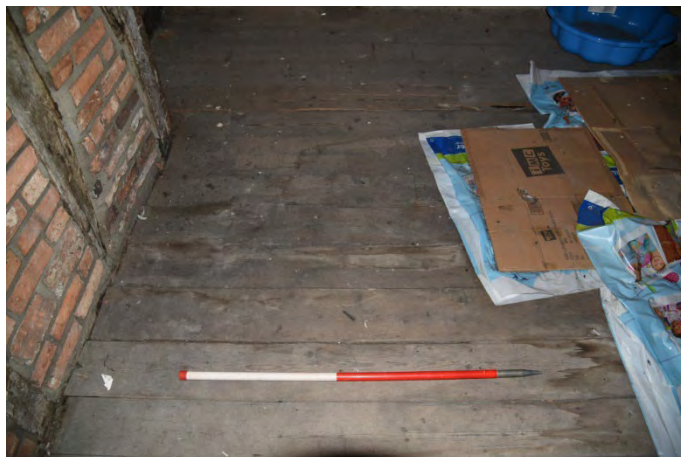
YCY036 Interior second floor looking northeast showing floor boards (1m scale)
