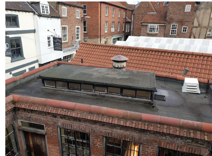
Figure 33 Present roof covering and skylight on the c.1960 kitchen range.
