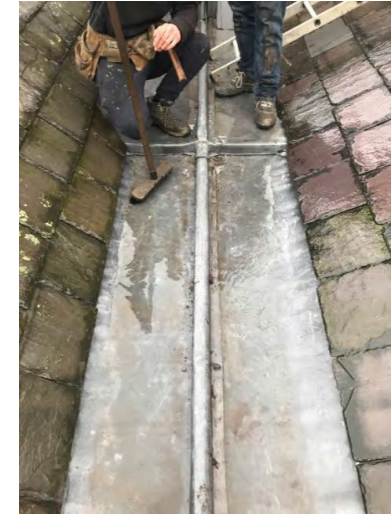
MAINTENANCE Example of valley gutter cleaning at York Theatre Royal, this needs to be undertaken on a 3-month cycle.
