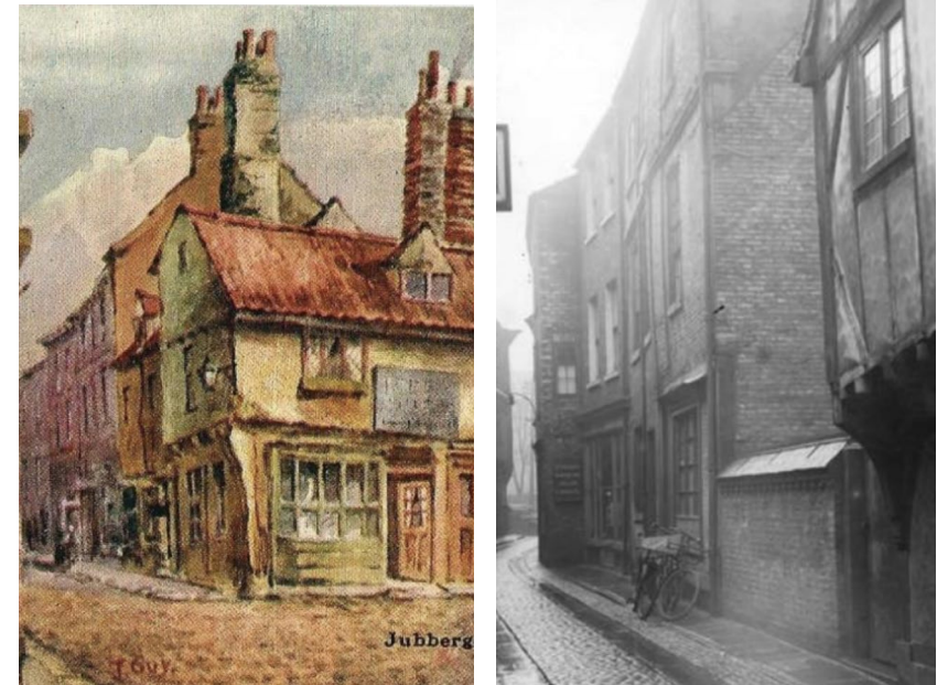
Figure 16 Left (16A) Detail from late C19th painting by Thomas Guy in which a jettied timber framed building can be seen on Newgate behind the C14th range; Right (16B) Detail from a 1933 photograph showing new courtyard, with the roof scar of the now lost range on the site of the present kitchens © York Explore
