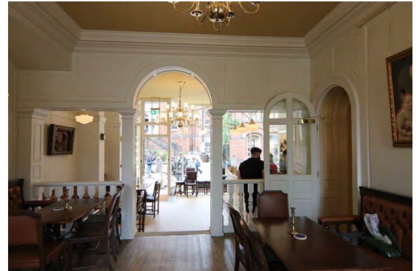
RESTORATION Archway restored to ground floor of 14 Lendal. New timberwork made to exactly replicate the original fabric by tracing their outline in the original paintwork
