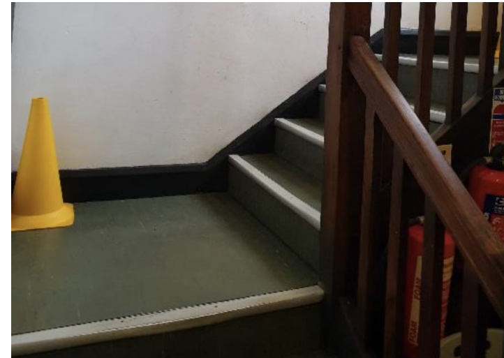
Figure 31 Existing stair covering (stair 2).
