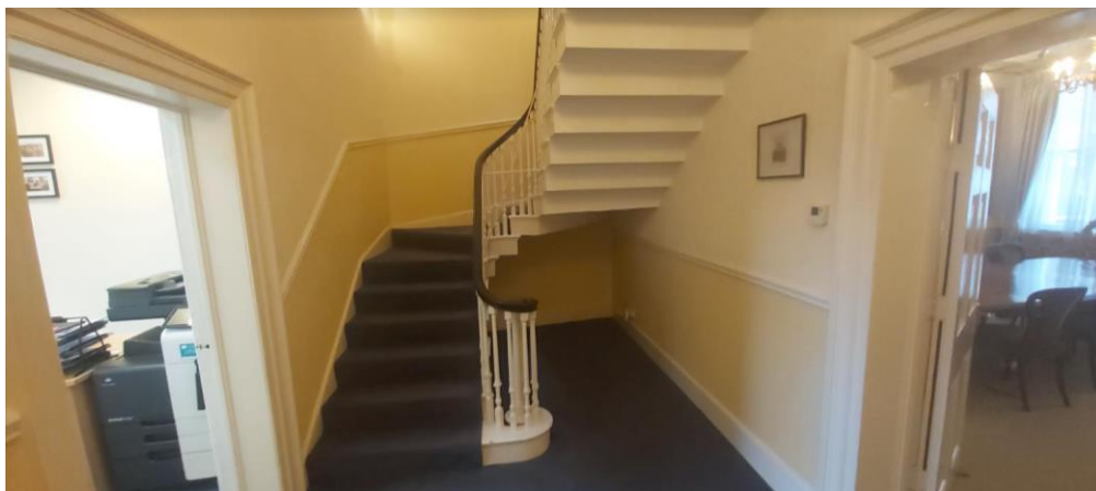
Fig 15 Cantilevered staircase, swept handrail, slender balusters and dado rail
