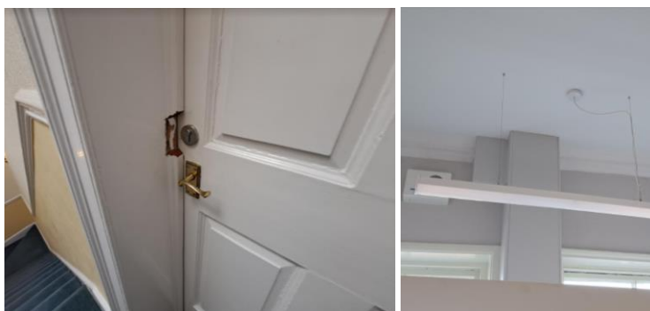
Fig 61 Harmful works repaired
