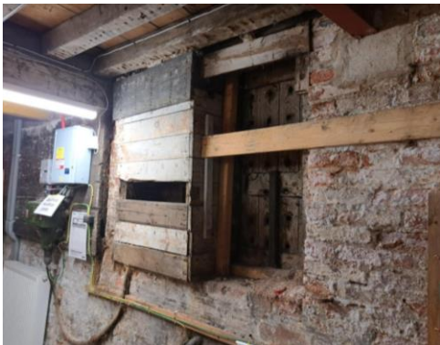
Fig 39 Blocked opening in front elevation Fig 40 Evidence of former cellar ceiling
