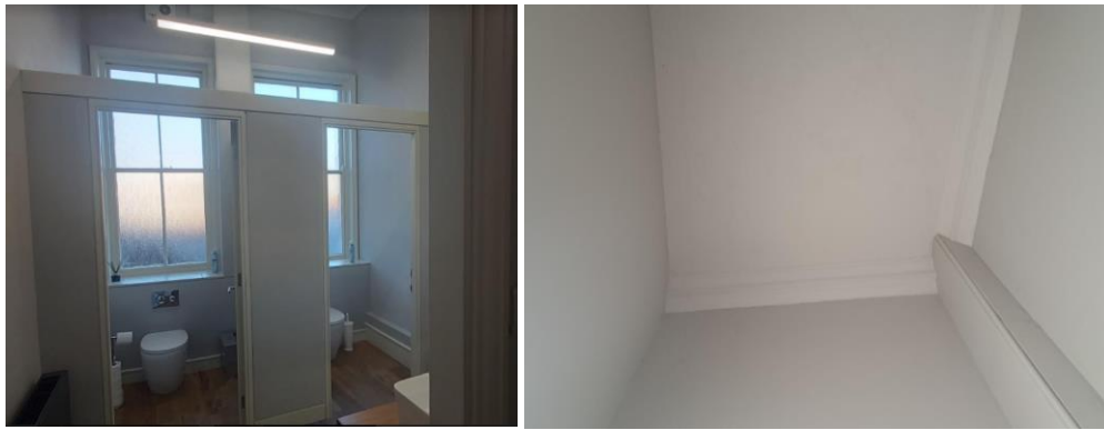
Figs 66 & 67 Modern w.c. stalls and conduit to ff, rear, left room to be removed
