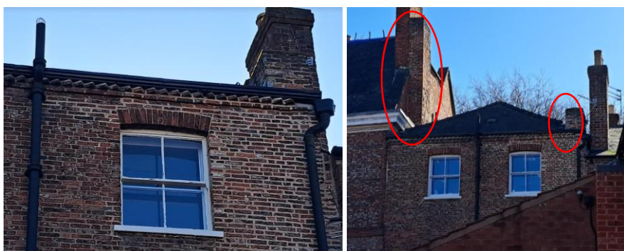
Fig 9A Eaves band & enlarged window Fig 9B Tall gable and truncated corner chimney
