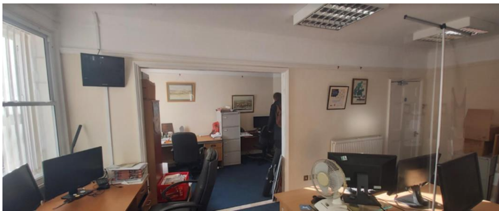
Fig 75 Modern opening between sf, front rooms will be infilled & modern lights removed
