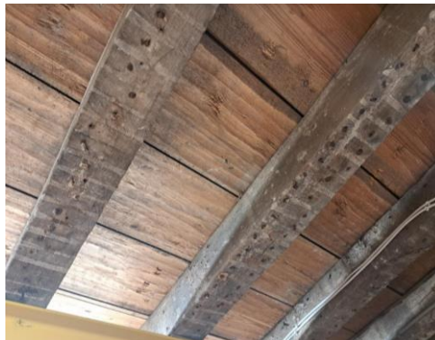
Fig 39 Blocked opening in front elevation Fig 40 Evidence of former cellar ceiling
