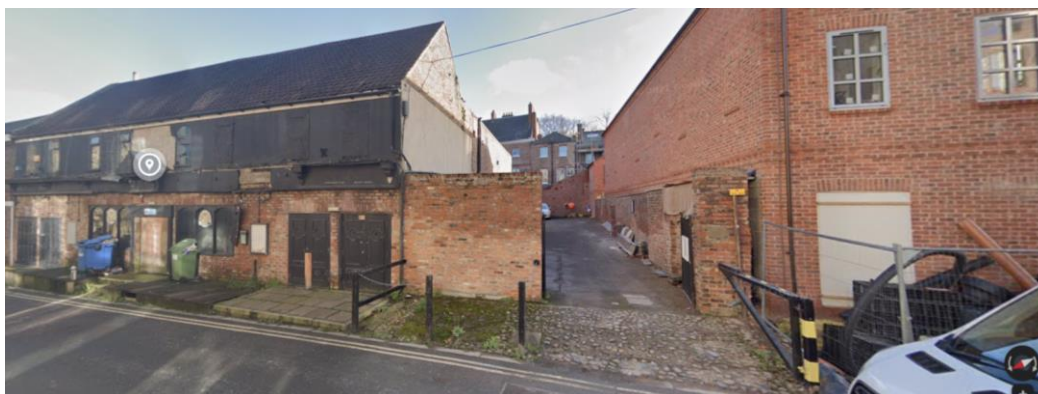
Fig 55 Application site: similar in character to the 'development opportunity' in the CAA
