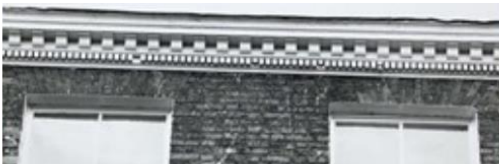
Fig 9 Cornice to front elevation of 92 Micklegate
