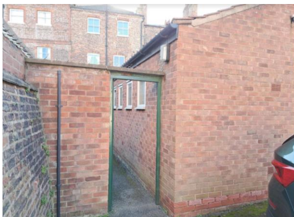
Fig 79 Dense brick wall & conduit to be removed
