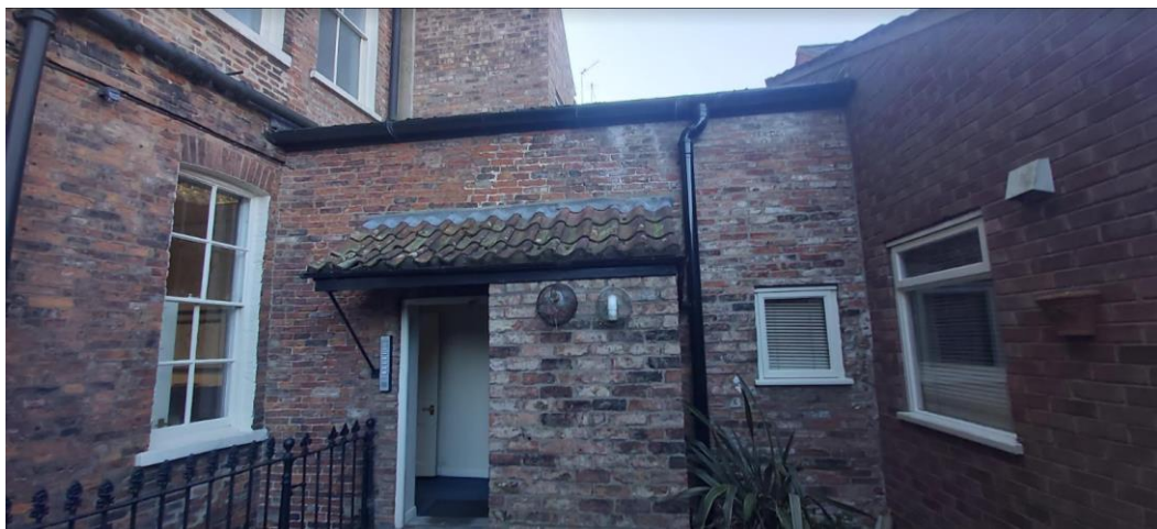
Fig 11 Historic fabric to the ground floor link with later porch
