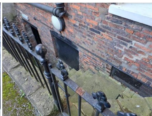
Fig 57 Missing finial on rear gate reinstated
