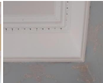
Fig 18 ff front room
