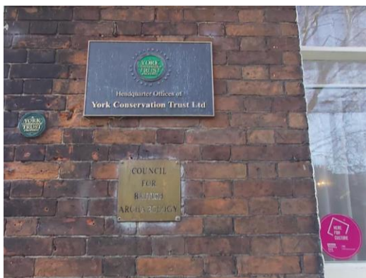
Fig 56 Four signs to be removed
