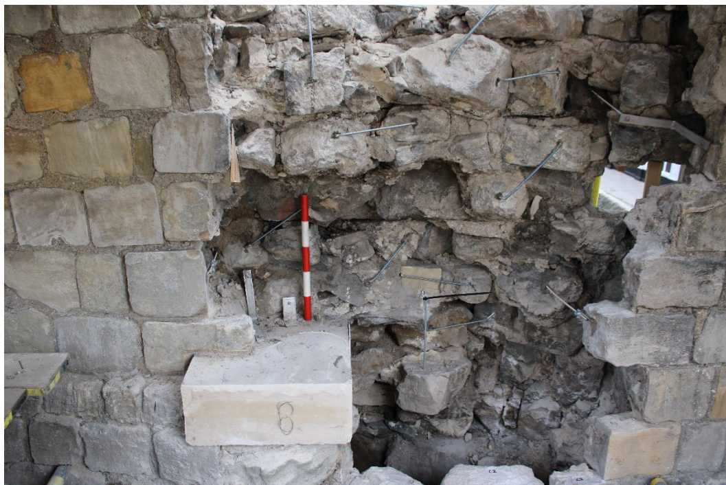
Plate 7 Wall core (0.5m scale).
