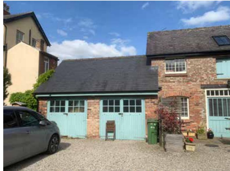
Figure 17 - View of garage
