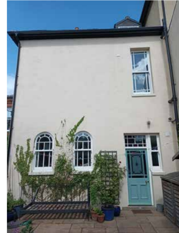
Figure 16 - Current rear elevation of rear wing
