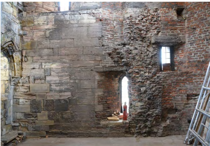
Plate 71 Southeast wall of the Chapel
