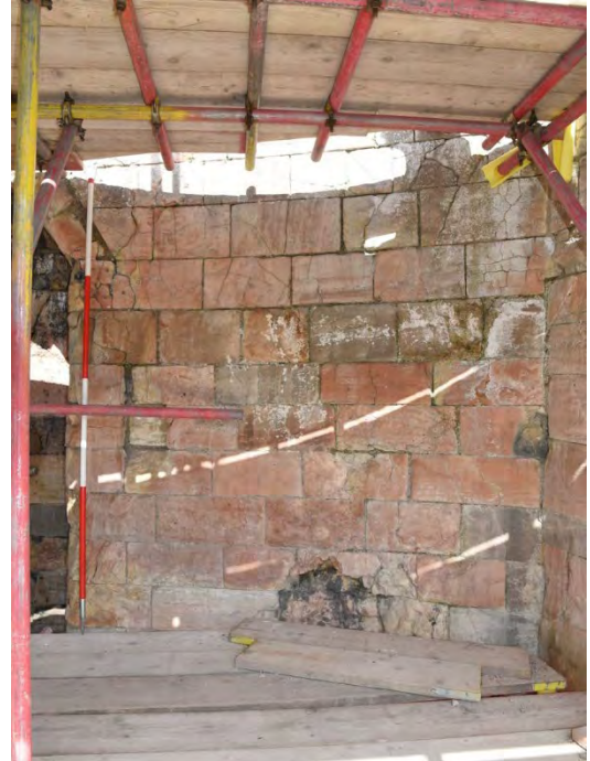
Plate 79 Pair of blocked sockets that would have supported a fire hood above the chased out fireback (Scale 2.0m)
