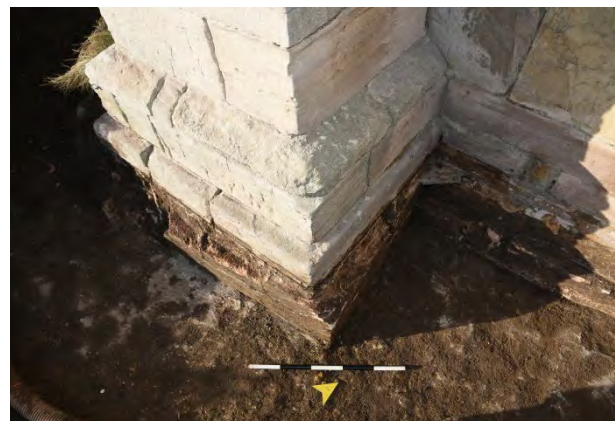
Plate 39 SW buttress of the forebuilding, showing lower courses and concrete underpinning
