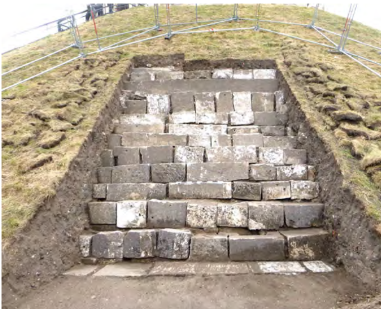
Plate 15 Gritstone blocks reinstating the slope of the motte
