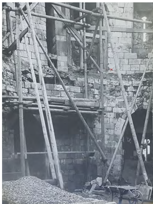
Plate 98 View of scaffold system erected in the tower in the 1920s
