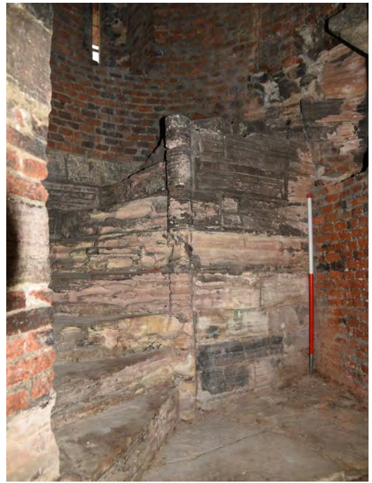
Plate 69 Newel staircase in the forebuilding (Scale 1.0m)
