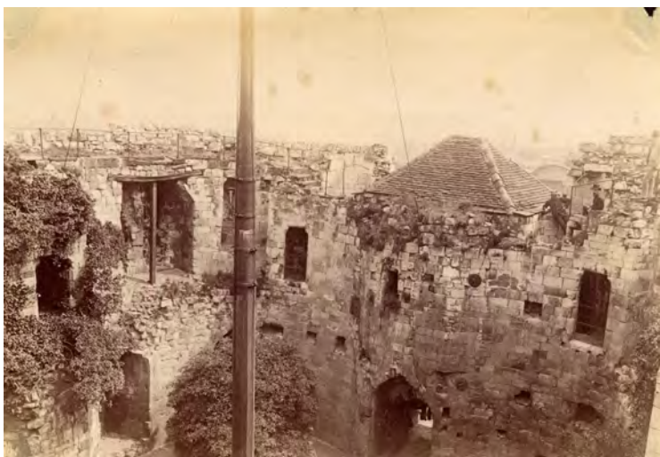
Plate 95 View of the large central flagpole and cable system
