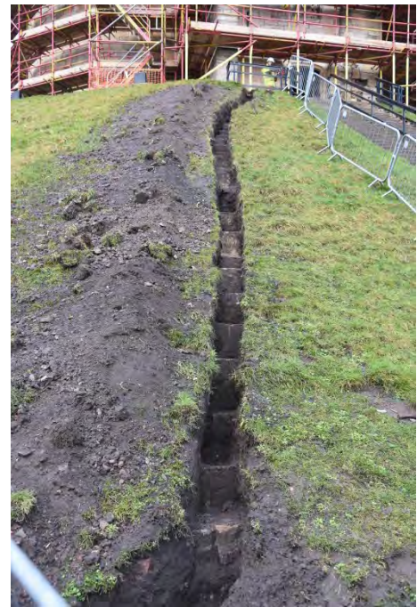
Plate 38 Electricity trench (Int 7) showing blockwork forming the motte profile (F25 C1036)
