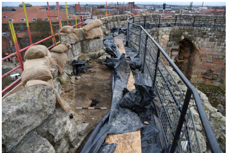
Plate 85 Small shaft from the wall-walk to the first floor garderobe (Scale 0.5m)
