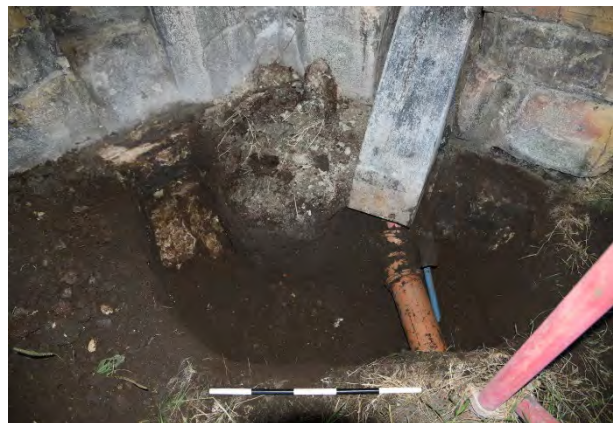
Plate 42 Drainage through the NW side of the tower
