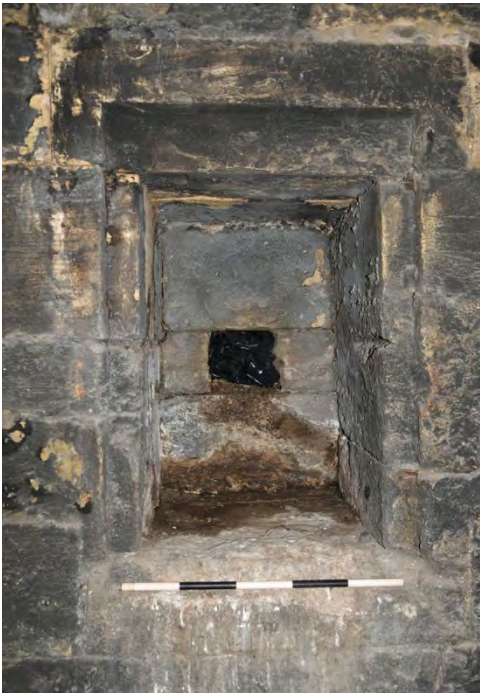
Plate 86 Wall cupboard opposite the first-floor garderobe seat (Scale 0.5m)
