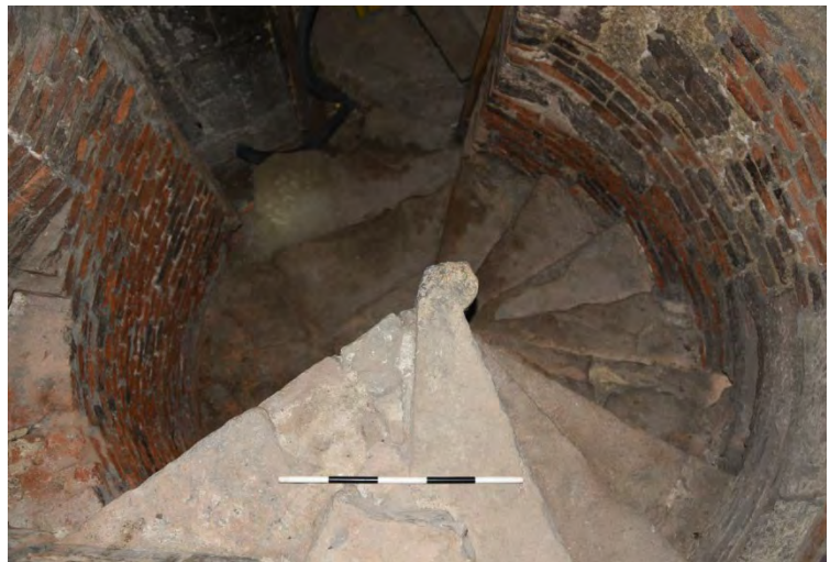
Plate 70 Stair risers of the newel staircase in the forebuilding (Scale 0.5m)
