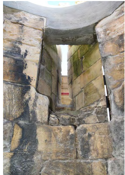
Plate 88 Loop embrasure in the bartizan stair turret (Scale 0.5m)
