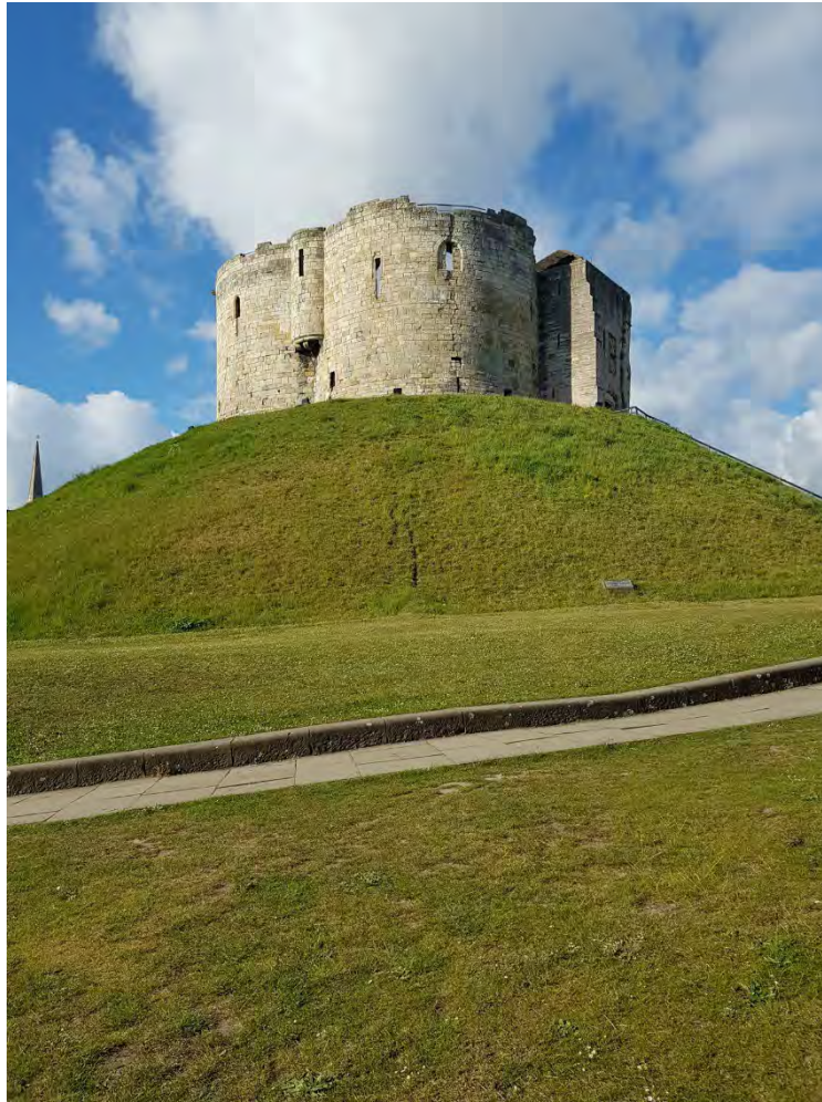
Plate 2 General view of the tower prior to the onset of works, looking north
