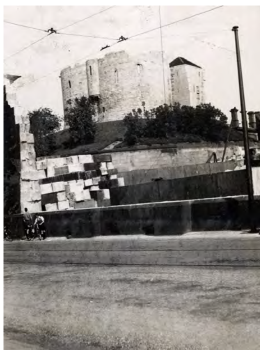
Plate 99 View of prison wall during demolition, the likely source of stone now buried in the motte
