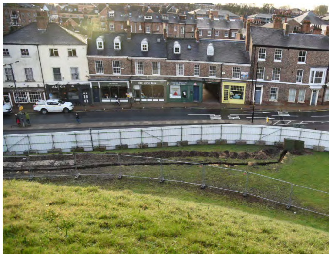
Plate 32 General view of electricity trench, looking west from the motte
