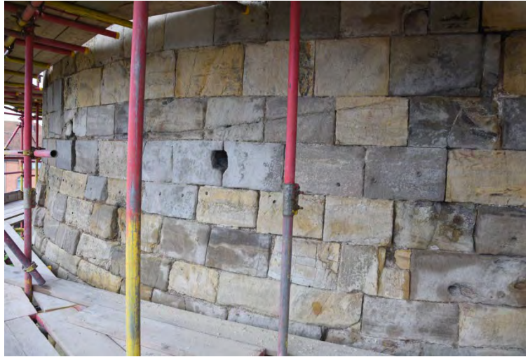
Plate 62 Roof scar and sockets on the exterior of the west lobe
