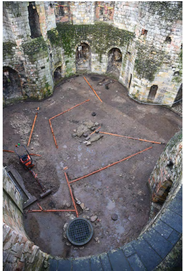
Plate 31 Drainage systems crossing Intervention 6
