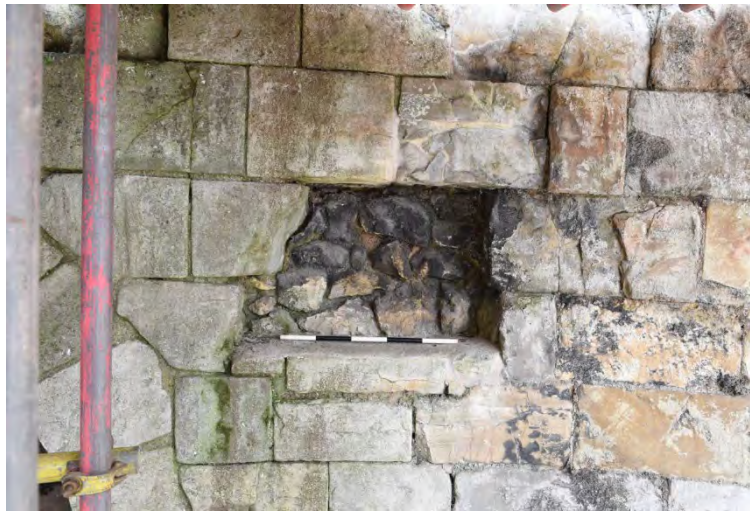
Plate 77 Large socket with pad stone in the west lobe (Scale 0.5m)
