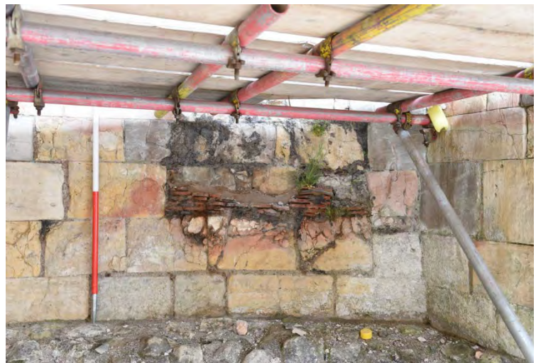
Plate 80 Fireplace at first-floor level in the north lobe (Scale 1.0m)
