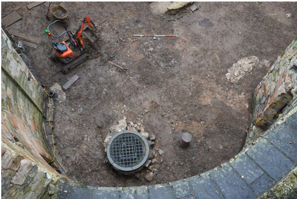
Plate 20 View of the east lobe looking west, showing rubble within the construction cut of the upper part of the well (Scale 2.0m)
