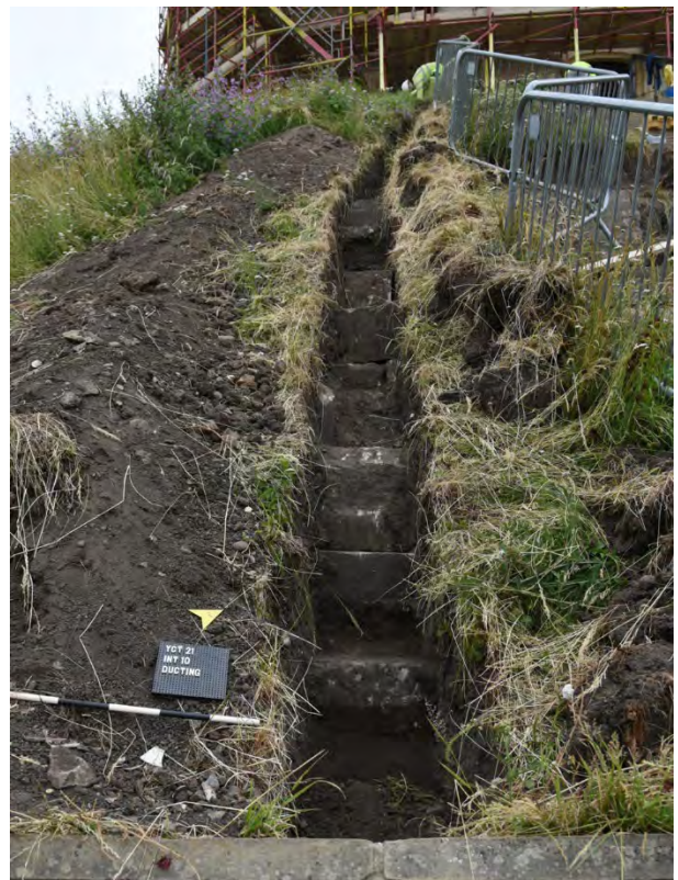
Plate 47 Ducting trench showing stepped makeup
