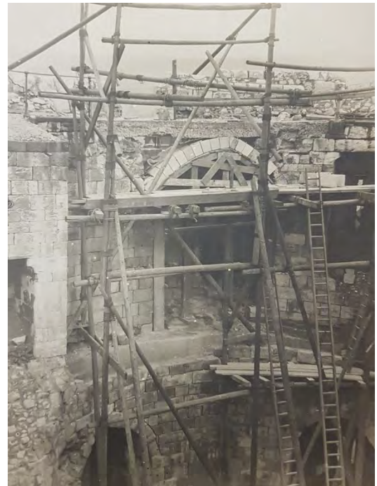
Plate 82 View of east lobe window opening being rebuilt in the 1920s
