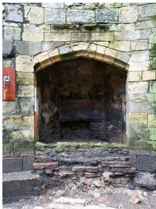
Plate 74 Ground-floor fireplace in the west lobe following ground reduction (Scale 1.0m)
