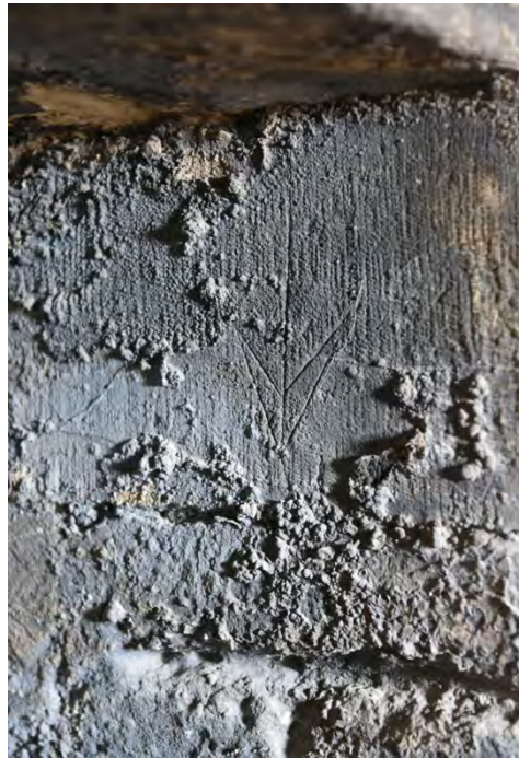
Plate 87 Mason's mark within the first-floor garderobe cupboard
