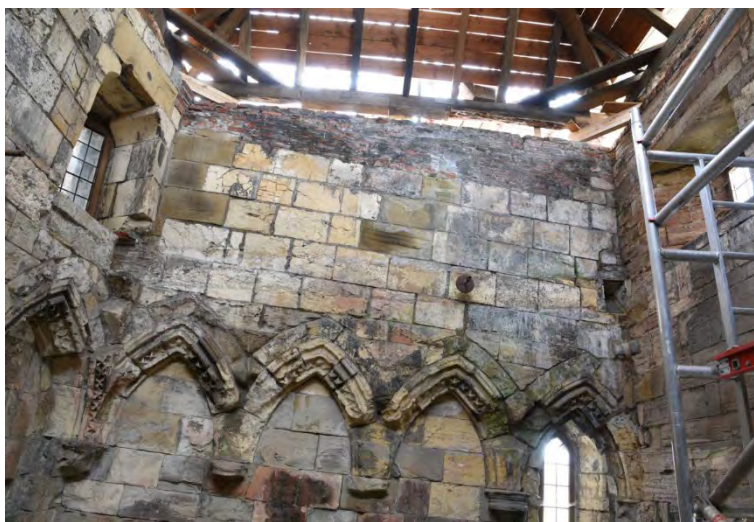
Plate 56 The roof structure undergoing repairs after being raised
