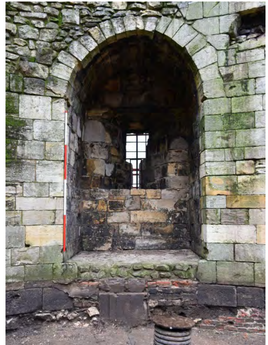
Plate 75 Bottom of the ground floor northern window embrasure in the west lobe (Scale 2.0m)
