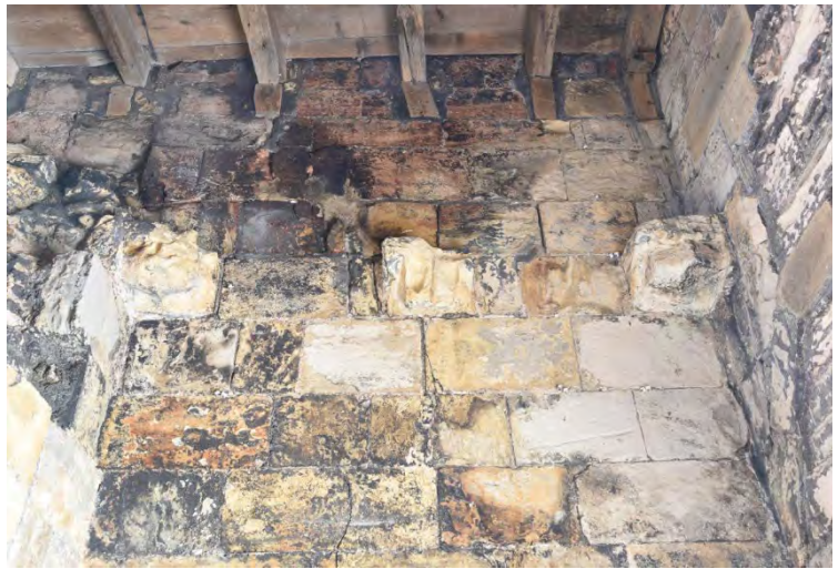
Plate 68 Stone corbels on the northeast wall of the outer lobby of the forebuilding (Scale 0.5m)
