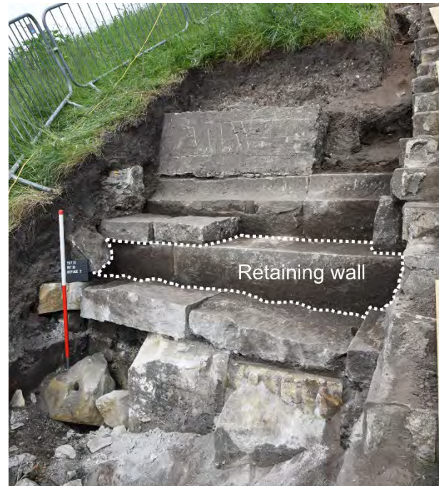
Plate 43 Retaining wall (F71 C1104), behind and beneath block make-up (F69 C1102)
