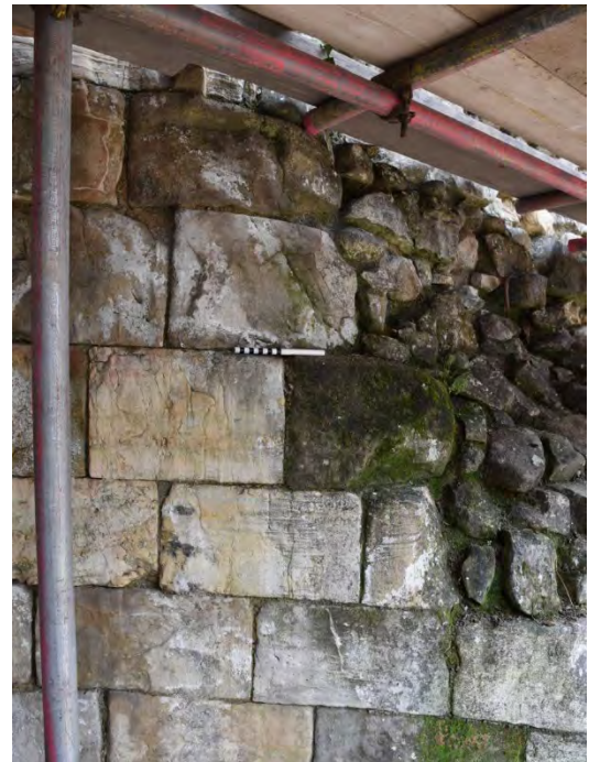
Plate 78 Offset that would have supported the first-floor boarding (Scale 1.0m)
