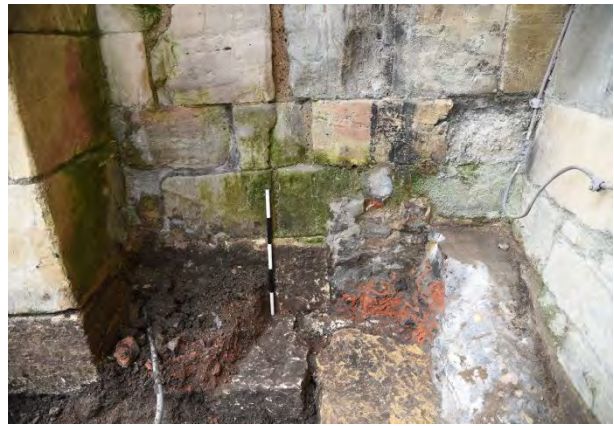
Plate 40 NE elevation of the forebuilding, looking SW. Scale 0.5m
