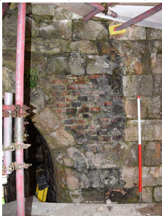
Plate 73 Brick blocked socket in the south lobe (Scale 1.0m)
