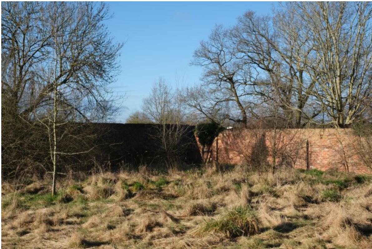
Plate 30: The south-eastern elevation of wall A, facing north-west, scale unit 0.5m.
