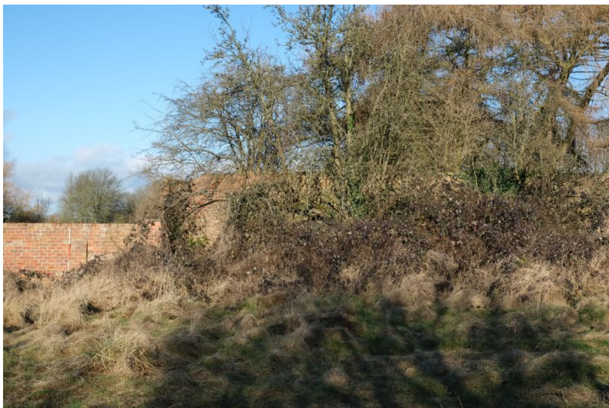
Plate 26: The overgrown north-eastern end of the south-eastern elevation of wall A.
