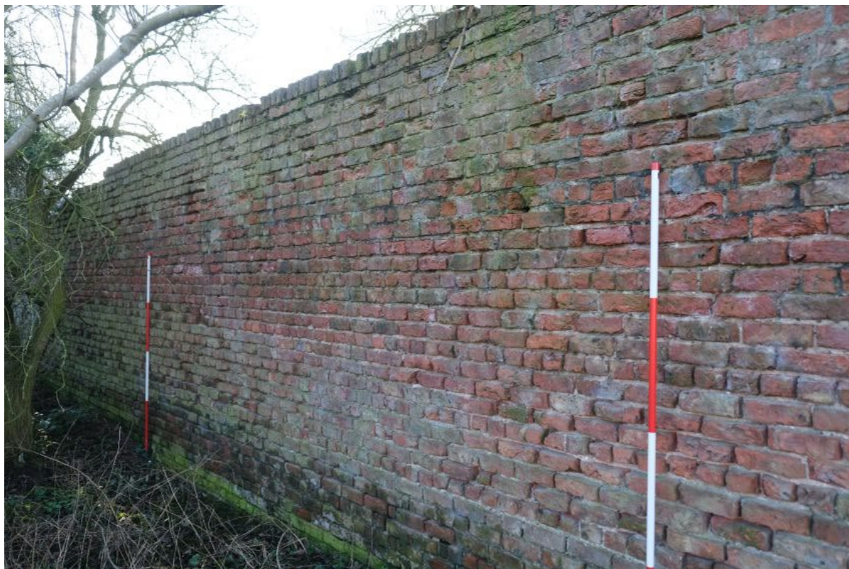
Plate 43: The north-eastern elevation of Wall B, facing south-east, scale unit 0.5m.
