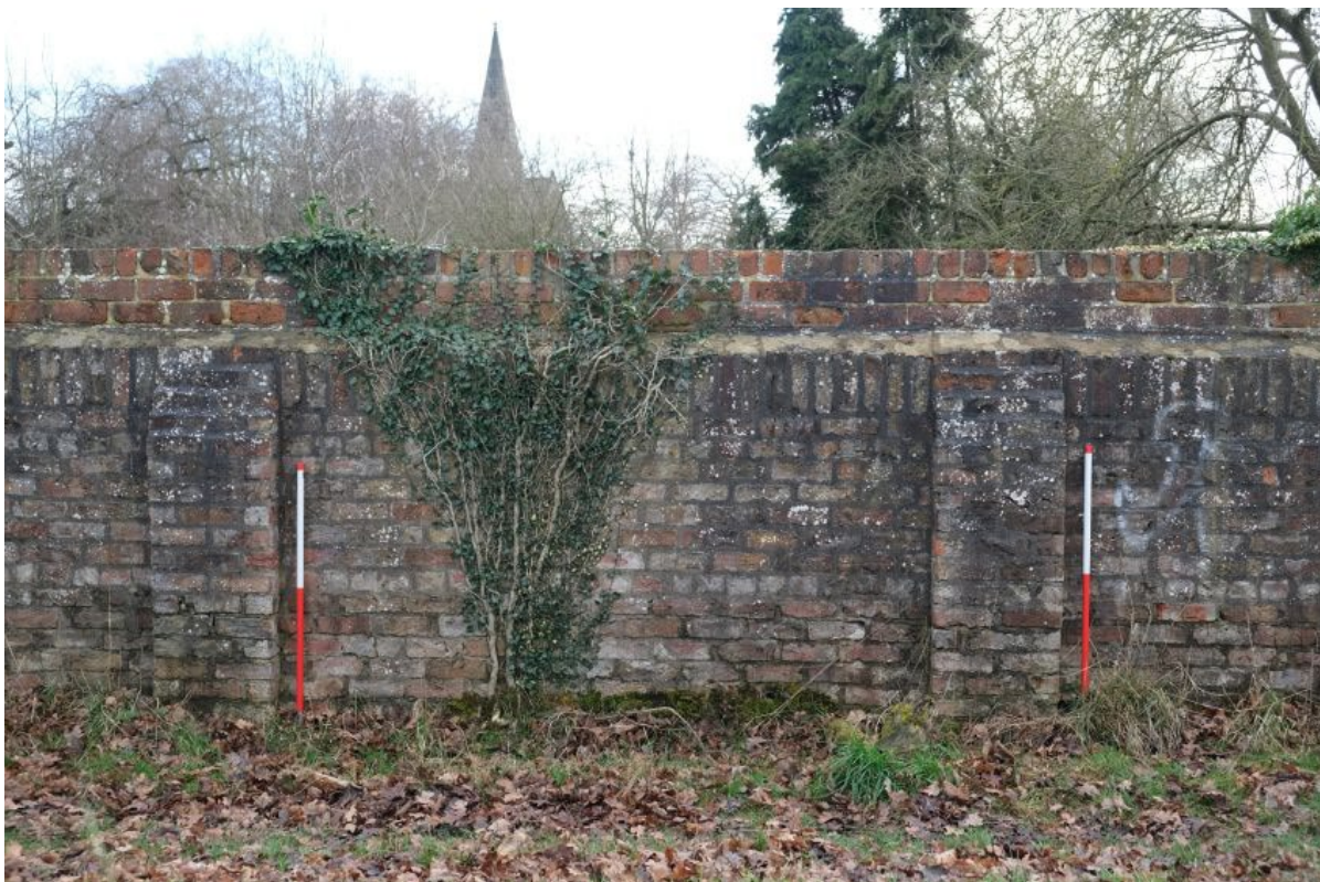
Plate 24: A creeper growing against the north-eastern elevation of Wall A, facing south-east, scale unit 0.5m.
