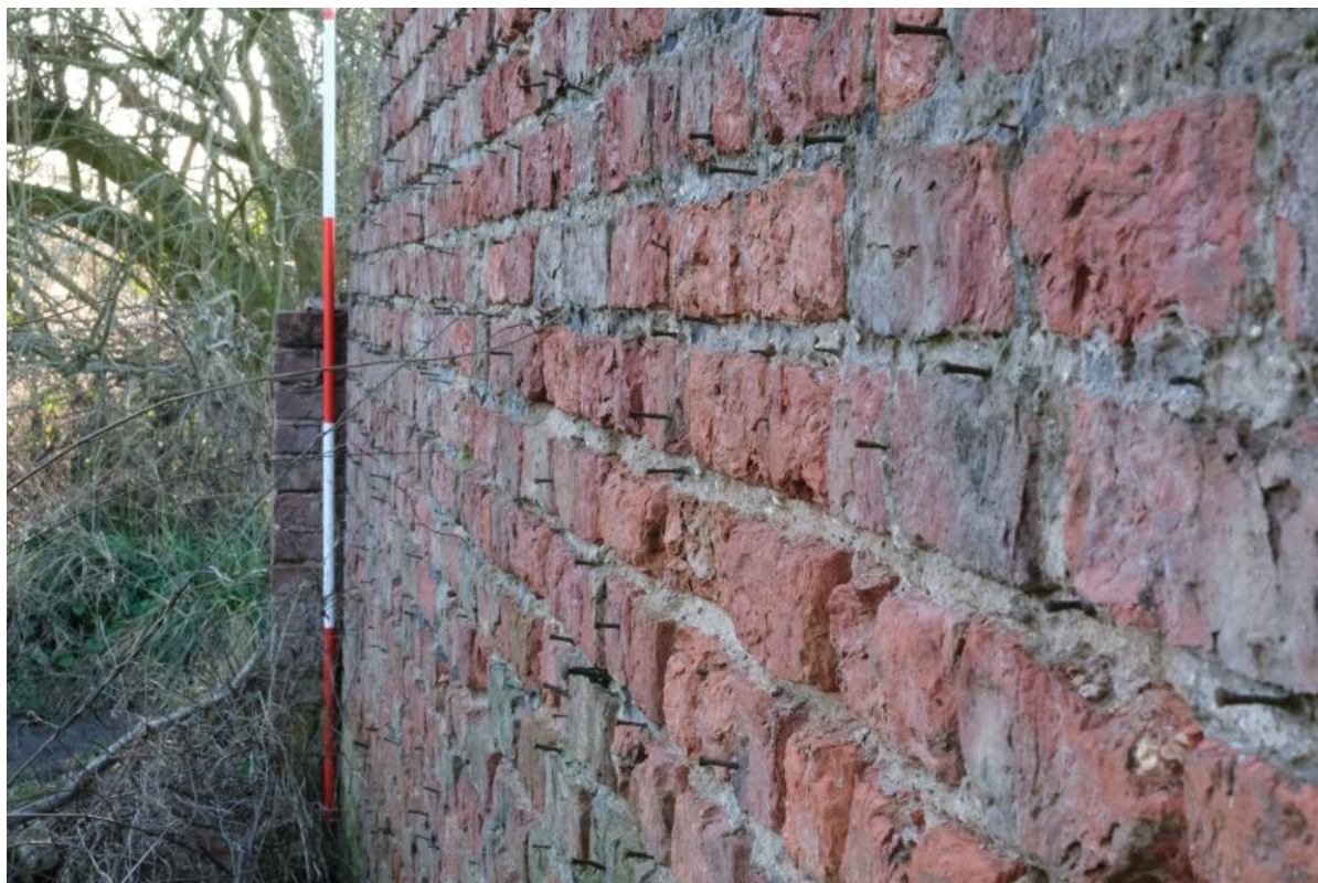
Plate 44: Nails in the north-eastern elevation of Wall B, facing south-east, scale unit 0.5m.
