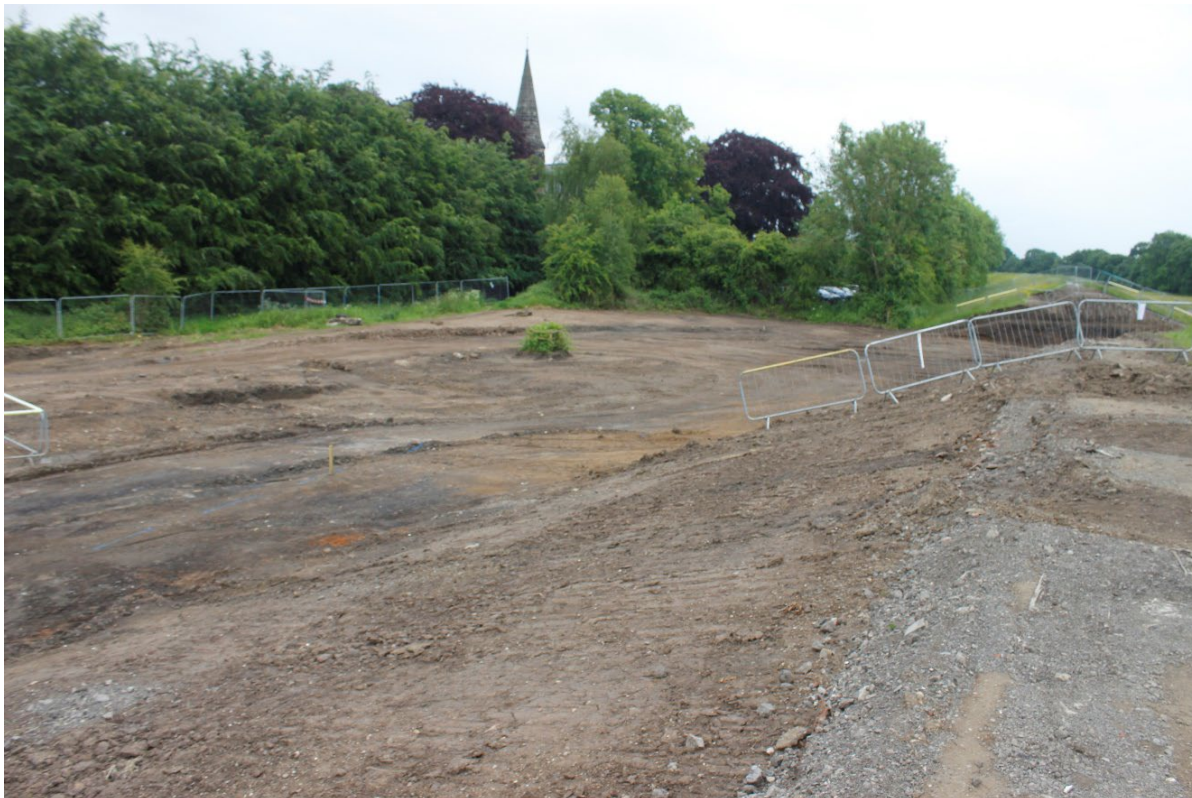
Plate 11: Northern Embankment area, looking northeast.
