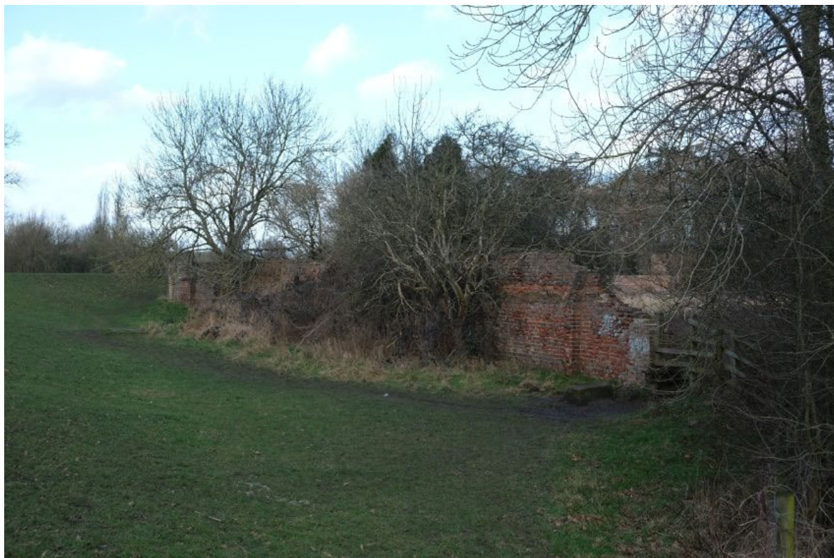
Plate 34: General view of the south-western elevation of Wall B, facing north.
