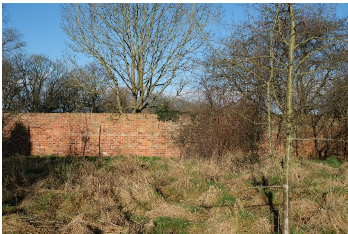
Plate 29: The south-eastern elevation of wall A, facing north-west, scale unit 0.5m.
