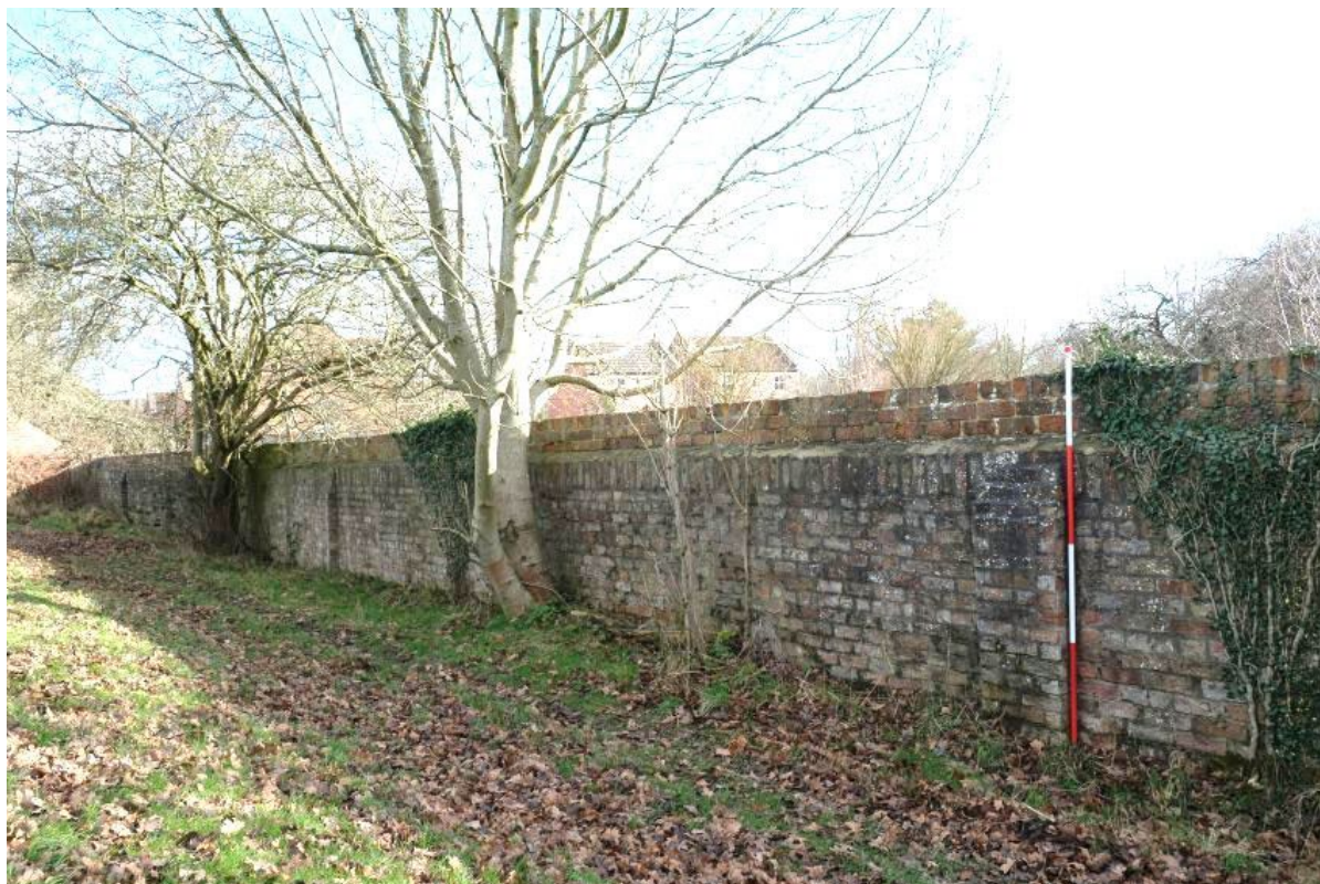
Plate 15: The north-eastern elevation of Wall A, facing north-north-east, scale unit 0.5m.
