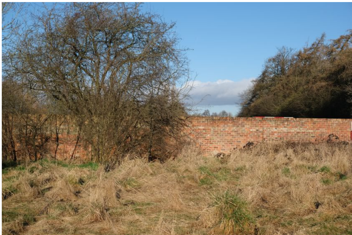
Plate 28: The south-eastern elevation of wall A, facing north-west, scale unit 0.5m.
