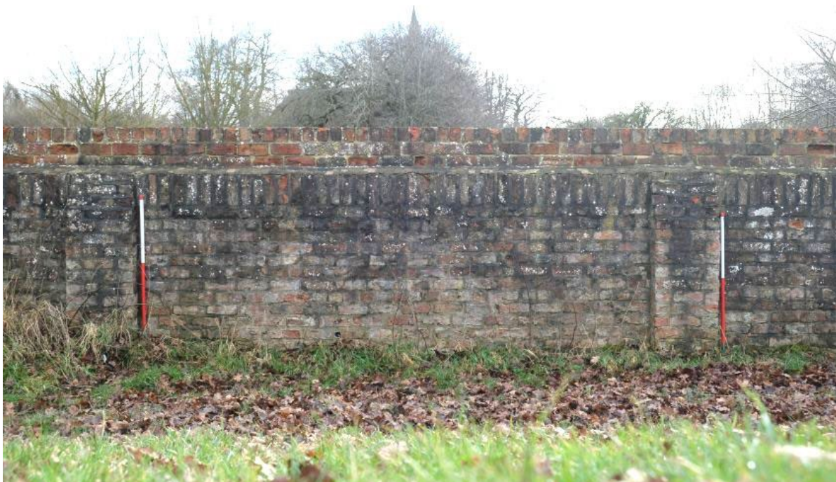
Plate 16: The brickwork in the north-eastern elevation of Wall A, facing south-east, scale unit 0.5m.
