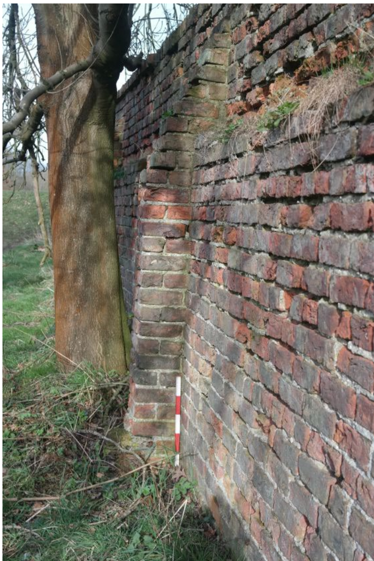
Plate 38: A buttress on the south-western elevation of Wall B, facing north-west, scale unit 0.1m.
