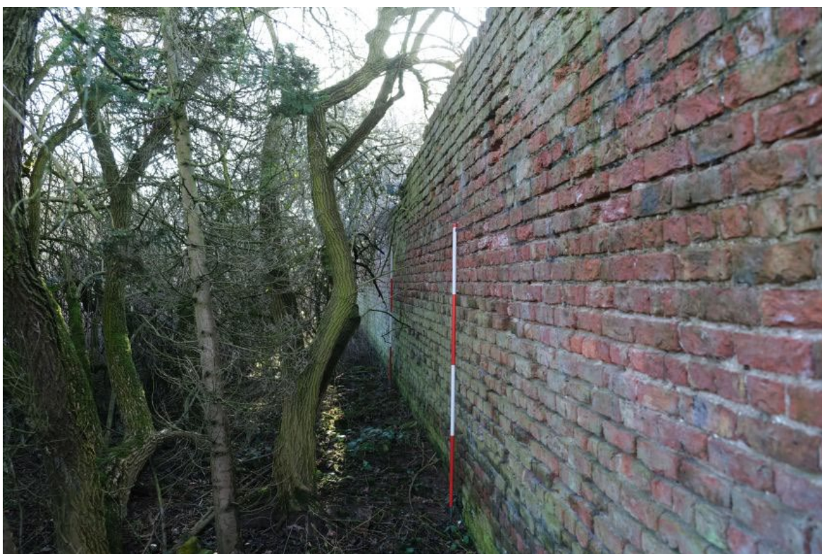
Plate 42: The north-eastern elevation of Wall B, facing south-east, scale unit 0.5m.
