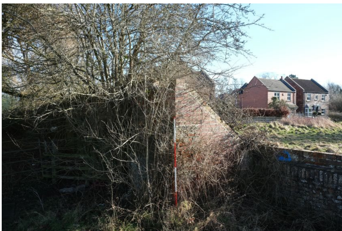
Plate 21: The dog-leg at north-eastern end of Wall A, facing north-east, scale unit 0.5m.
