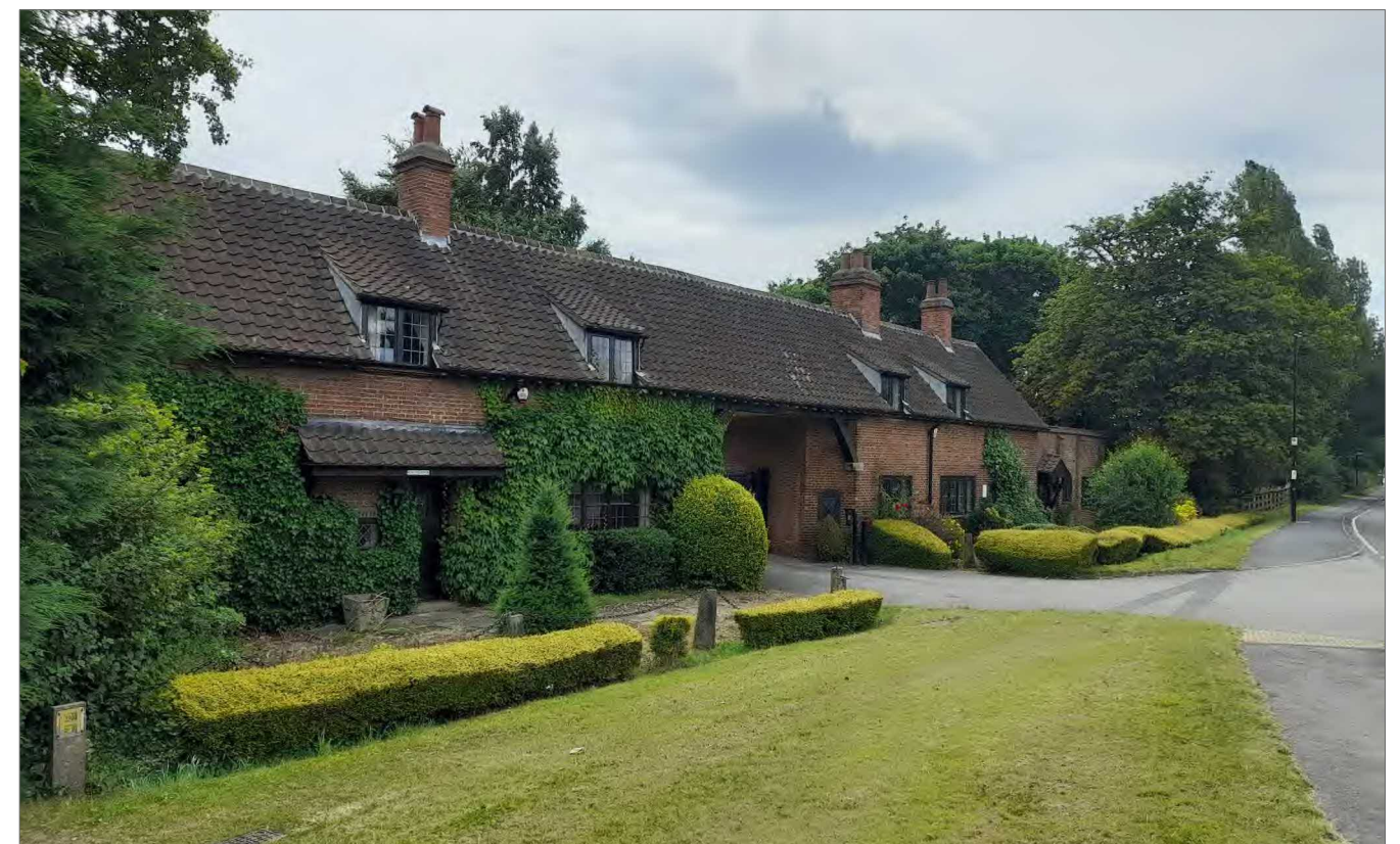
Plate 8: Garth Cottage and Garth Mews (1132494), facing south-east
