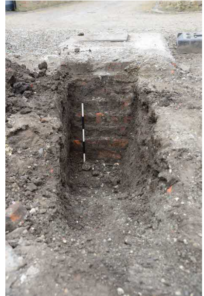
Plate 6 Excavations to connect to existing manhole, looking northeast, scale 0.50m
