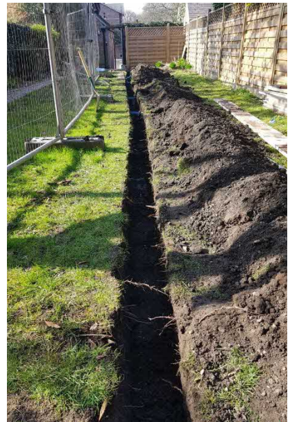
Plate 4 Service trench, looking south
