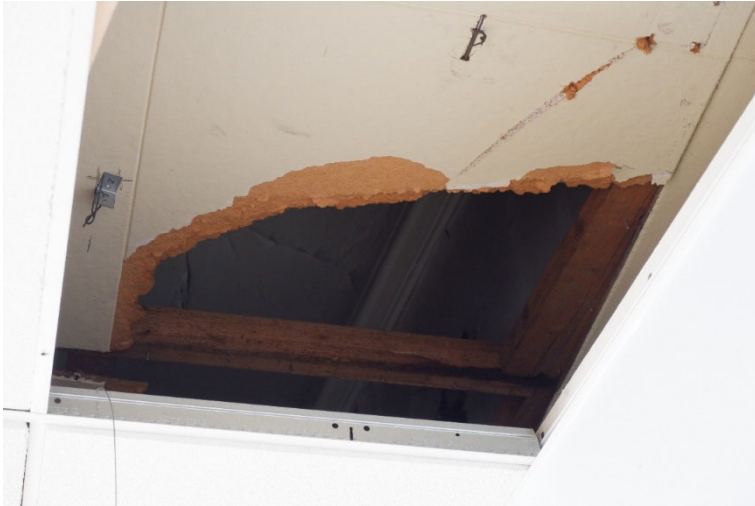
Surviving cornice above two suspended ceilings at ground floor.
