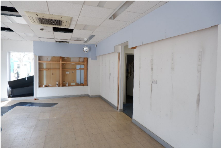
Ground Floor – Modern partitions, suspended ceiling and floor finish to be removed
