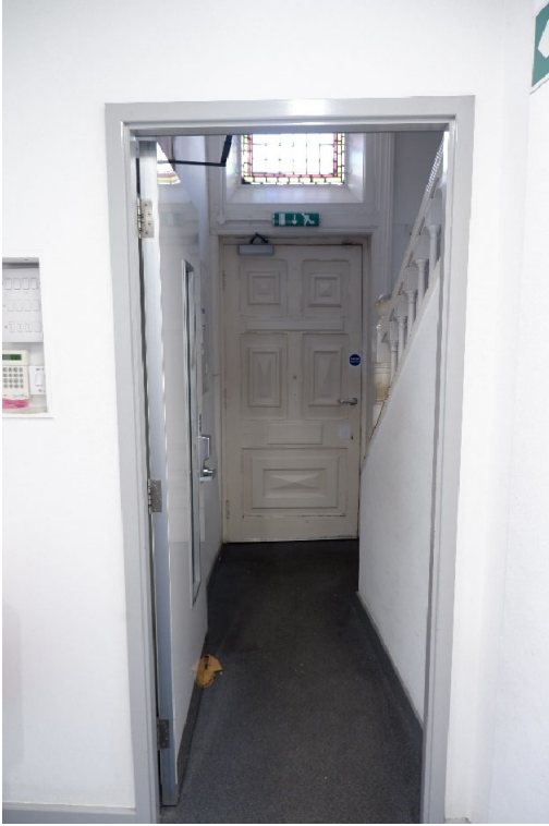
Ground Floor – Modern door to be removed (foreground)
