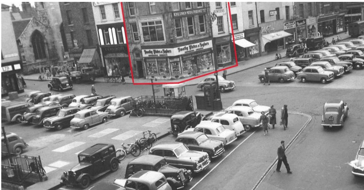
Photograph dating to 1957 showing the ground and first floors of 22-23 Parliament Street
