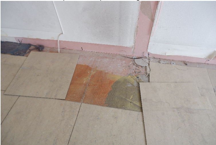
Ground Floor – Modern floor finish to be removed
