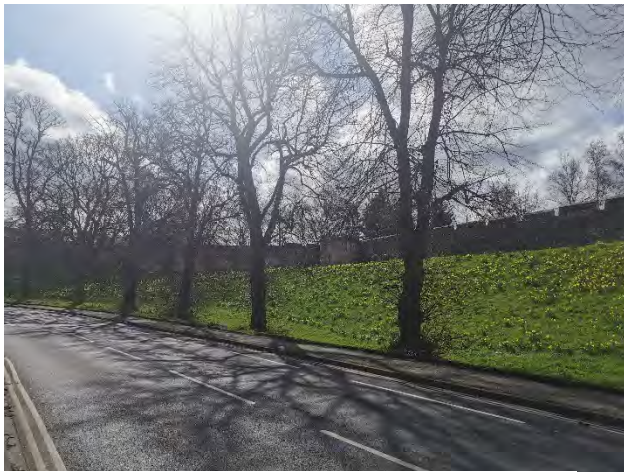
Photo 7) View of City Walls (NHLE 1004910) from Jewbury, south-west
