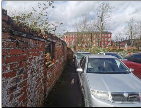
Photo 2) View of eastern Site boundary, looking north
