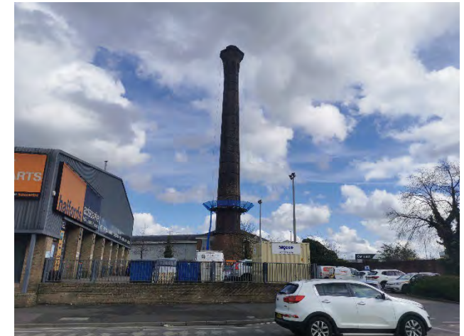
Photo 12) View of Chimney at Works and Services Depot of York City Council (NHLE 1257848), looking east
