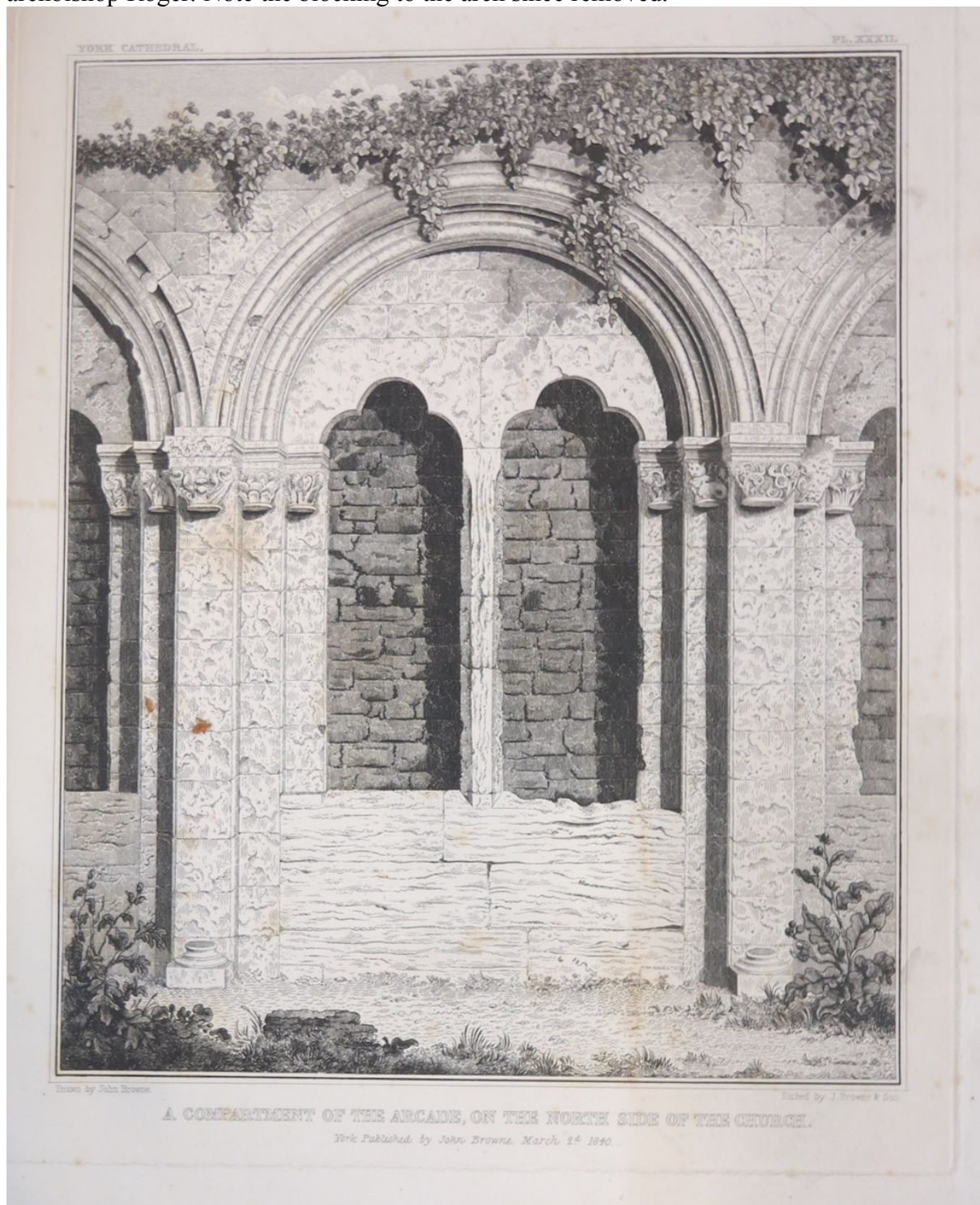
Below Fig 3: John Browne's drawing of one of the seven twelfth-century arches built by archbishop Roger. Note the blocking to the arch since removed.
