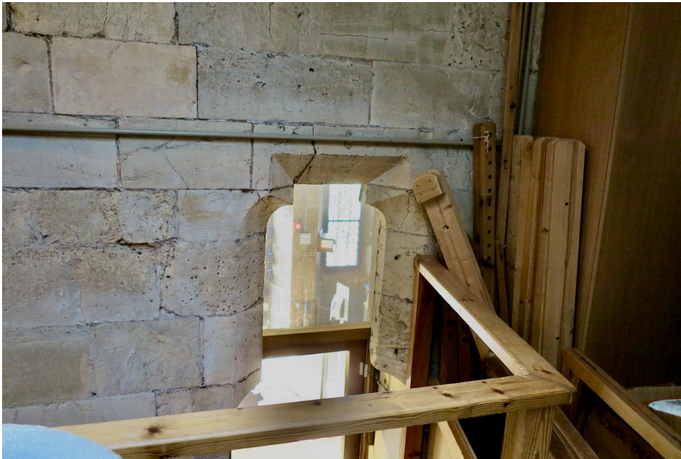
Below Fig 15: Caernarfon type of shouldered arch, actually a linteled opening in the east wall of the vestibule
