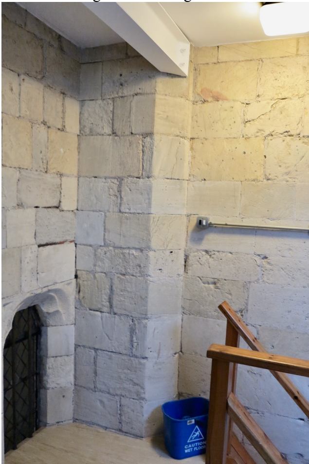
Below Fig 16: Corner junction between the chapel north wall and the vestibule east wall showing even coursing between the two walls.
