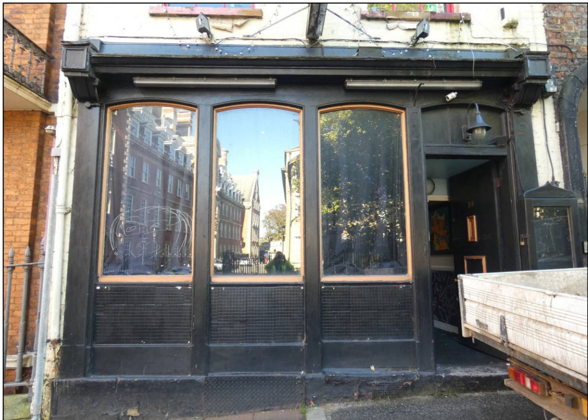
Plate 3: North (street) elevation, ground floor, looking SE (photo 1/815).
