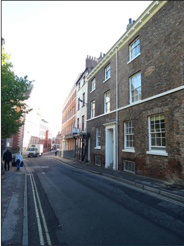
Plate 45: View of no. 39 along Tanner Row, looking E (photo 1/798).
