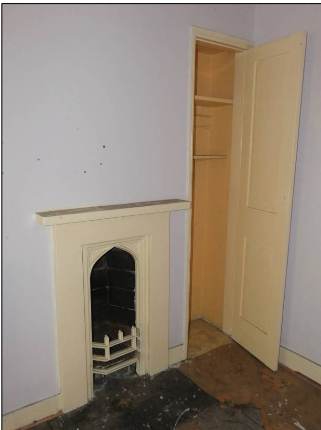
Plate 38: Room 3F3, fireplace and cupboard to east wall, looking S (photo 1/891).
