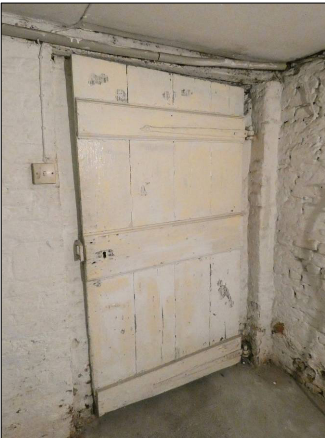
Plate 14: Cellar room B1, inside face of door, looking W (photo 1/857).
