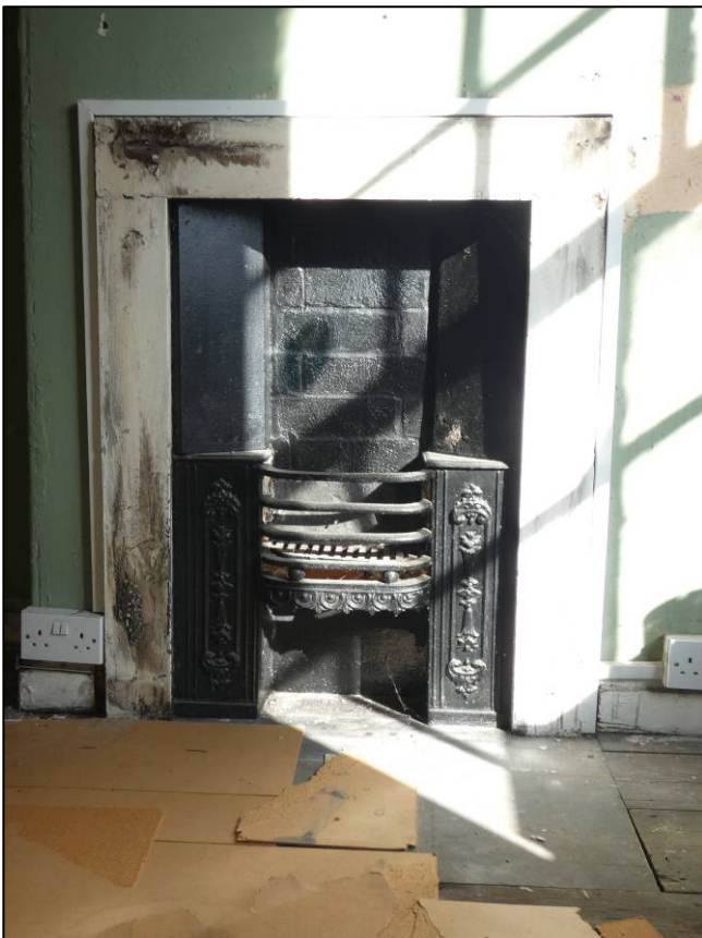
Plate 35: Room 2F4, fireplace to east wall, looking NE (photo 1/882).
