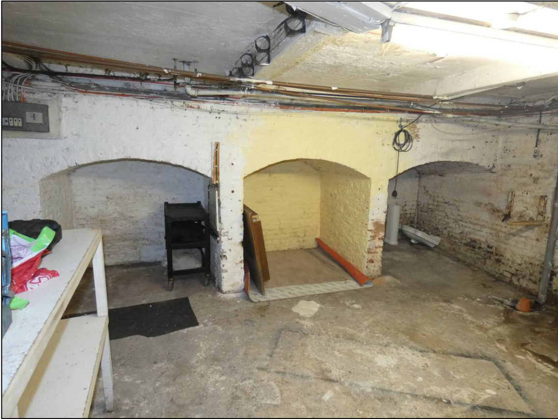
Plate 13: Cellar room B2, storage bins in west wall, looking W (photo 1/847).
