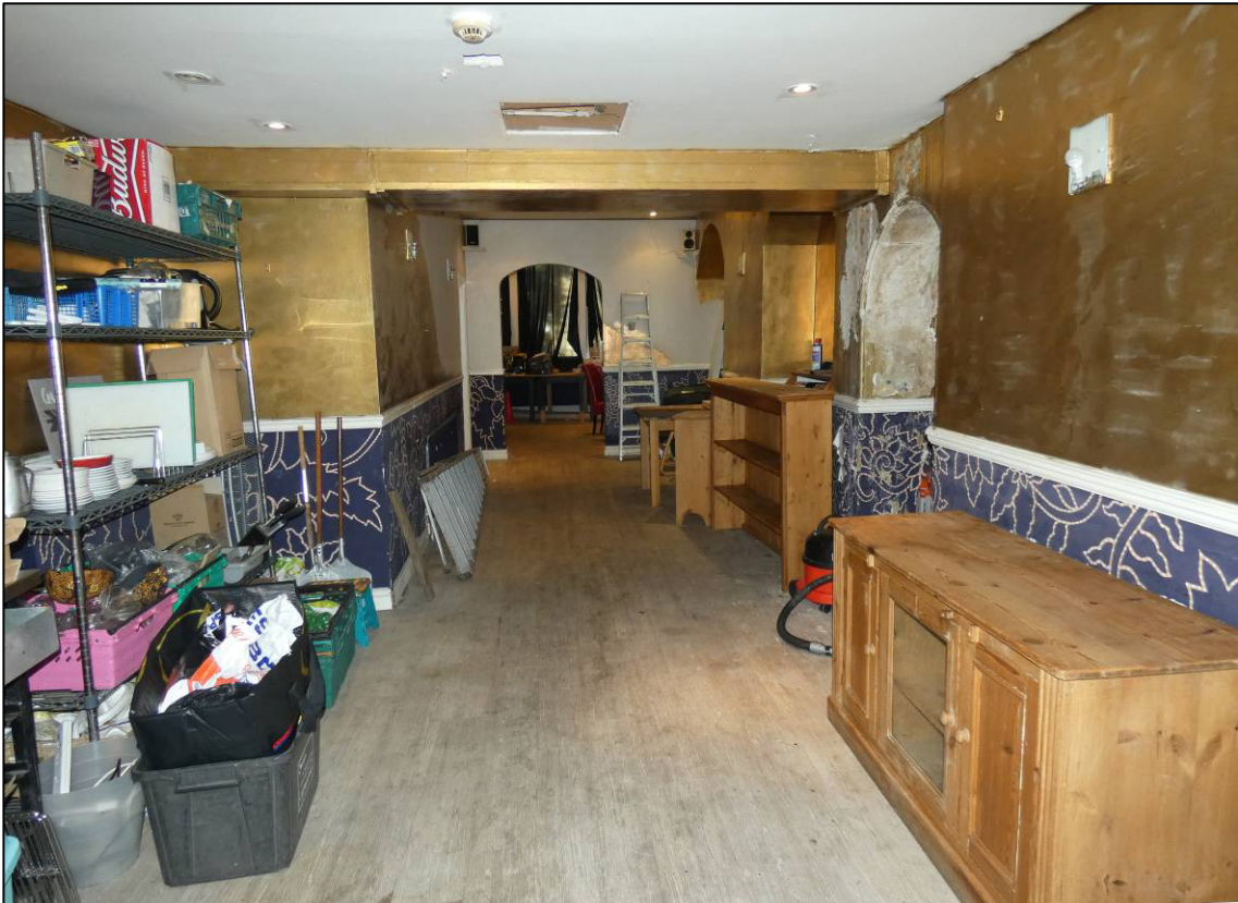
Plate 19: Room GF2, showing central ceiling beam, looking NW (photo 1/821).
