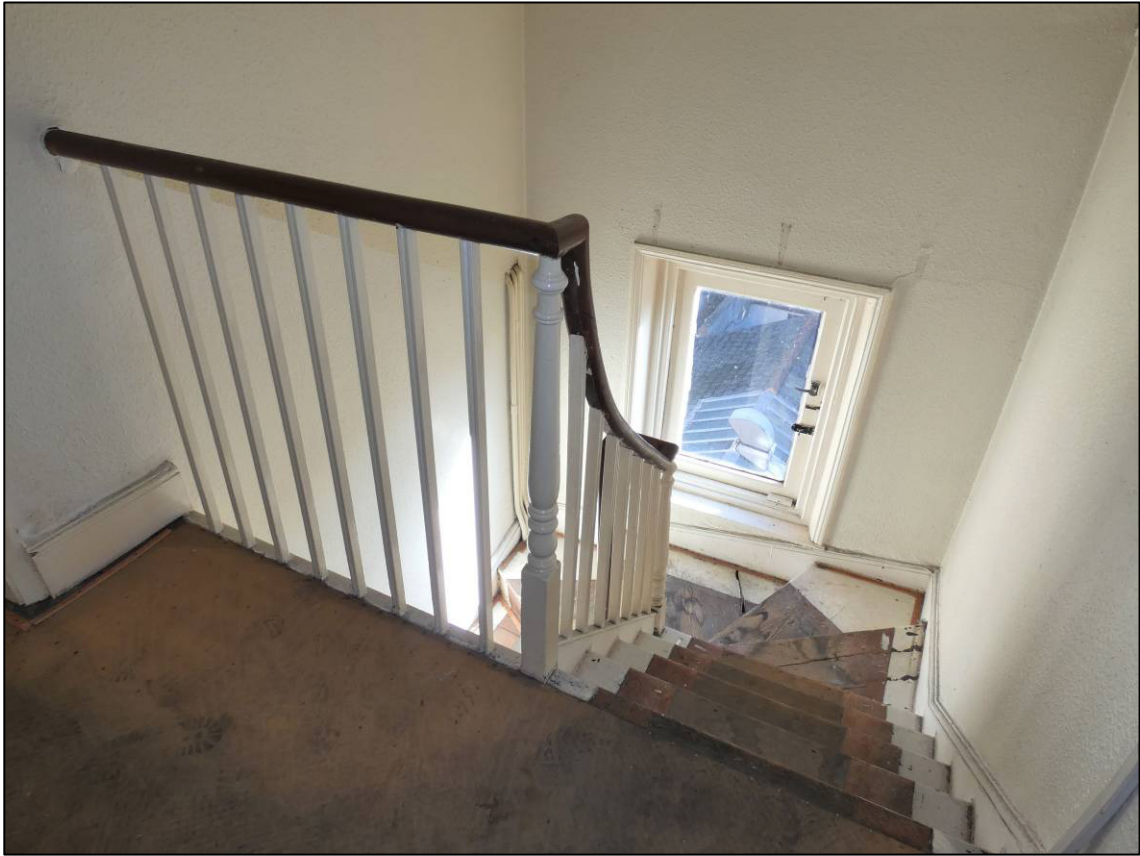
Plate 37: Room 3F1, looking SW (photo 1/897).
