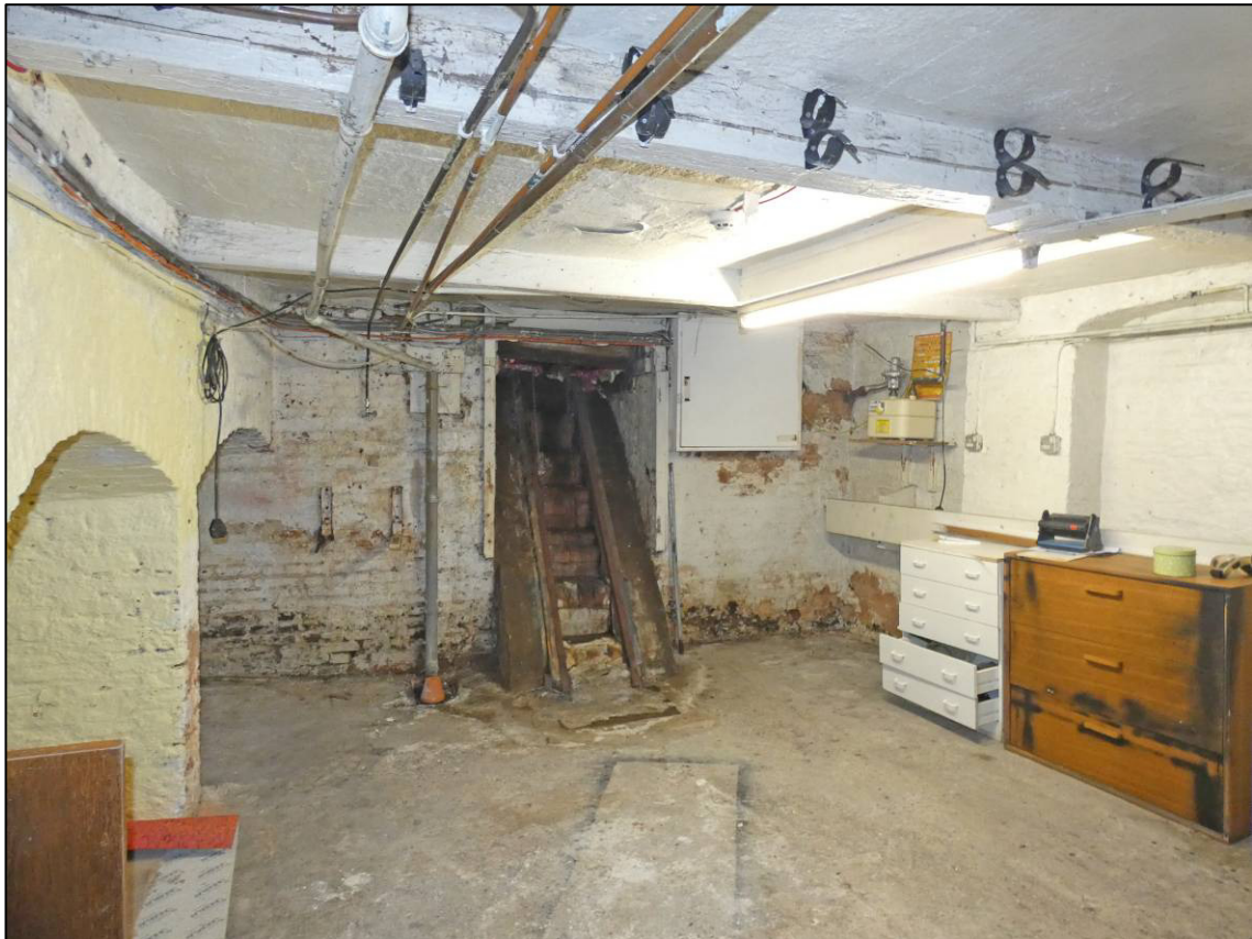
Plate 12: Cellar room B2, north wall, looking NW (photo 1/845).
