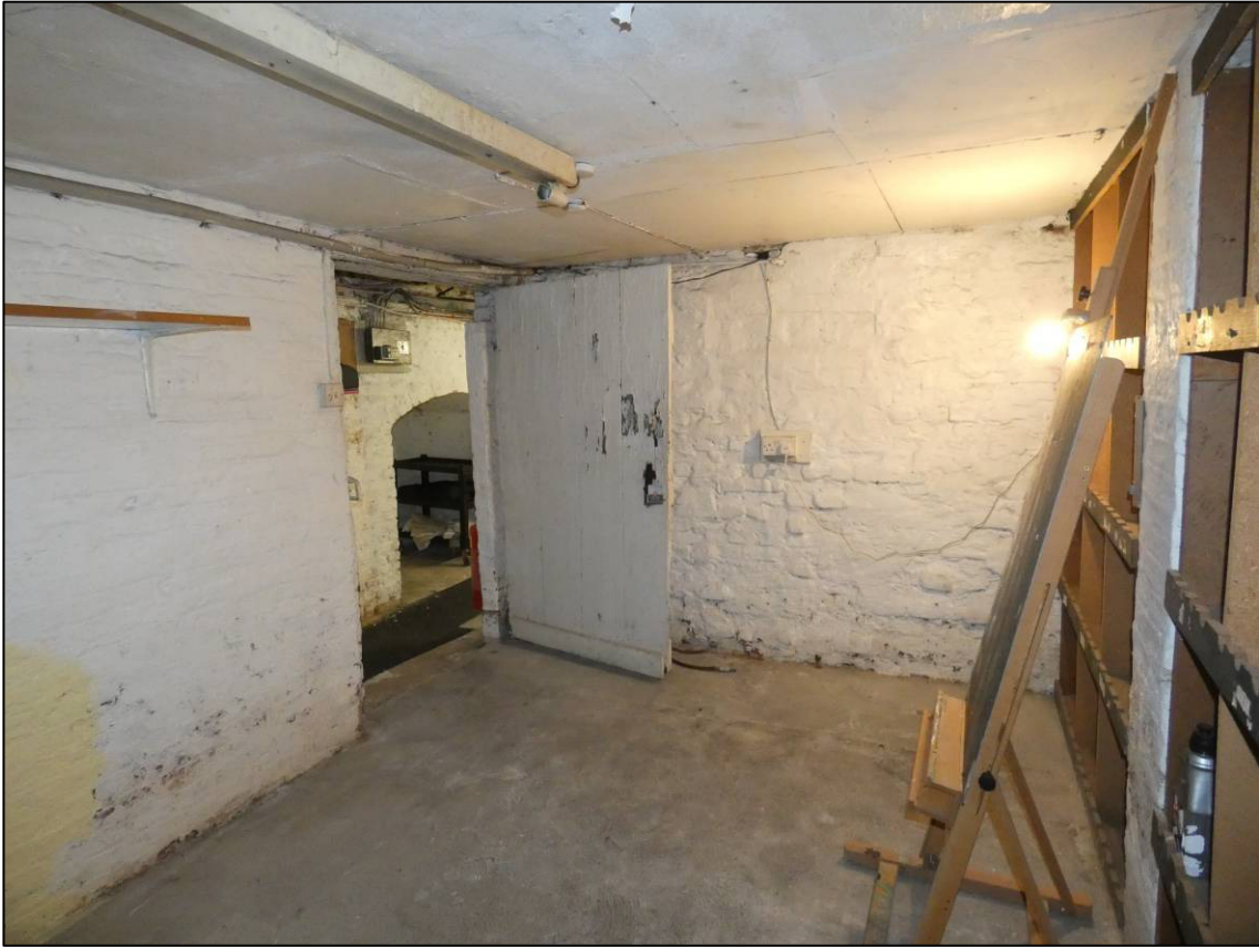
Plate 16: Cellar room B1, looking NW (photo 1/850).
