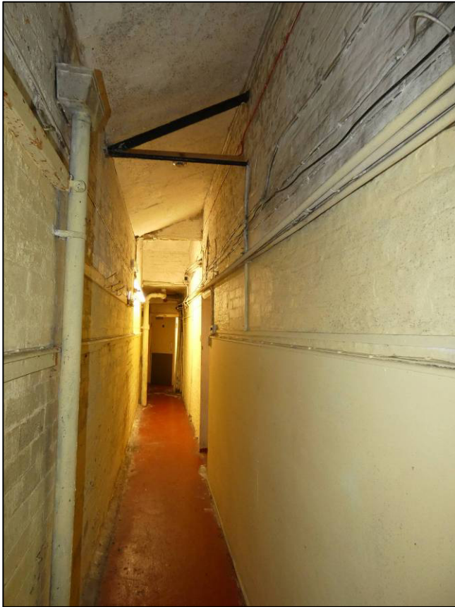
Plate 24: Passage GF3, blocked window to east wall, looking NW (photo 1/844).
