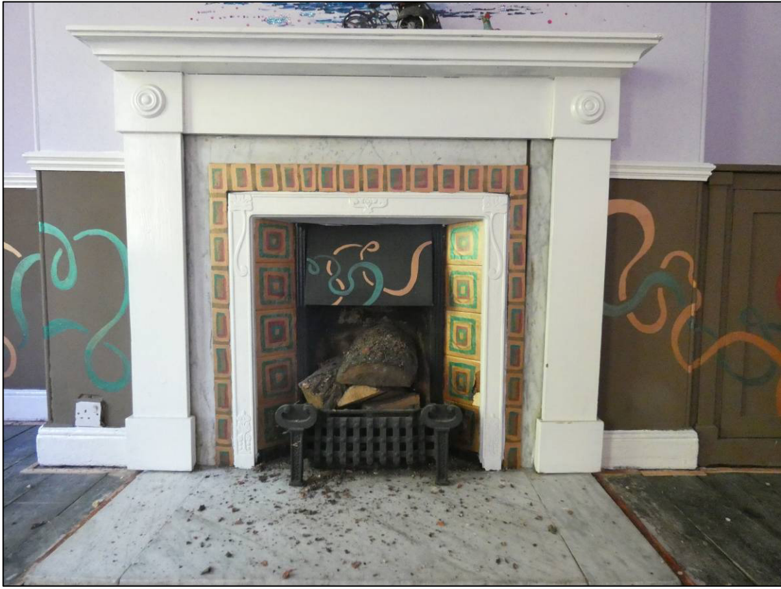
Plate 27: Room 1F2, fireplace to east wall, looking NE (photo 1/864).
