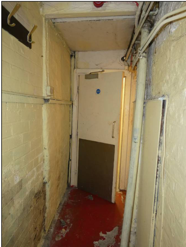
Plate 22: Passage GF3, north end, showing thickened west wall, looking NW (photo 1/841).
