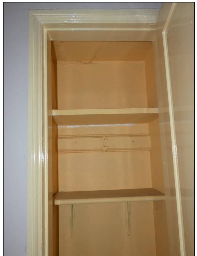
Plate 39: Room 3F3, cupboard to east wall, looking E (photo 1/892).
