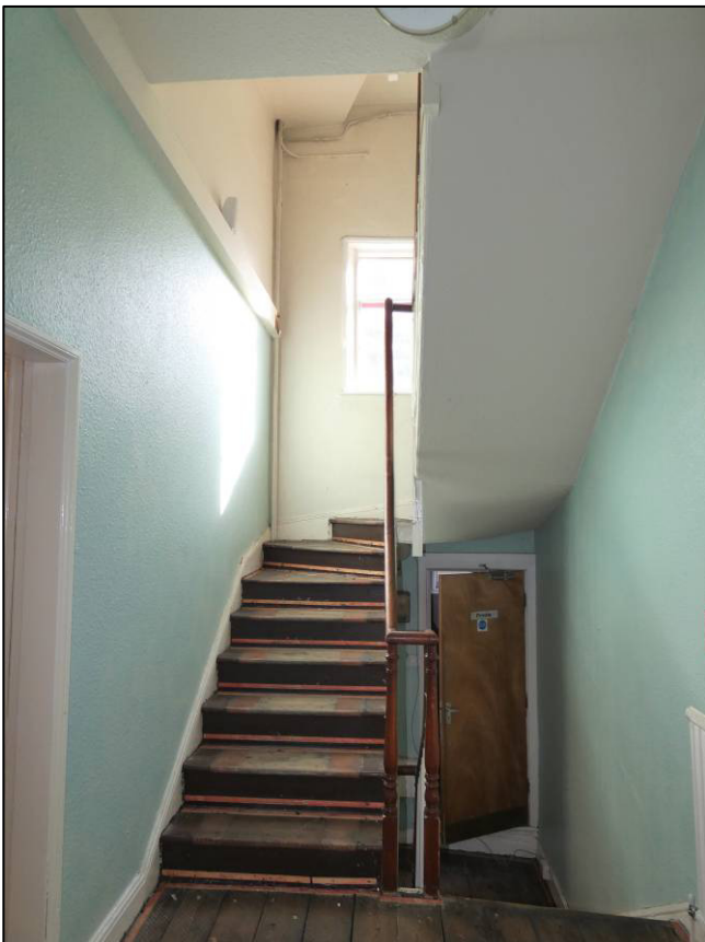
Plate 31: Room 1F1, stairs and door to toilet, looking SE (photo 1/870).
