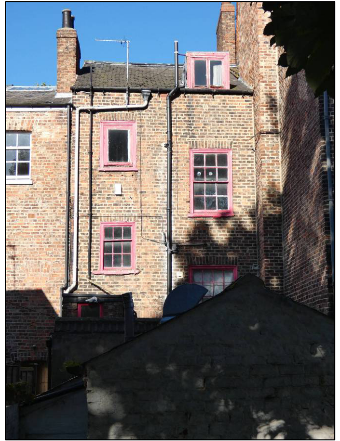
Plate 5: South (rear) elevation, looking NW (photo 1/836).
