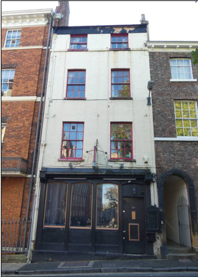
Plate 1: North (street) elevation, looking SE (photo 1/788).
