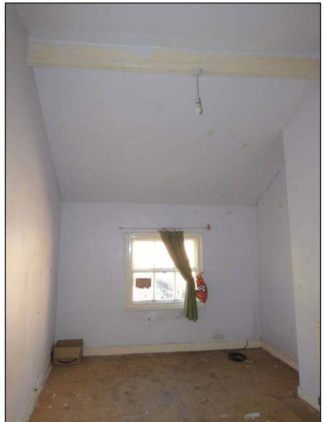
Plate 36: Room 3F3, looking NE (photo 1/890).
