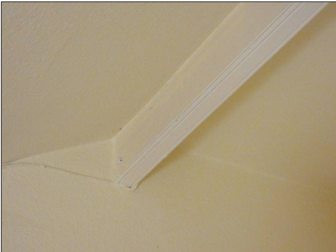
Plate 42: Room 3F4, visible part of roof truss over, looking NE (photo 1/888).
