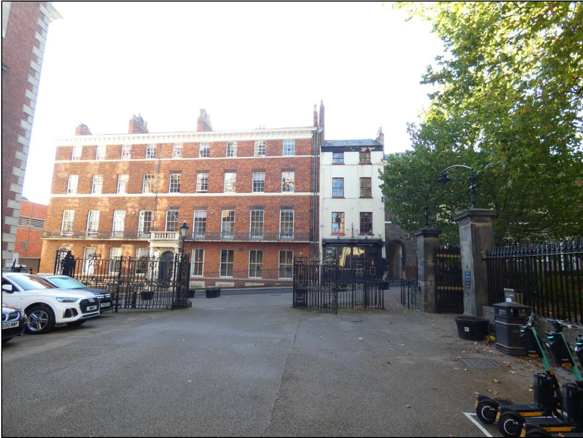
Plate 43: View of nos 37 and 39 Tanner Row from Station Rise, looking SE (photo 1/791).
