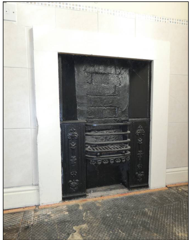
Plate 30: Room 1F3, fireplace to east wall, looking NE (photo 1/868).
