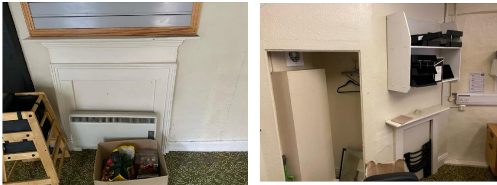
Figure 17 Blocked up fireplace on the second floor of 46 and 50.
