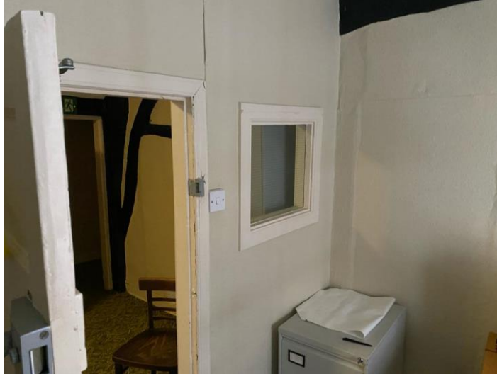
Figure 16 Partition dividing the room on the second floor of 48
