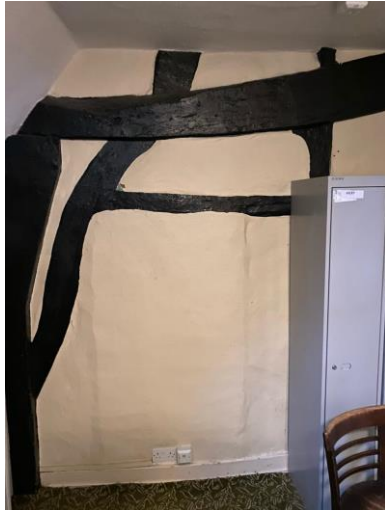
Figure 18 Timber posts and braces visible on the second floor between 46 and 48
