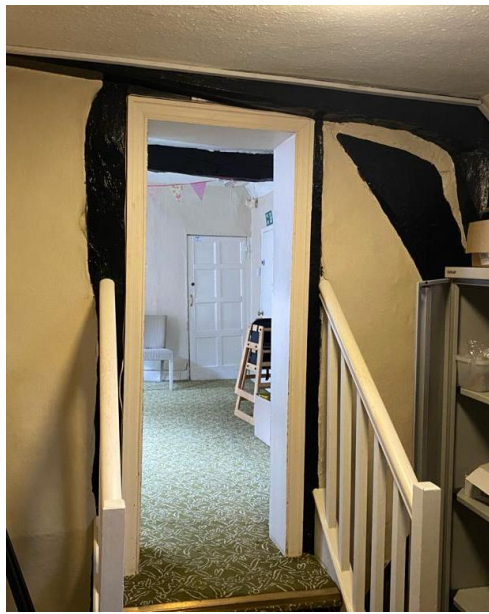
Figure 6 Existing doorway inserted in between 46 and 48 to connect the two buildings.
