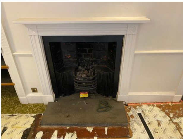
Figure 4 Fireplace on the first floor front room of 46
