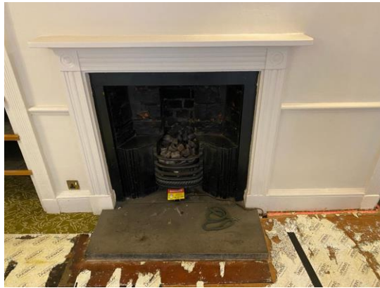
Figure 13 Fire place on first floor of 46
