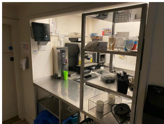
Figure 15 Existing prep kitchen on first floor, infill opening
