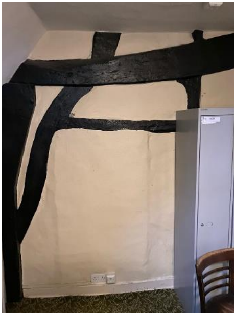
Figure 7 Timber posts and braces visible on second floor
