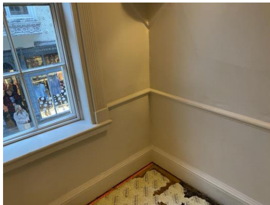
Figure 12 Reeded window architrave on first floor of 46
