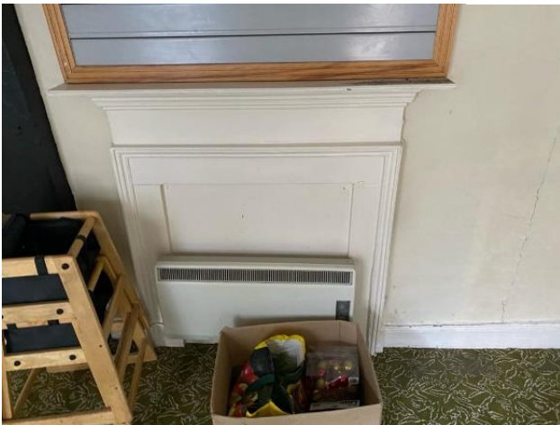
Figure 5 Blocked 18th century fireplace on the second floor of 46
