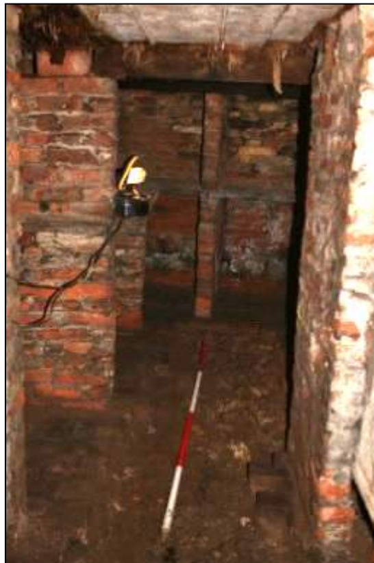
Plate 2. The northern “store-room” area. Looking East.
