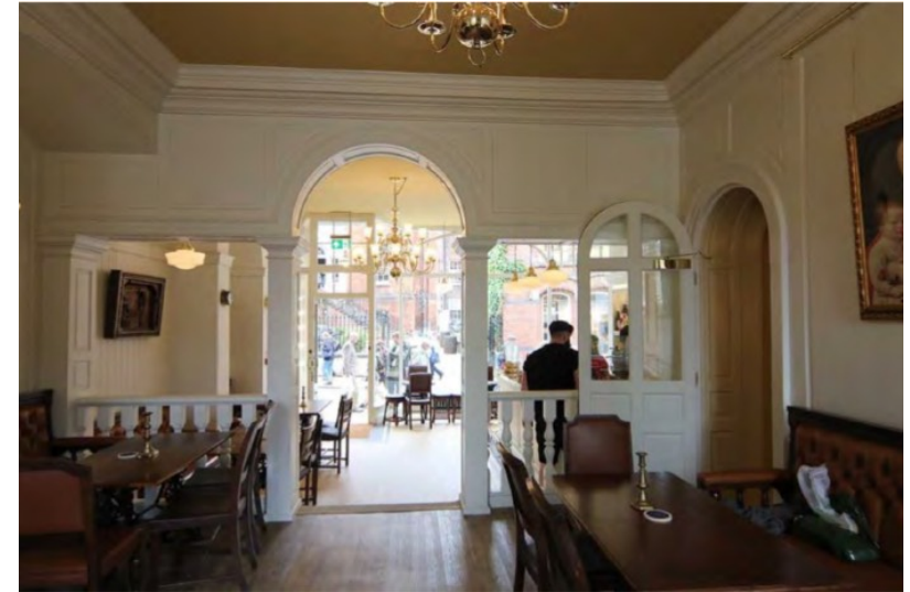
RESTORATION Archway restored to ground floor of 14 Lendal. New timberwork made to exactly replicate the original fabric by tracing their outline in the original paintwork
