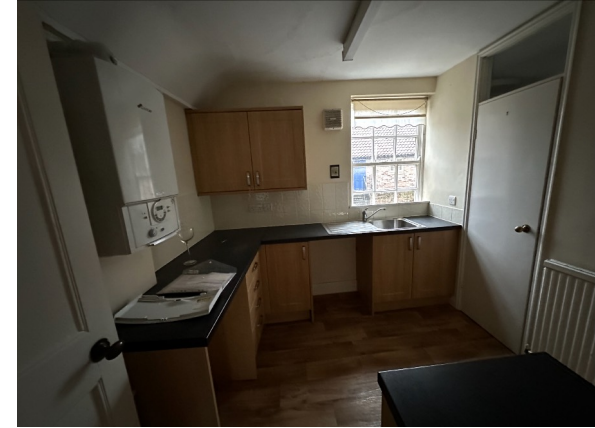
Redundant FF kitchen with bathroom beyond - a spatial arrangement created in 1980.
