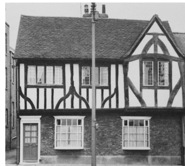
Figure 9 1970s photo showing the building following its 1930s restoration, including the new doorcase and two canted oriel windows at ground floor © RCHME.
