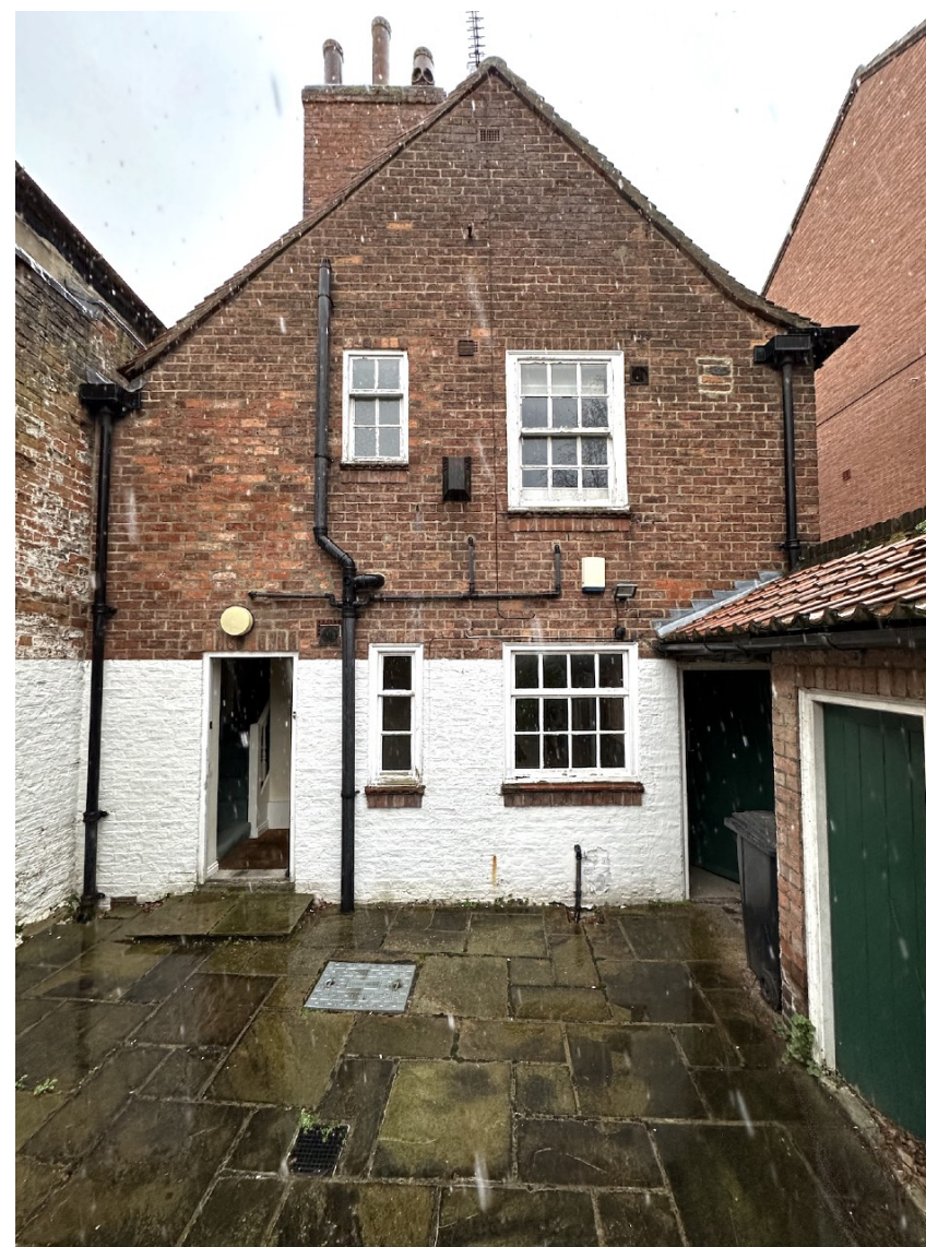
Figure 1 Existing rear elevation of no.77 Walmgate., with yard and outbuilding seen to the right.
