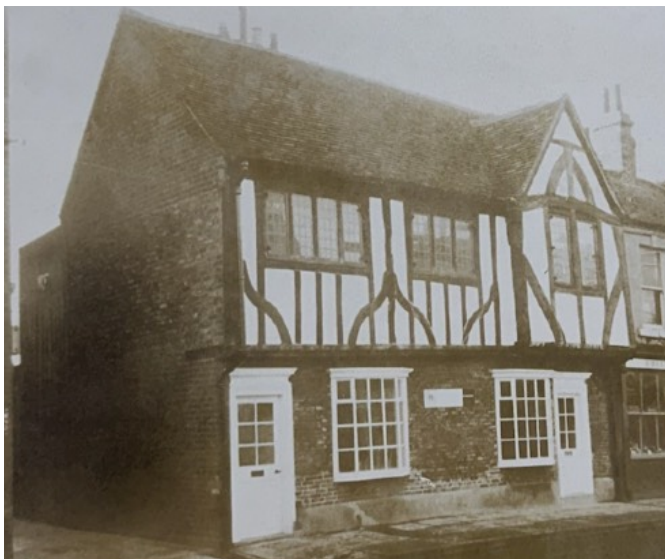
Figure 13 Photograph showing the front elevation following the 1980 alterations to form 2no. shops.
