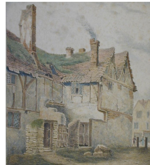
Figure 6 Example of a lost timber-framed building on Walmgate, by Henry Cave (1823) - showing its dilapidation and a common L-shaped plan with yard © YMT
