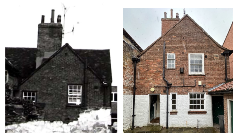
Figure 12 Left - 1971 photo showing the rear elevation and yard. Note the 1935 stair window on the left, prior to its infilling and creation of new bathroom window in 1980 (seen on current photo right).
