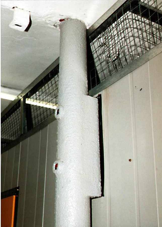
Plate 13 Warehouse - cast-iron column and bolting head
