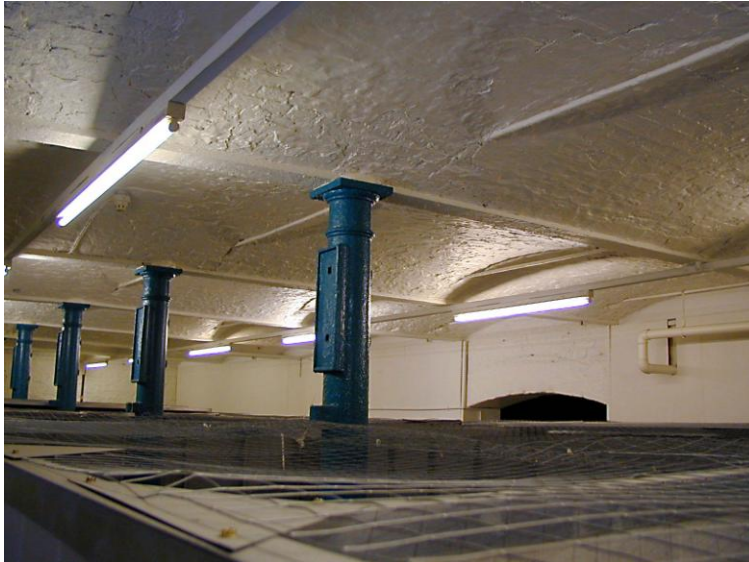
Plate 19 New Mill - detail of fireproof structure
