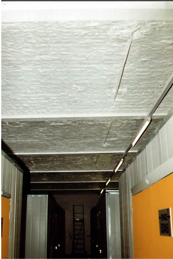
Plate 14 Warehouse - brick jack-arches
