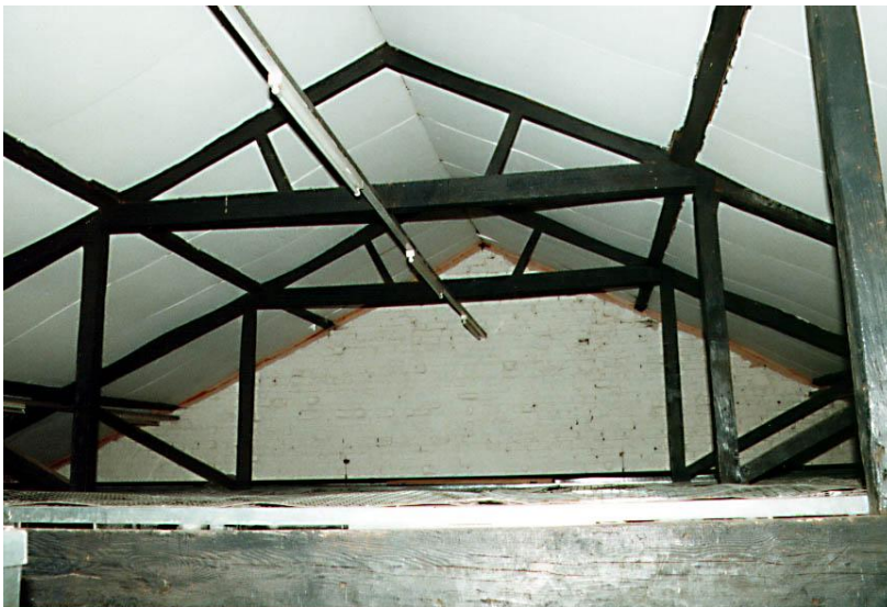
Plate 26 Boiler House - roof
