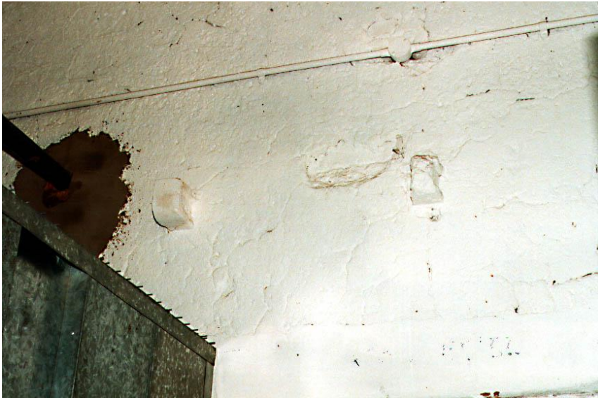
Plate 24 Engine House - corbels for internal stair
