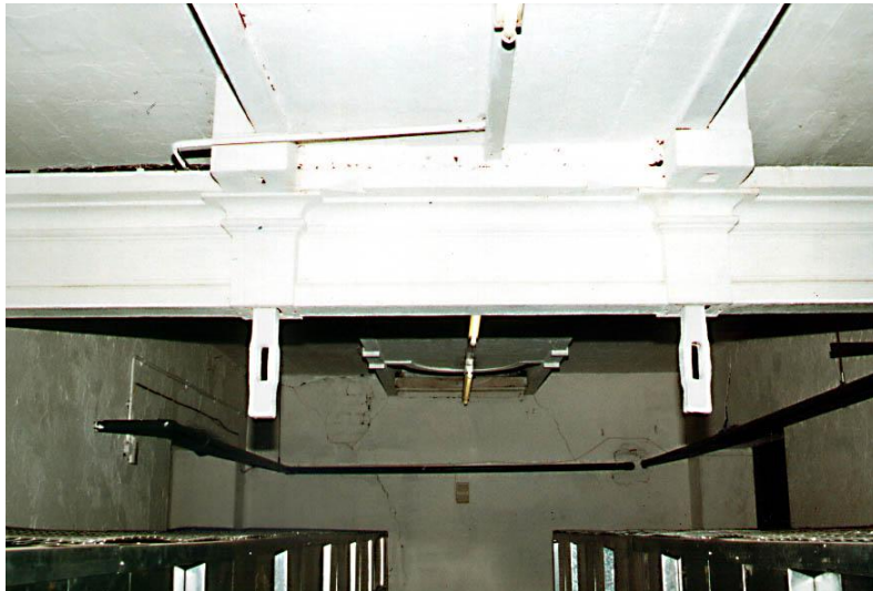
Plate 22 Engine House - entablature beam and lugs
