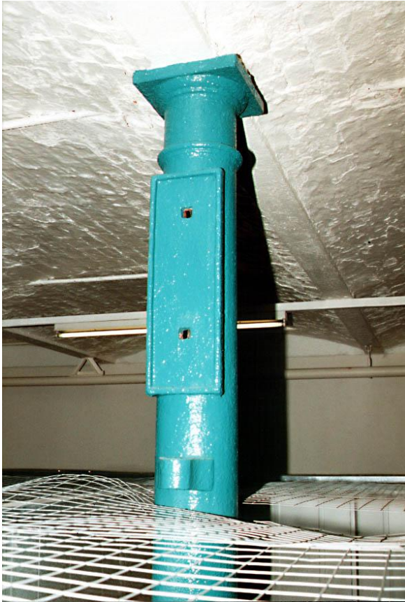
Plate 16 New Mill - cast-iron column
