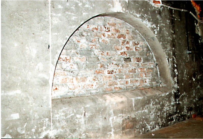
Plate 9 Old Mill - lunette window to north gable
