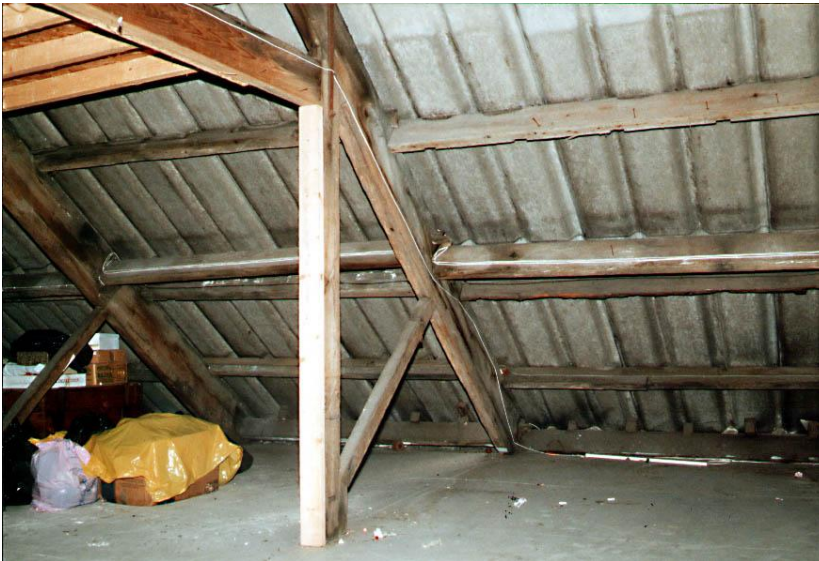
Plate 10 Old Mill - Roof Truss
