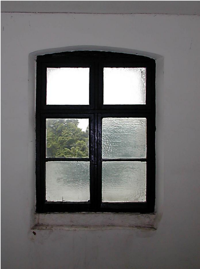
Plate 18 New Mill - window with obscured glass
