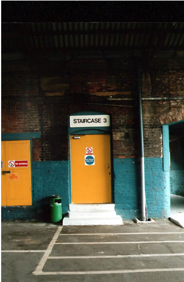
Plate 5 Old Mill - doorway to fireproof stair
