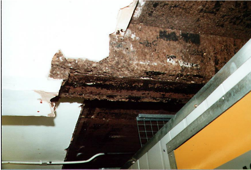
Plate 6 Old Mill - cork-lined steel and concrete structure to first floor
