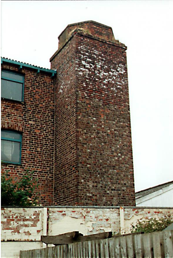
Plate 28 Chimney from south-west
