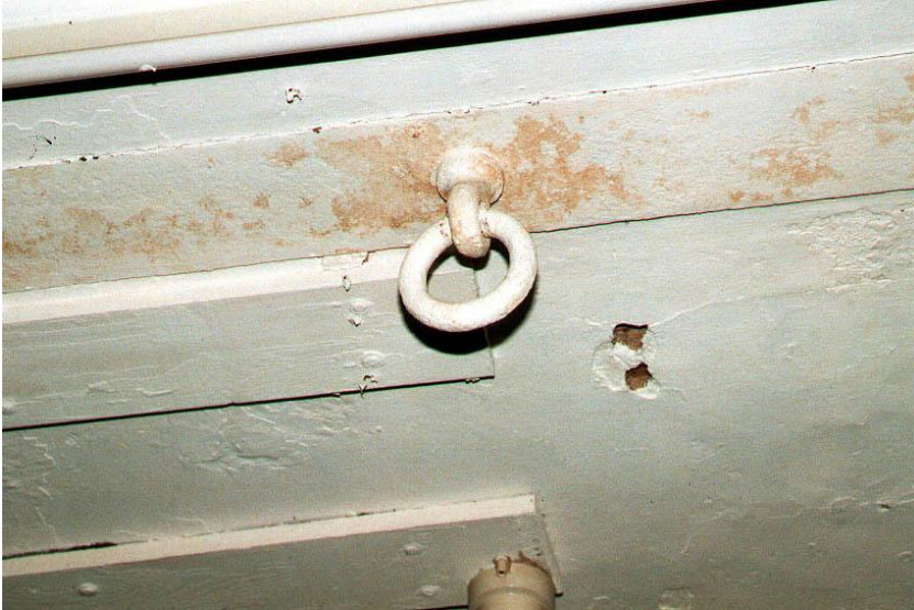
Plate 23 Engine House - cast iron joints and ring bolts for lifting gear
