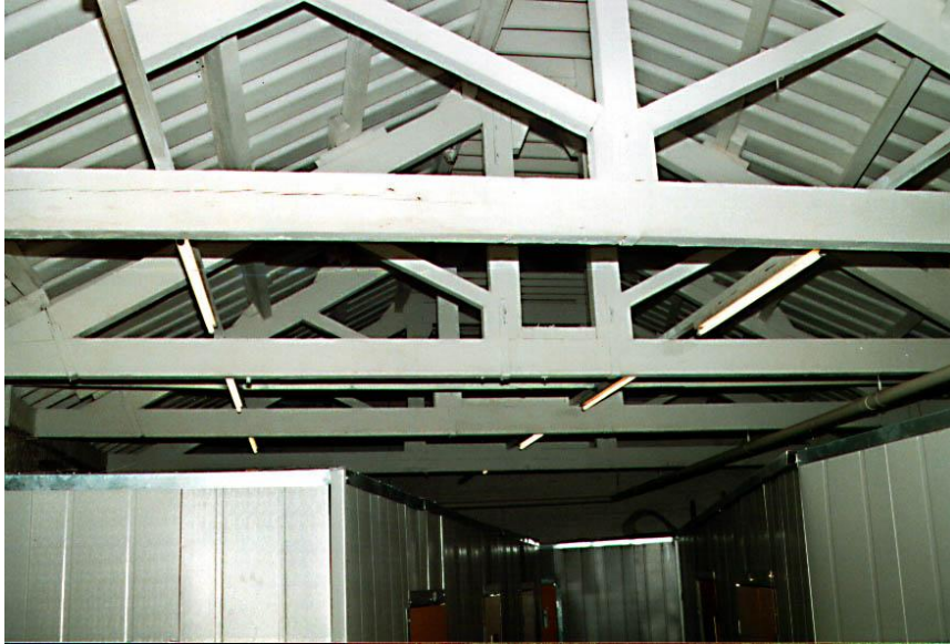
Plate 29 New Mill - roof to extension to west of mill
