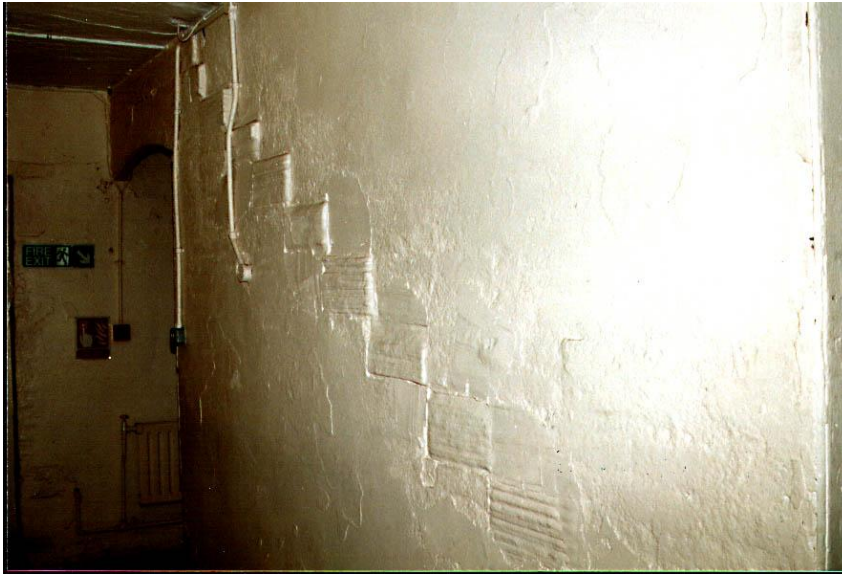
Plate 7 Old Mill - treads to fireproof stair
