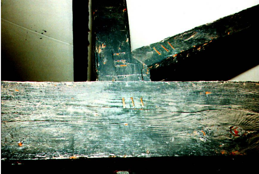
Plate 27 Boiler House - detail of truss to boiler house
