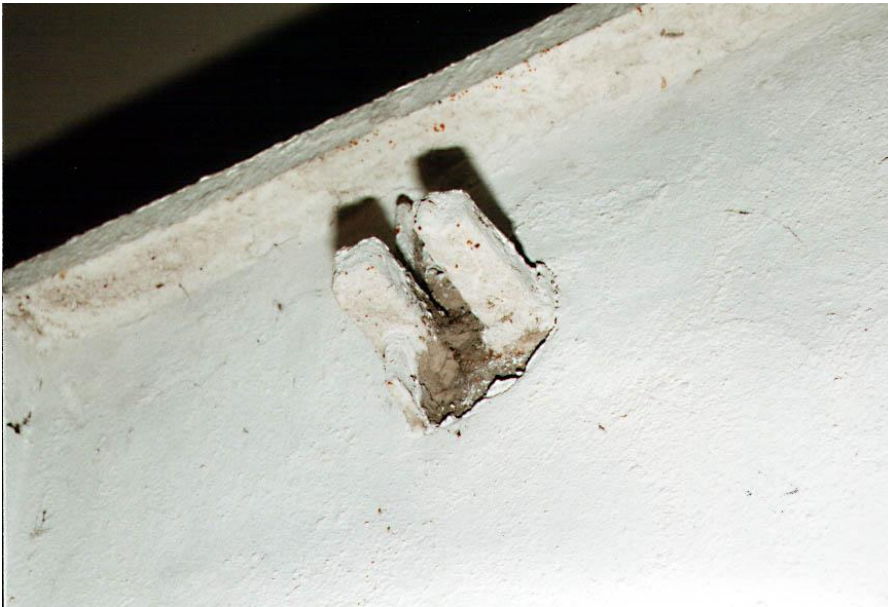
Plate 15 New Mill - detail of fixing of tension rods
