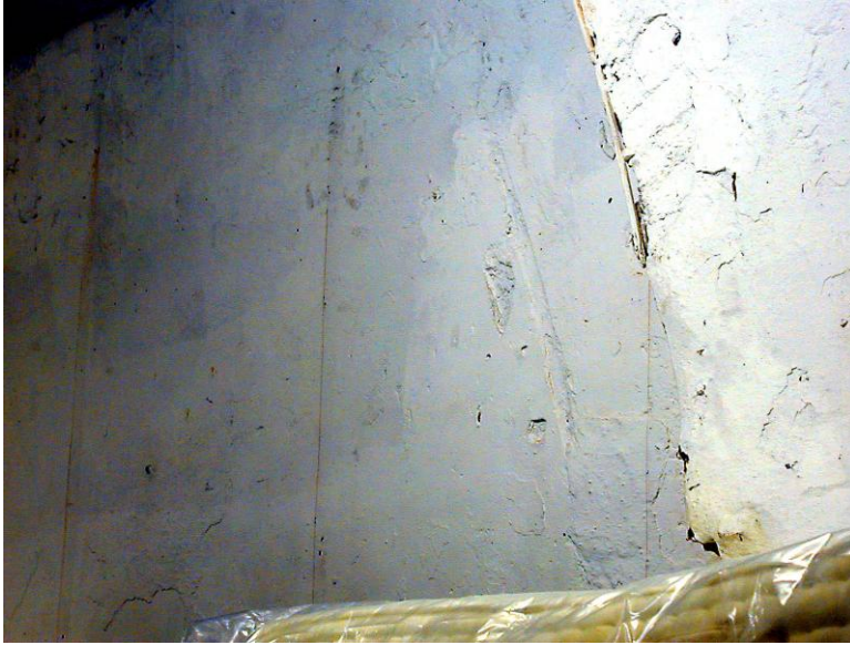
Plate 25 Engine House - detail of scoring of flywheel embrasure
