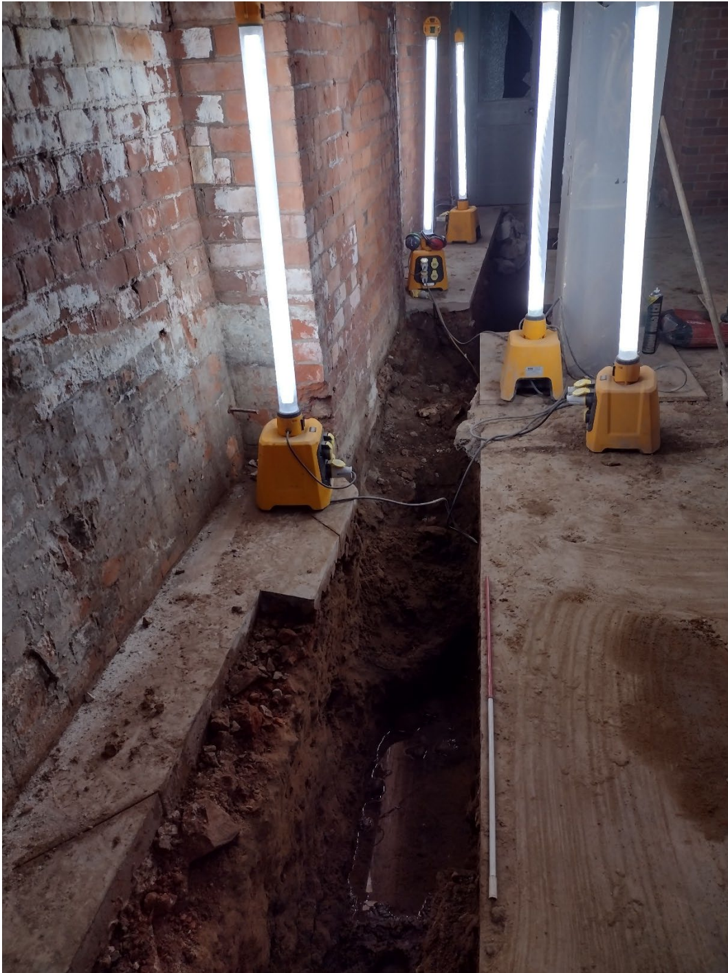
Plate 2: Trench 1, looking north-west, scale unit 0.50m
