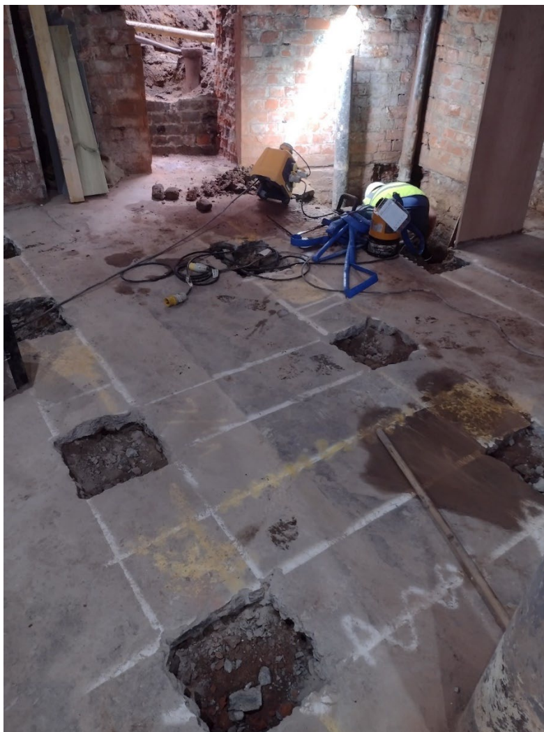
Plate 25: Working shot, basement pile positions, looking south-east
