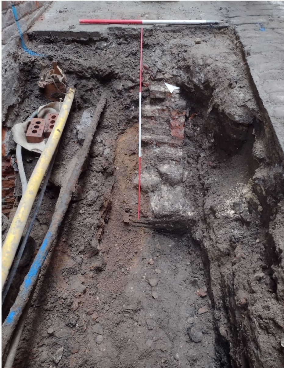
Plate 14: Trench 3 looking north-east, re-used medieval limestone wall blocks below post-medieval wall, scale unit 0.50m
