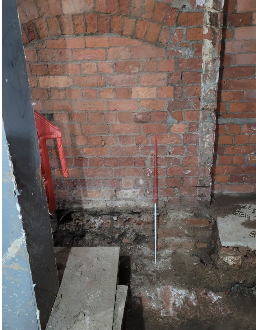
Plate 27: Blocked fireplace arch in south-western basement wall, scale unit 0.50m
