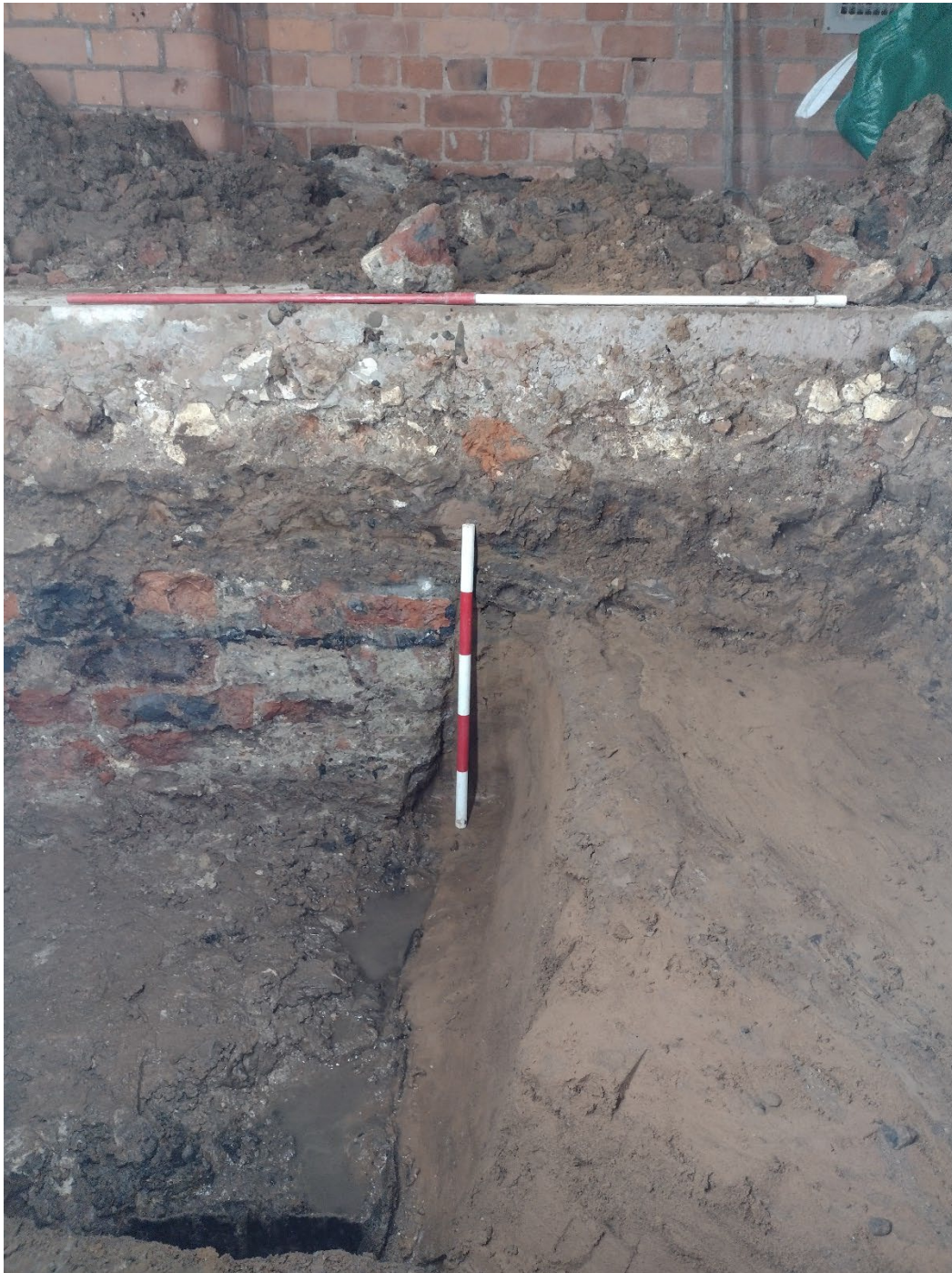
Plate 8: Trench 2 south-east facing section of wall C2021 and construction cut [C2023] with shuttering C2024 and bedding C2027, scale units 0.50m, 0.10m
