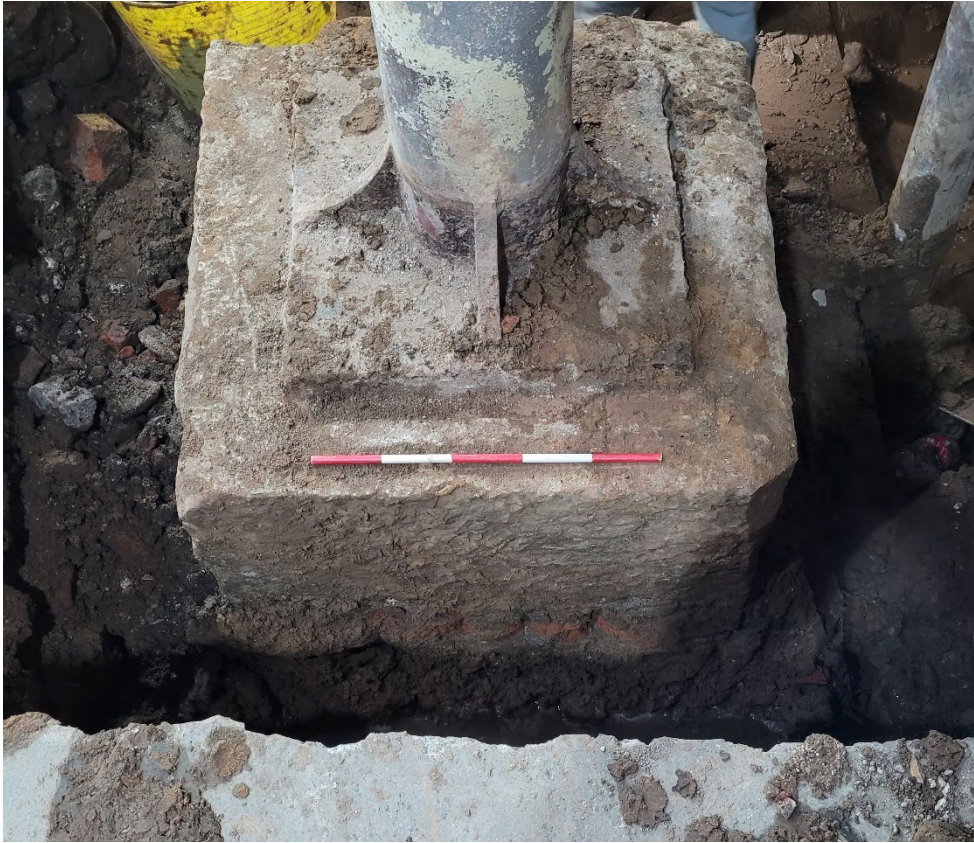
Plate 26: Re-used medieval limestone block in basement column foundation, looking east, scale unit 0.10m
