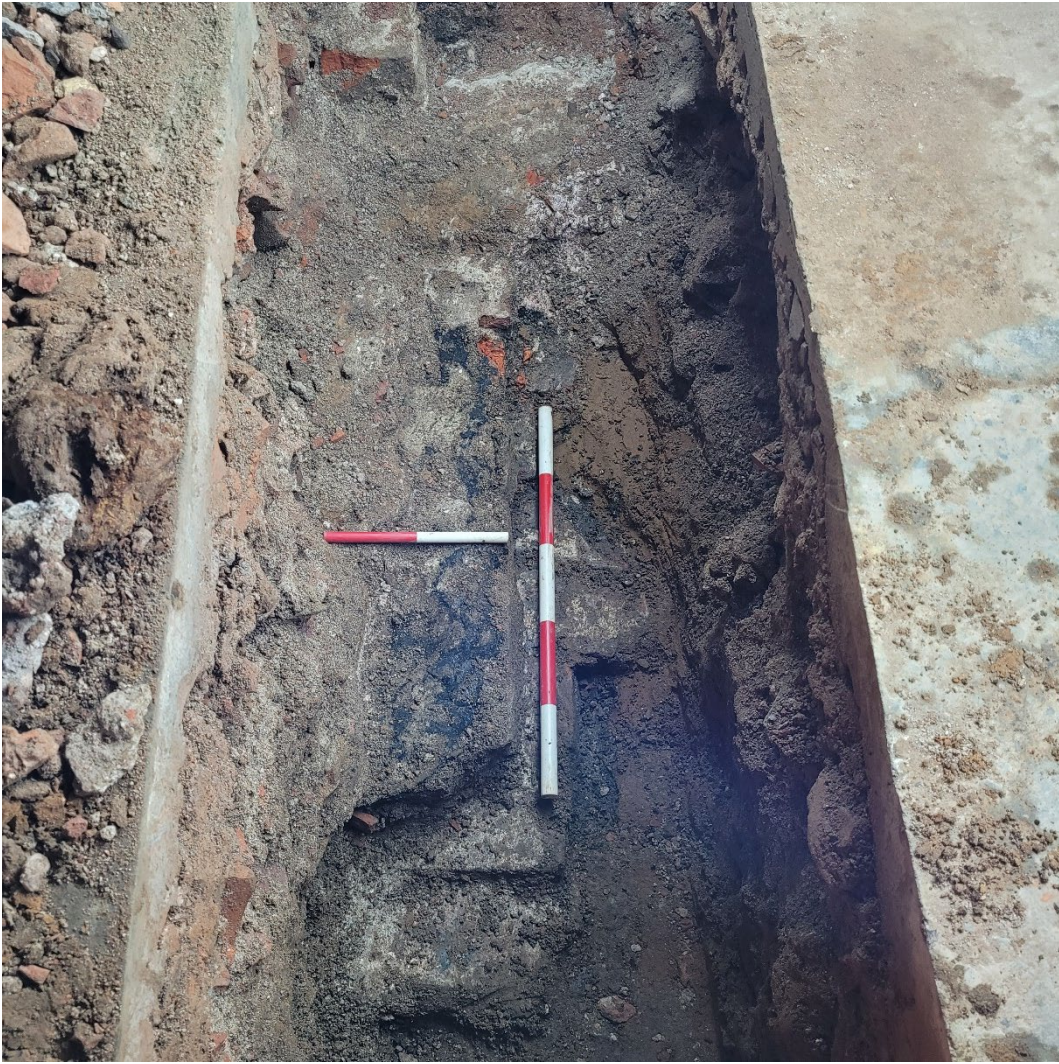
Plate 9: Trench 2 the south-west end of wall C2021 showing bitumen DPC and limestone foundation, scale unit 0.10m
