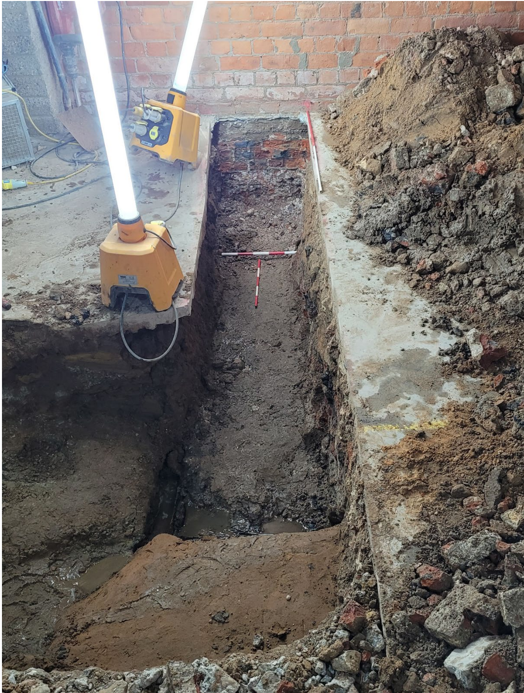
Plate 4: Trench 2 base looking south-west, scale unit 0.10m
