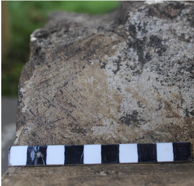
Plate 15: Masons marks on limestone block C1021 (AF1), Scale unit 0.01m
