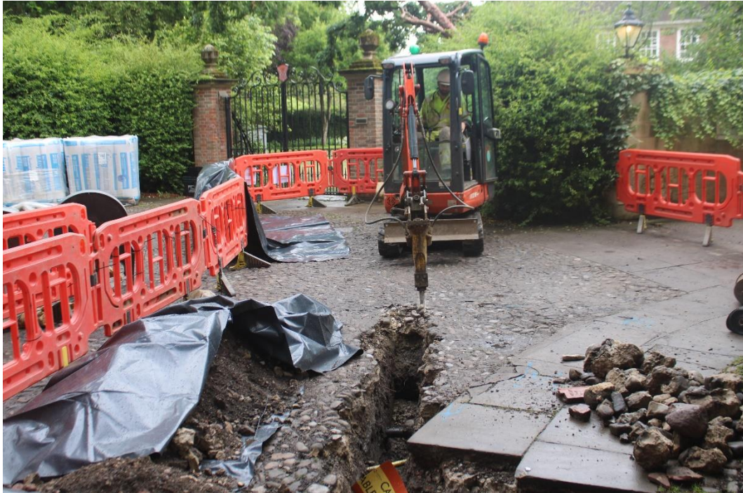
Plate 4: Removal of cobble yard surface C1001, looking north
