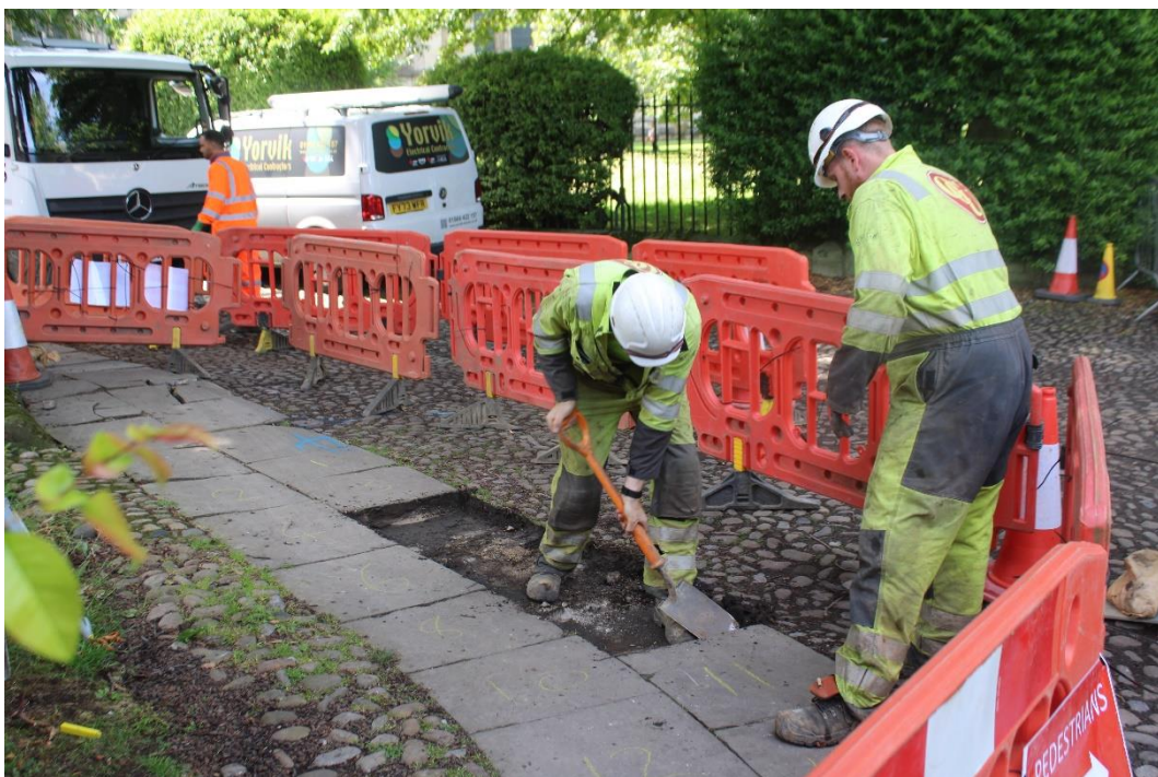
Plate 2: Removal of paving C1002, looking south-west
