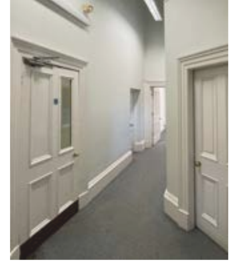
R105 Fire corridor created with modern partitions
