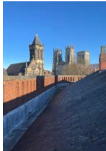
Parapet Roof facing Museum Street
