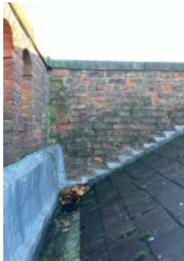
Parapet and associated lead work
