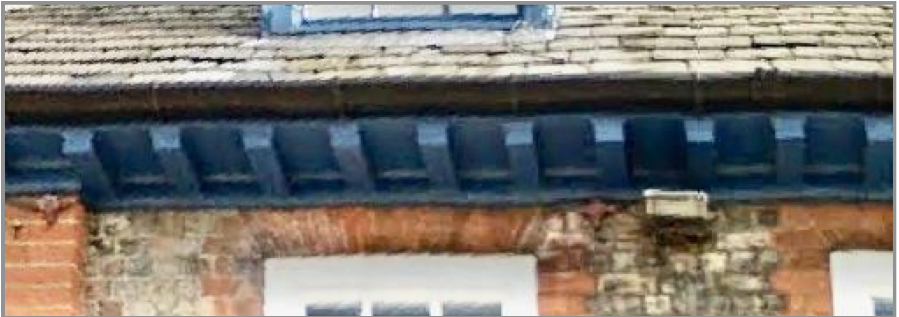
Figure 21. Detail of eaves showing soffit and modillions. Source: Google Streetview (2012, http://tinyurl.com/yewnx9mx ).
