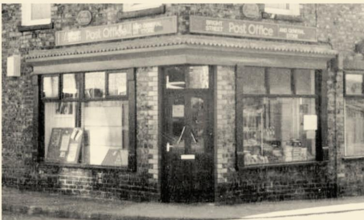
Figure 10. 'A social history of the local economy of a corner of York'. Source: Waddington (2021).
