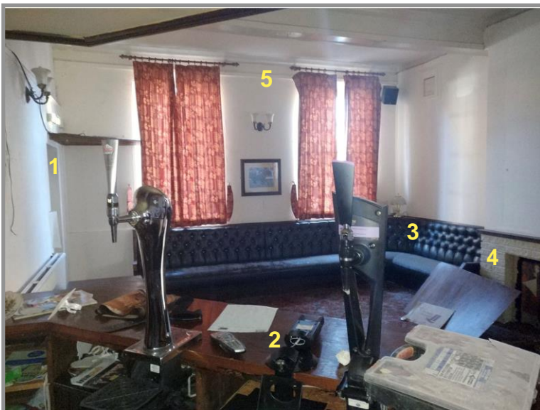
Figure 60. Northeast lounge leading off door to main entrance (1). A modern angular bar was fitted to this lounge (2). Fitted furnishing (3) and fire surround (4) appear to date from the mid to late 20th century. This otherwise plain room may originally have been decorated with wallpaper. Vestiges of picture rail are still present (5). The original fire-surround may have been similar to that still seen in the games room. See Figure 49 below. Source: Taylor (2023).
