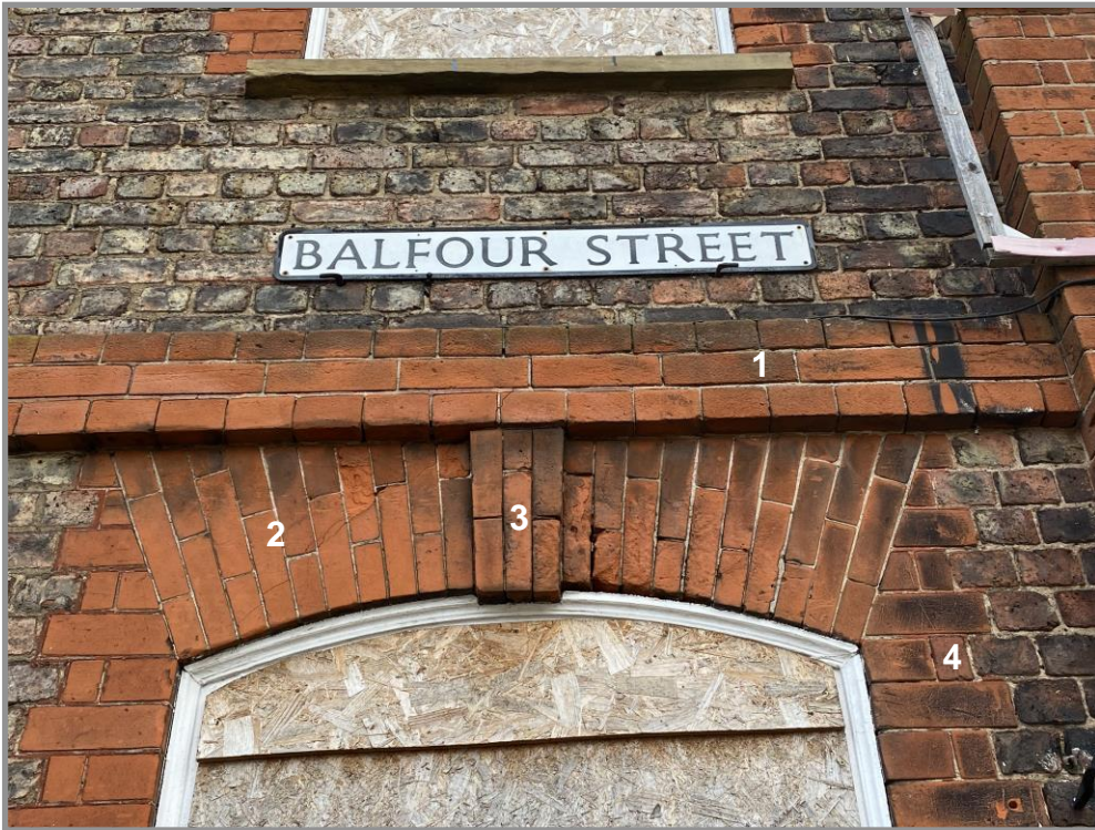
Figure 44. Ground floor window and string-course detail (1). The string-course brick set out on this elevation is the reverse of the Salisbury Terrace elevation. See Figure 30. Rubbed brick voussoirs (2) and (3) keys are carefully shaped to form a segmental arch. The arches spring from perfectly aligned red brick quoins, which have been formed by meticulously formed closers (4). The brickwork has high technical and aesthetic merit and is a defining element of the design.
