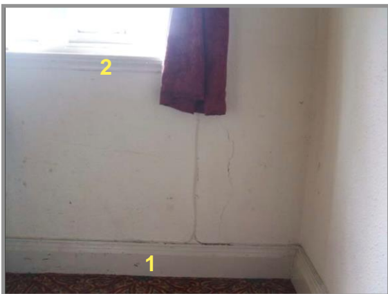
Figure 71. Throughout the property it appears that the deep and finely moulded skirtings are still present (1). Moulded window board details are seen throughout (2). Source: Taylor (2023).
