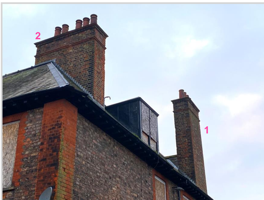
Figure 24. Left. Northwest chimney (1), set opposite the southwest chimney (2). The northeast chimney is set within the plan. Stacks are constructed in York common buff brick laid in English bond with red brick quoins. The brickwork set out is of a very high standard, with closers carefully positioned to form the distinctive quoin pattern.
