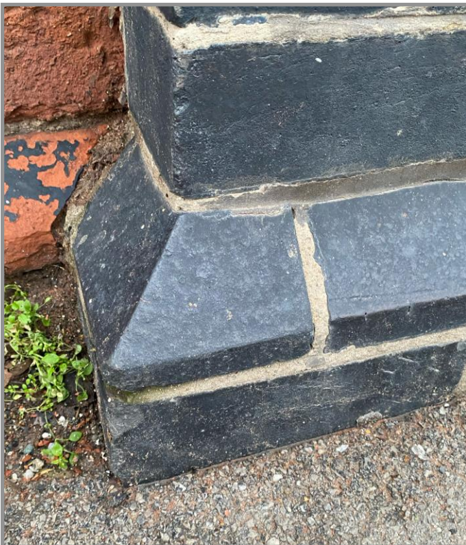
Figure 39. Detail of ground floor window brick quoin set-out. Lower brick work is in harder, black brick with this detail is followed through horizontally to the pilasters. See figure 18. Softer red bricks at ground floor level are heavily inscribed with graffiti.
