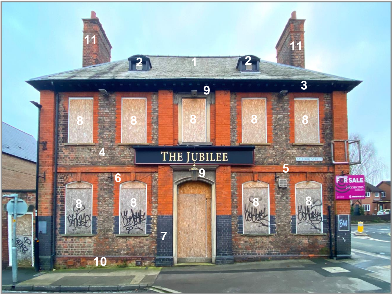
Figure 29. Balfour Street elevation, 2024. Cumberland slate with rolled lead hips (1). Lead-clad small vent dormers (2). Boarded eaves soffit with moulded modillions (3). York common brick in English bond (4). Terracotta brick sting-course with alternating English bond set-out on each façade (5). Rubbed brick voussoirs and keys (6). Black brick bases to giant order pilasters (7). 6-over-6 sash windows (8). Stuccoed central bay with main entrance and stucco window head at first floor (9). 1 Black bevelled brick plinth (10). Paired chimneys serving bar lounges and upper functions room (11).
