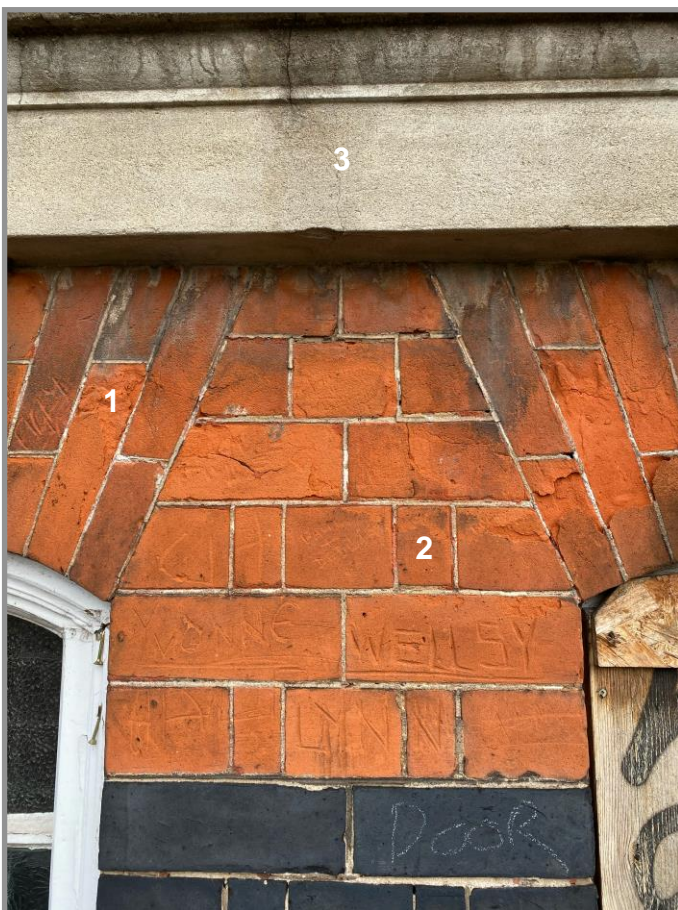
Figure 44. Ground floor window and string-course detail (1). The string-course brick set out on this elevation is the reverse of the Salisbury Terrace elevation. See Figure 30. Rubbed brick voussoirs (2) and (3) keys are carefully shaped to form a segmental arch. The arches spring from perfectly aligned red brick quoins, which have been formed by meticulously formed closers (4). The brickwork has high technical and aesthetic merit and is a defining element of the design.
