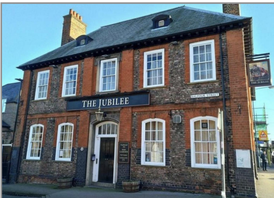
Figure 30. The Balfour Street elevation seen in its heyday and prior to boarding-up in 2016. Source: yorklocalist.org.uk (2024).
