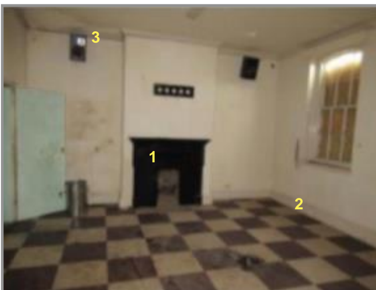
Figure 61. Games room to southeast with period fire surround and coal grate (1). Deep moulded skirting (2) appears to be intact, and the ceiling has a moulded cornice (3). Source: Taylor (2023).
