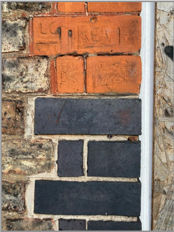
Figure 39. Detail of ground floor window brick quoin set-out. Lower brick work is in harder, black brick with this detail is followed through horizontally to the pilasters. See figure 18. Softer red bricks at ground floor level are heavily inscribed with graffiti.
