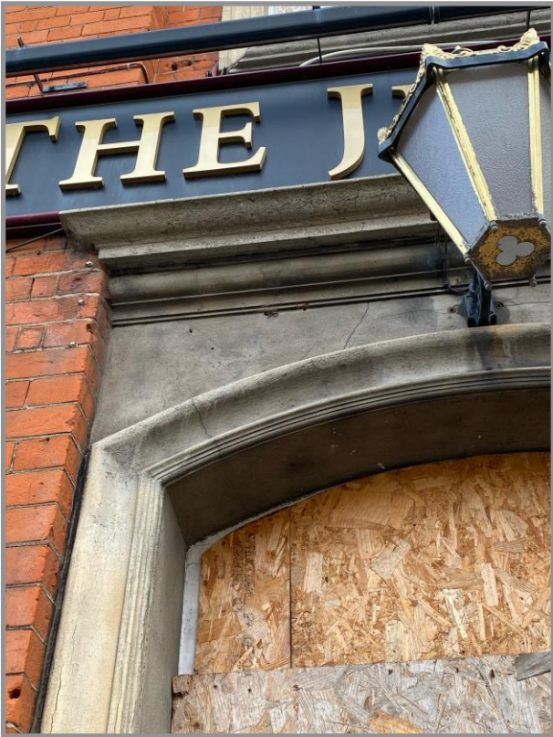
Figure 46. Detail of stucco work to the main entrance. The profiles and finishes are all very finely detailed and executed.
