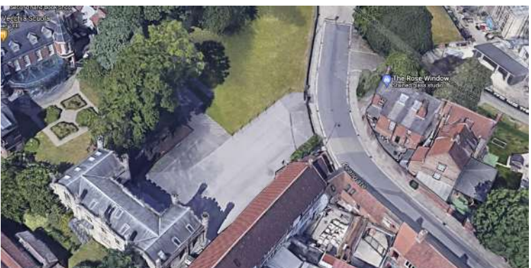
Relationship between No1 Deangate and the Refectory, looking west.
