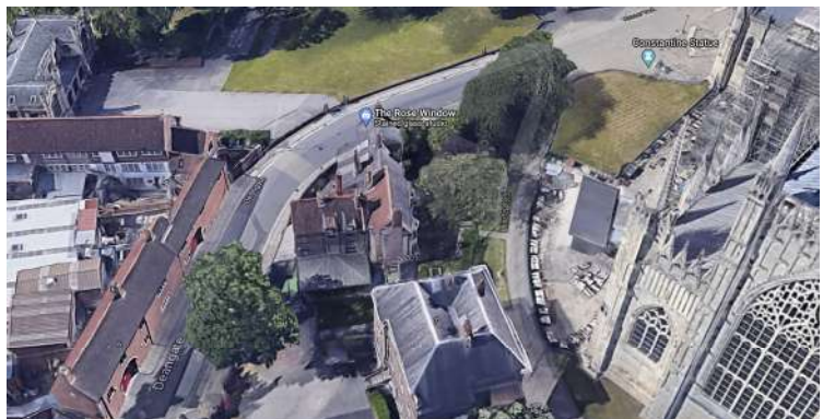
View of No1 Deangate from the east.
