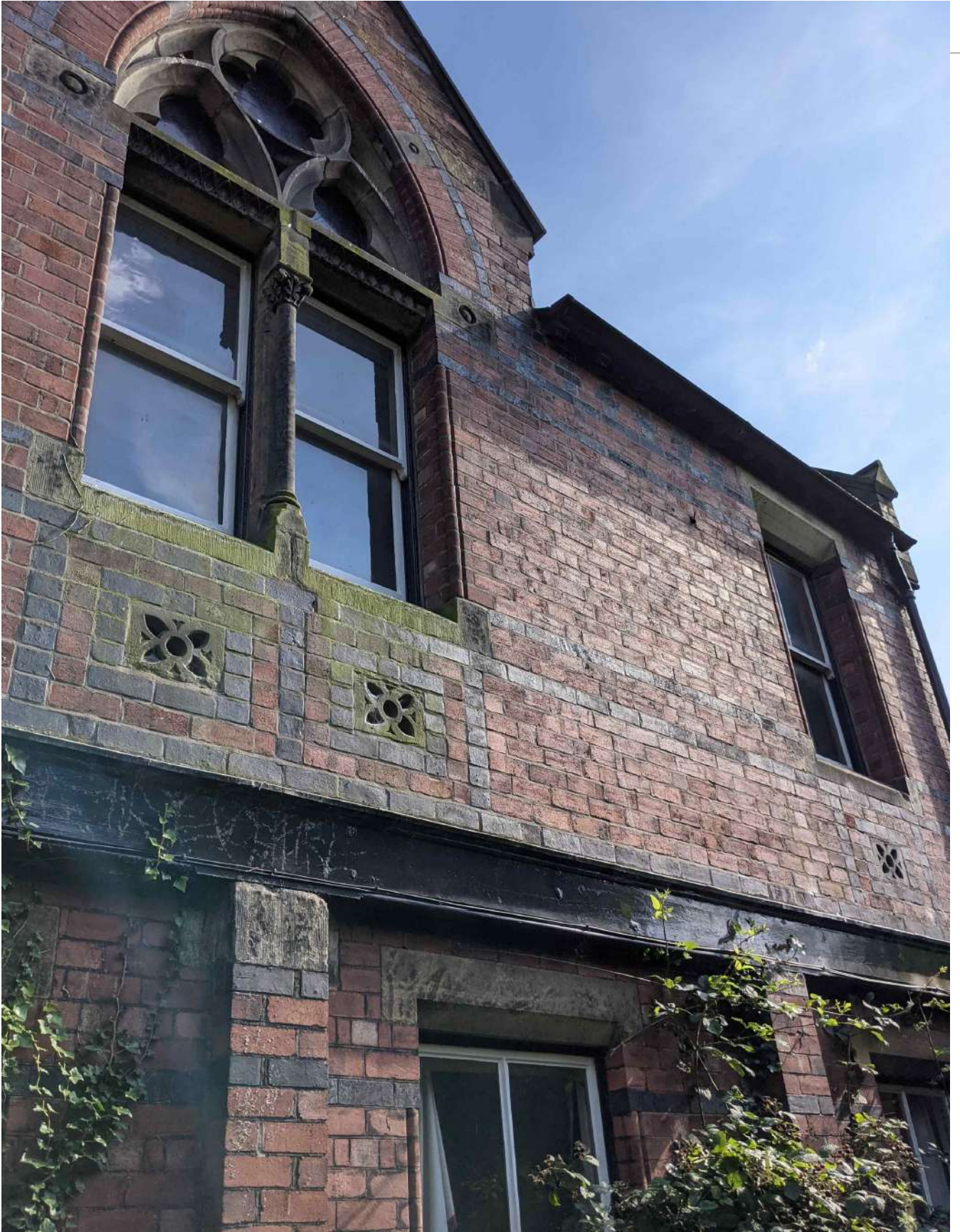
Figure 1: Northwest elevation of No. 1 Deangate.
