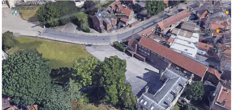
Relationship between No1 Deangate and the Refectory, looking north.
