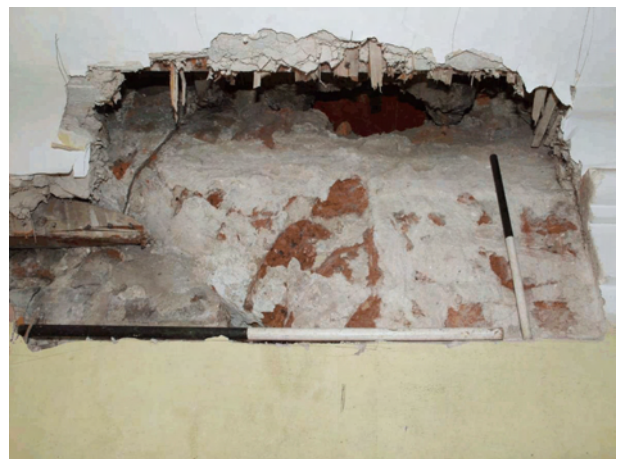
Plate 25 Intervention 5 - brick voussoirs of window head
