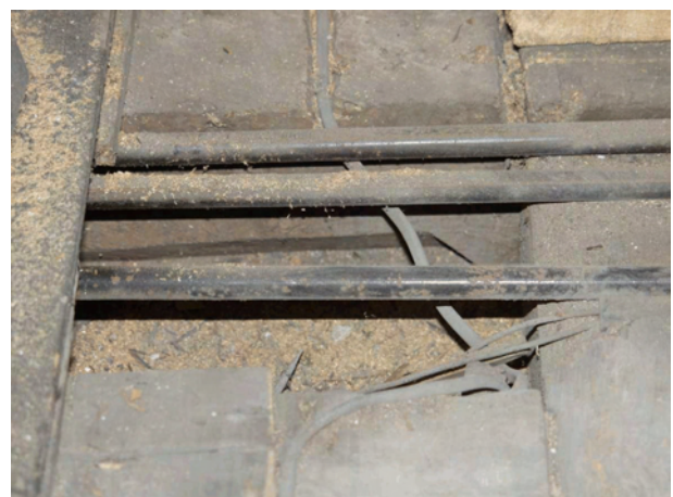
Plate 21 Intervention 5 - chamfer stop on joist
