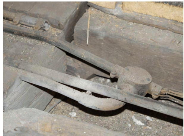
Plate 20 Intervention 5 - chamfer stop on joist
