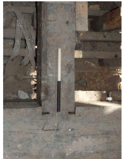
Plate 23 Intervention 5 - dovetail joint on reused joist
