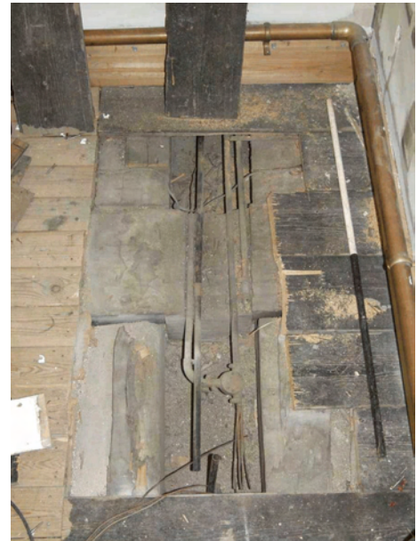
Plate 19 Intervention 5 - bridging beam and joists exposed at first floor level
