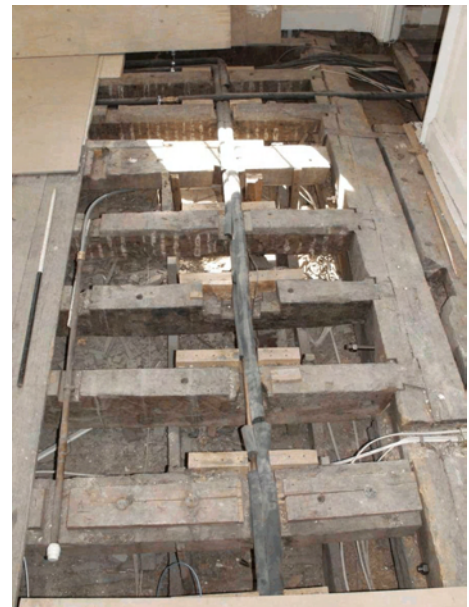
Plate 22 Intervention 5 - reused joists
