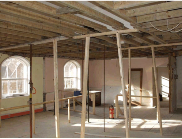
Plate 26 Intervention 5 - ceiling exposed in east range
