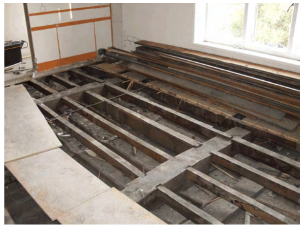
Plate 28 Intervention 5 - floor structure above chapel
