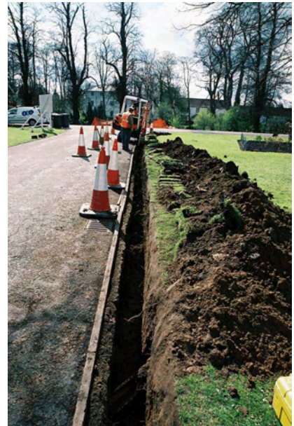
Plate 17 Intervention 4 - general shot, looking south
