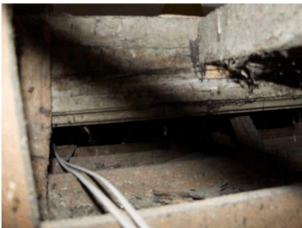
Plate 24 Intervention 5 - moulding on bridging beam
