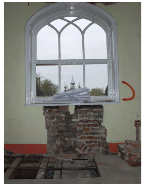
Plate 29 Intervention 5 - brick relieving arch above chapel windows
