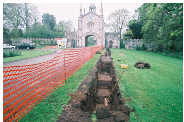
Plate 5 Intervention 2 - general shot, looking east
