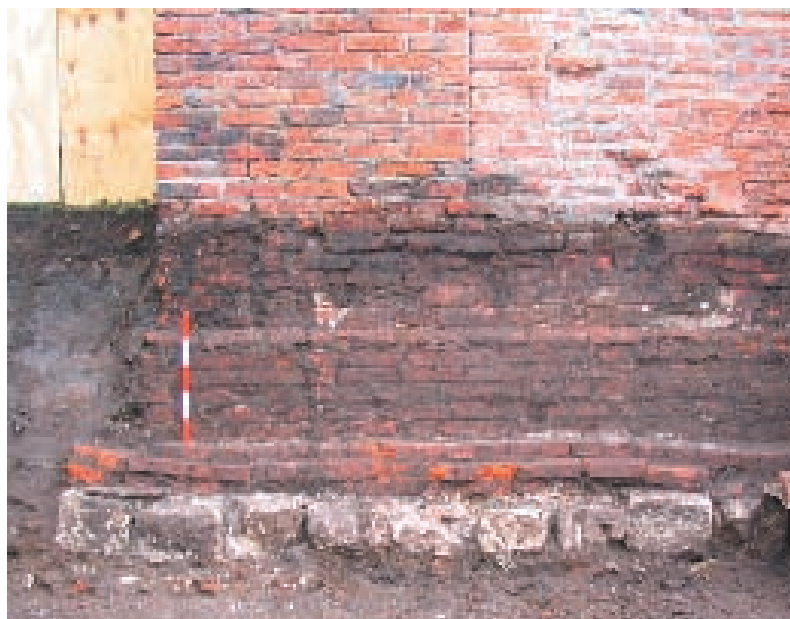
Plate 1 Exposed wall foundations, south-east facing section
