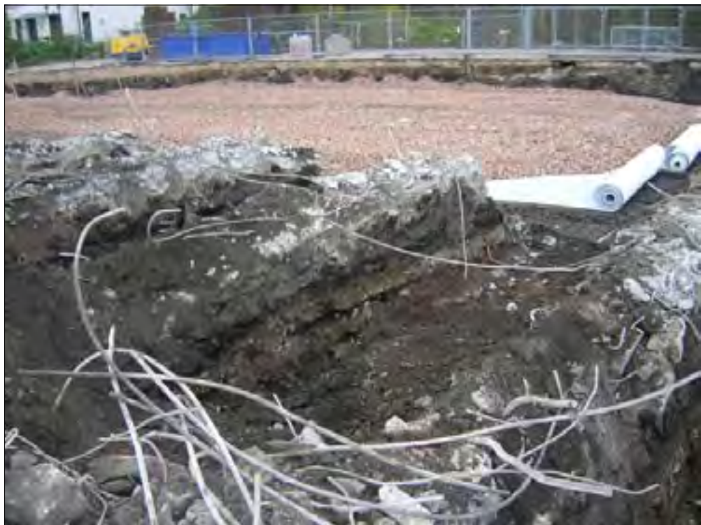
Plate 4 Levelling deposits and concrete raft, Block C, looking north-east
