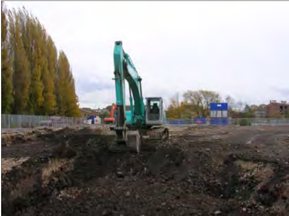
Plate 1 Initial site stripping, central Block A, looking south east
