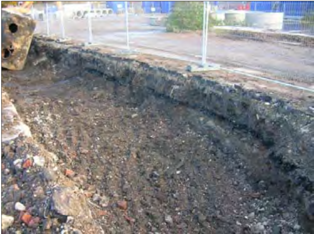
Plate 3 Levelling deposits, north-west end of Block C, looking south-east
