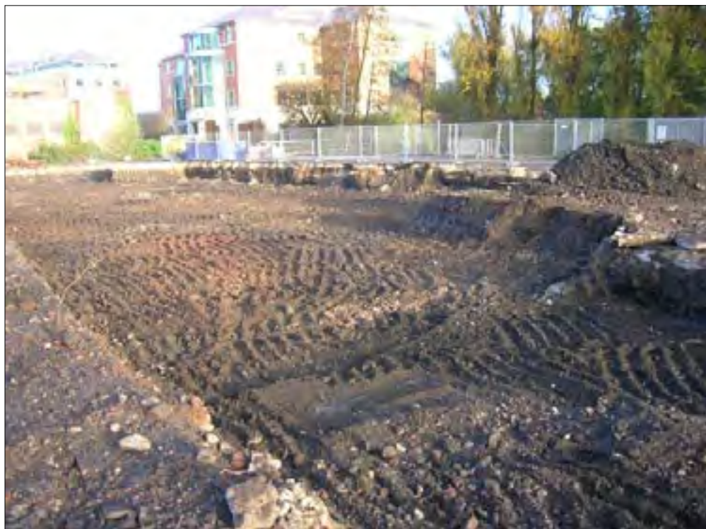
Plate 2 Initial site stripping, Block A, looking north
