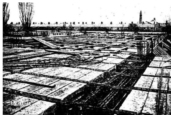
The Dining Block under construction showing the hollow block floor
