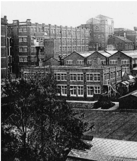
The rear of the Almond Block with the Cream Room extension completed in 1915 in the foreground
