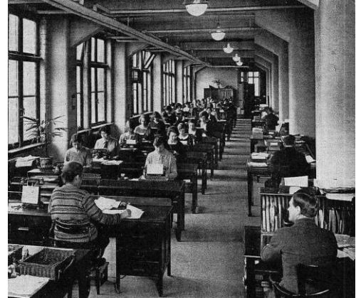
The 1914 Office Block designed by W J Swain and built by the Rowntree building department using Swain's patented cross brace or Lattice Truss system.
