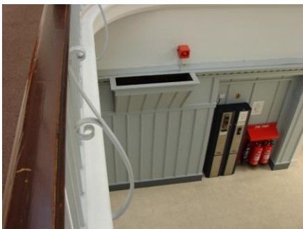
The General Office building constructed in 1896 originally providing accommodation for the directors. The building ventilation system provides ducted air from outside to a series of termination at ground floor level within the panelling.
