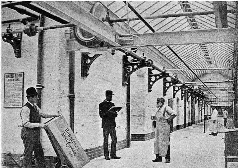
The main corridor 1893 with patent glazed rooflights
