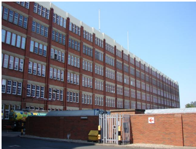
The east elevation of the Cream Block and extension facing Haxby Road. A later dated single storey amenity block has been built in the position of the original entrance
