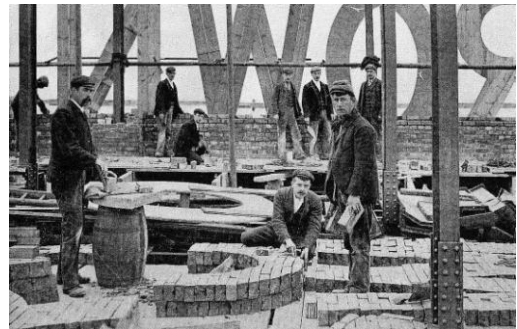
The Elect Block completed in 1903 to designs by Fred Rowntree. The tank at the top of the tower serves a sprinkler system for fire protection. The steel frame can be clearly seen as brickwork external walls are constructed.
