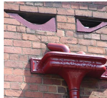
The General Office building constructed in 1896 originally providing accommodation for the directors. The building ventilation system provides ducted air from outside to a series of termination at ground floor level within the panelling.
