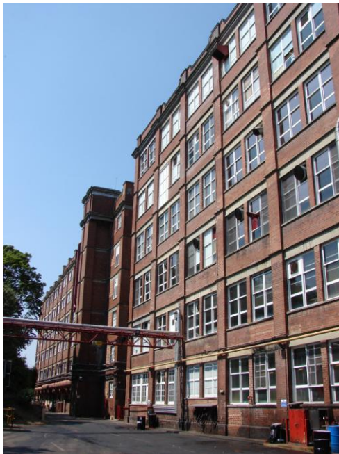
Built in 1907 using a patented, licensed reinforced concrete frame by the Yorkshire Hennibique Contracting Co Ltd. The extension was built in 1911 using Swain's patented reinforced concrete frame design.
