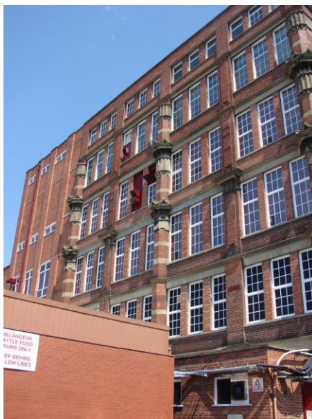
Built in 1906 using a patented, licensed reinforced concrete frame by the Yorkshire Hennibique Contracting Co Ltd. A sixth floor was added in 1962
