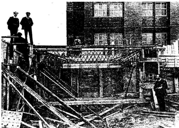
The construction of the lattice truss before covering with concrete
