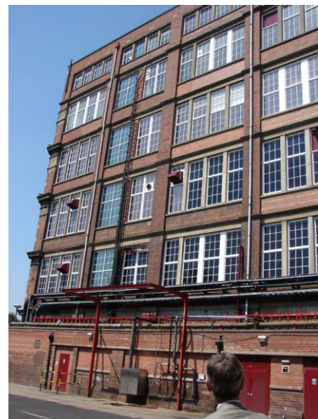
The ground floor of the block is dedicated to servicing with an abundance of pipework evident
