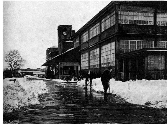
The Card Box Mill, one of the last reinforced concrete buildings to be erected on site. The building was well lit with patent glazed north lights and large expanses of windows. The numbers of staff employed in the Card Box Mill were more than employees on the Cocoa Works site in 1892.
