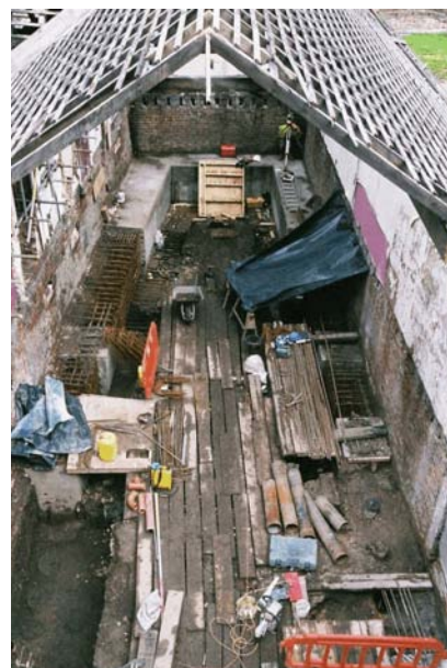
Plate 6 General view of site at the closing stages of excavation
