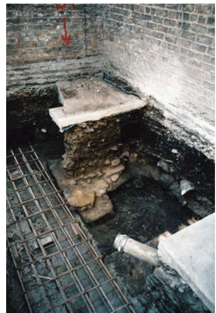
Plate 10 Portion of wall foundation F36 pre-excavation (scale 0.5m)
