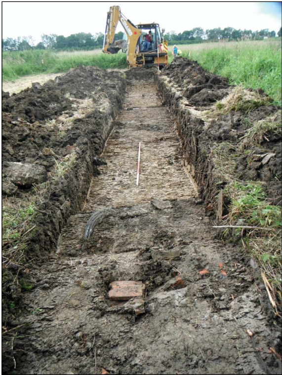
Plate 1. Trench 1 looking south-west, with area of cables in foreground
