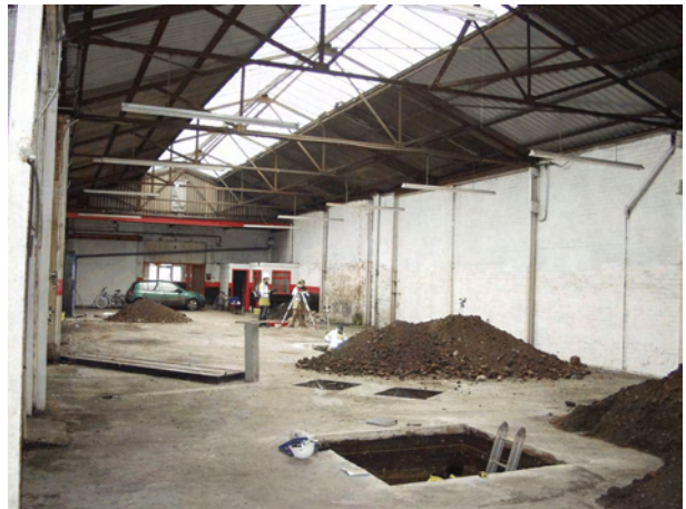
Plate 22 Internal view of the central shed looking south
