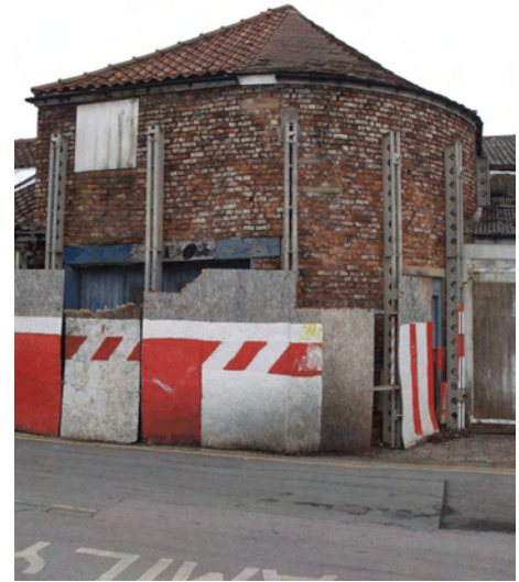
Plate 20 Southeast elevation of Structure 3
