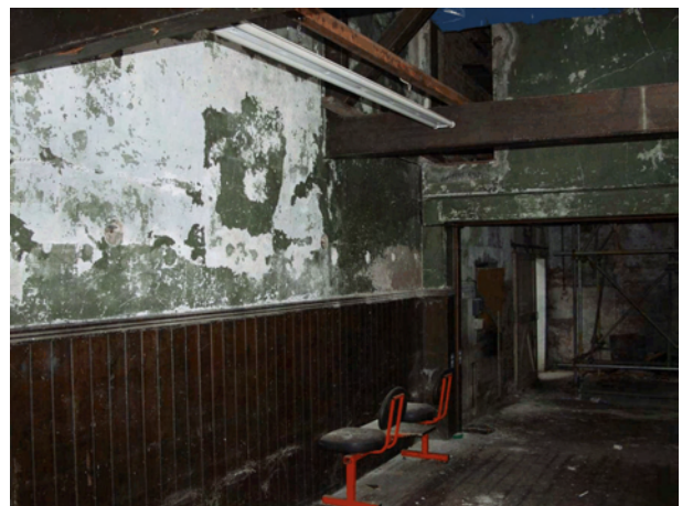
Plate 28 Internal view of the ground-floor room of Structure 2
