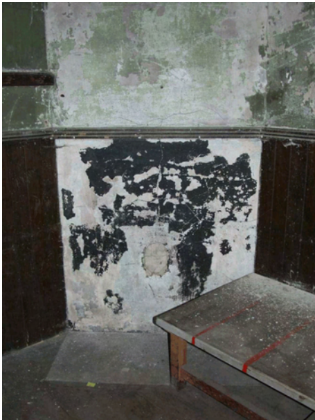
Plate 30 Corner chimney stack with blocked flue
