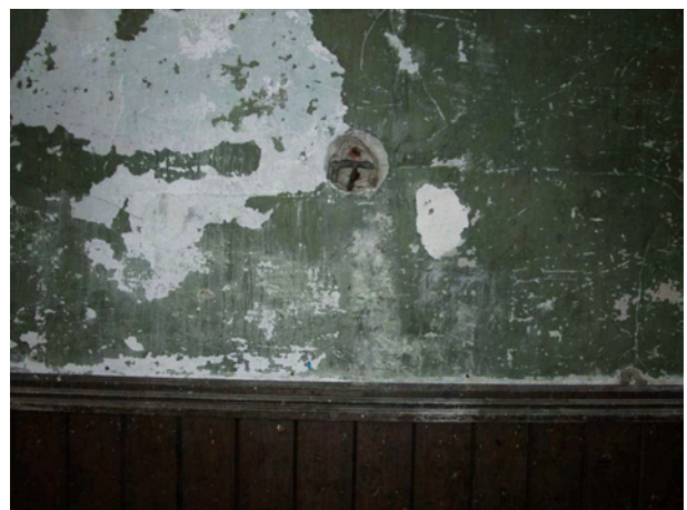
Plate 29 Position of former gas light fitting
