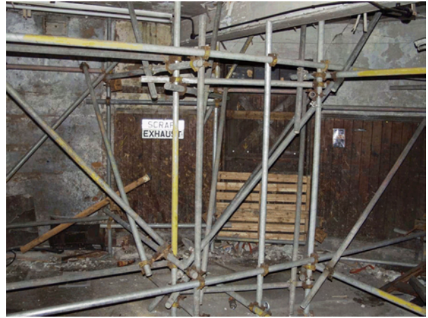
Plate 27 Incomplete panelling in the ground-floor room of Structure 3
