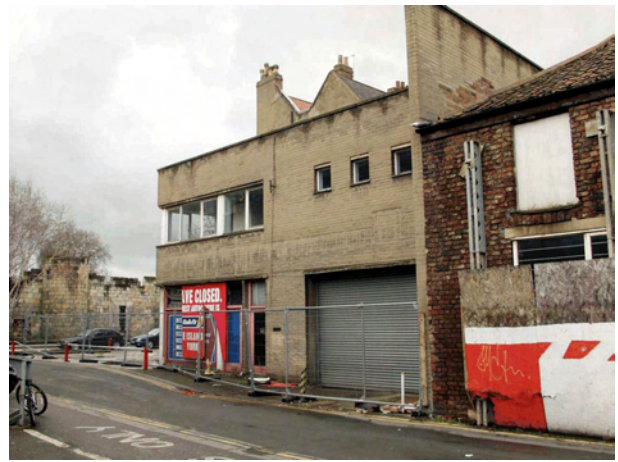
Plate 17 Southeast elevation of the reception building
