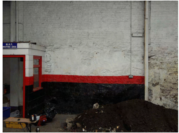
Plate 23 Area of earlier walling and plastered surfaces in the northwest elevation of the central shed
