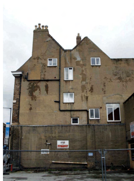
Plate 15 Southeast elevation of No. 33 Bootham
