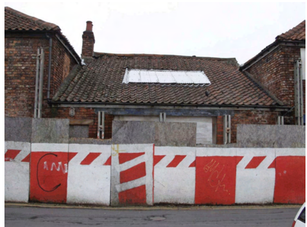
Plate 19 Southeast elevation of Structure 2
