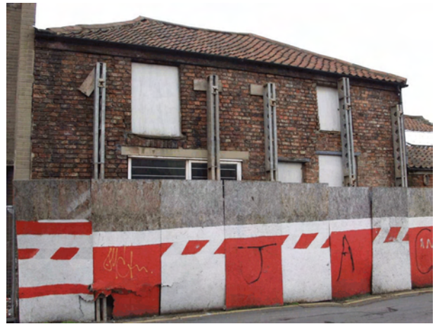
Plate 18 Southeast elevation of Structure 1
