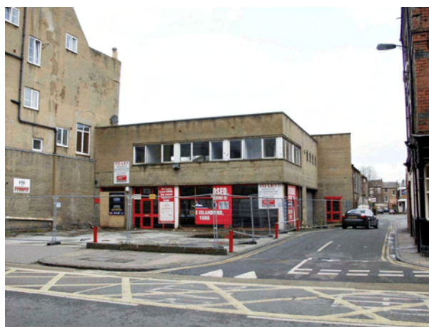
Plate 14 Southwest elevation and forecourt
