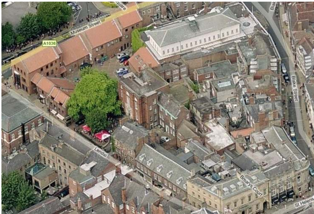
Aerial view from the south - Judges Lodgings in centre Fig 2
