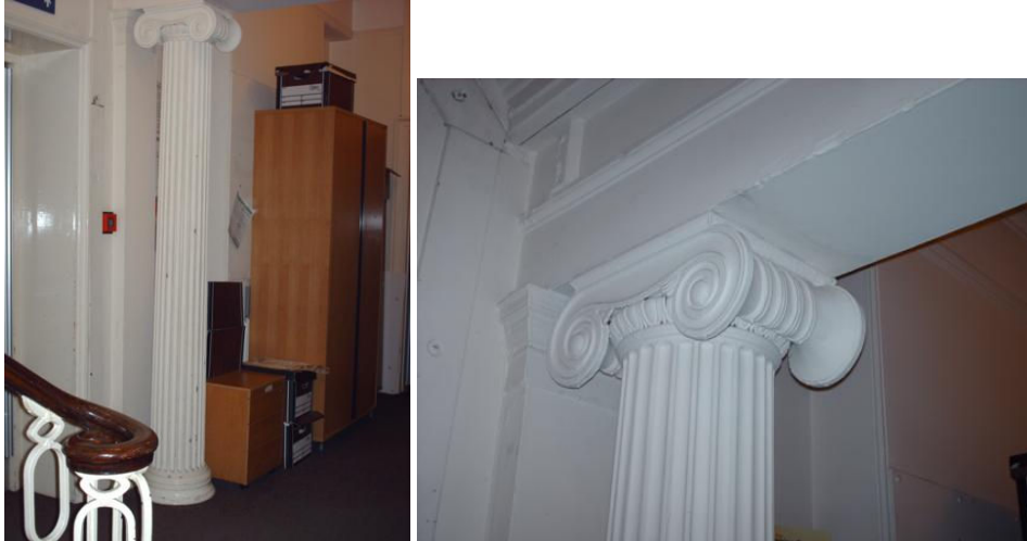
Figure*39 – Ground floor hallway, No.8 St Leonard's Place (icosse, March 2008)
