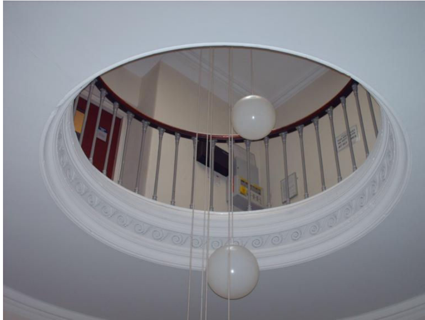
Figure*48 – Principal stairwell, 4 Museum Street (icosse, March 2008)
