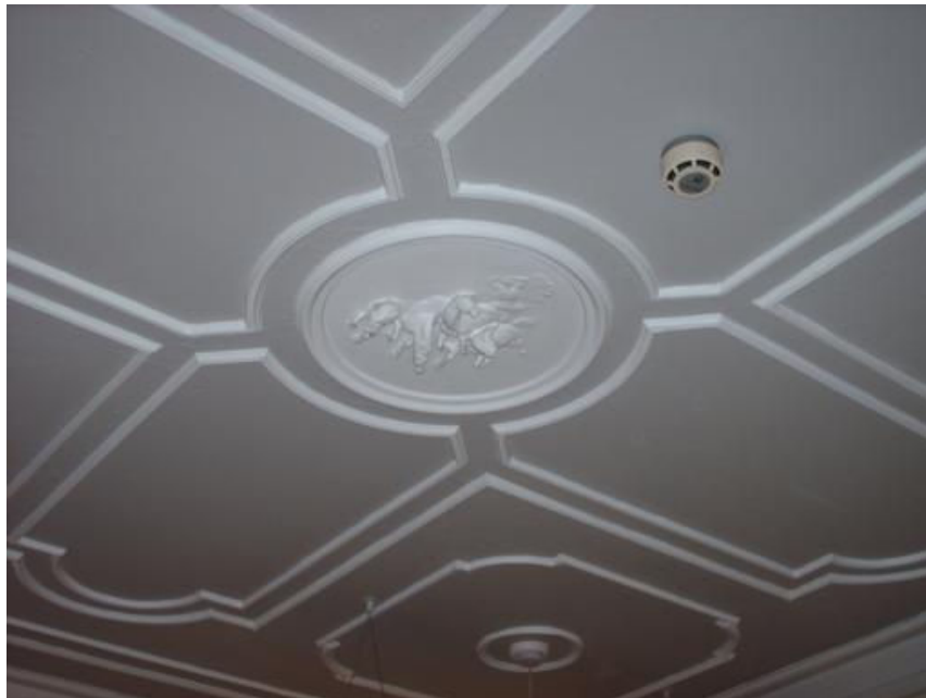
Figure*31 – Decorative roof panel, No.6 St Leonard’s Place (icosse, March 2008)
