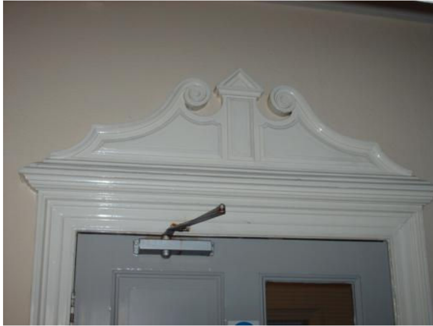
Figure*40 – First floor doorcase, No.4 St Leonard’s Place (icosse, March 2008)
