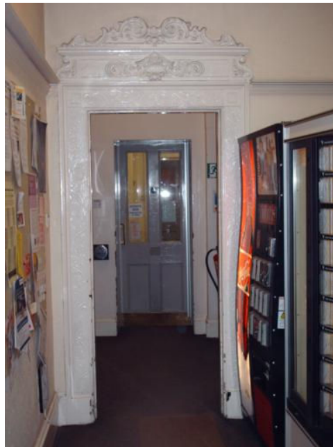
Figure*40 – First floor doorcase, No.6 St Leonard's Place (icosse, March 2008)
