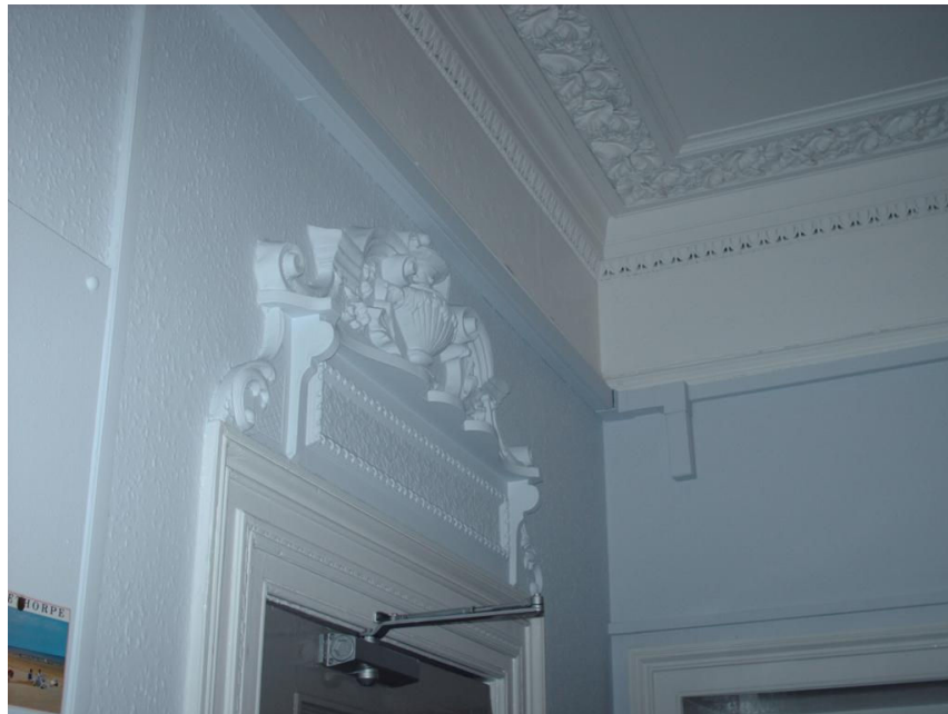
Figure*41 – First floor doorcase, No.7 St Leonard’s Place (icosse, March 2008)
