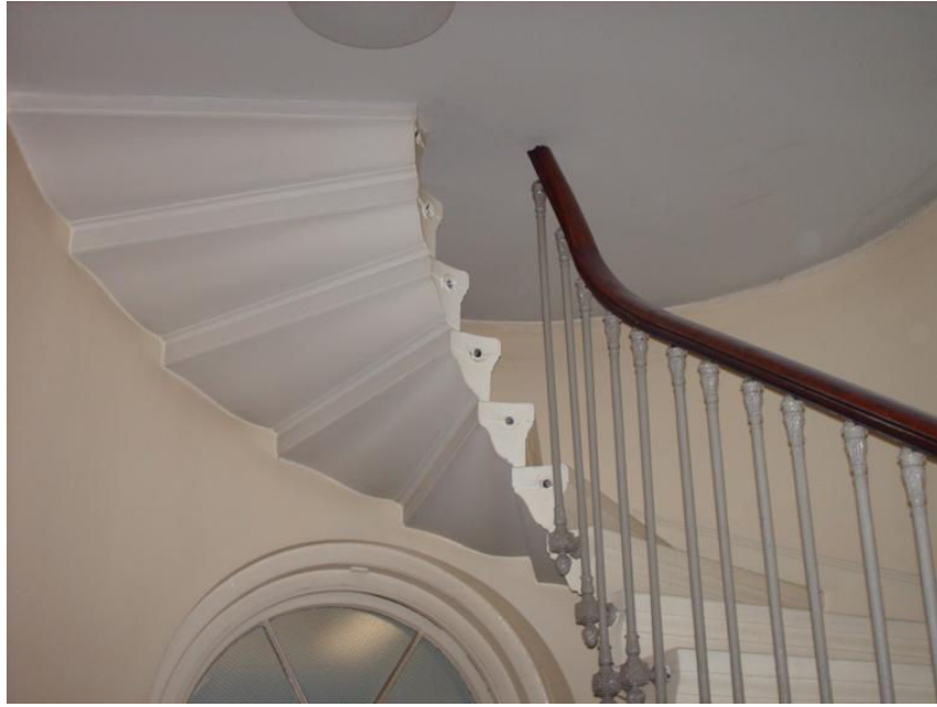
Figure*47 – Staircase, 2 Museum Street (icosse, March 2008)
