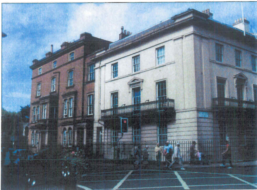
Plate 3 The Museum Street frontage, looking west
