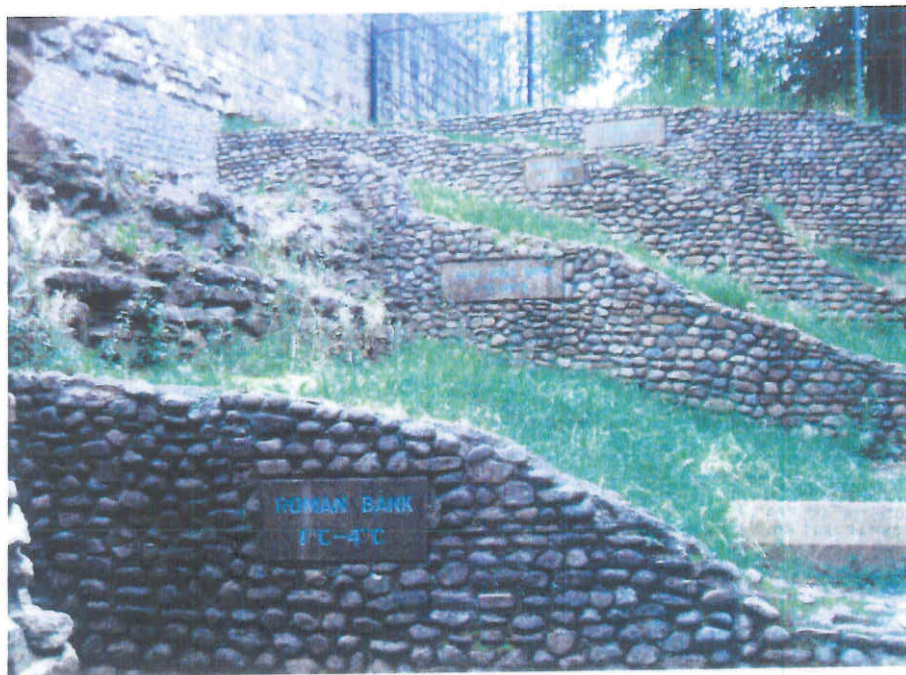
Plate 9 The exposed ramparts south-west of St. Leonard's Place, looking north-east
